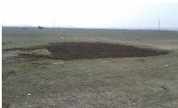
Photo 5. Excavation area after backfilling.
