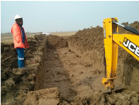
Photo 1. Trial excavation using machinery.
