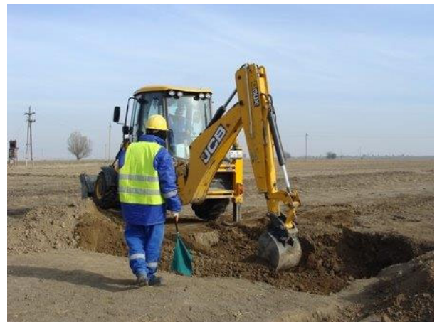
Photo 2. Trial excavation process using machinery.
