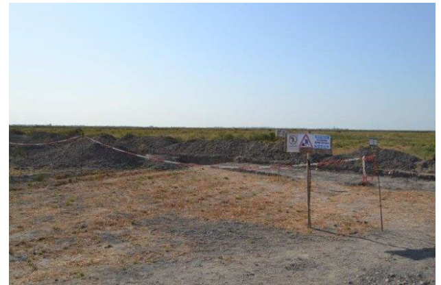
Photo 4. Signs and fencing near excavation.
