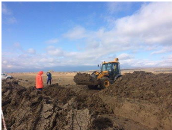
Photo 3. Excavation trench backfill.
