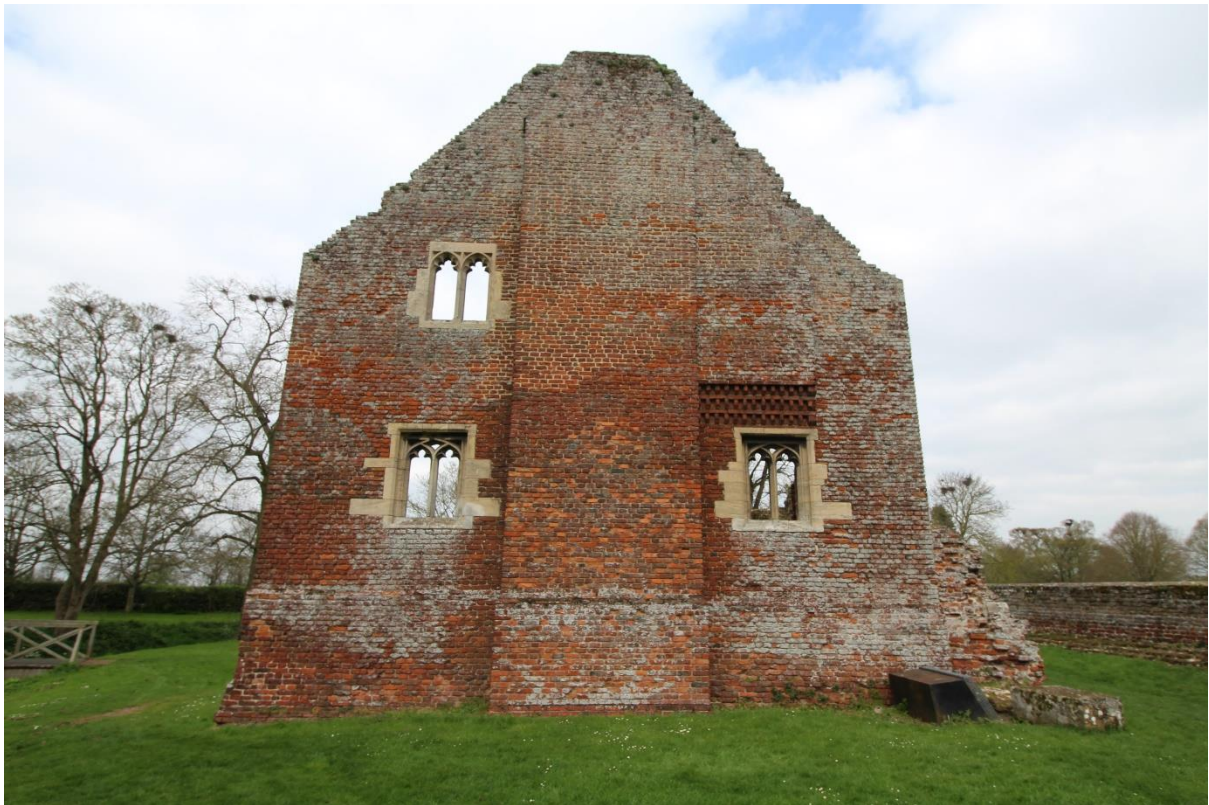
Figure 24 South elevation of the south range, looking north
