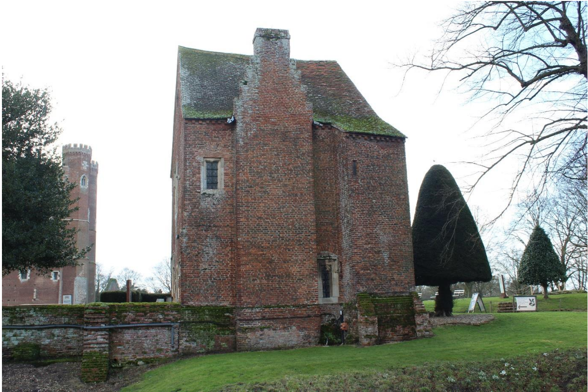
Figure 36 East elevation of the Middle Ward lodging, looking west. Note the projecting latrine block to the right
