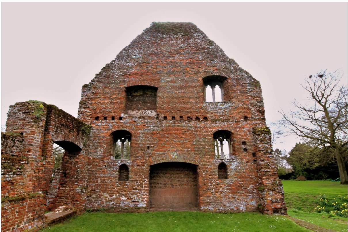
Figure 25 South elevation of the south range, looking south
