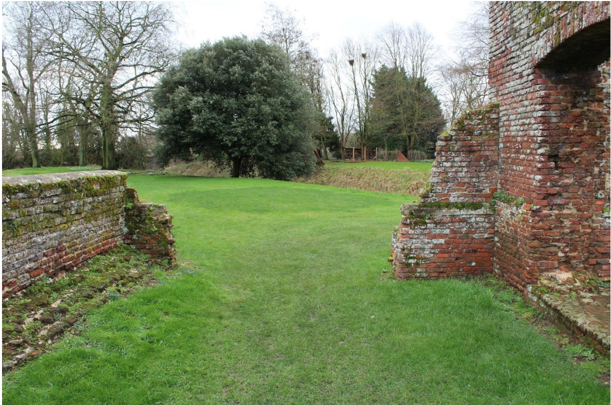
Figure 30 Possible gateway between the building (right) and Inner Moat wall (left), looking south
