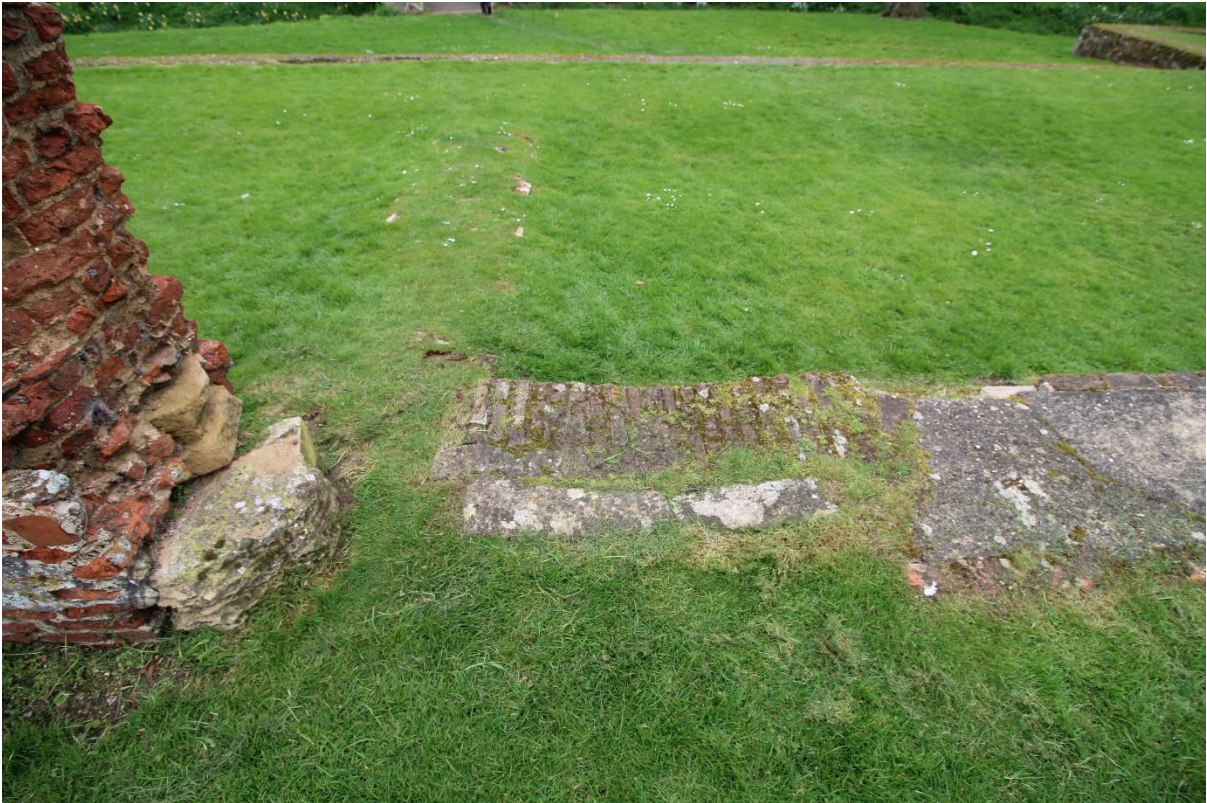
Figure 34 Threshold to the north of the surviving east elevation wall, looking west. Note the partially buried stone foundation of the transverse wall
