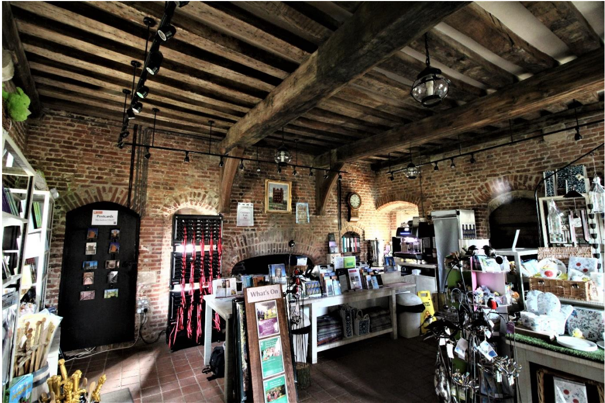
Figure 32 Ground floor of the Middle Ward lodging, looking south-east. Note the posts and knee braces supporting the bridging beams
