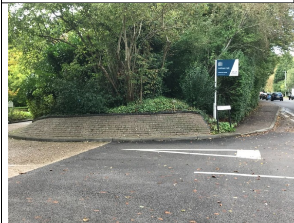
Plate 12: Bank visible behind Modern embankment wall
