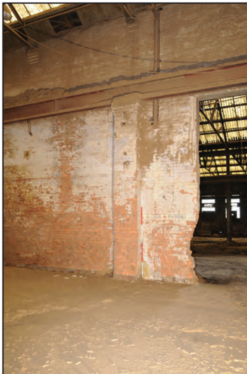
Photograph No. Washwood172 Description: Brick pilaster on north elevation with entry into A2 Site Location: A3 Direction From: SE
