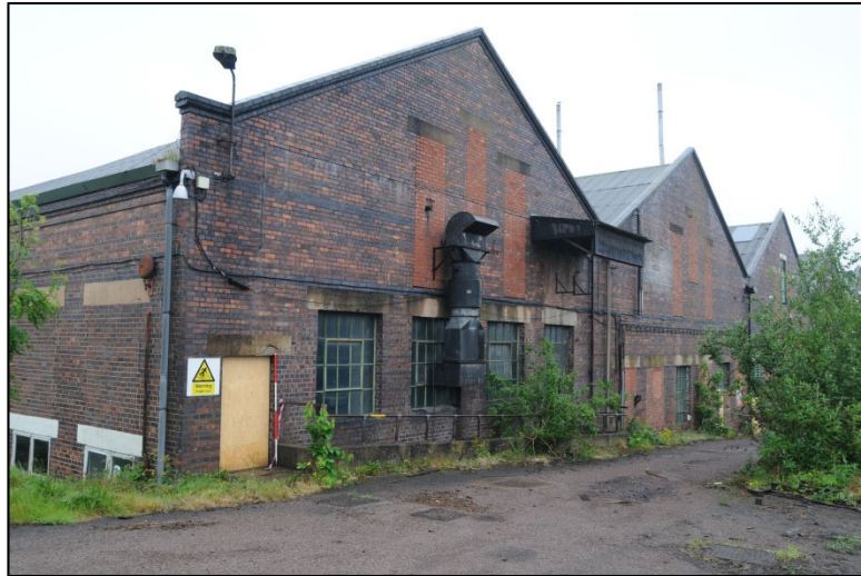
Plate 7: Window openings at the western end of A6
