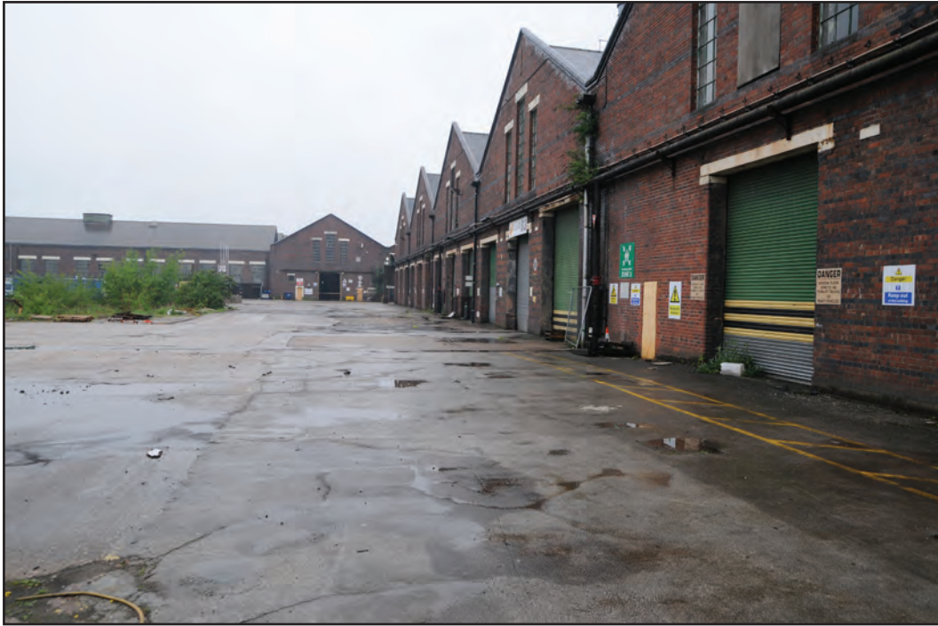
Photograph No. Washwood221 Description: General view of relationship between Buildings B, E and F Site Location: B/E/F Direction From: S
