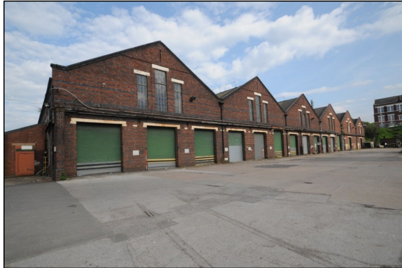
Plate 8: Western gable end of Block B
