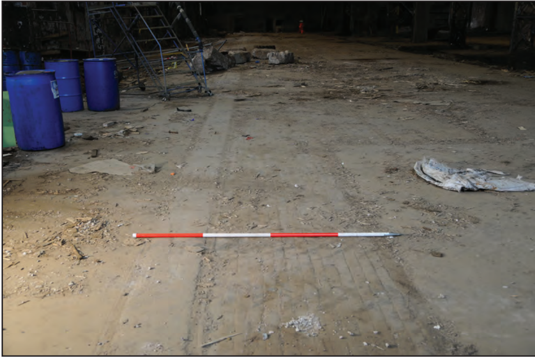
Photograph No. Washwood179 Description: Concrete cast floor with brick infill at west end of shed interior Site Location: A1 Direction From: W
