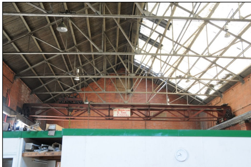
Plate 4: Travelling crane over the former Engine House C6c
