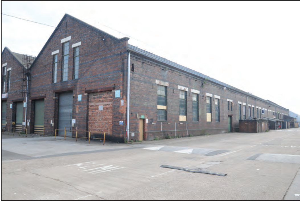
Photograph No. Washwood161 Description: east end of exterior north elevation and exterior east gable end Site Location: B1 Direction From: NE
