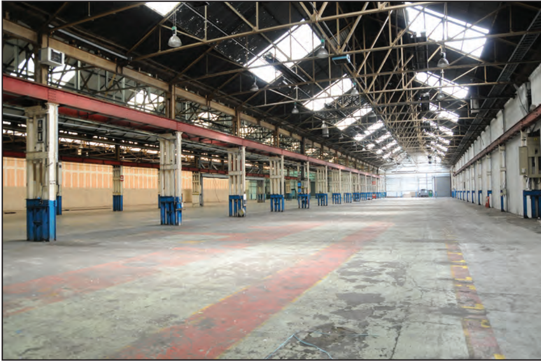
Photograph No. Washwood035 Description: View across shed interiors. Taken from within C3 Site Location: C1-C3 Direction From: SW
