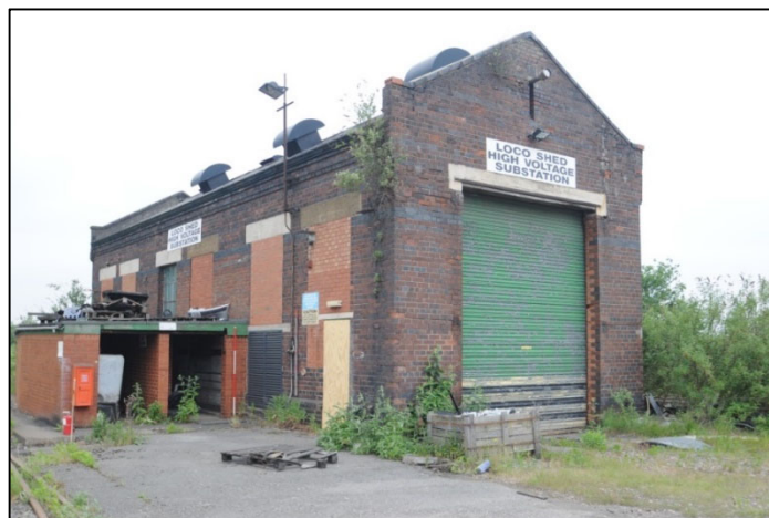
Plate 10: Loco shed at the north-west end of the site
