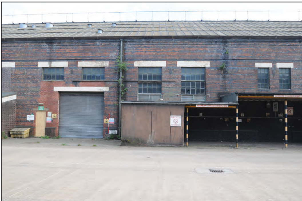
Photograph No. Washwood158 Description: Exterior north elevation with varying windows and inserted openings Site Location: B1 Direction From: N
