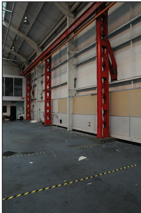
Photograph No. Washwood216 Description: Combination of original and modern stanchions on south wall Site Location: H2 Direction From: WNW
