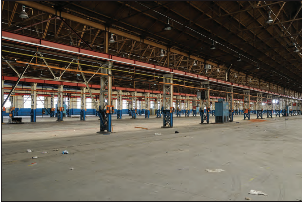
Photograph No. Washwood083 Description: View across sheds interior Site Location: F2-F5 Direction From: NE
