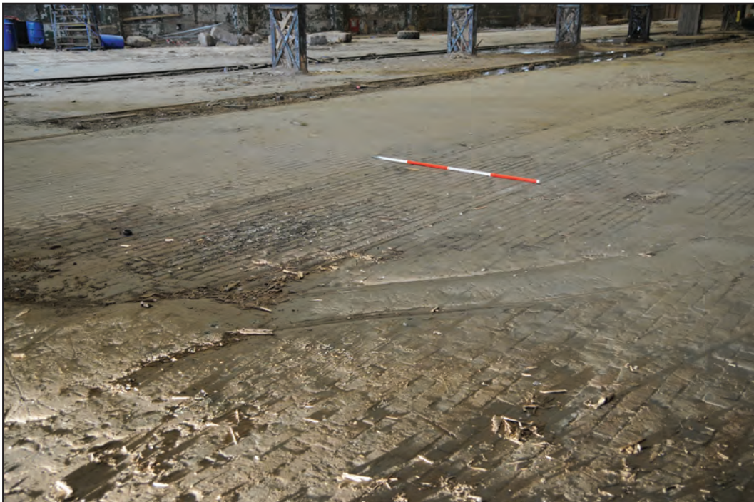
Photograph No. Washwood176 Description: Brick floor with train and cart rails at west end of shed interior Site Location: A2 Direction From: SW
