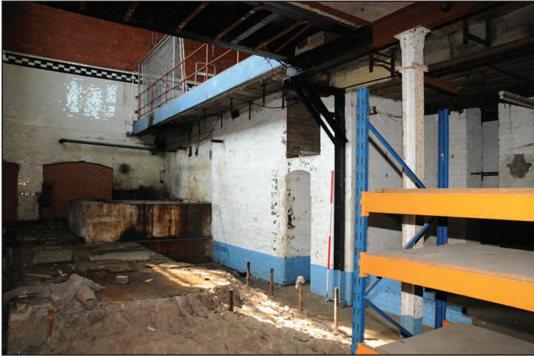
Photograph No. Washwood061 Description: Steam engine footings Site Location: C6d Direction From: SE
