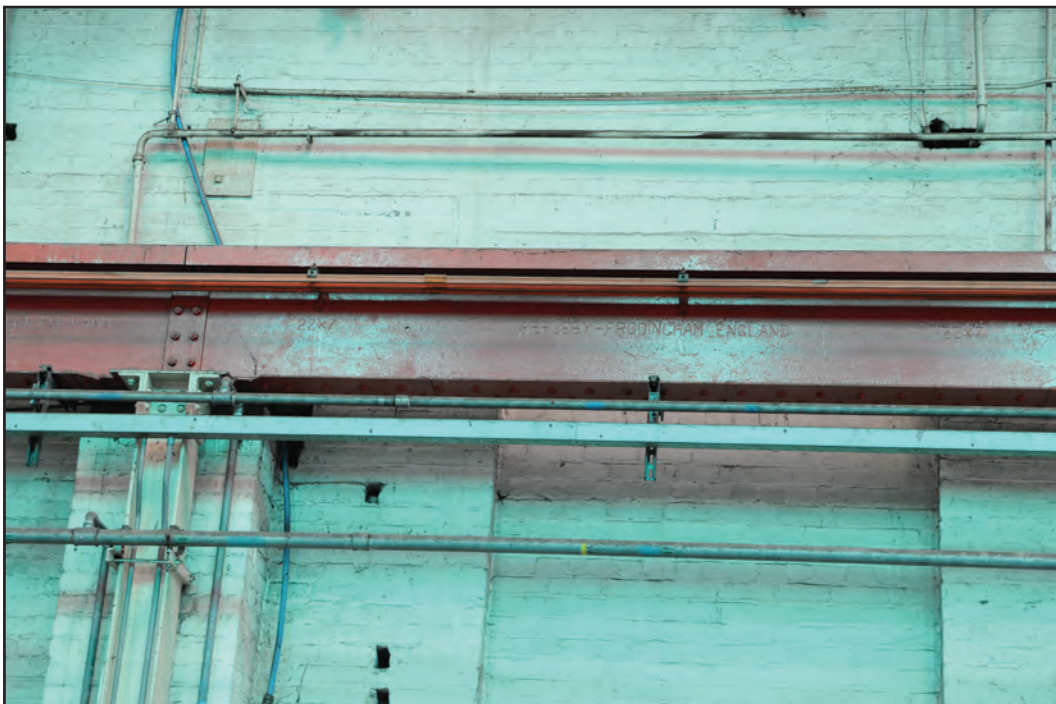
Photograph No. Washwood030 Description: APPLEBY-FRODINGHAM ENGLAND 22 X 7 foundry mark on north side rail at west end of shed Site Location: G3 Direction From: S
