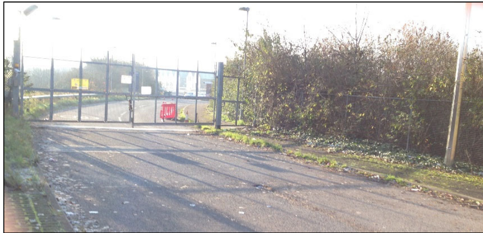
Plate 12: View showing the entrance gate to the site on the north side of the complex
