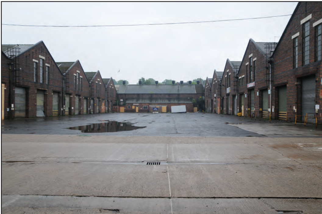
Photograph No. Washwood226 Description: Relationship between Buildings A and B Site Location: A/B Direction From: N
