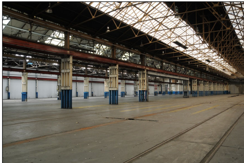
Plate 3: Showing the interior of Block C
