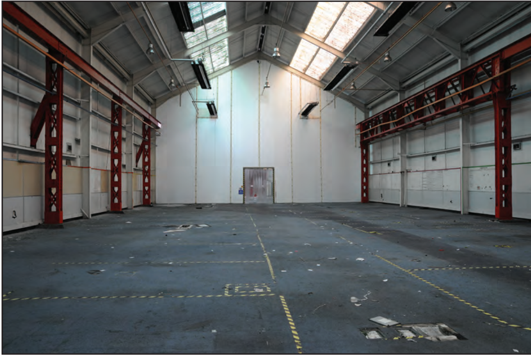
Photograph No. Washwood211 Description: Large shed area interior Site Location: H2 Direction From: E
