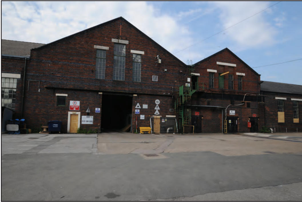
Photograph No. Washwood153 Description: Exterior south gable ends Site Location: E1/E2 Direction From: SSW
