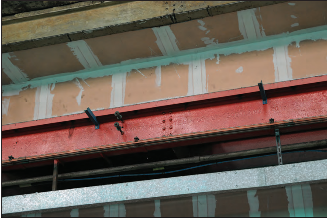
Photograph No. Washwood027 Description: LANARKSHIRE STEEL CO LD SCOTLAND 20 X 7 1/2 Foundry mark on steel rail on south side of shed Site Location: G4 Direction From: NNW
