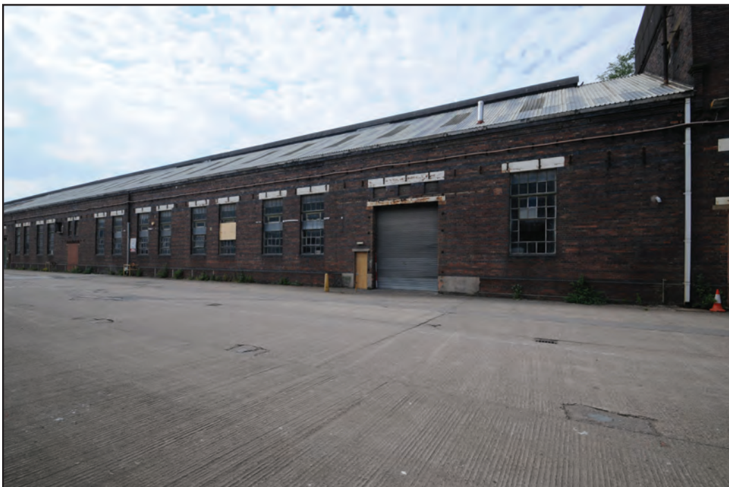
Photograph No. Washwood148 Description: Exterior south elevation, east end Site Location: C5 Direction From: SSE
