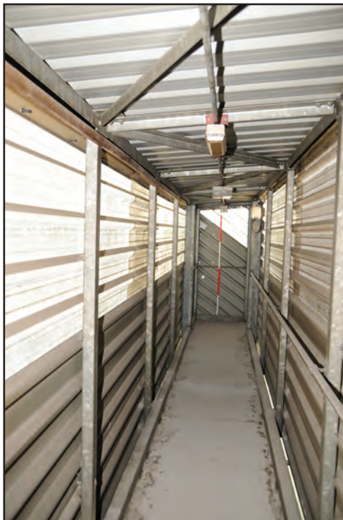
Photograph No. Washwood018 Description: Bridge on 1st floor to gain access from external staircase on north Site Location: G7 Direction From: S
