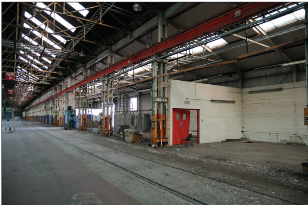
Photograph No. Washwood004 Description: Shed interiors with detail of breeze block internal division in G2 Site Location: G2/G3 Direction From: SE
