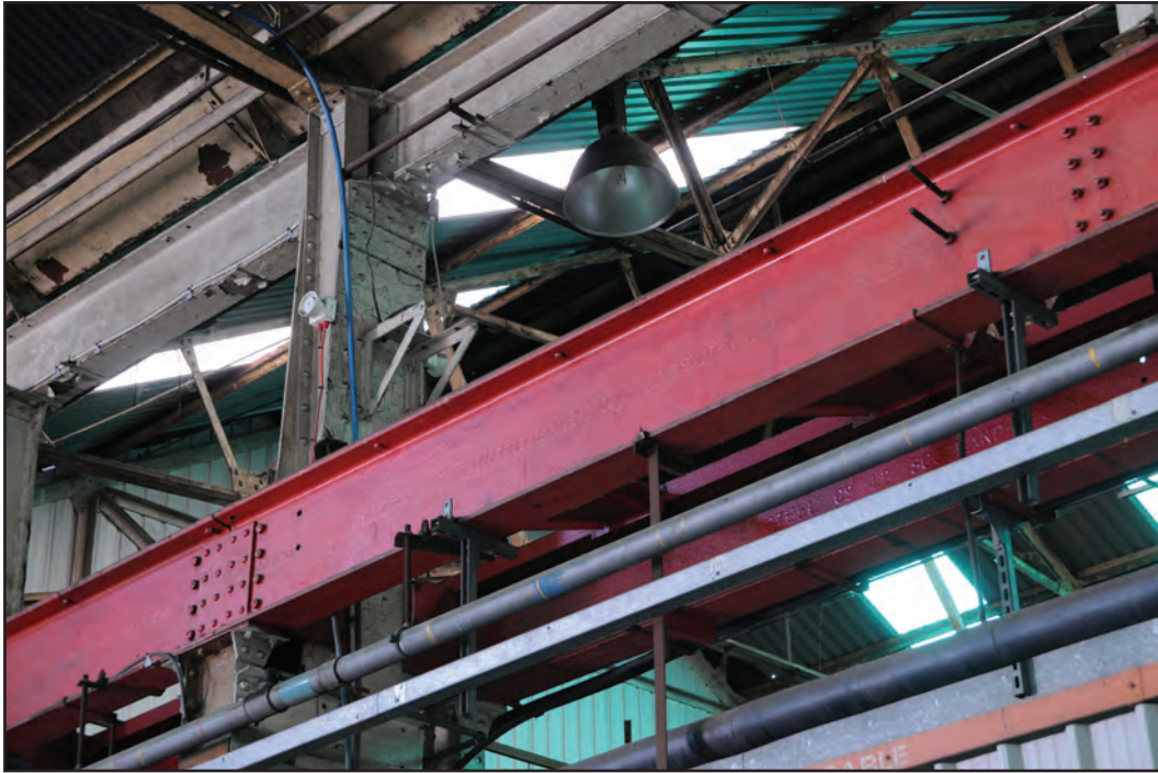
Photograph No. Washwood029 Description: DORMAN LONG & CO LD MIDDLESBROUGH 22 X 7 foundry mark on south side rail at E end of shed Site Location: G3 Direction From: NW
