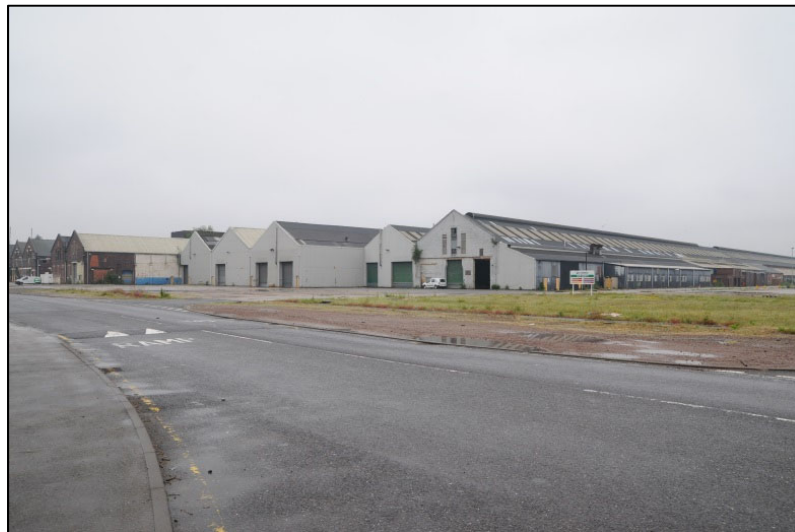
Plate 1 View from the current entrance to the north-east with Block G in the foreground
