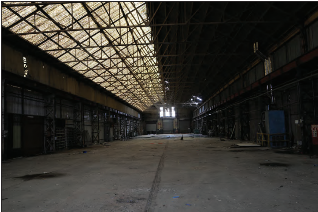
Photograph No. Washwood204 Description: Shed interior Site Location: B3 Direction From: W
