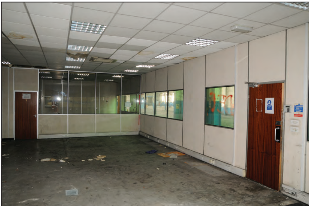
Photograph No. Washwood078 Description: General view of office space interior showing internal glass divisions Site Location: E1/E2 Direction From: NW
