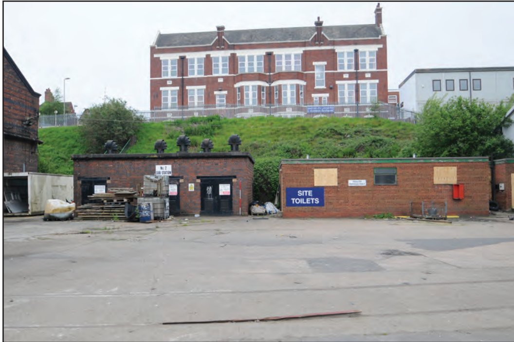
Photograph No. Washwood125 Description: Exterior north elevation and modified brick building to the west Site Location: No. 2 sub-station Direction From: N
