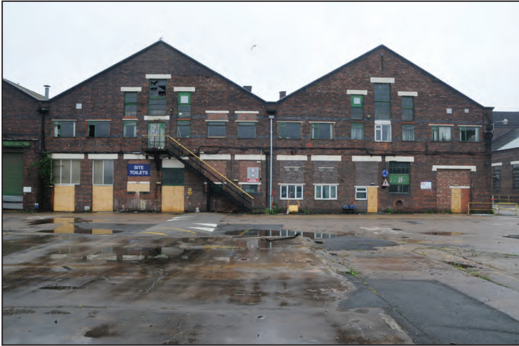
Photograph No. Washwood227 Description: Exterior east gable ends (offices) Site Location: A1/A2 Direction From: E
