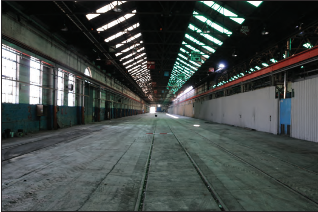
Photograph No. Washwood013 Description: Shed interior with rail tracks Site Location: G3 Direction From: W
