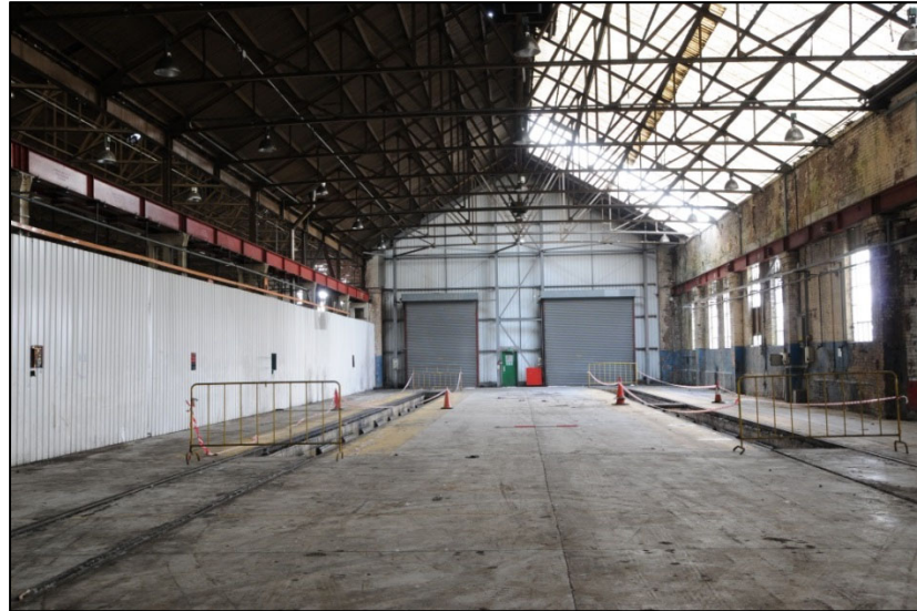
Plate 6: Inspection pit at the western end of F1
