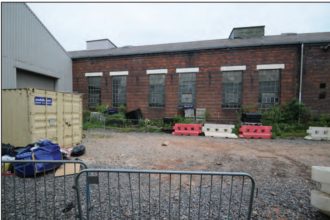
Photograph No. Washwood136 Description: west end of exterior south elevation Site Location: F5 Direction From: SE
