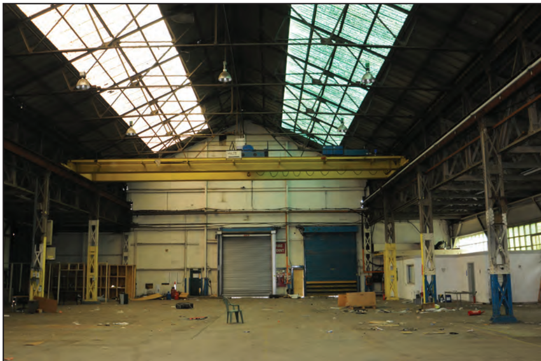
Photograph No. Washwood130 Description: Interior east gable end with travelling crane in front Site Location: H1 Direction From: W
