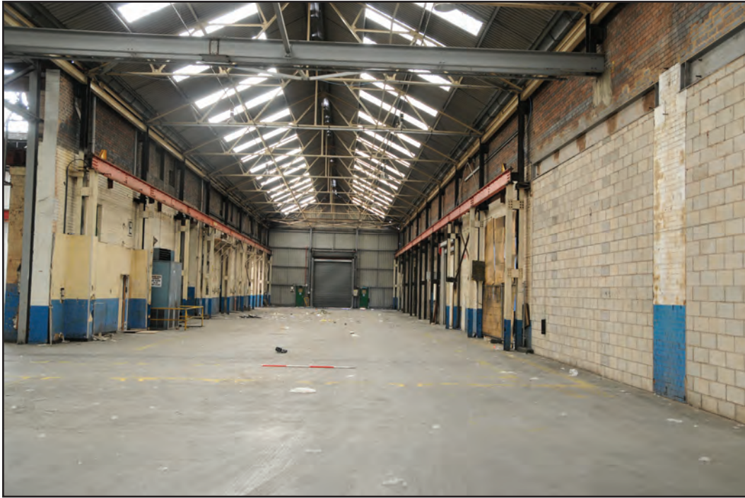
Photograph No. Washwood041 Description: Shed interior and south gable end interior elevation Site Location: D10 Direction From: N
