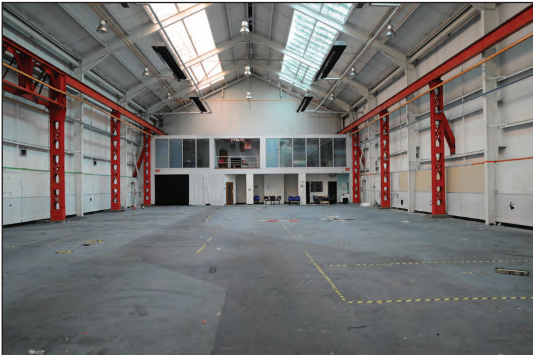
Photograph No. Washwood212 Description: Large shed area interior and offices to the east Site Location: H2 Direction From: W
