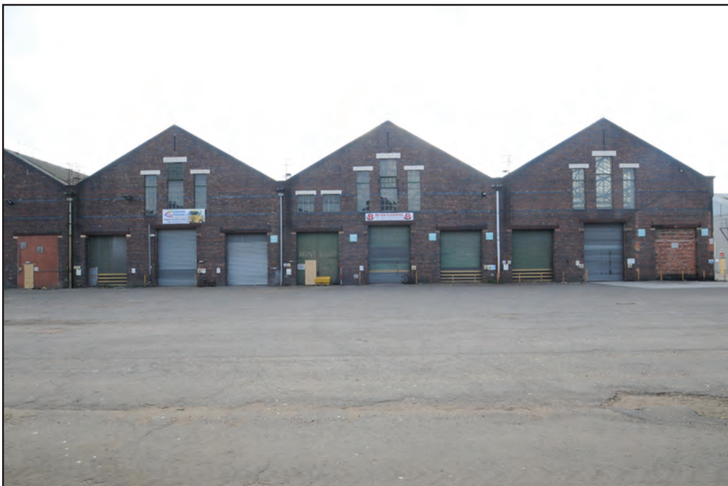
Photograph No. Washwood162 Description: Exterior east gable ends Site Location: B1-B3 Direction From: E
