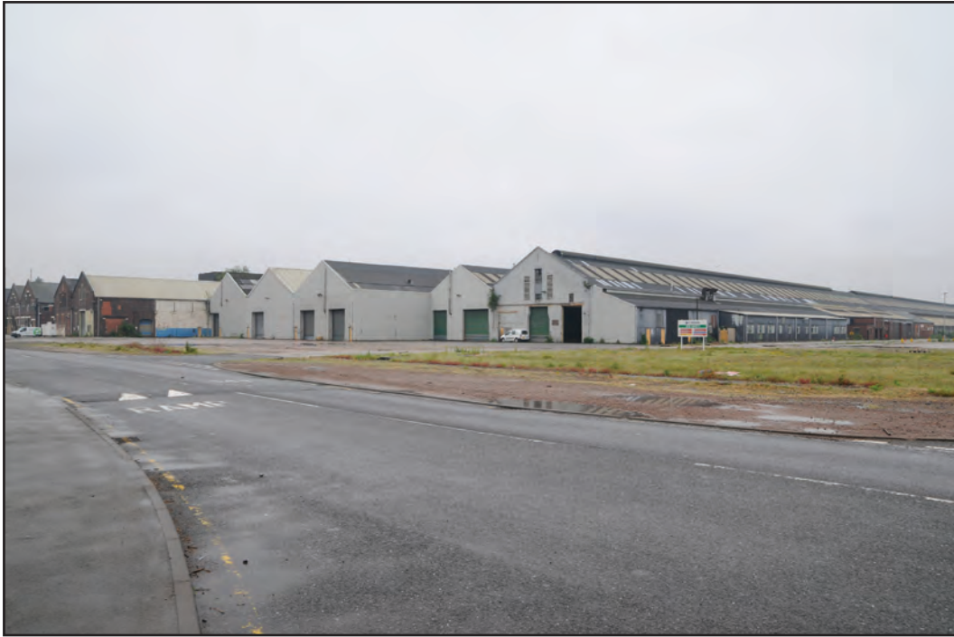
Photograph No. Washwood237 Description: View of relationship between buildings C and G, E gable ends Site Location: G/C Direction From: NE
