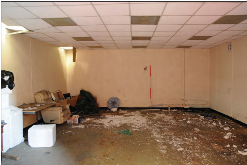
Photograph No. Washwood006 Description: Cabin office interior at west end of G2 Site Location: G2 Direction From: E
