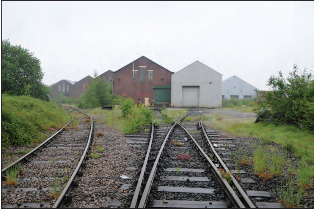
Photograph No. Washwood219 Description: Train rails leading into the west end gables of Building F Site Location: F Direction From: W
