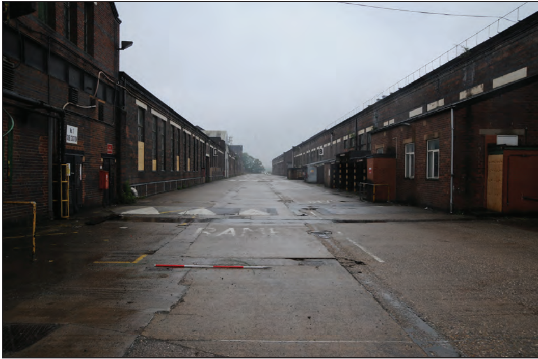
Photograph No. Washwood225 Description: Relationship between Buildings A, B and C Site Location: A/B/C Direction From: W
