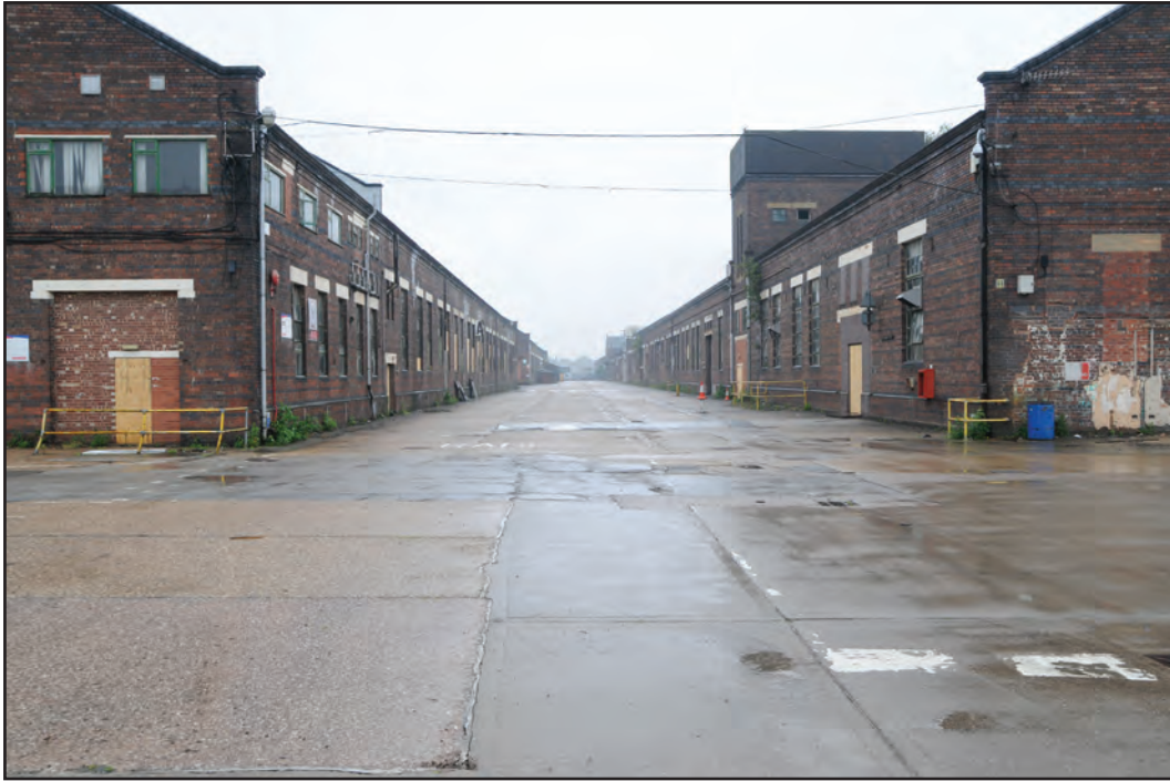
Photograph No. Washwood229 Description: Relationship between Buildings A and C Site Location: A/C Direction From: E
