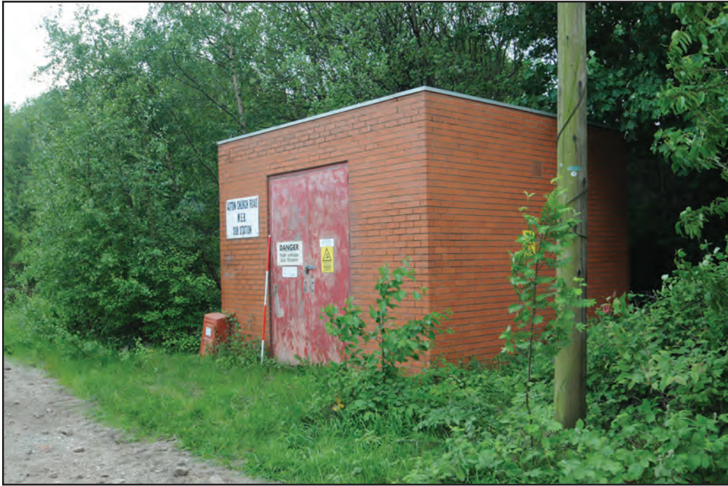
Photograph No. Washwood135 Description: Exterior north and west elevations of small sub-station at southwest corner of site Site Location: Sub-station Direction From: NW
