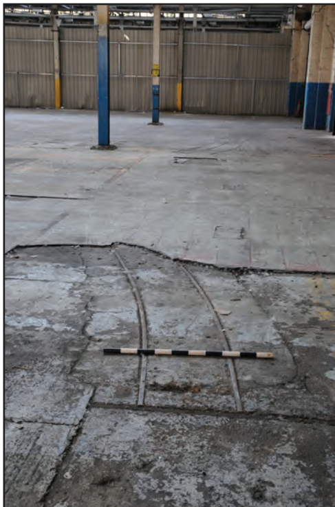
Photograph No. Washwood072 Description: Curved cart tracks at interior east end of shed Site Location: D7 Direction From: S
