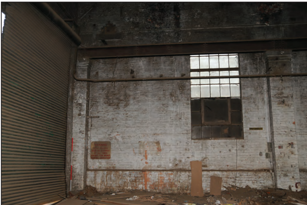
Photograph No. Washwood180 Description: west end of north wall interior elevation with low and high bricked openings Site Location: A1 Direction From: S
