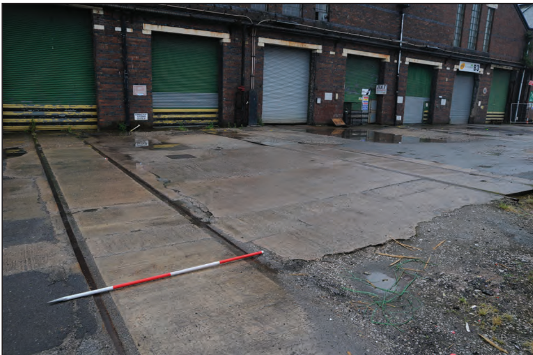
Photograph No. Washwood224 Description: Rail lines leading into west gable ends of Building B Site Location: B Direction From: WNW
