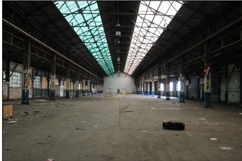
Plate 9: Interior of Shed H1
