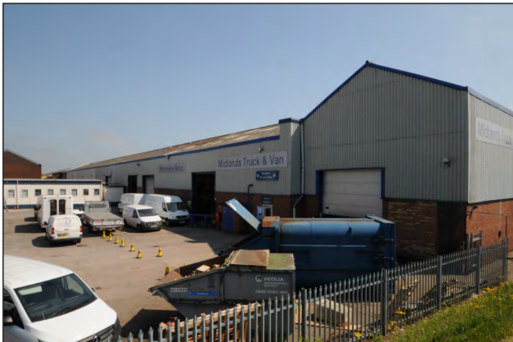
Photograph No. Saltley030 Description: General view of exterior west elevations Site Location: Midlands/Mercedes Direction From: SW
