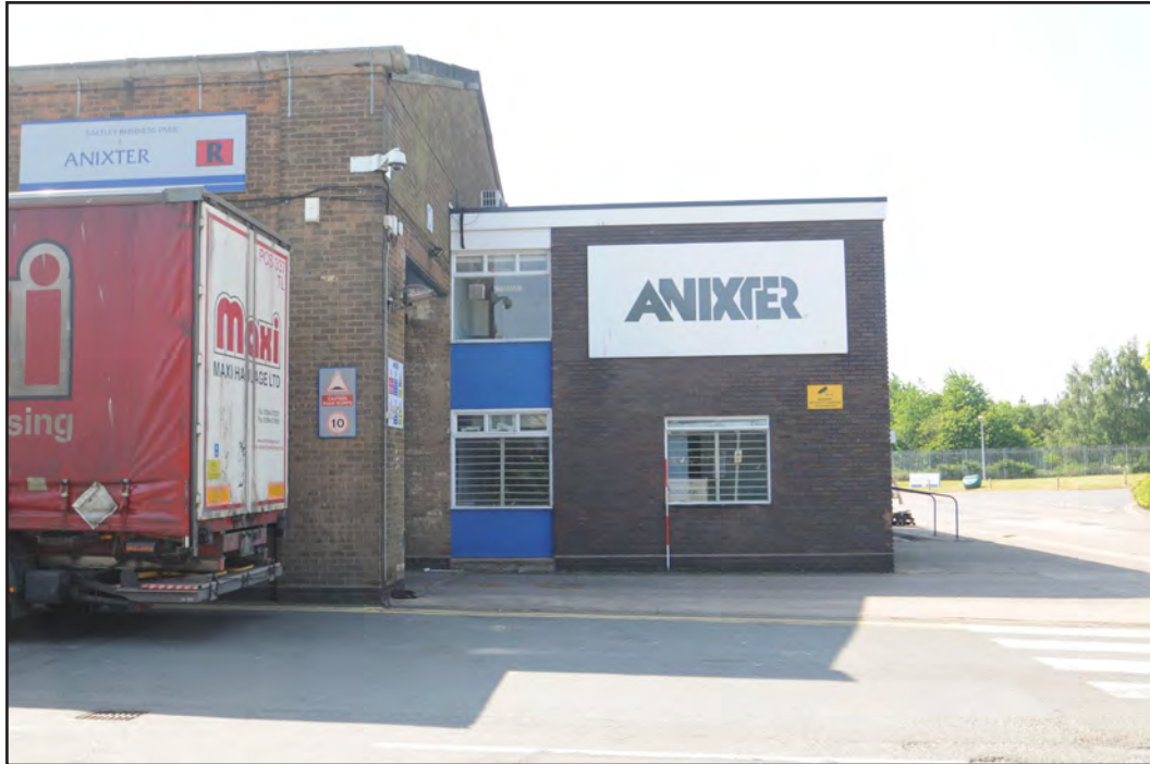
Photograph No. Saltley061 Description: Exterior east elevation, north end of shed and office area Site Location: Anixter Direction From: E
