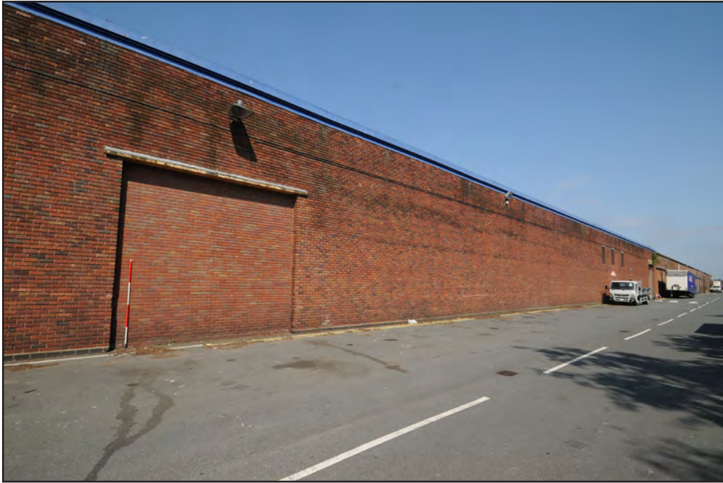
Photograph No. Saltley025 Description: General view of exterior east elevation, central area Site Location: Mercedes-Benz Direction From: SE
