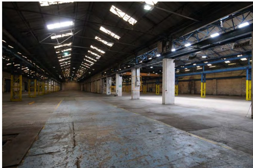
Plate 2: Internal view of Shed A
