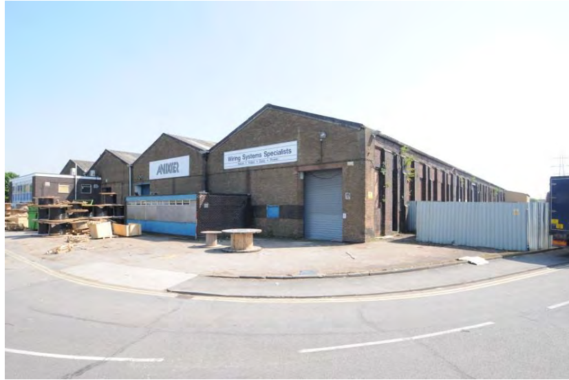
Plate 1: Shed A with modern offices attached to the north elevation
