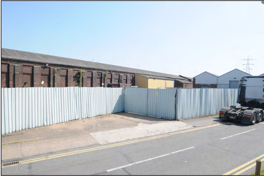
Photograph No. Saltleyo67 Description: Exterior west elevation, south area Site Location: Anixter Direction From: NW
