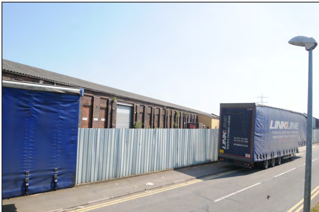
Photograph No. Saltley066 Description: Exterior west elevation, central area Site Location: Anixter Direction From: NW
