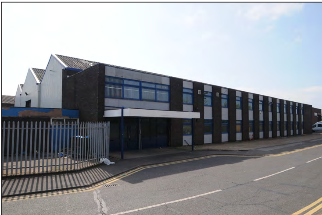
Photograph No. Saltley010 Description: General view of exterior west elevation - offices Site Location: Unit 5 Direction From: NW
