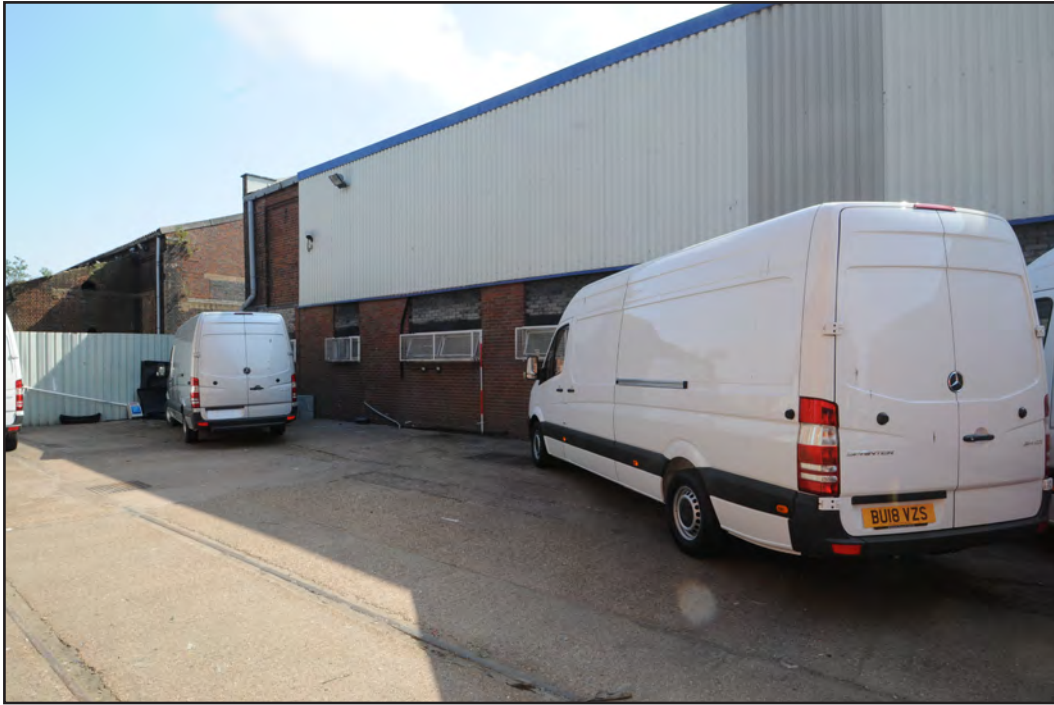
Photograph No. Saltley013 Description: General view of exterior west elevation, north end Site Location: Mercedes-Benz Direction From: SW
