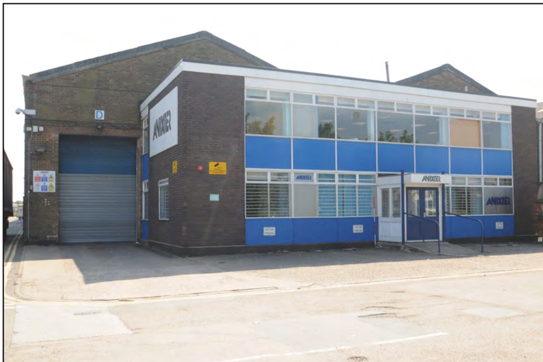
Photograph No. Saltley062 Description: Exterior north elevation of shed and northeast office area Site Location: Anixter Direction From: NNE
