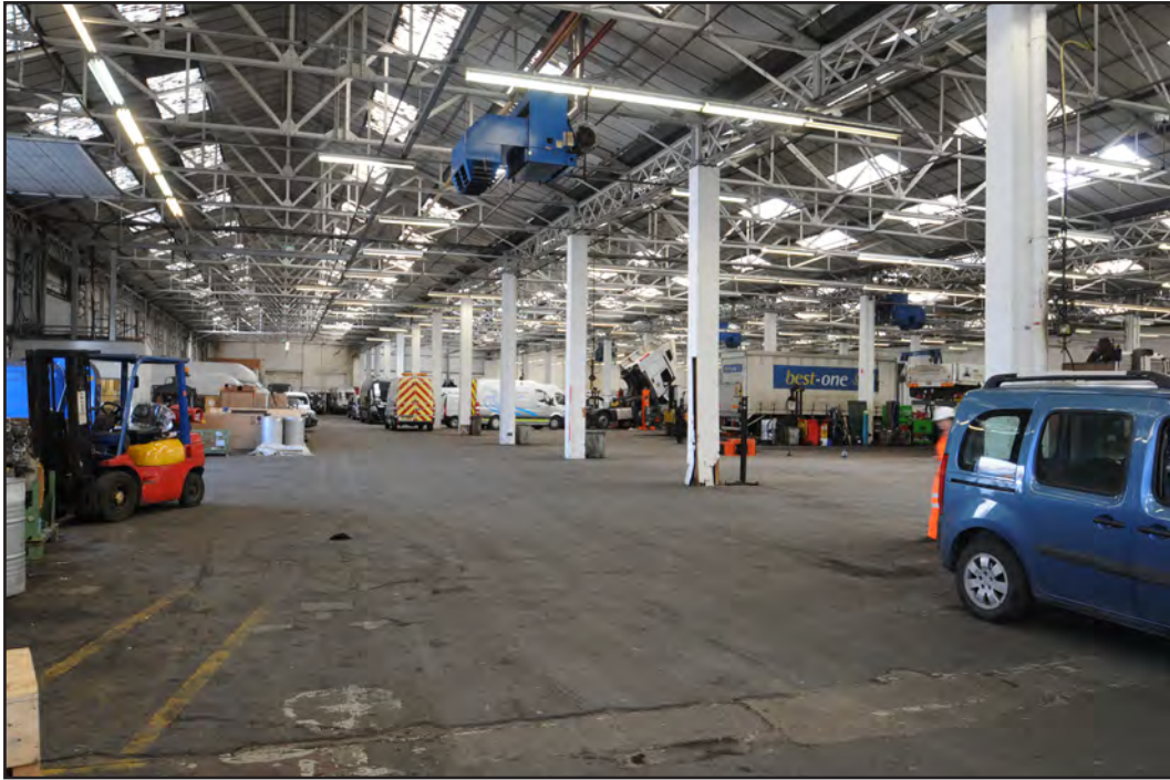
Photograph No. Saltley017 Description: General view of shed interior Site Location: Mercedes-Benz Direction From: SW
