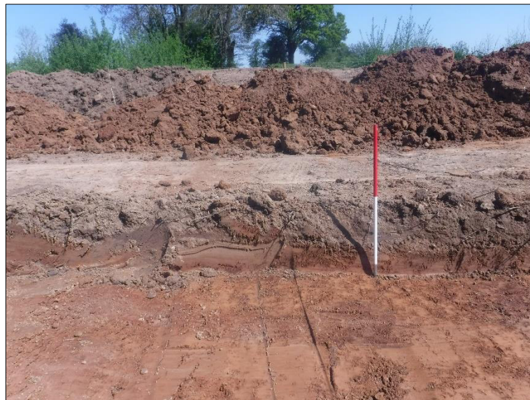
Plate 3: Representative section of haul road excavation
