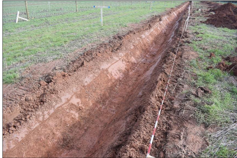
Plate 2: Post-excavation shot of drainage ditch
