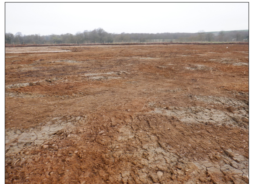
Plate 18: Post-excitation shot of Area C32098, looking W
