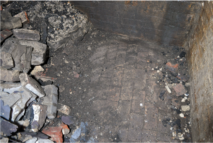
Plate 13: Detail of brick floor in Cell 2.
