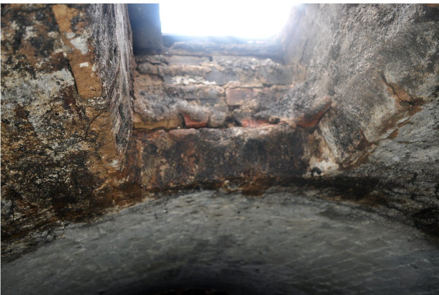
Plate 15: Detail of brickwork in access hatch in vault of Cell 2.
