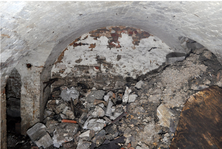
Plate 11: Cell 2 looking east with concrete from blocking of Cell 3 to right.
