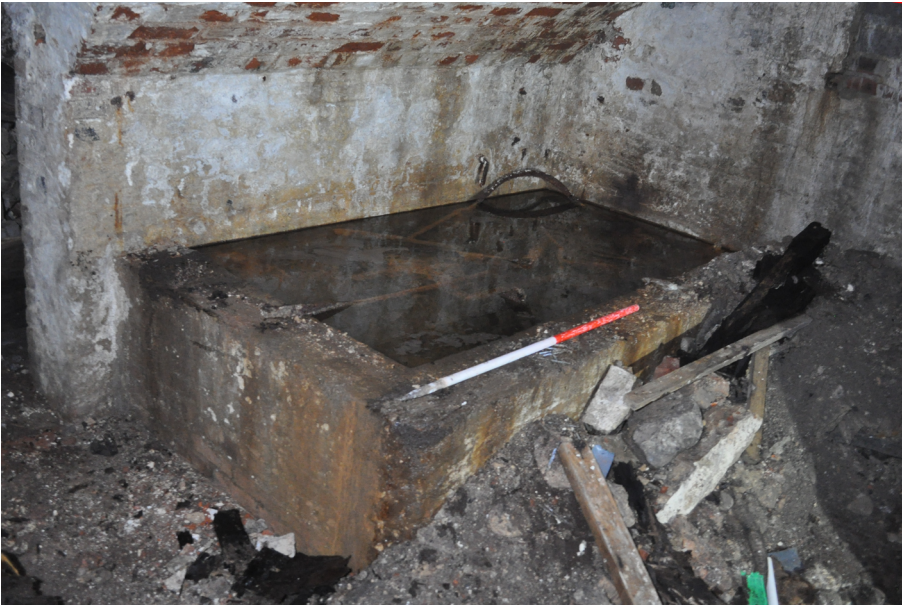
Plate 10: Vat against south wall of Cell 1. 1m scale.
