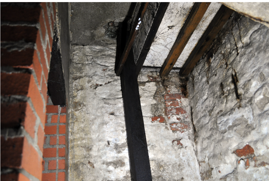
Plate 6: Detail of north west corner of Cell 1 showing detail of blocking of opening.
