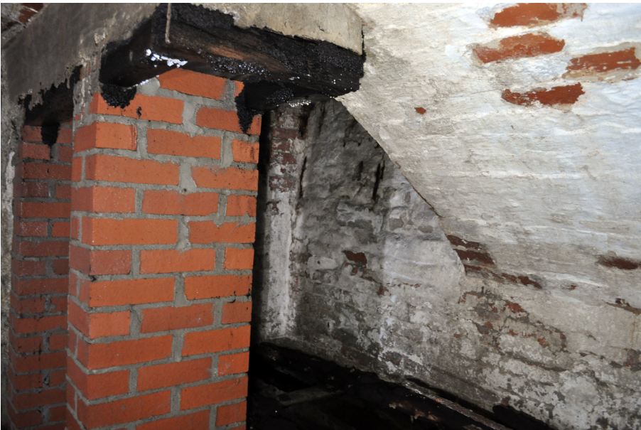
Plate 5: View of north west corner of Cell 1.
