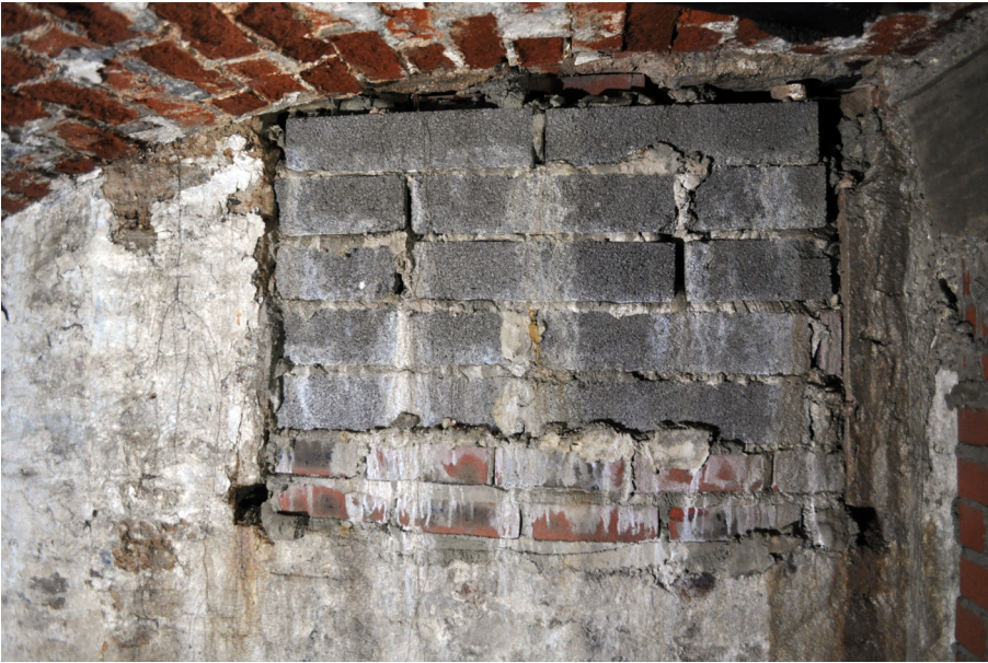
Plate 4: Blocked window in west wall of Cell 1.
