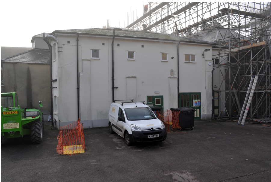
Plate 2: View of area of proposed new extension with locations of boreholes BH02 and BH03 surrounded by orange netlon fencing, looking south.
