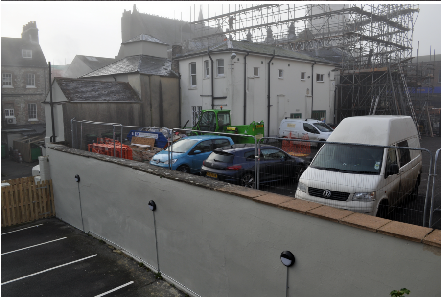
Plate 3: View of retaining wall of terrace constructed for nineteenth century Market House, looking south.
