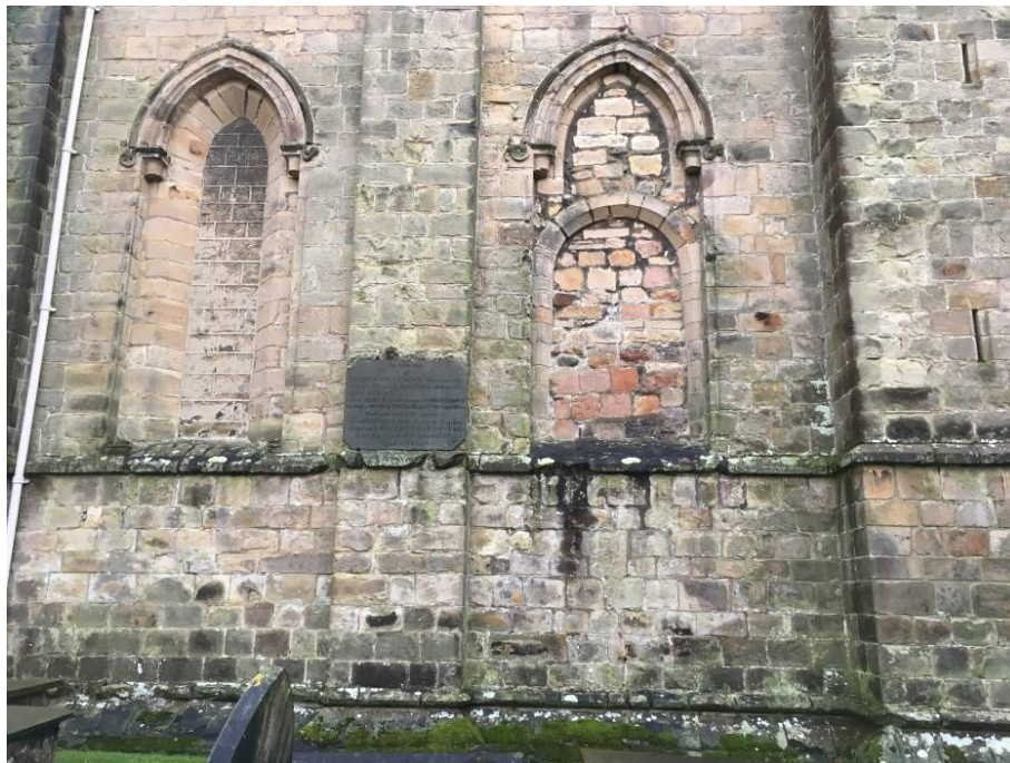
Fig.13: north wall of north transept
