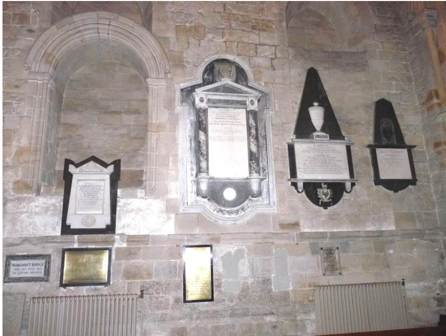
Fig.19: north wall of north transept with blocked openings and later memorials
