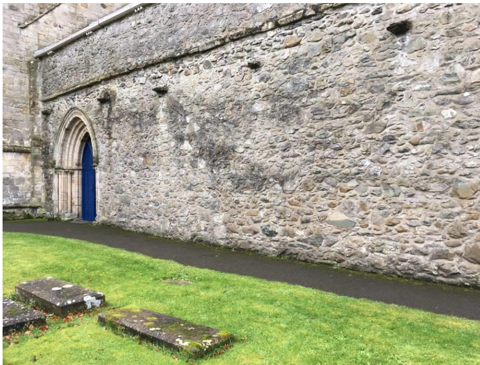
Fig.12: north aisle wall, from north-west
