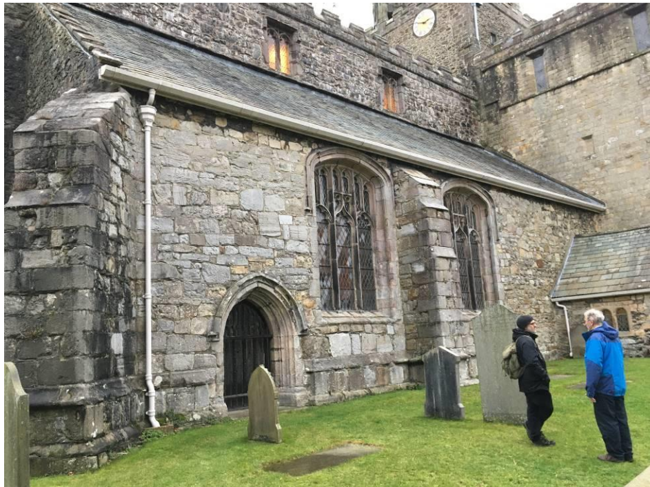
Fig.9: the south aisle, from the south-west
