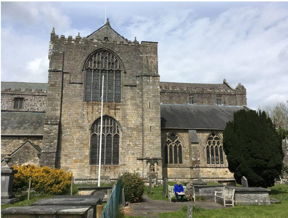
Fig.8: the church from the south
