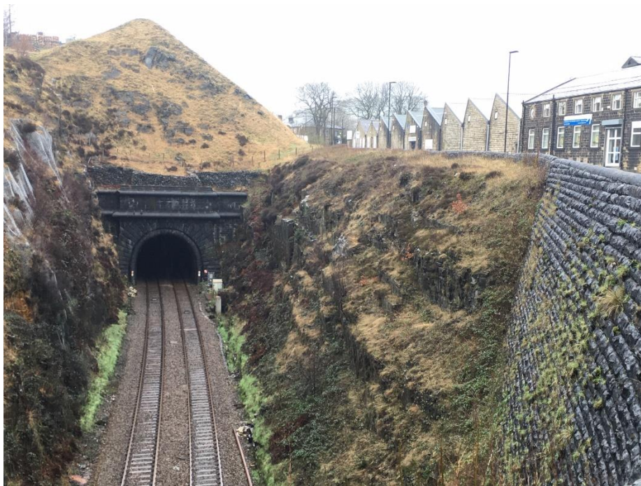
Fig.2: south portal of Summit Tunnel and Sladen Wood Mill, from the south
