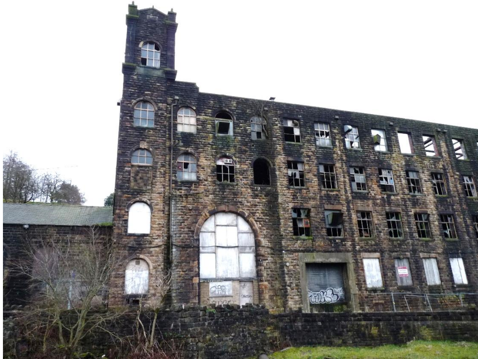
Fig.10: the north end of the mill from the west, with 1898 tower to the left and engine house position marked by the wide arched opening
