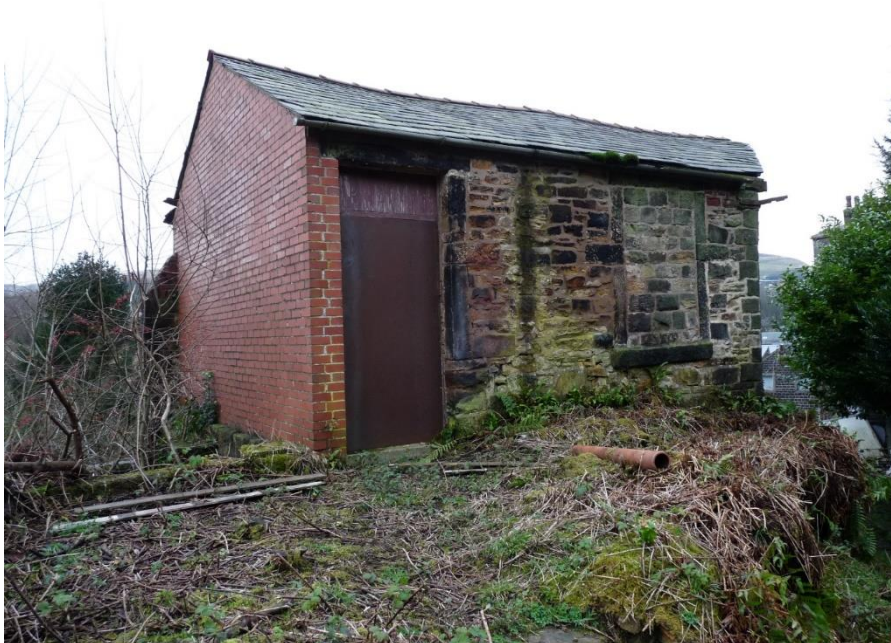
Fig.23: Summit Quarry building from the east
