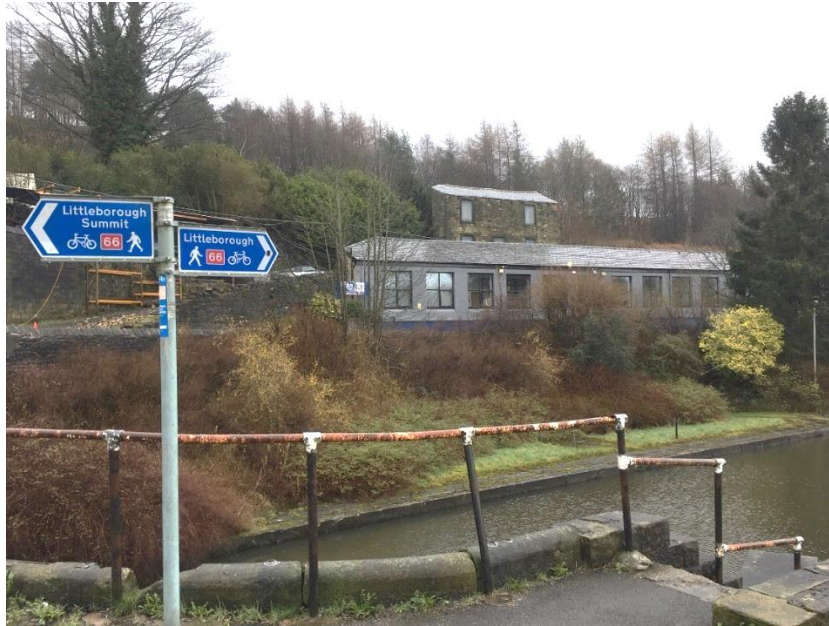
Fig.4: footpath signage on restored canal at Punch Bowl Bridge
