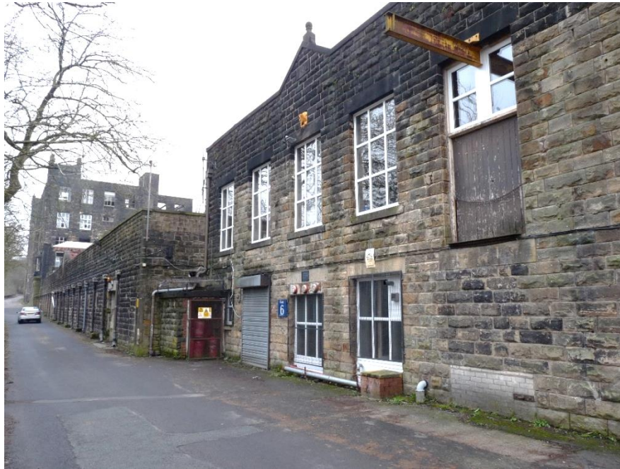
Fig.19: Building 4: warehouse built 1892, from the south
