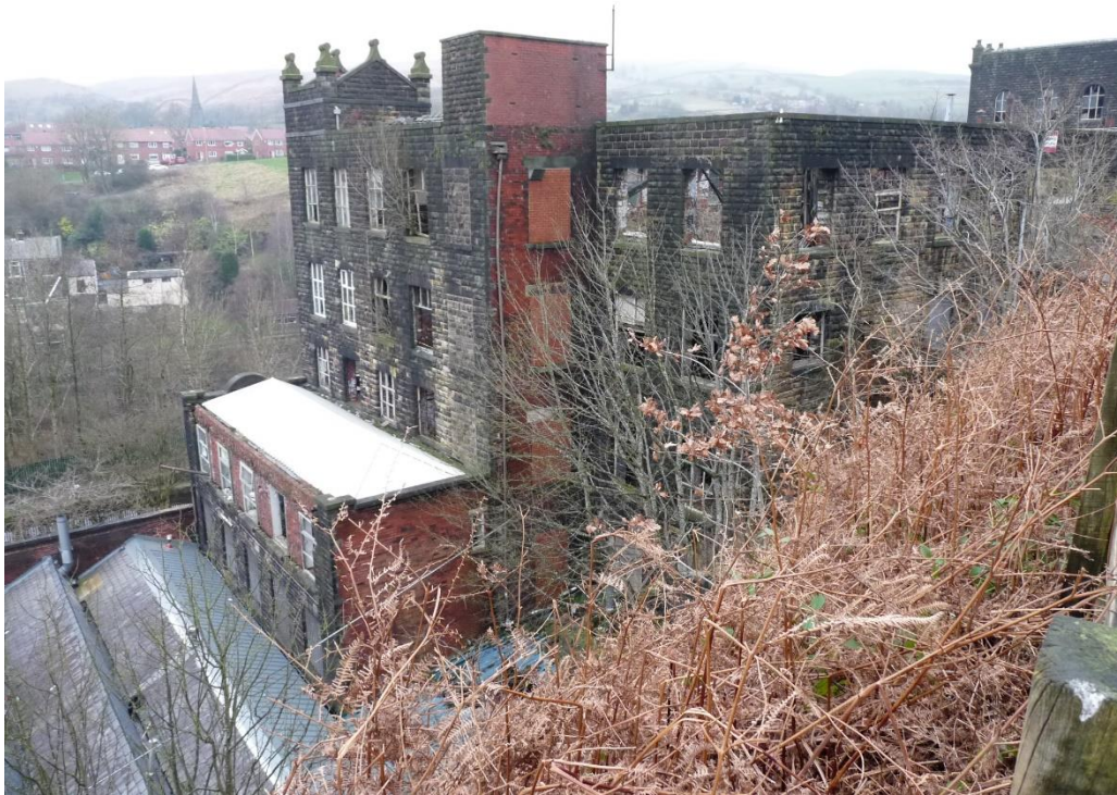
Fig.14: south-east corner of mill from the east, with 3-storey office to left
