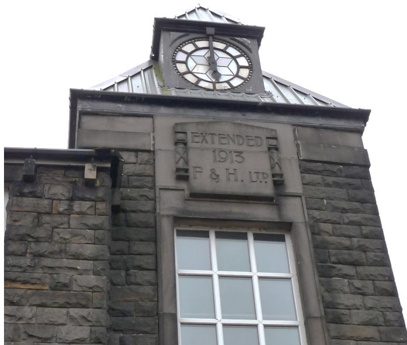
Fig.8: stair tower to Fothergill & Harvey Ltd 1913 extension
