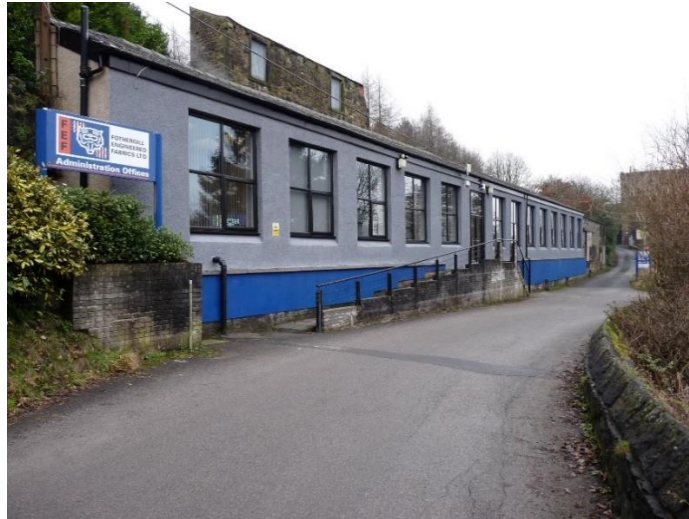
Fig.28: Fothergill Engineered Fabric Ltd offices, from the north
