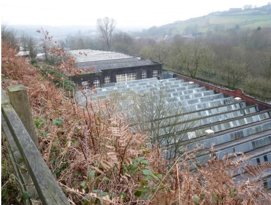
Fig.20: view onto roofs of Buildings 3, 4 and 5, from the north-east
