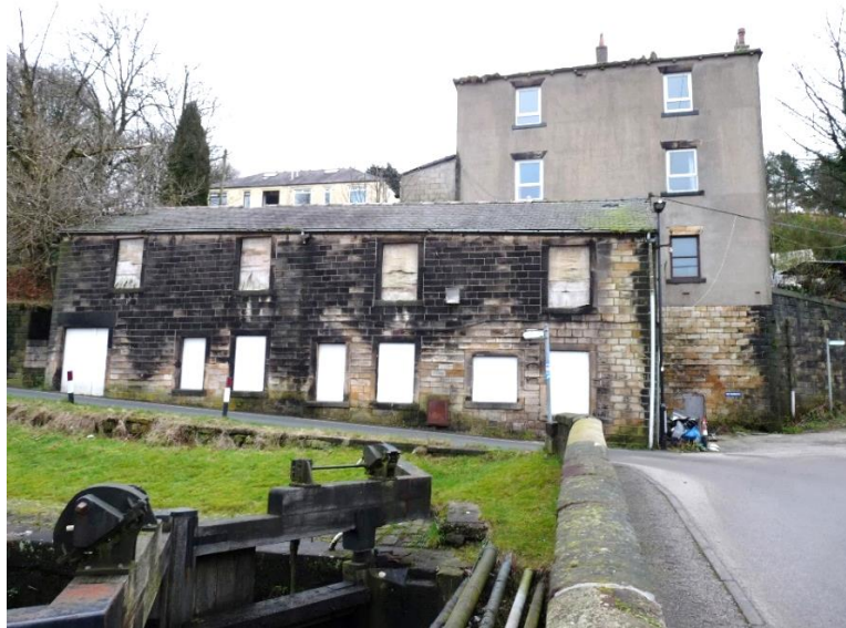
Fig.26: Prospect House and the former stable and cottages, from the west
