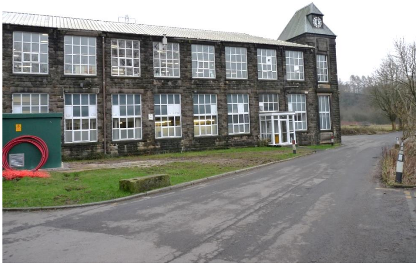
Fig.21: Building 6: 1913 additions to the mill, at south end of complex
