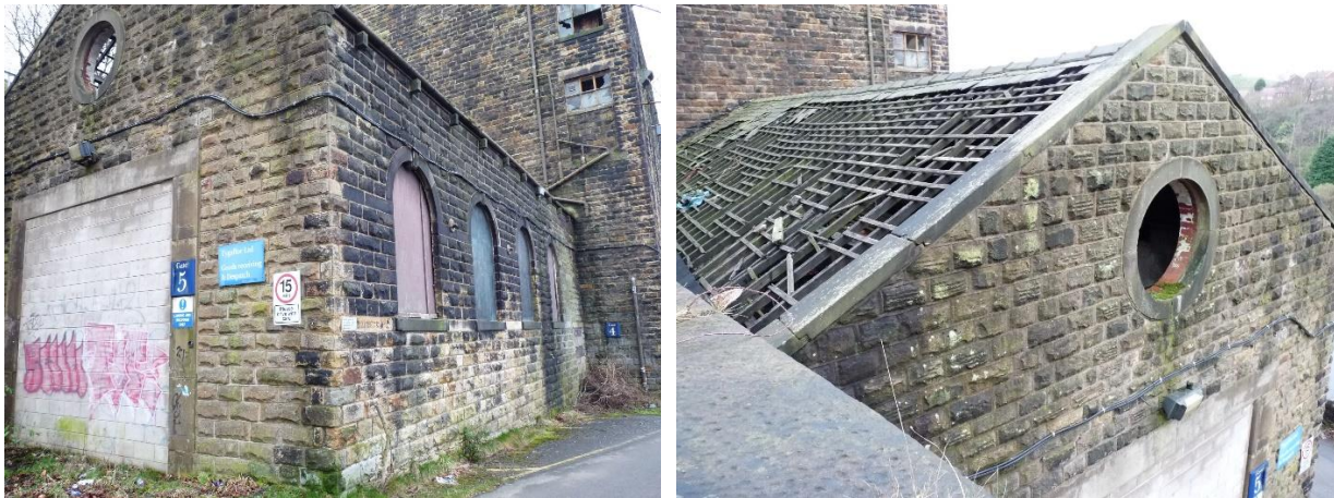
Fig. 17: the boiler house at the north end of the mill
