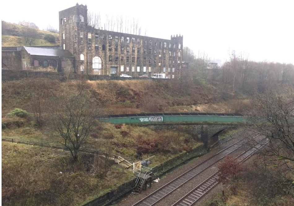
Fig.30: Rock Nook Mill seen from Todmorden Road over the railway line and Roch aqueduct
