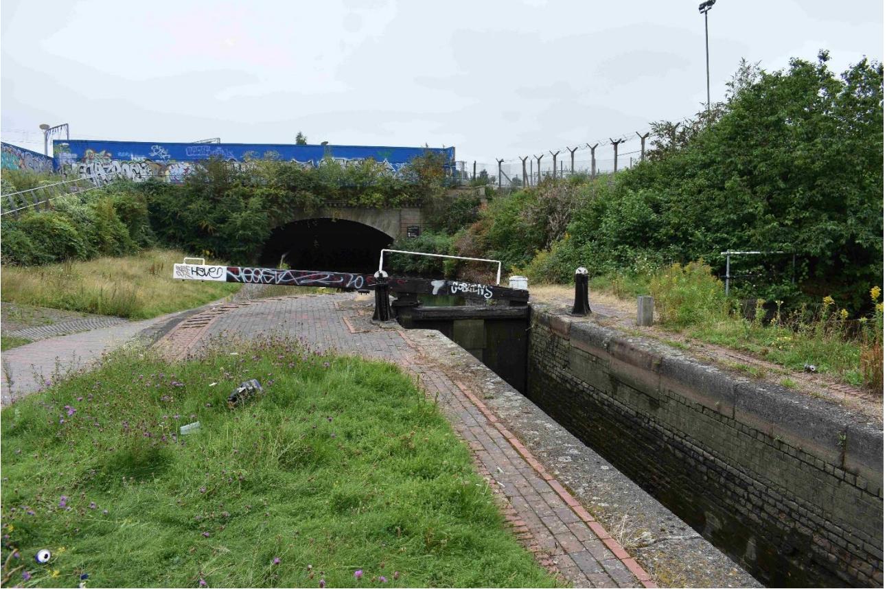
Plate 16: Ashted Bottom Lock viewed from the north (taken 14 August 2020)
