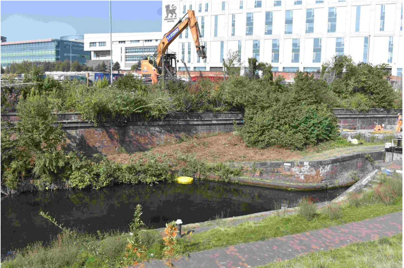
Plate 20: General view of wall after vegetation removal (taken 21 September 2020)
