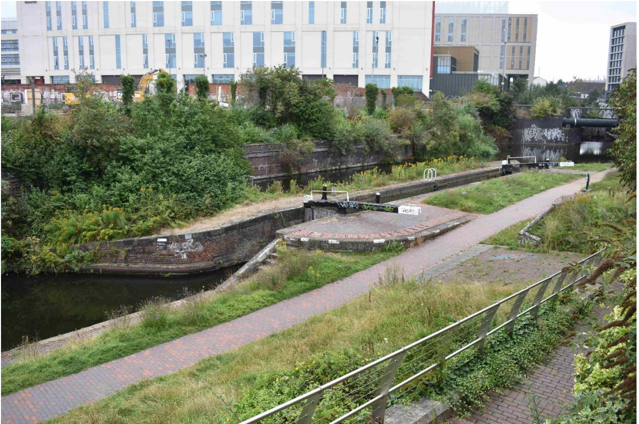
Plate 1: General view from south-east of Digbeth Branch Canal with the retaining wall in background (taken 14 August 2020)
