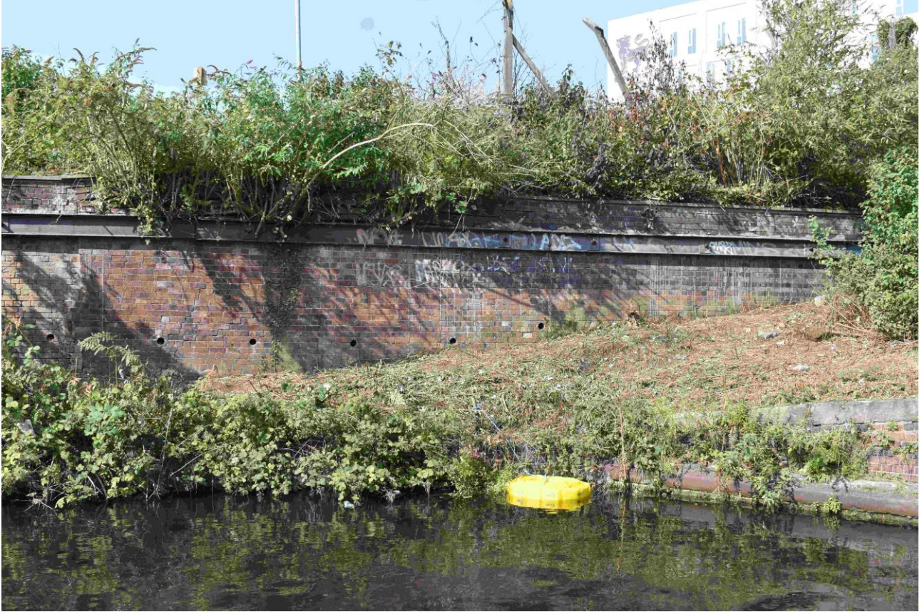
Plate 17: Northern part of Section C following vegetation removal (taken 21 September 2020).
