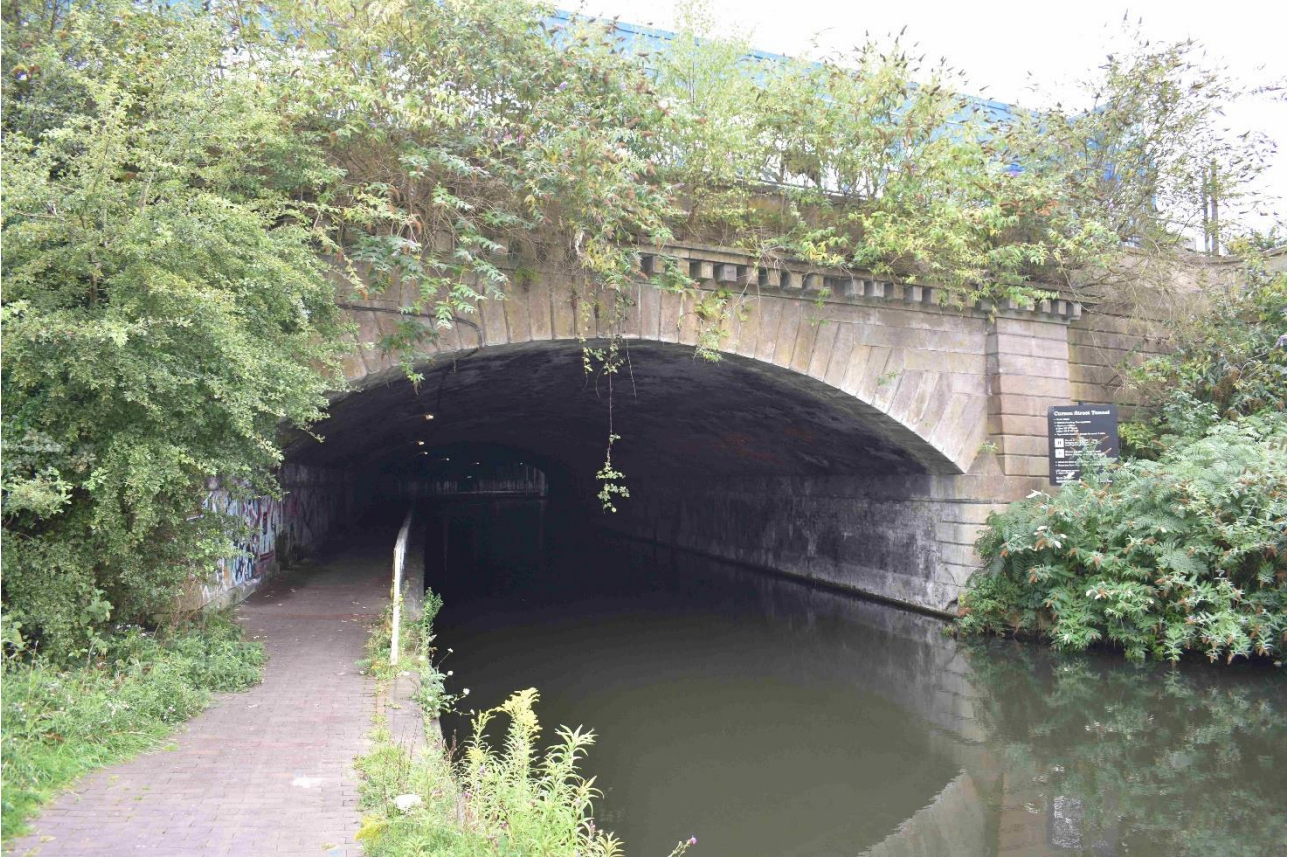
Plate 14: North portal of the former railway bridge (taken 14 August 2020)
