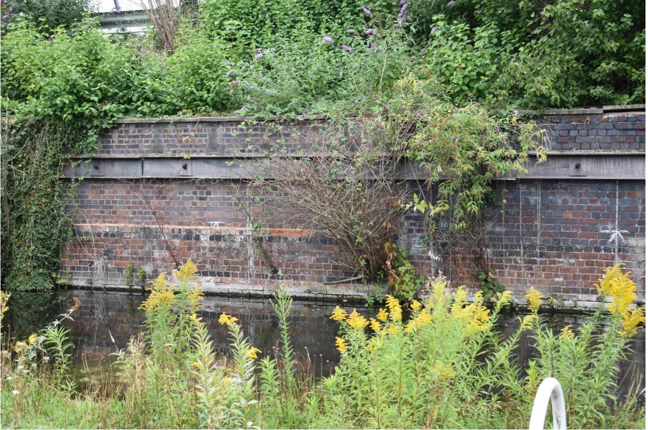
Plate 9: Section B (central part of the canal wall) taken 14 August 2020. The upper part of the brickwork to the left side of the photo is probably of late 20th-century date. Note vegetation and poor condition of the canal wall.
