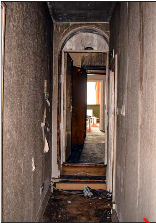
Plate 158: First floor corridor of manager’s house looking north
