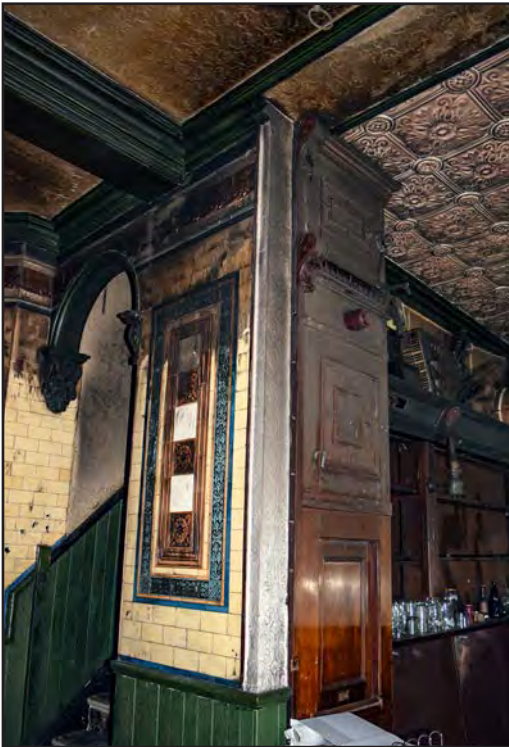
Plate 57: Former dumb waiter at east end of bar
