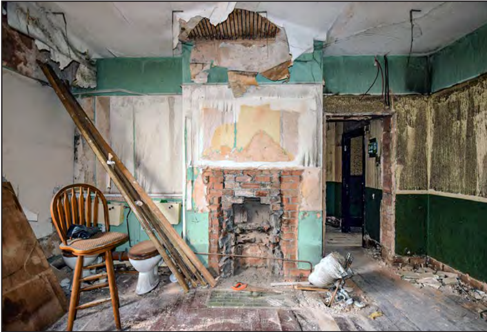
Plate 153: Room F6 after soft-strip looking west
