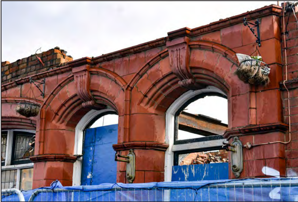
Plate 17: Detail of New Canal Street elevation during demolition
