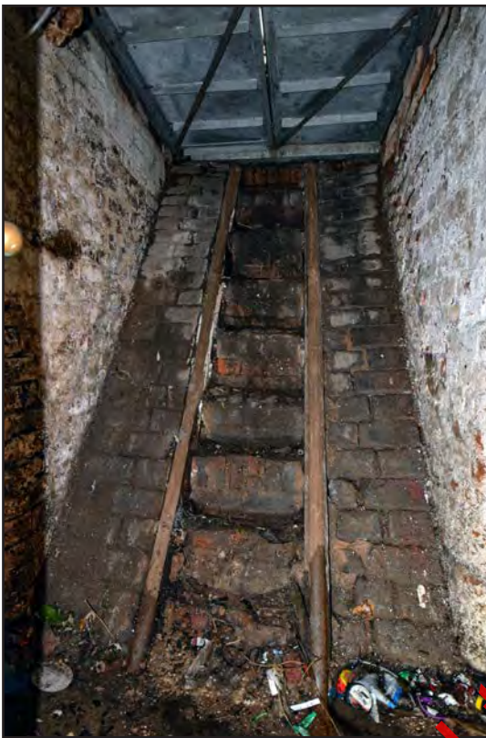
Plate 124: Barrel chute on south side of B2
