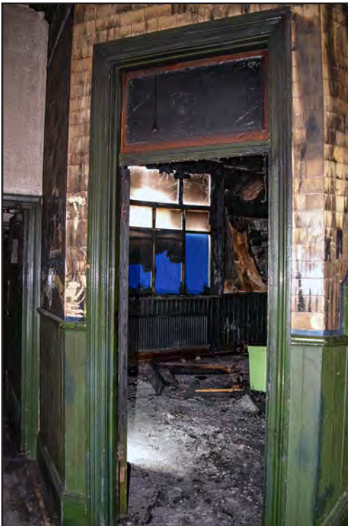
Plate 85: Entrance to Smoke Room from former corridor (before cleaning)
