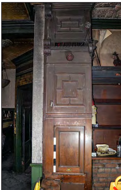
Plate 60: Front of dumb waiter at eastern end of bar
