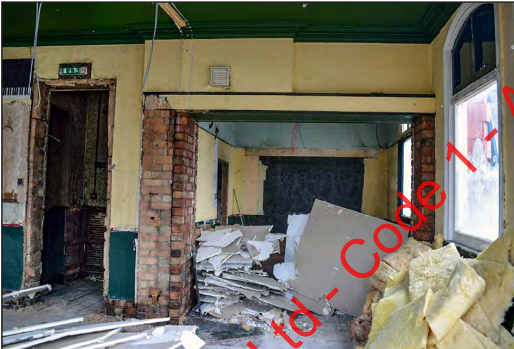
Plate 142: West end of Room F1 looking south
