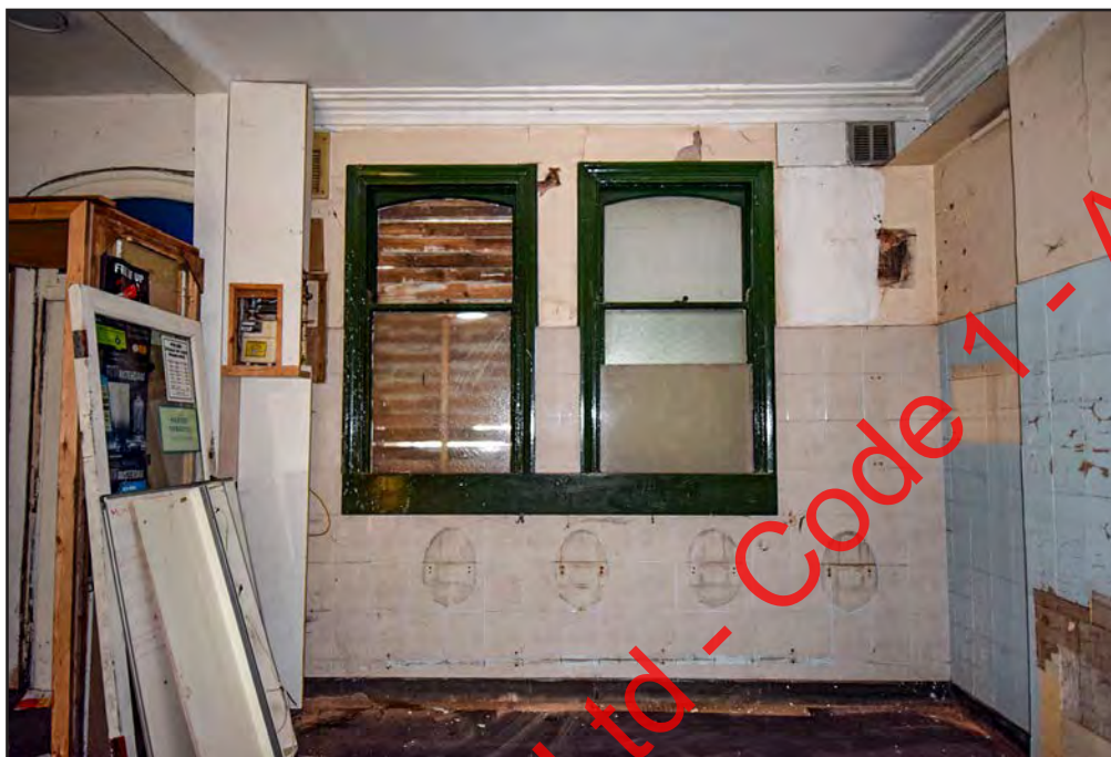
Plate 108: Ground floor windows to Pub Manager’s House to north of entrance
