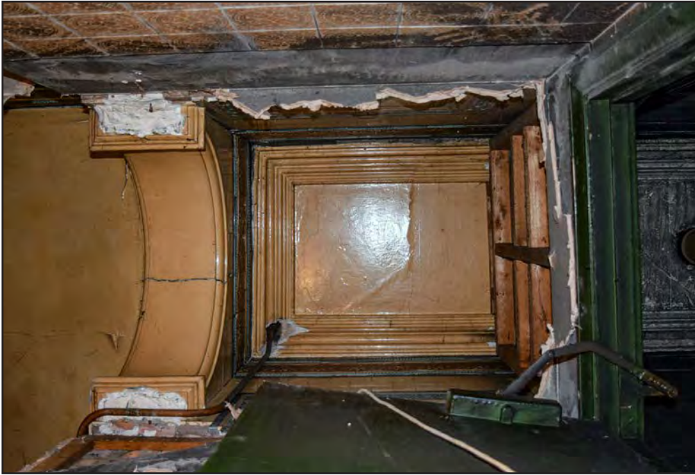
Plate 97: Primary ceiling exposed by removal of ceiling in passage towards WCs
