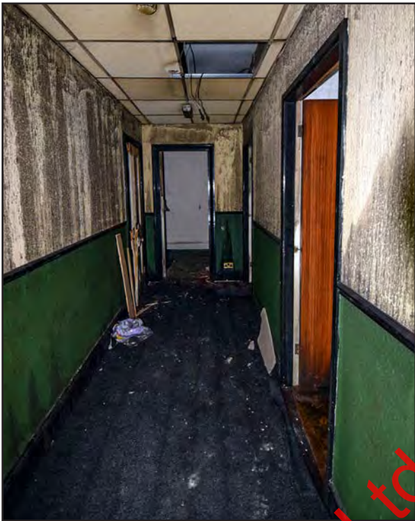
Plate 150: Room F6a looking east prior to soft-strip
