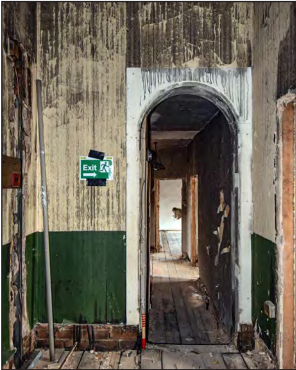
Plate 149: Room F4 looking south during soft-strip
