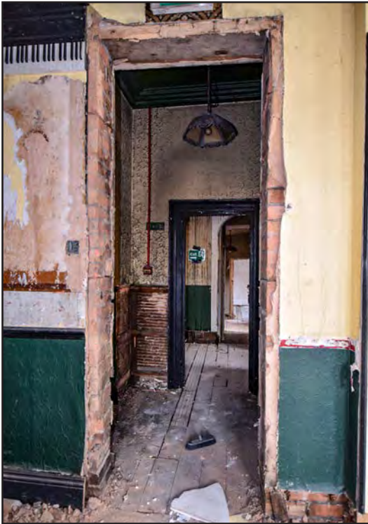
Plate 147: Southwards view from F1 through F3 and F4
