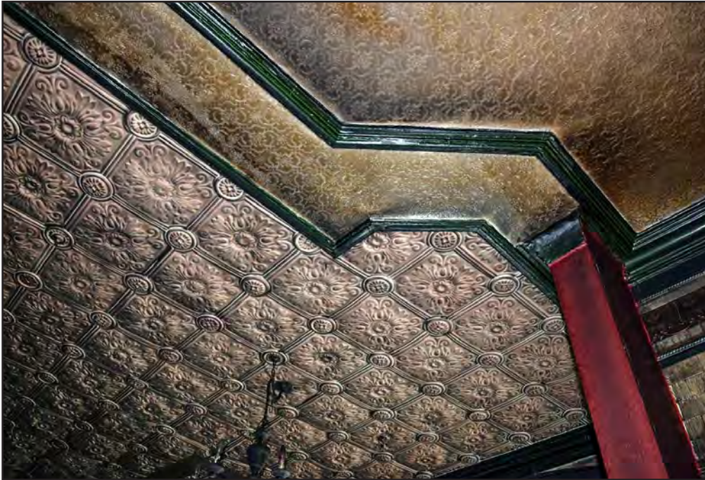
Plate 53: Outline in ceiling of former partition between bar and corridor from Banbury Street entrance
