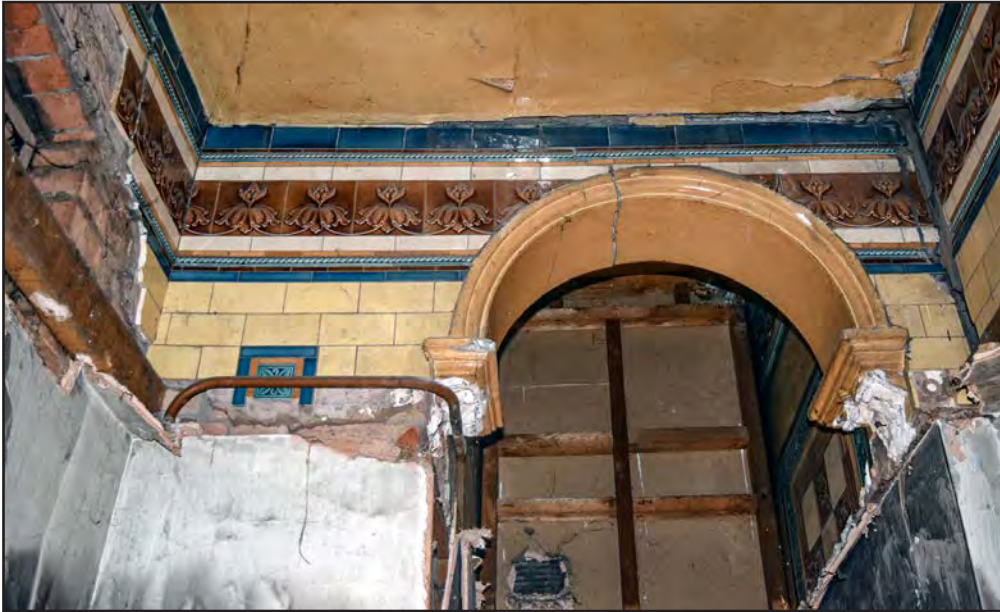
Plate 95: Decorative tiles exposed by removal of ceiling in WCs
