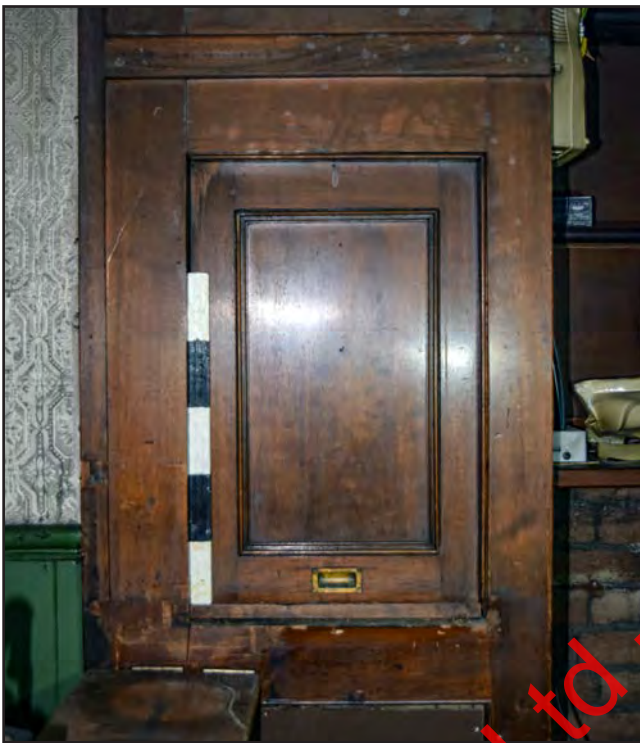
Plate 62: Front panel of dumb waiter
