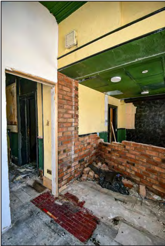
Plate 143: West end of Room F1 looking south
