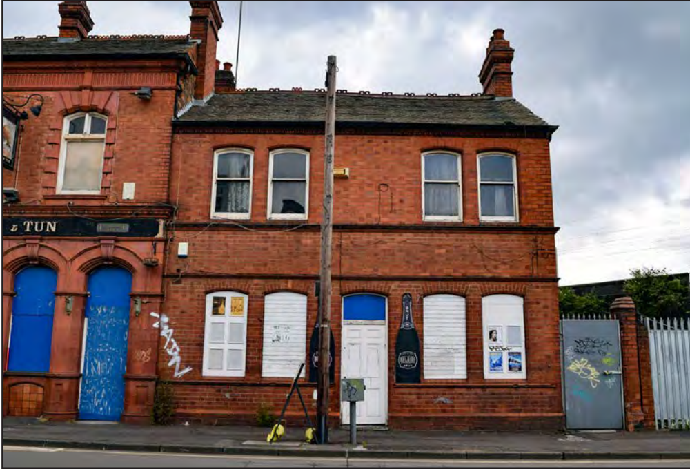
Plate 7: West elevation of pub manager's house
