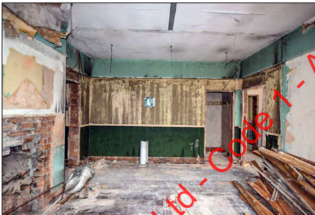
Plate 152: Room F6 after removal of modern partitions
