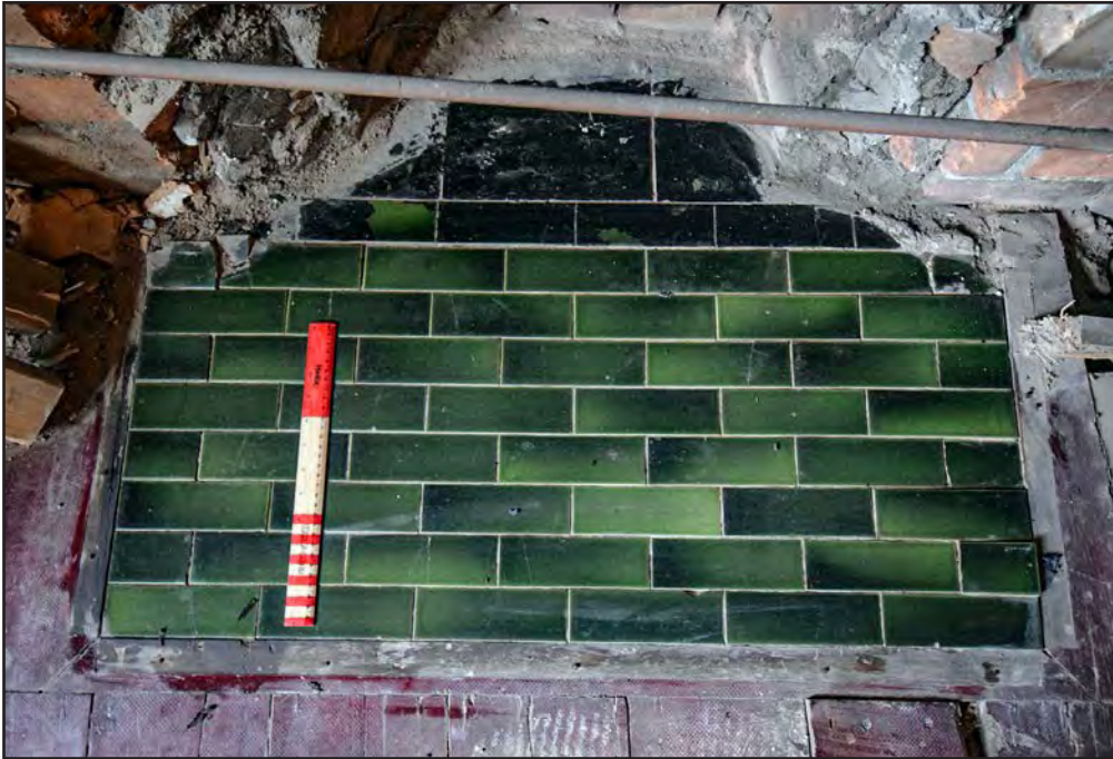
Plate 155: Hearth exposed from fireplace in Room F6 after soft-strip
