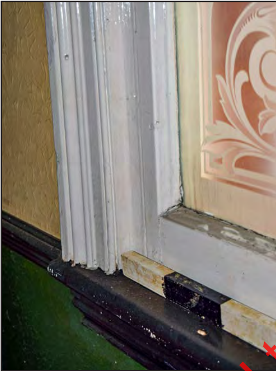
Plate 132: Architrave of window in F1 facing New Canal Street
