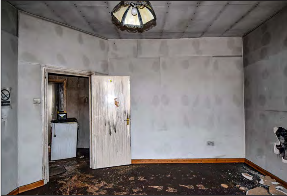
Plate 159: Room F10 looking east
