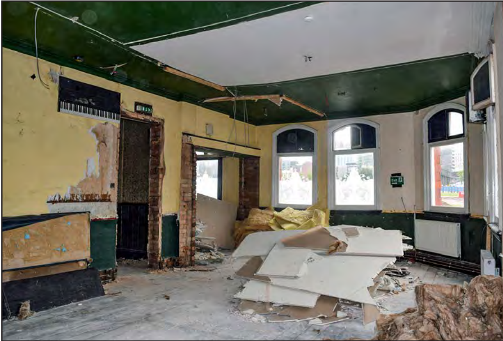
Plate 133: Room F1 looking west after removal of modern partitions
