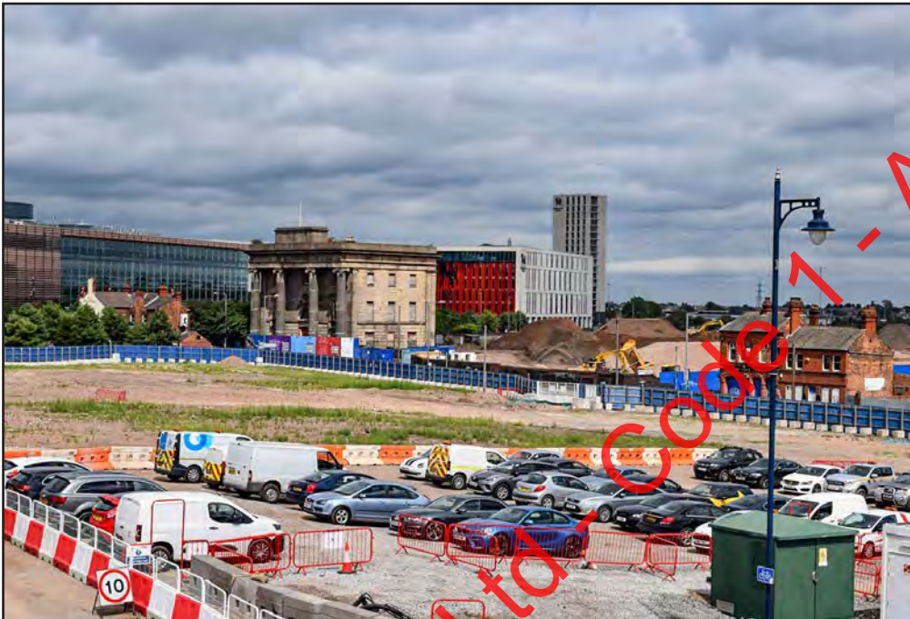
Plate 24: Distant view of Eagle and Tun and former Curzon Street Station building
