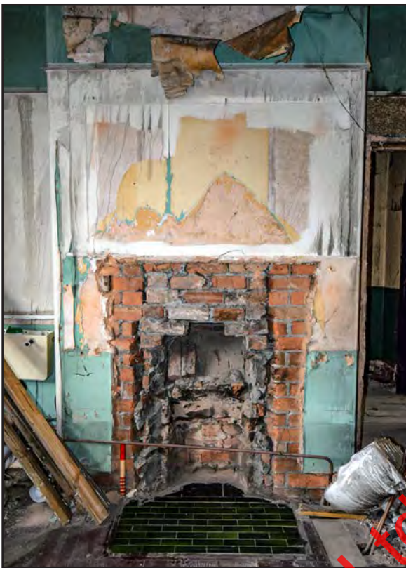
Plate 154: Fireplace in Room F6 after soft-strip
