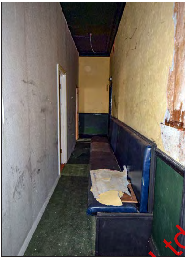
Plate 134: Corridor along south side of F1 before removal of modern partition
