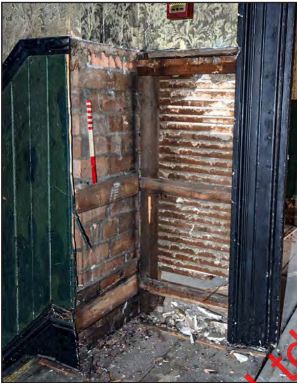
Plate 148: Exposed walls in lobby (F3) at top of stairs
