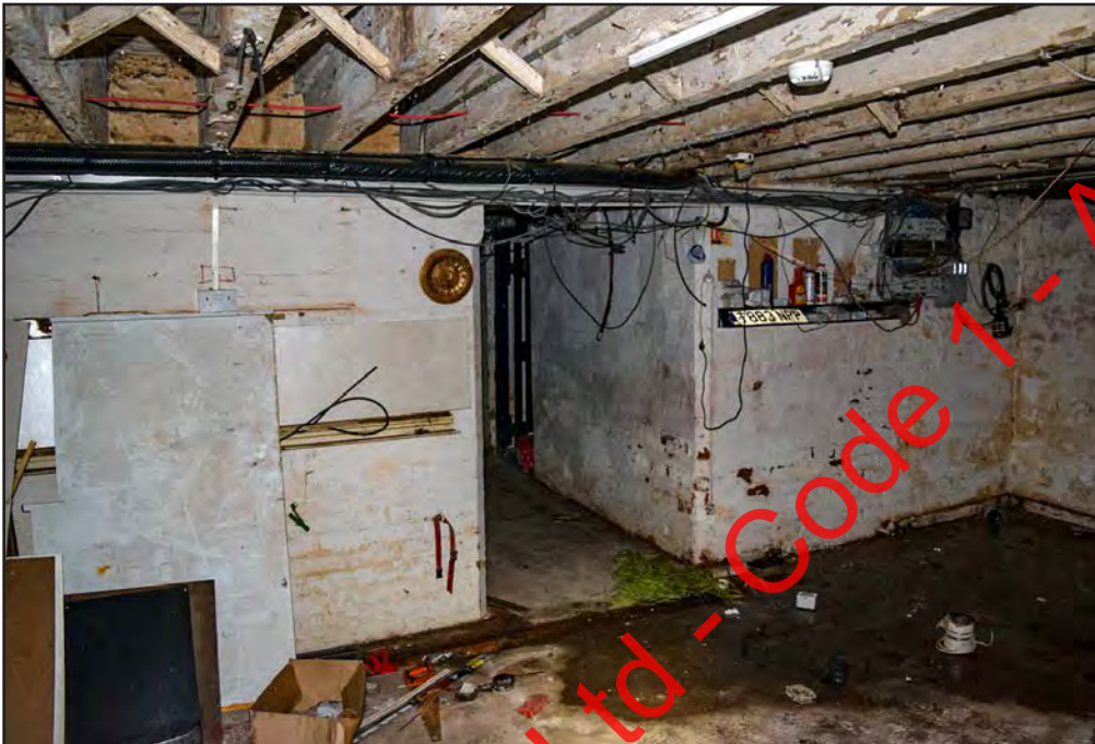
Plate 122: Opening from corridor into Room B1
