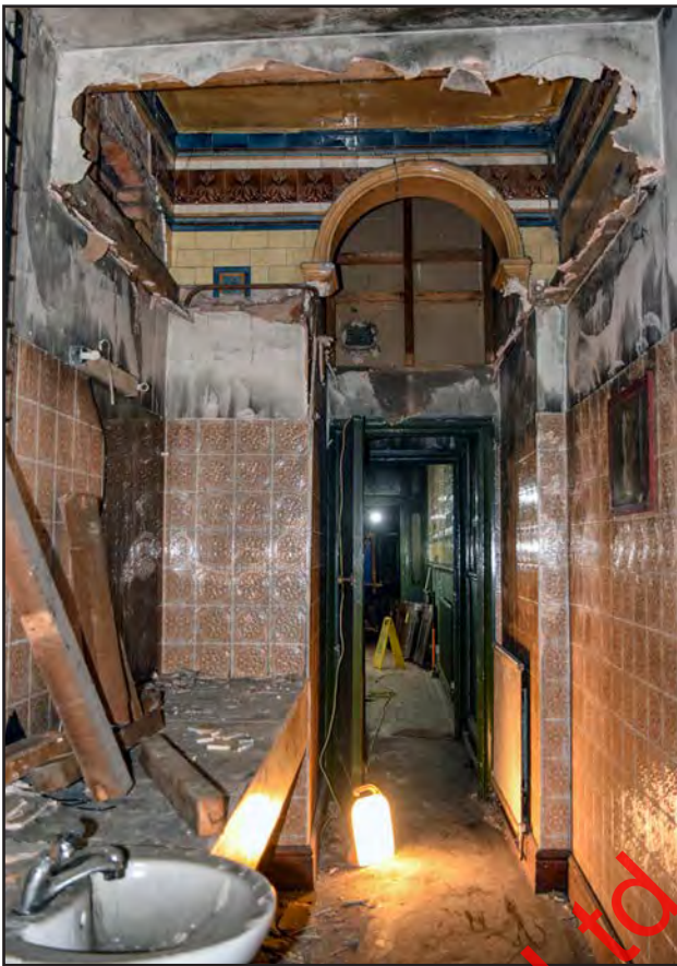
Plate 96: Decorative tiles exposed with later WC tiles below
