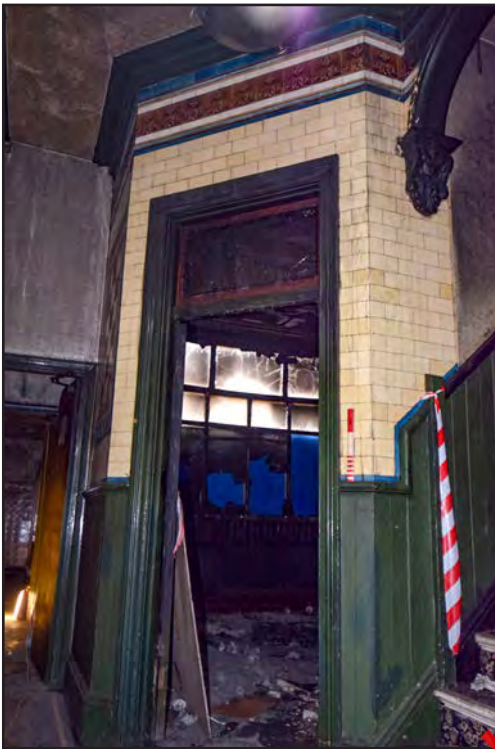
Plate 86: Entrance to Smoke Room from former corridor (after cleaning)
