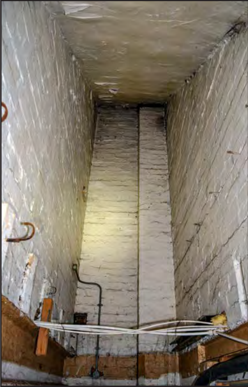
Plate 125: Underside of stairs on north side of B2
