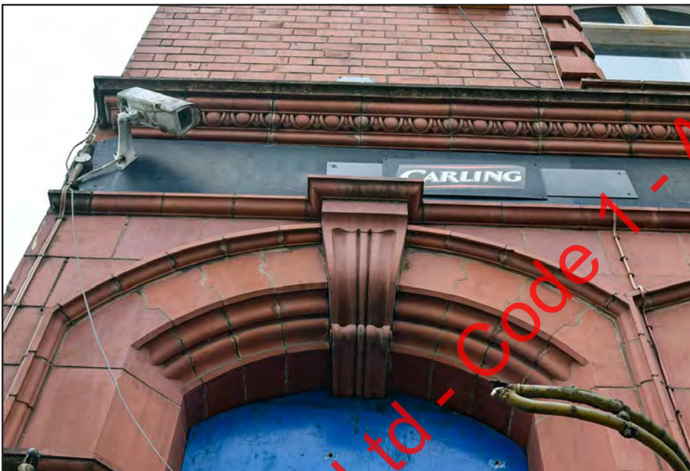
Plate 14: Terracotta detailing in Banbury Street elevation
