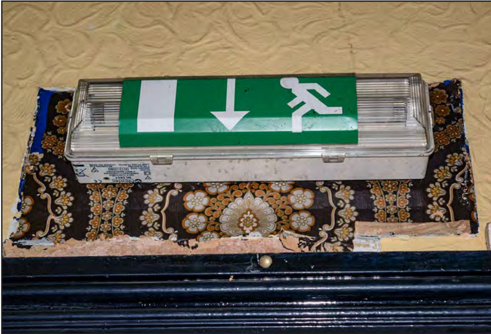
Plate 141: Scrap of wallpaper exposed above doorway on south wall of Room F1
