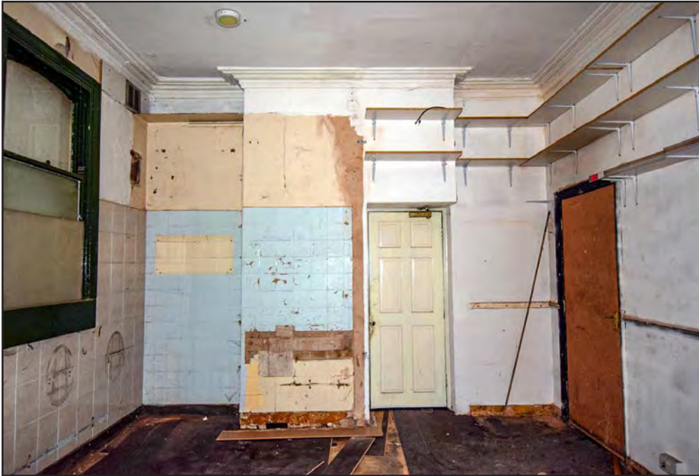
Plate 105: Ground floor of Pub Manager's House looking north
