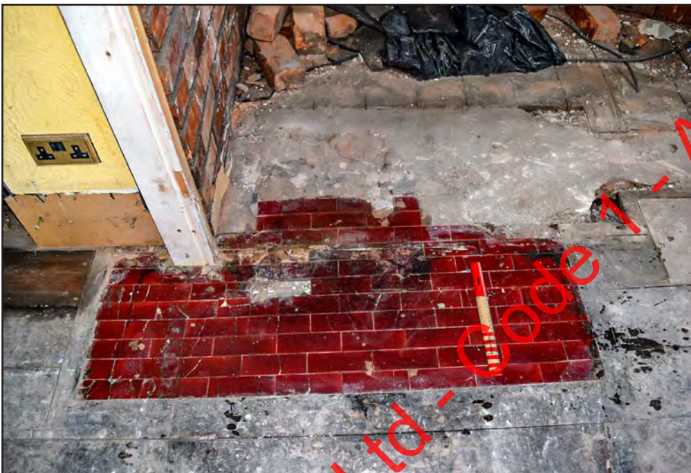
Plate 144: Hearth exposed from former fireplace towards SW corner of F1
