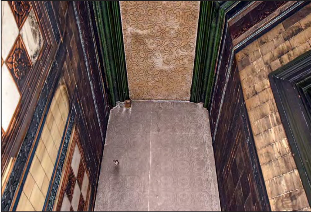
Plate 93: Passage towards WCs with inserted partition abutting cornice
