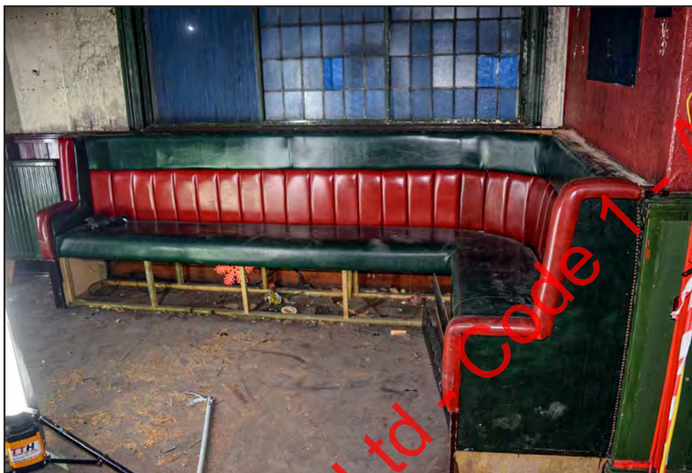
Plate 44: Benches within bar during soft-strip
