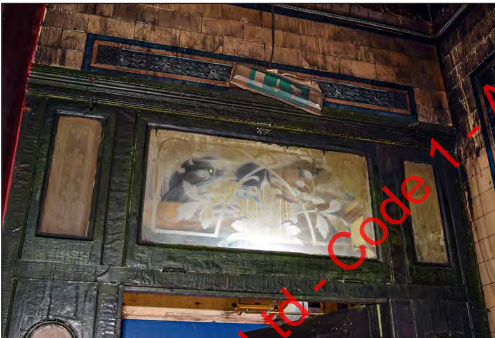
Plate 70: Glazed panel over entrance at north-east corner of pub
