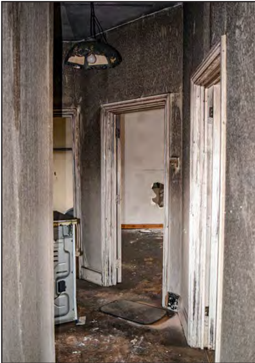
Plate 157: First floor corridor of manager’s house looking south
