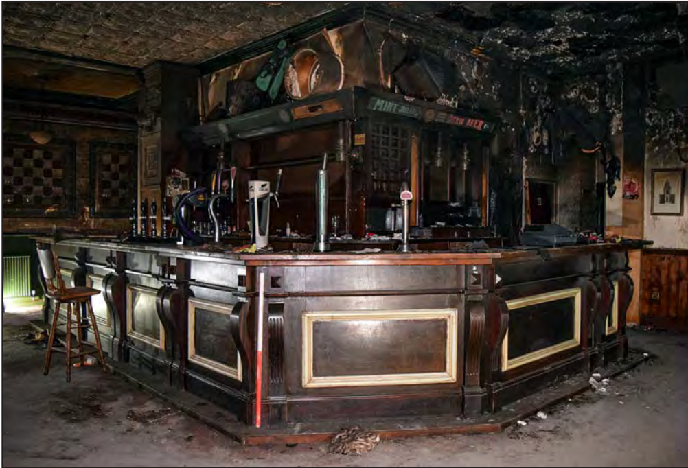
Plate 41: Bar looking south-east
