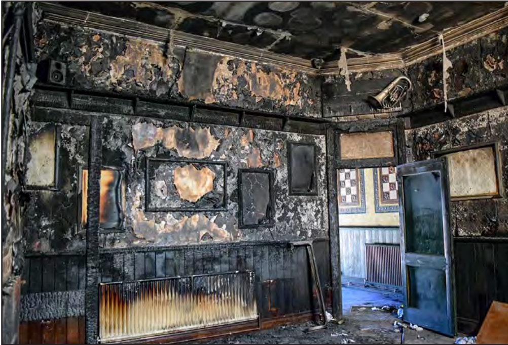
Plate 8g: Smoke Room looking north
