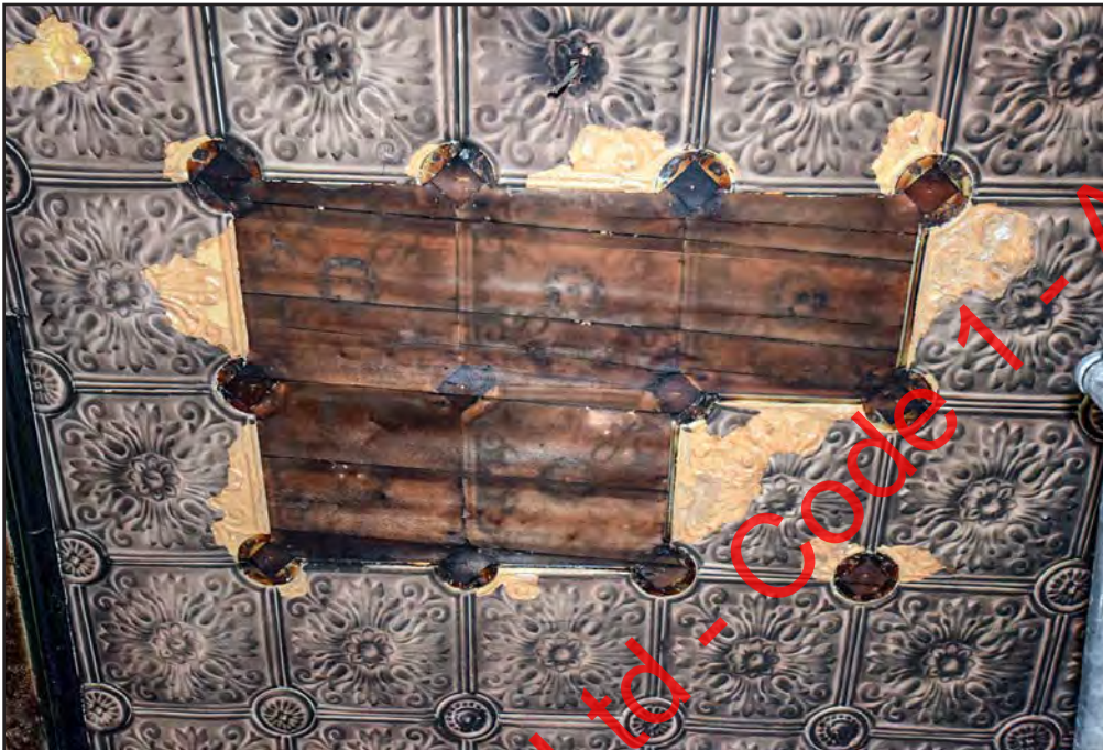
Plate 54: Public bar ceiling during removal of panels
