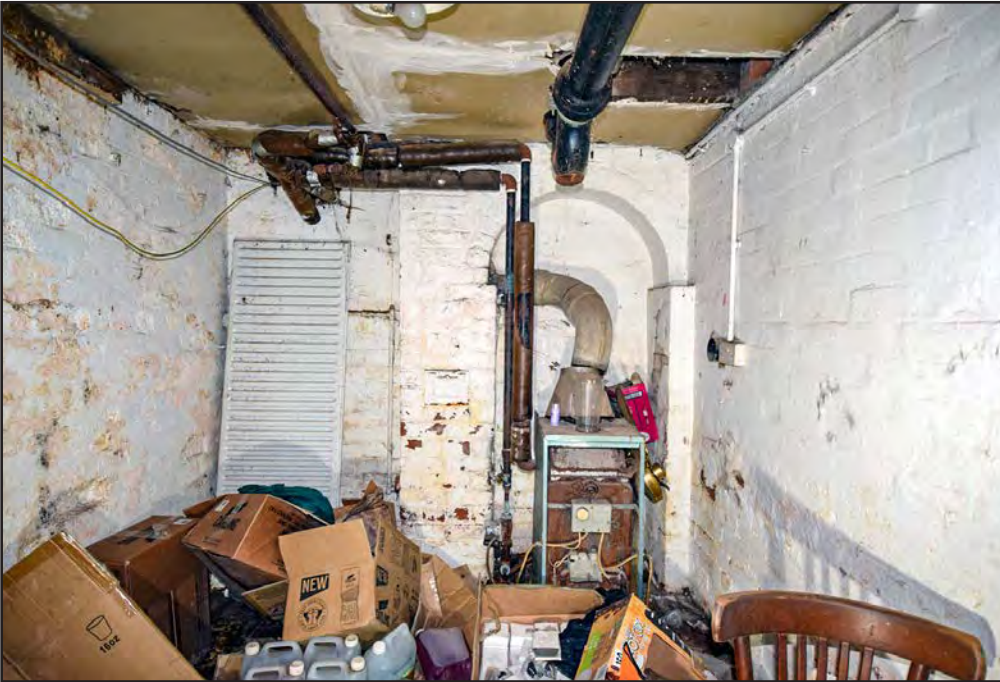
Plate 109: Basement room B4 looking north
