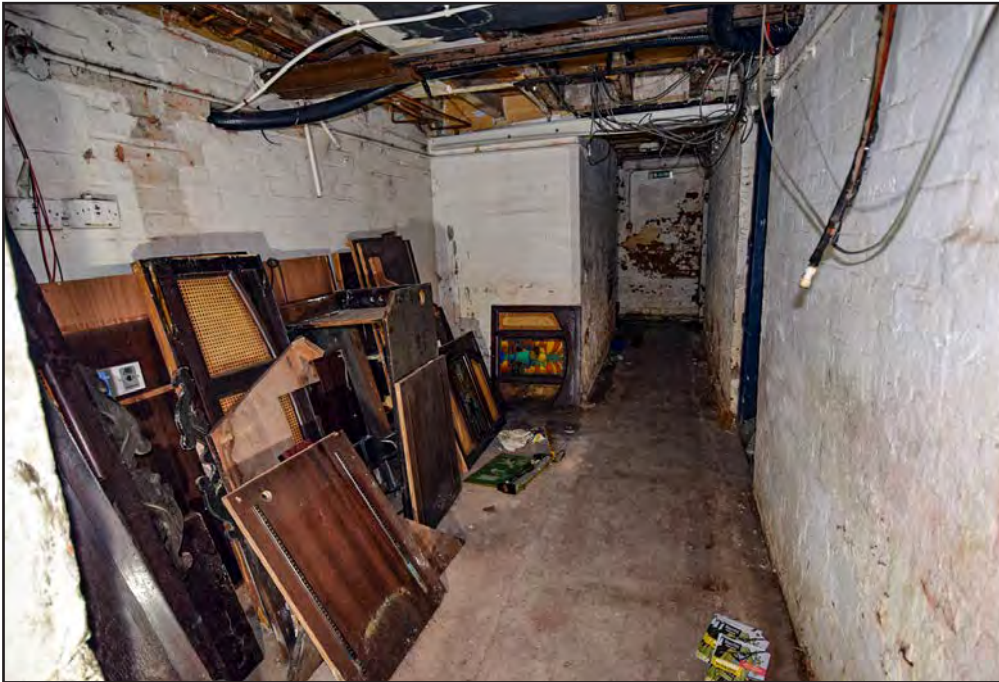
Plate 111: Basement corridor looking north
