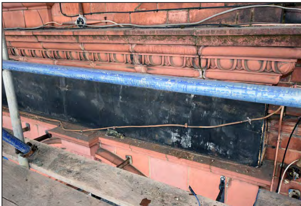
Plate 15: Detail of cornice at first floor level
