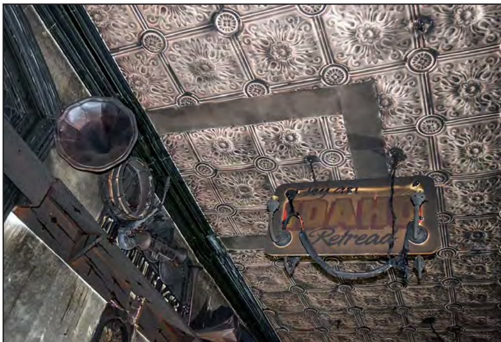
Plate 51: Scar in ceiling of former lobby to doorway from Banbury Street
