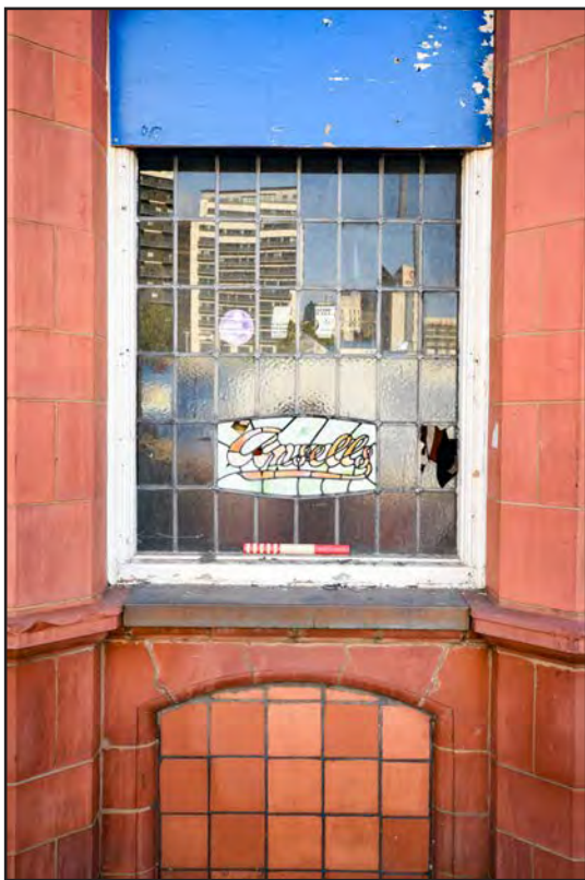
Plate 3: Detail of window facing New Canal Street
