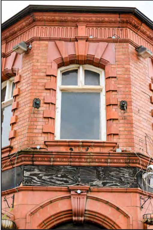
Plate 9: First floor window at street corner
