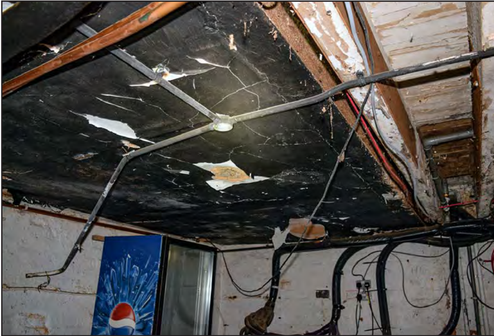
Plate 121: Underside of concrete floor on east side of Room B1
