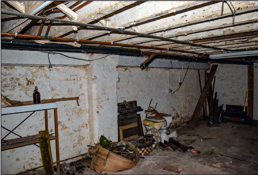
Plate 119: Room B1 looking north-west
