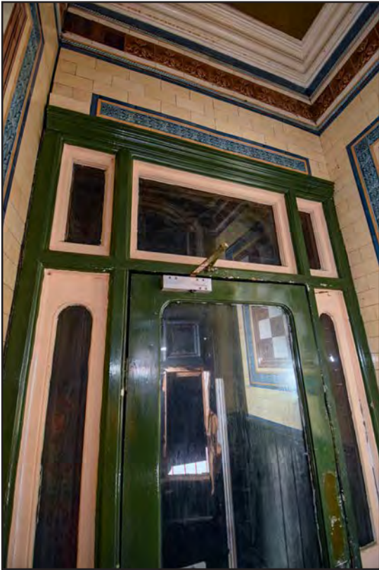
Plate 75: Entrance lobby from Banbury Street
