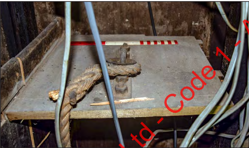
Plate 64: Top of box within dumb waiter
