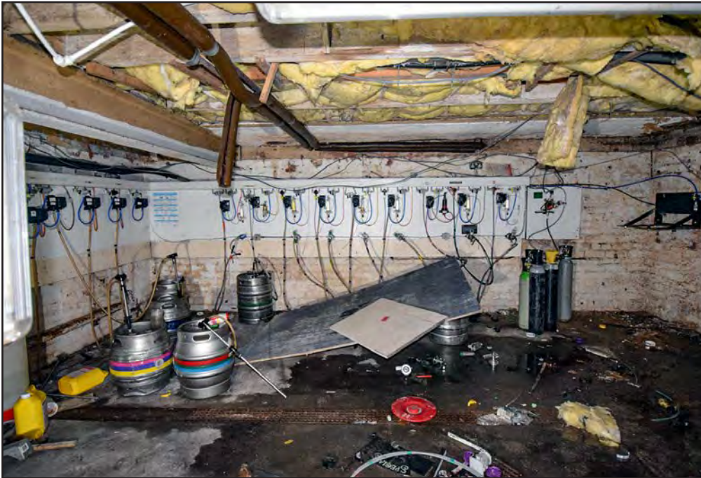
Plate 123: Room B2 looking west
