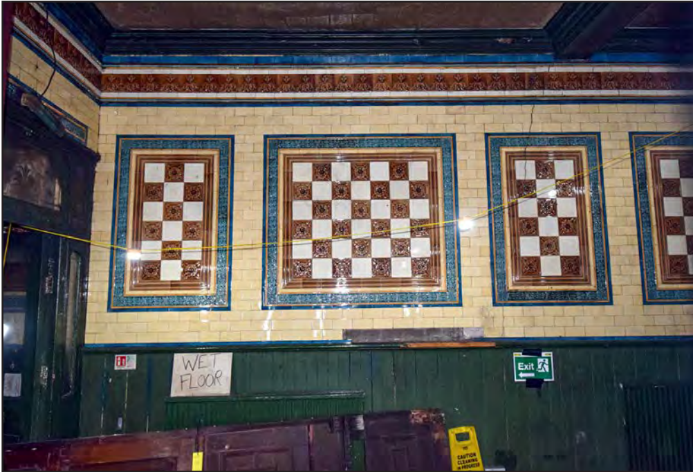
Plate 65: Glazed tiles to east wall (former corridor) after cleaning
