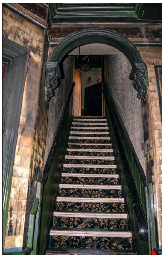
Plate 100: Main flight of stairs behind public bar
