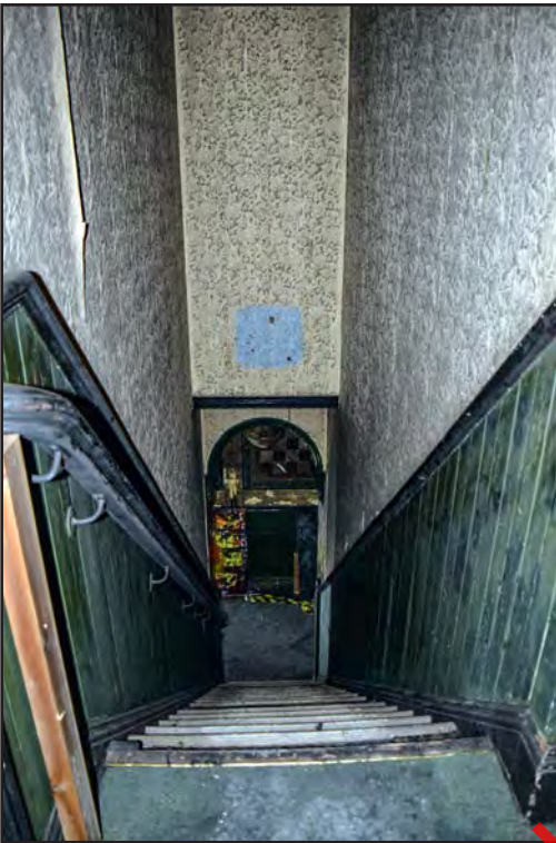
Plate 126: Looking down main stairs from first floor landing (F3)
