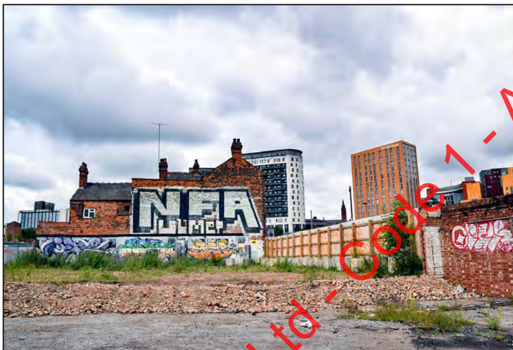
Plate 20: View of pub from east
