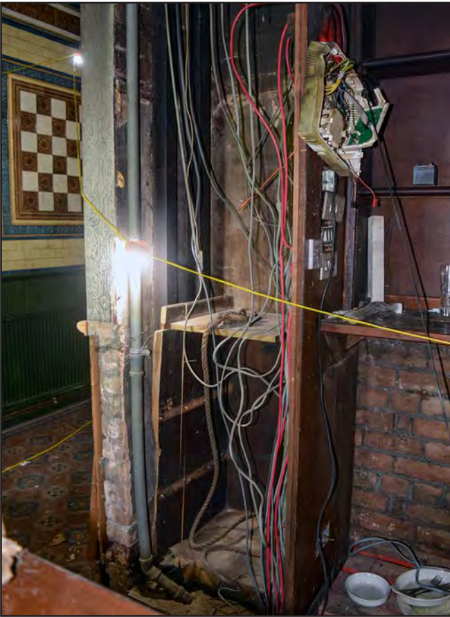
Plate 63: Dumb waiter after removal of front
