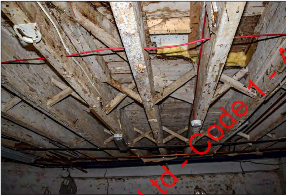
Plate 120: Herringbone struts in Room B1
