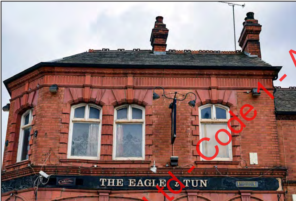
Plate 6: Upper windows facing New Canal Street
