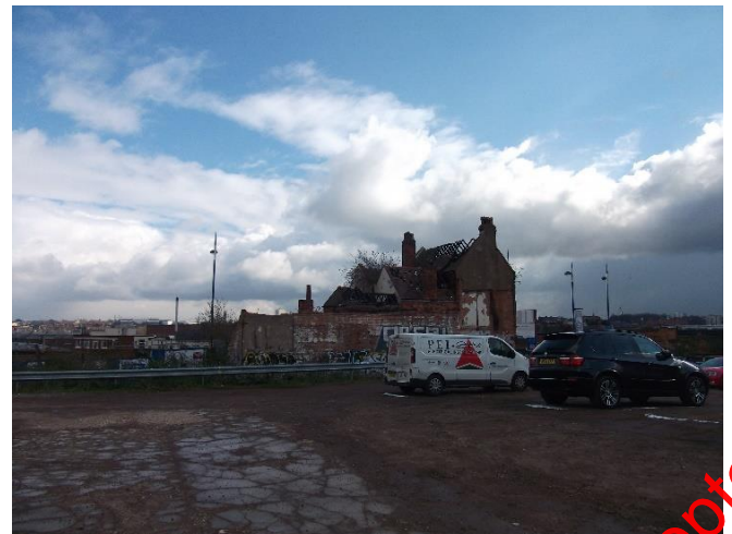
D: View of Fox and Grapes from the west of the Fox and Grapes showing an aspect of the building in its setting
