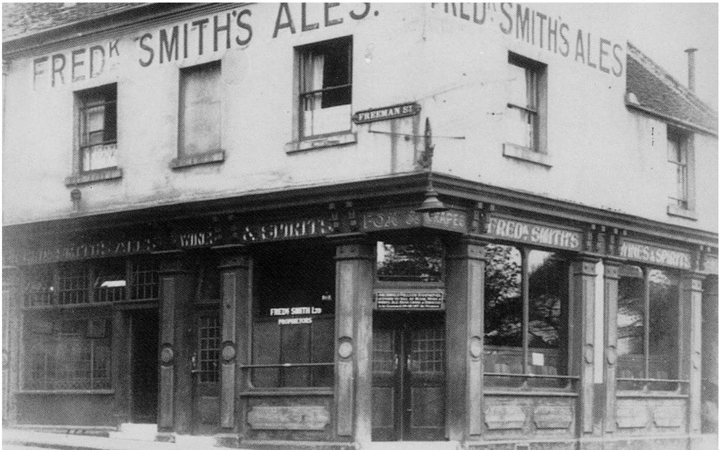
Photograph of Fox and Grapes under ownership of Frederick Smith Ltd, pre-1955 (source unknown)
