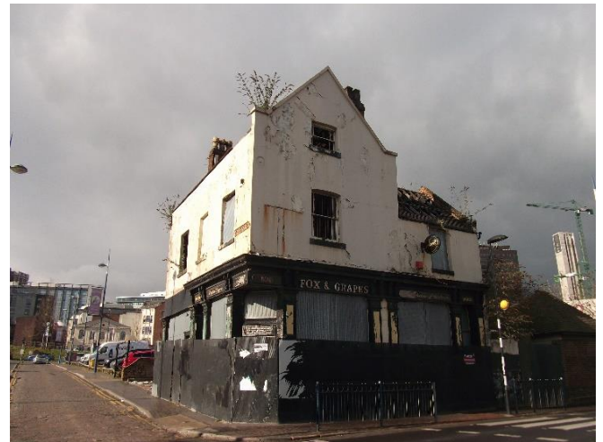
B: Fox and Grapes, Park Street (east) elevation, showing the relationship with Freeman Street and its cobbled surface, 2018
