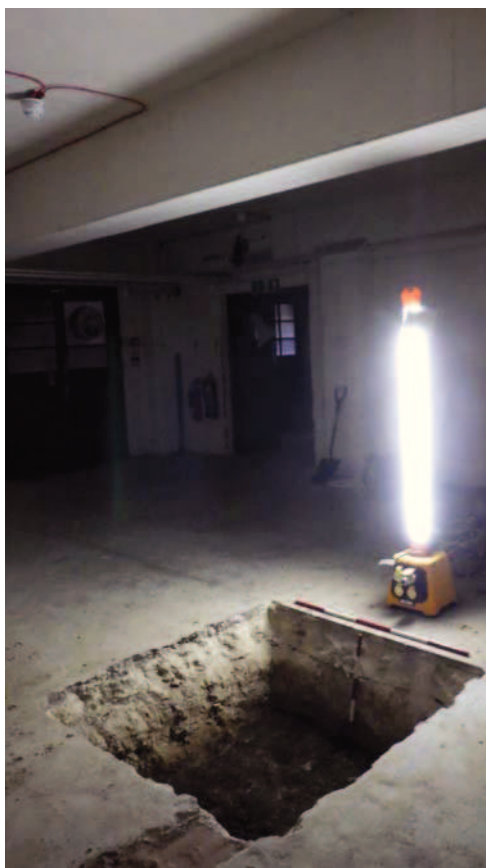
Plate 1: The excavation of Test Pit 1 within the basement of the site
