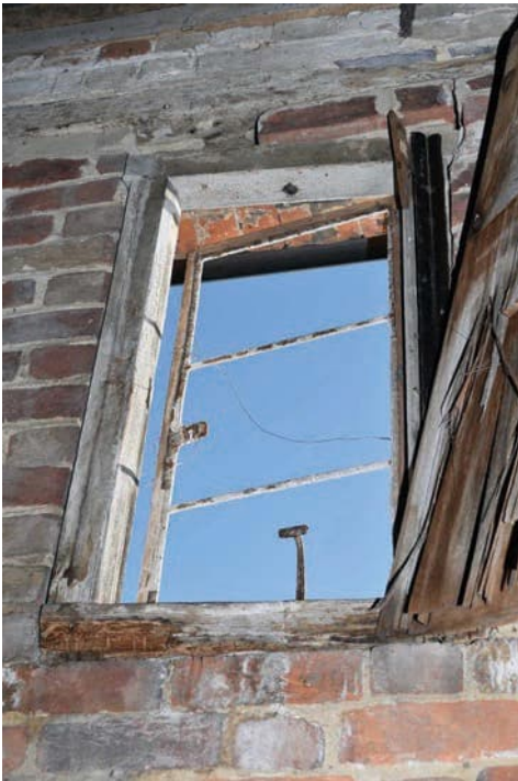
Photo B 88: Window details upper storey south wall
