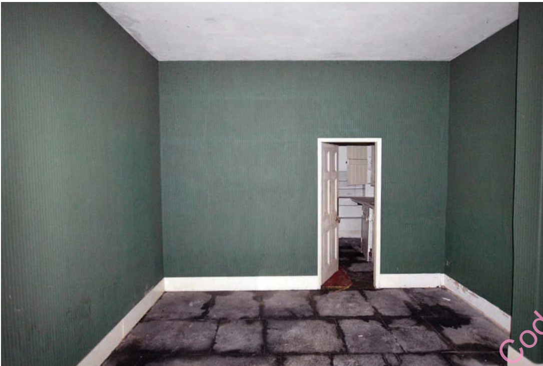
Photo B 31: Room to rear G1 looking towards the kitchen G5
