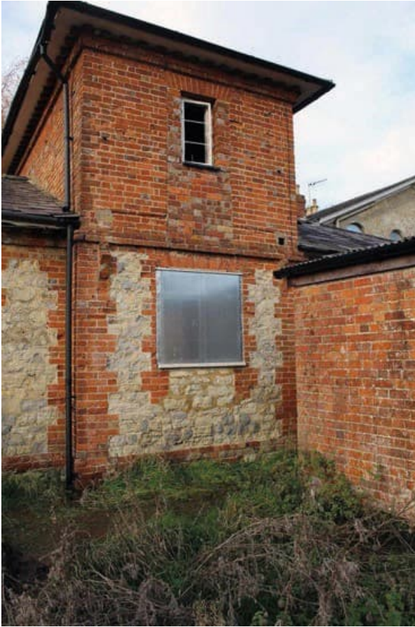
Photo B 71: Front, south elevation of 2-storey central element
