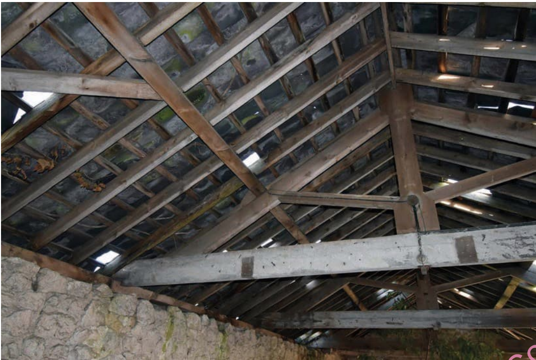
Photo B 120: Detail of roof structure
