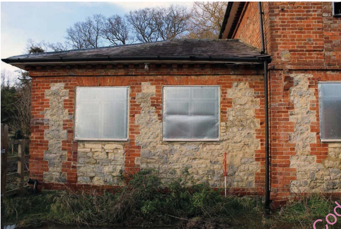
Photo B 70: Western part of south, front elevation
