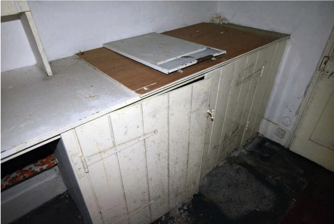
Photo B 43: Cupboards alongside east wall in kitchen G5
