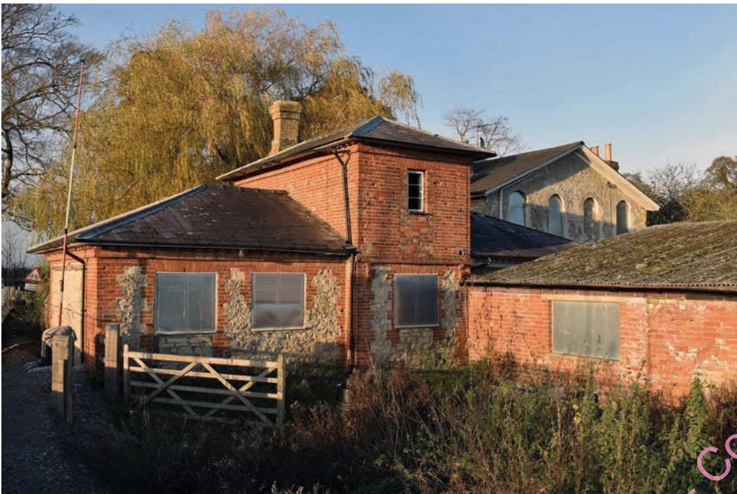
Photo B 68: Front elevation dairy-yard
