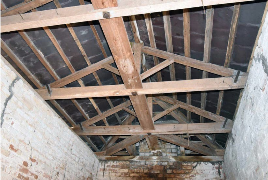
Photo B 89: Roof structure over central bay looking north
