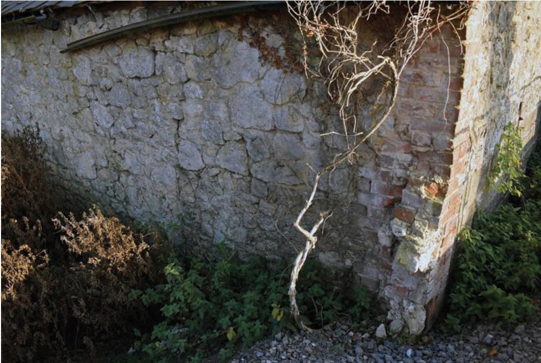
Photo B 111: North-western corner showing bonding to boundary wall (removed).
