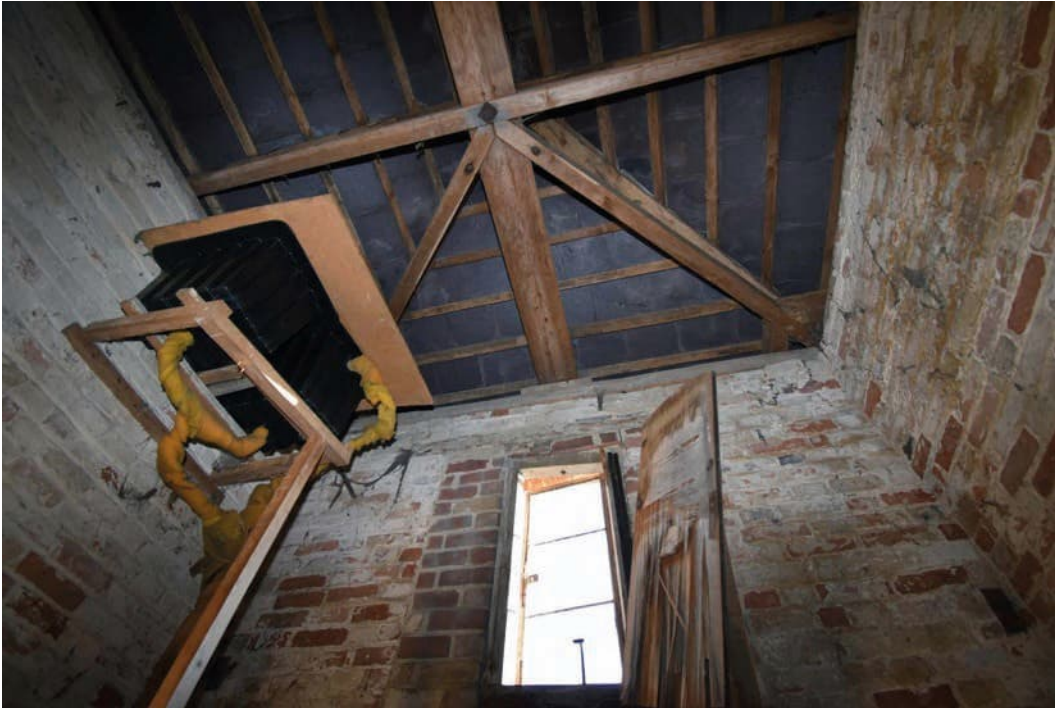
Photo B 87: Window inserted into loading bay, upper storey south wall
