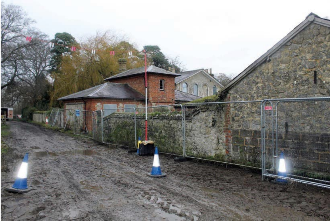
Photo B 123: Boundary wall, general aspect looking north east towards Oxford Road
