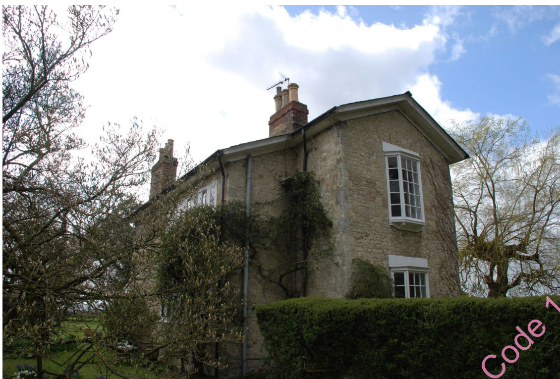
Photo 19: North east aspect, 2017
