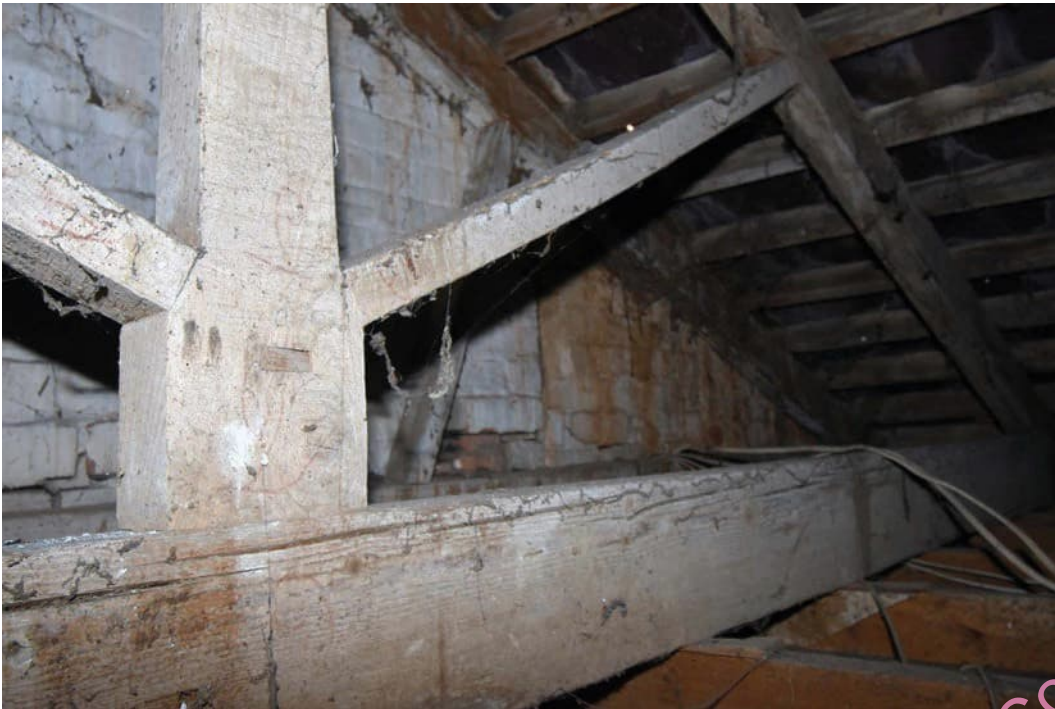
Photo B 92: Roof structure over western bay
