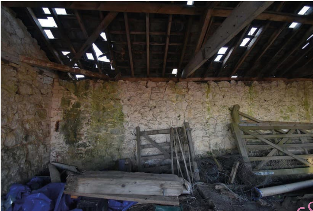
Photo B 116: Interior face of north wall, west end
