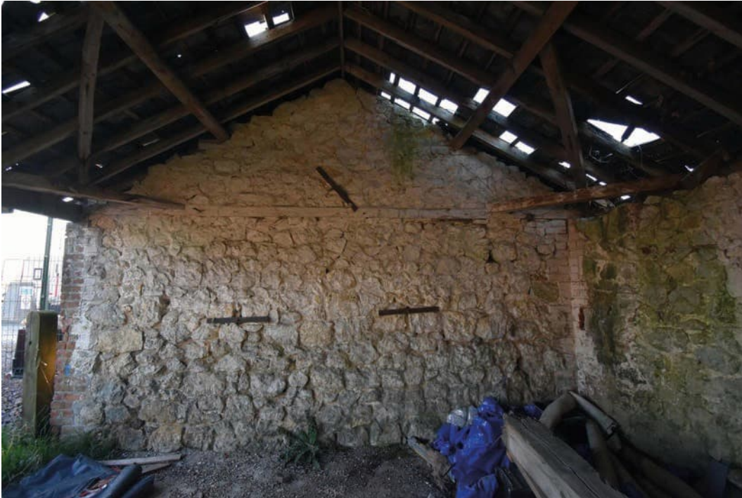
Photo B 115: Interior west wall
