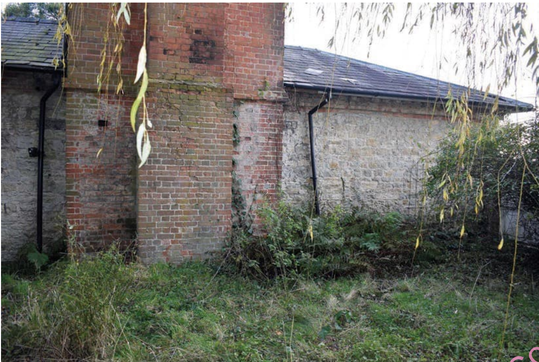
Photo B 78: Rear elevation, central and west bays
