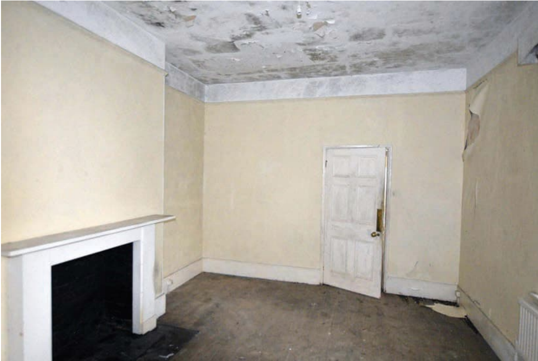
Photo B 28: Front room G2 looking to the rear
