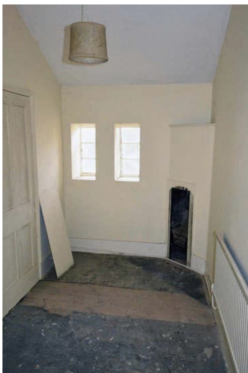
Photo B 62: East internal elevation to small bedroom F3
