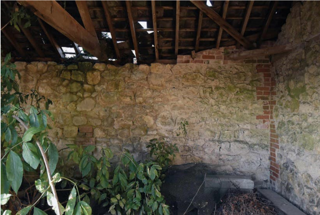
Photo B 117: Interior face of north wall, east end
