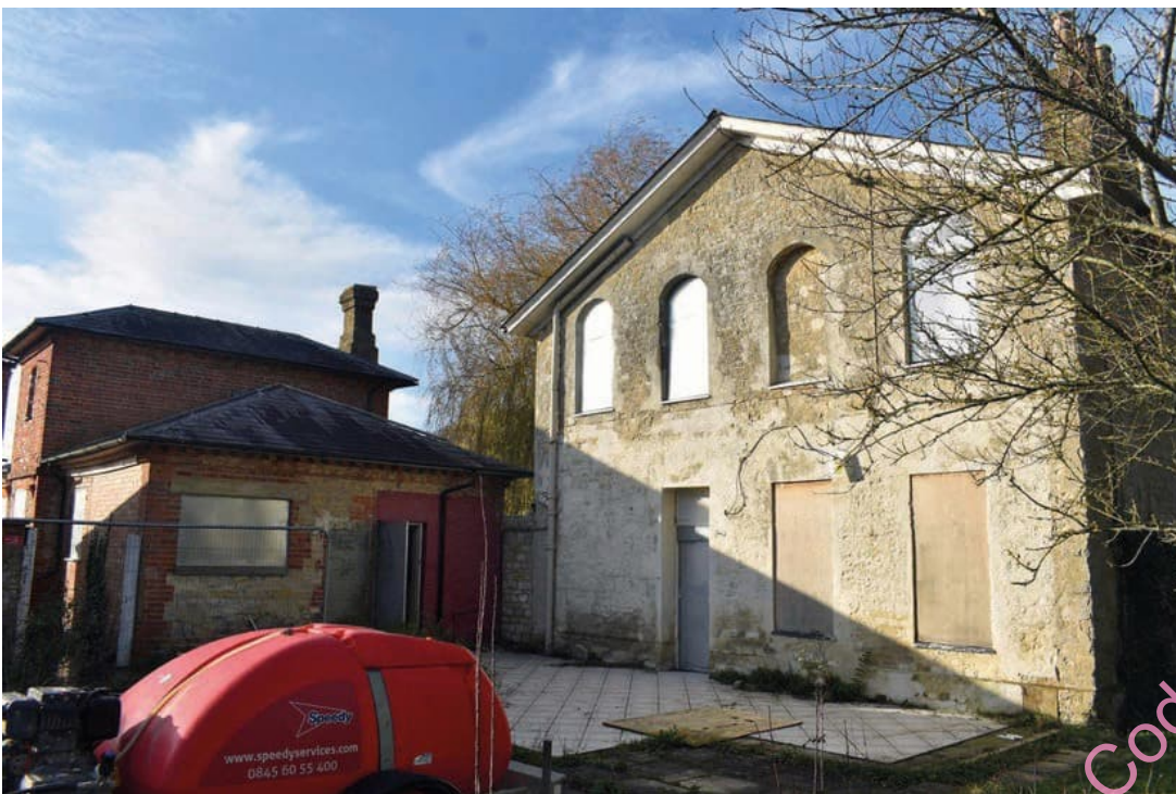
Photo B 21: South (rear) elevation looking to north west towards dairy
