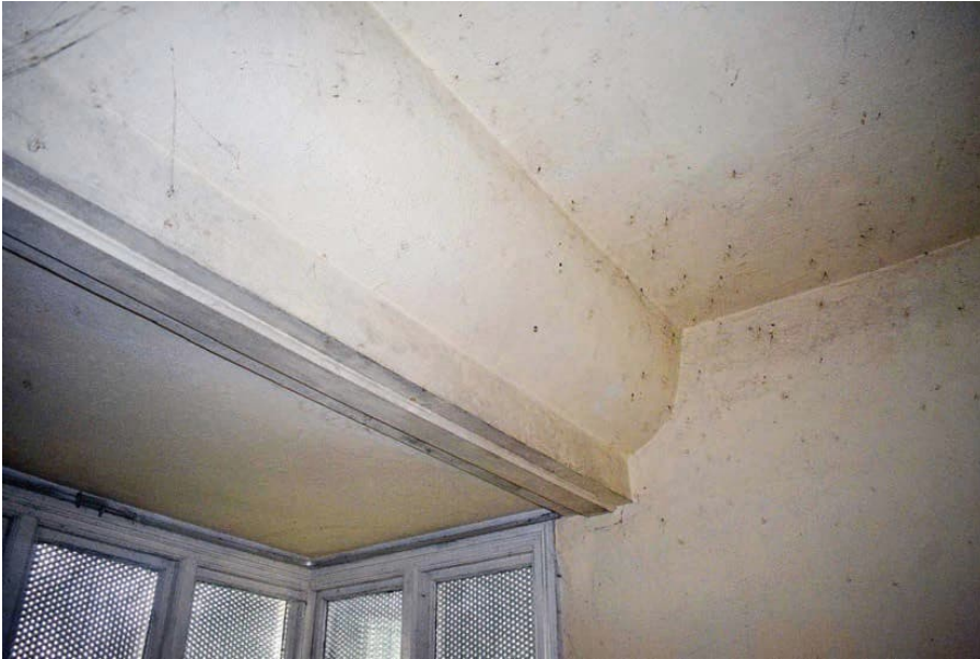
Photo B 49: Ceiling cornice detail over west bay window G4
