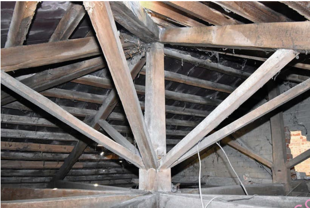
Photo B 90: Roof structure over eastern bay
