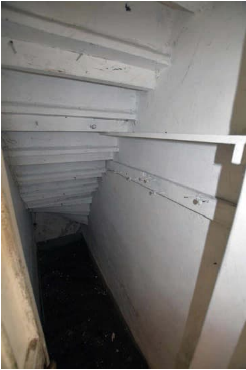
Photo B 26: Under stairs space
