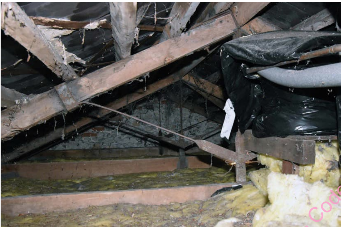
Photo B 66: Structural detail of roof truss
