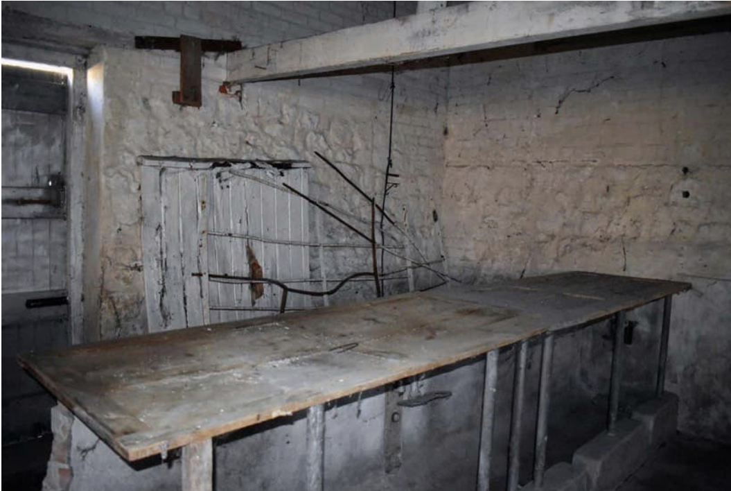
Photo B 103: Reused doors forming bench over the cattle trough
