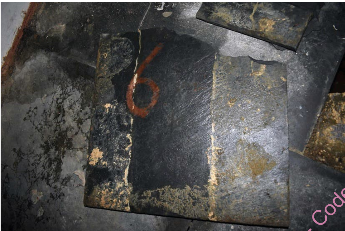
Photo B 37: Number marked on back of slate flooring in rear room G1
