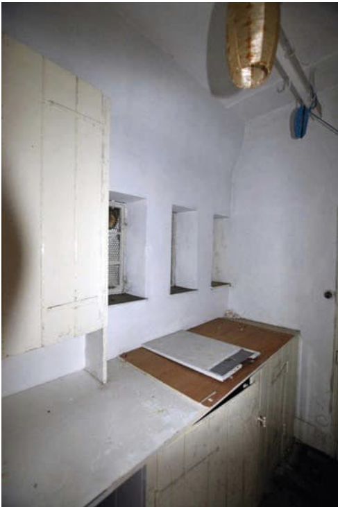
Photo B 39: East elevation to kitchen G5 from the north
