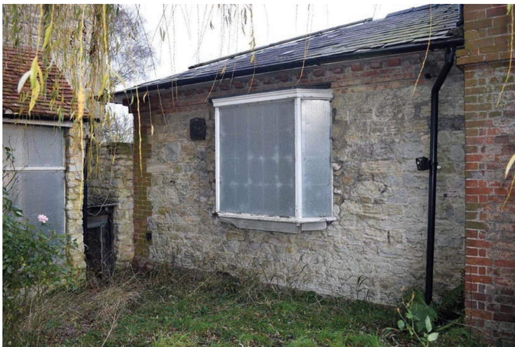
Photo B 79: Rear elevation east bay
