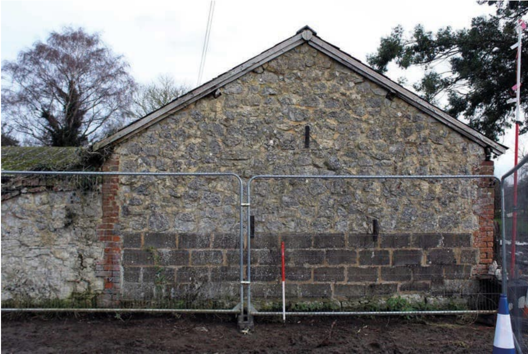
Photo B 109: West gable elevation to trackway
