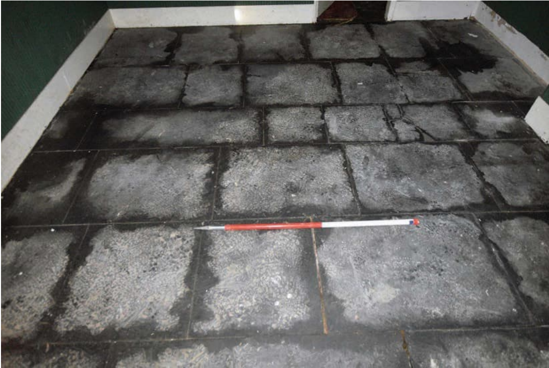
Photo B 34: Slate floor within the rear room G1
