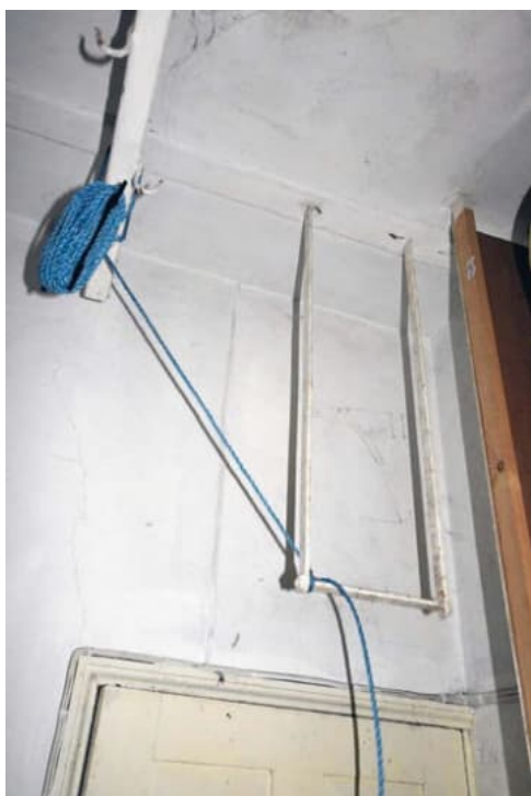
Photo B 42: Hanging rail with hooks and bracket within kitchen ceiling, G5
