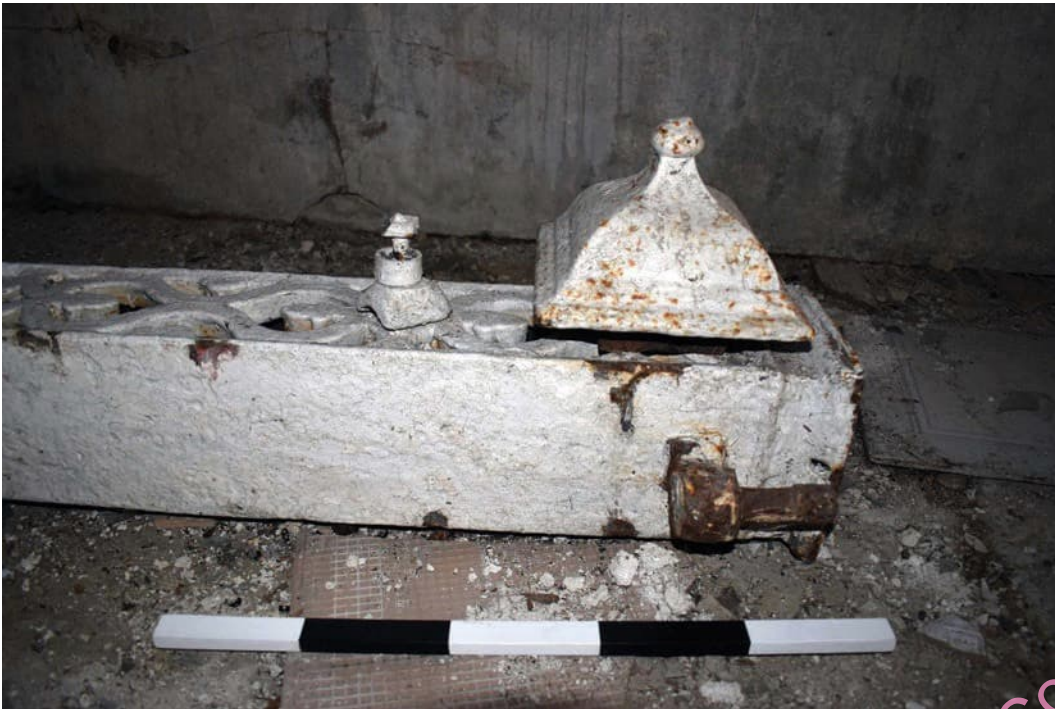
Photo B 128: Decorative finial to Oxford Road gate pier with fixing bolt and pintle
