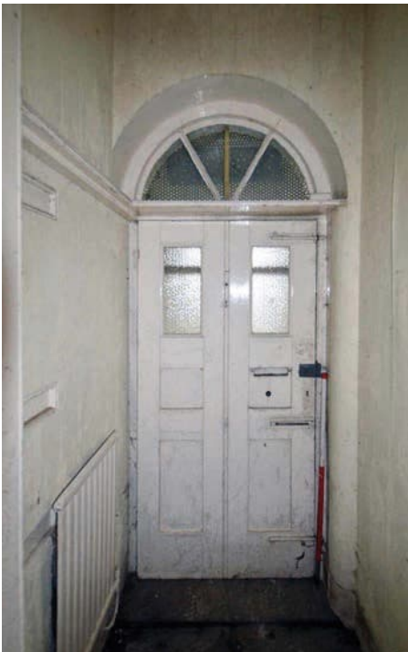
Photo B 23: Interior of front doorway
