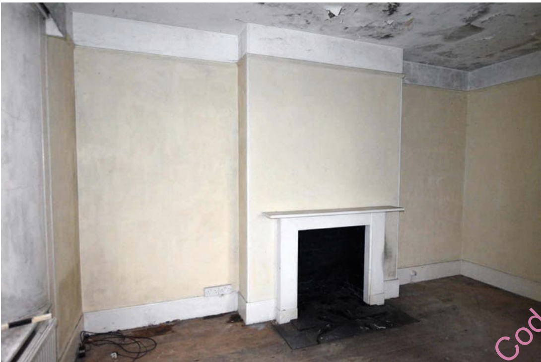
Photo B 29: Fire place within front room G2
