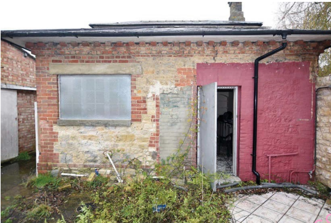
Photo B 76: East elevation
