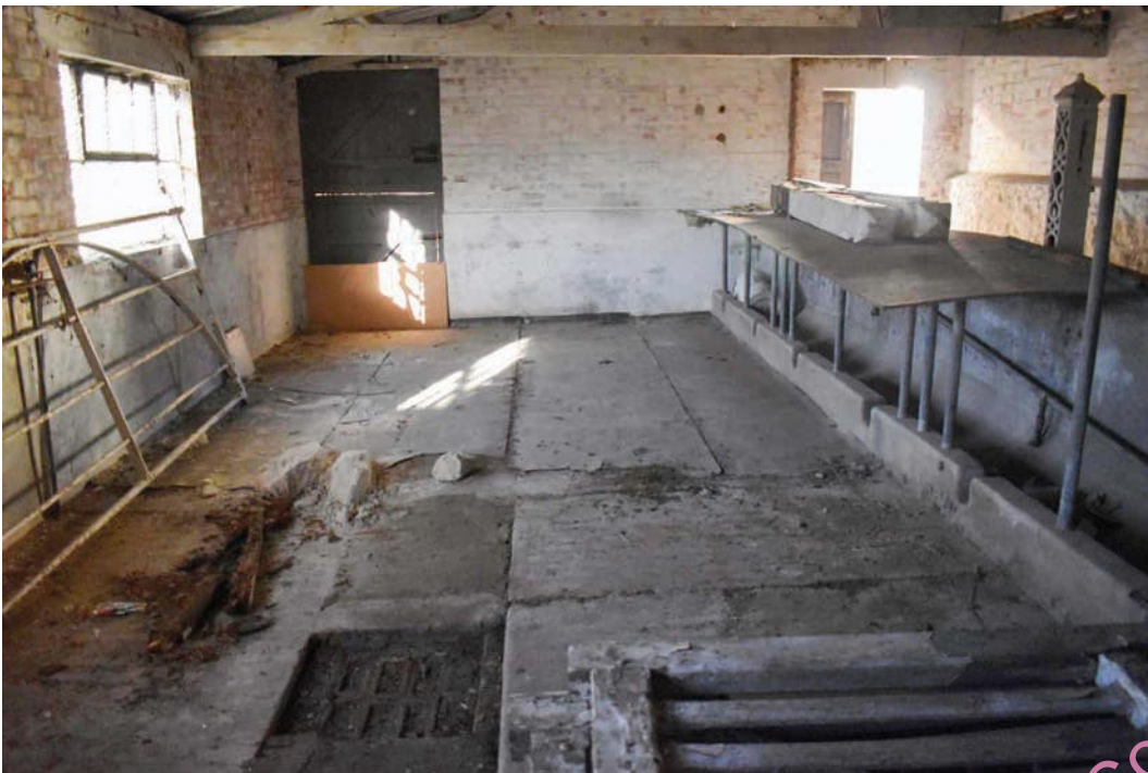
Photo B 106: Floor structure looking north
