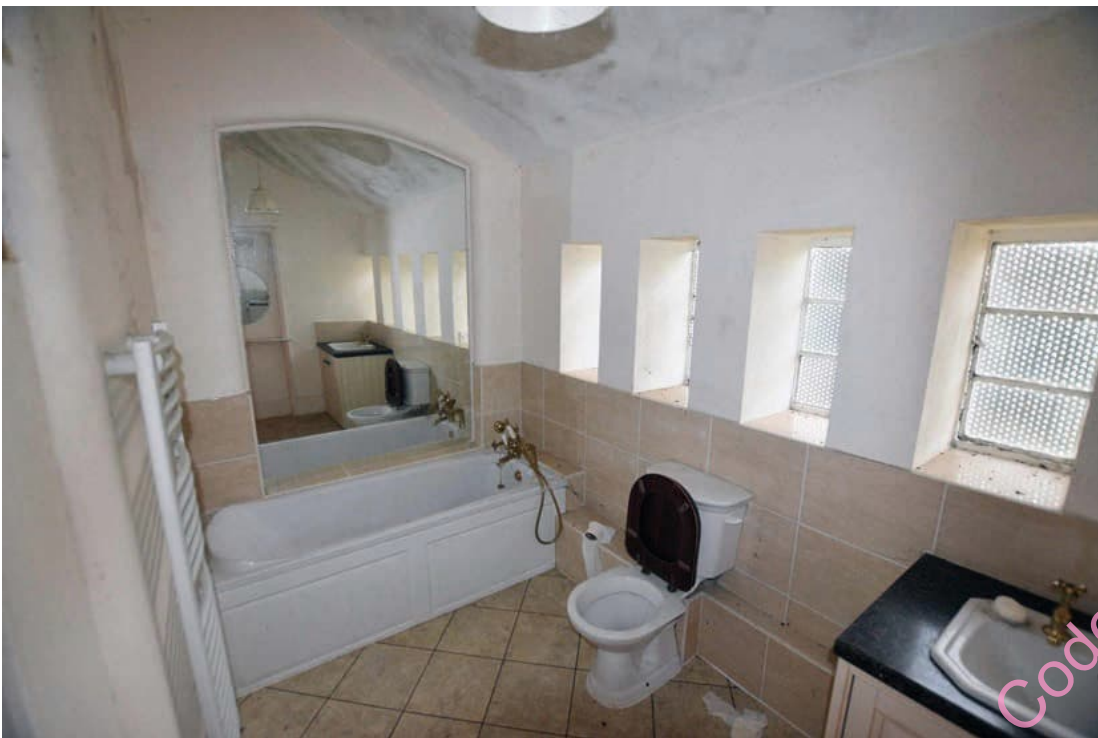
Photo B 58: First floor bathroom F4 alongside east elevation
