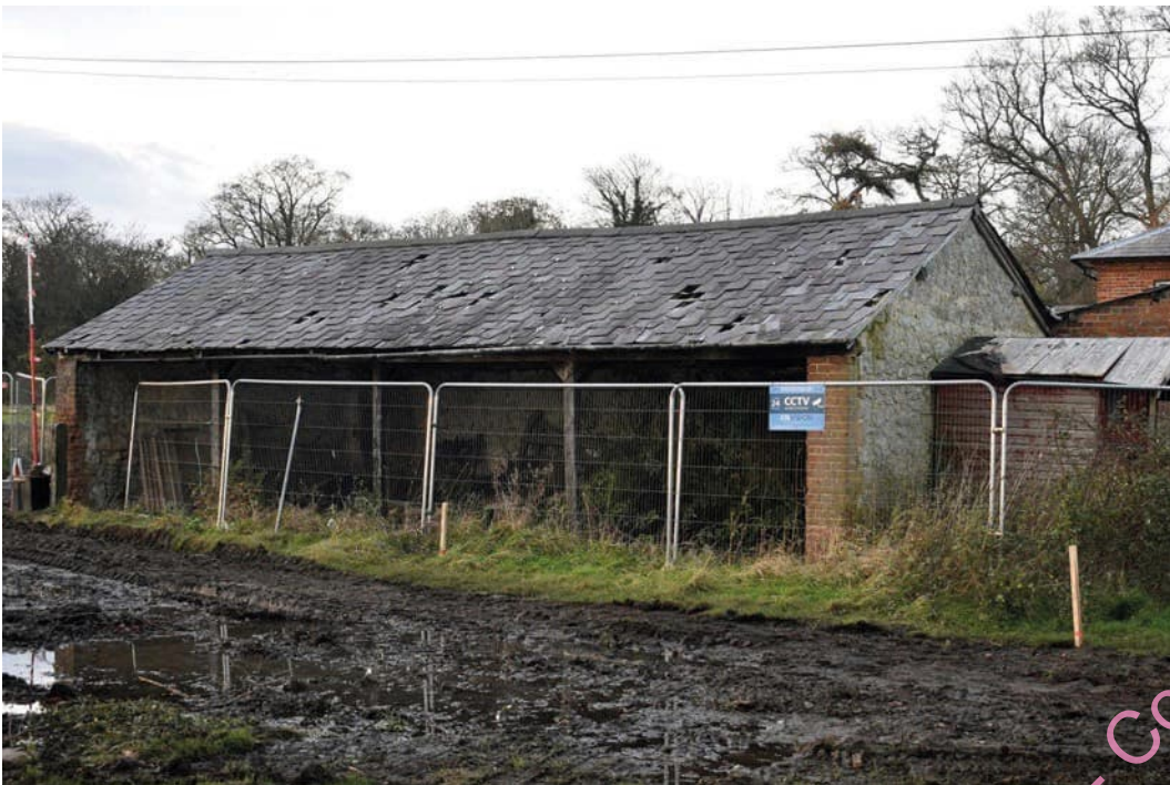
Photo B 108: South, front elevation
