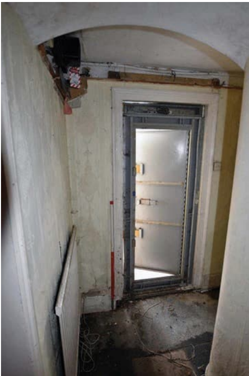
Photo B 25: Rear doorway from within hallway
