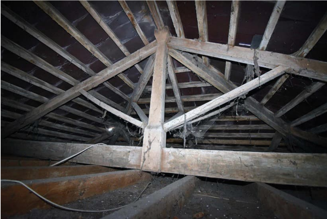
Photo B 91: Roof structure over western bay
