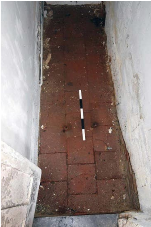
Photo B 27: Tiled floor in space beneath stairs
