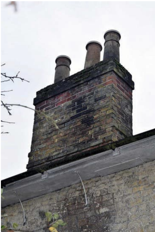
Photo B 19: Chimney stack on east elevation
