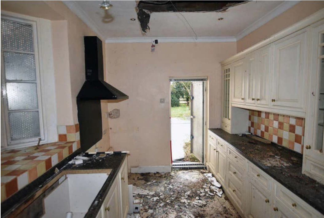
Photo B 81: East kitchen area G6 looking out to east
