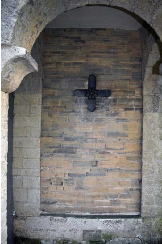
Photo B 14: Secondary stone skin to south side of porch
