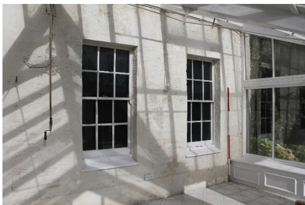
Photo 23: Ground floor windows, rear elevation 2017
