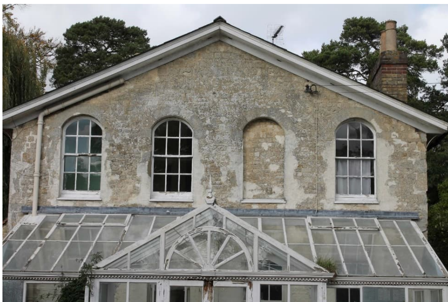
Photo 22: South, rear elevation, first floor openings, 2017
