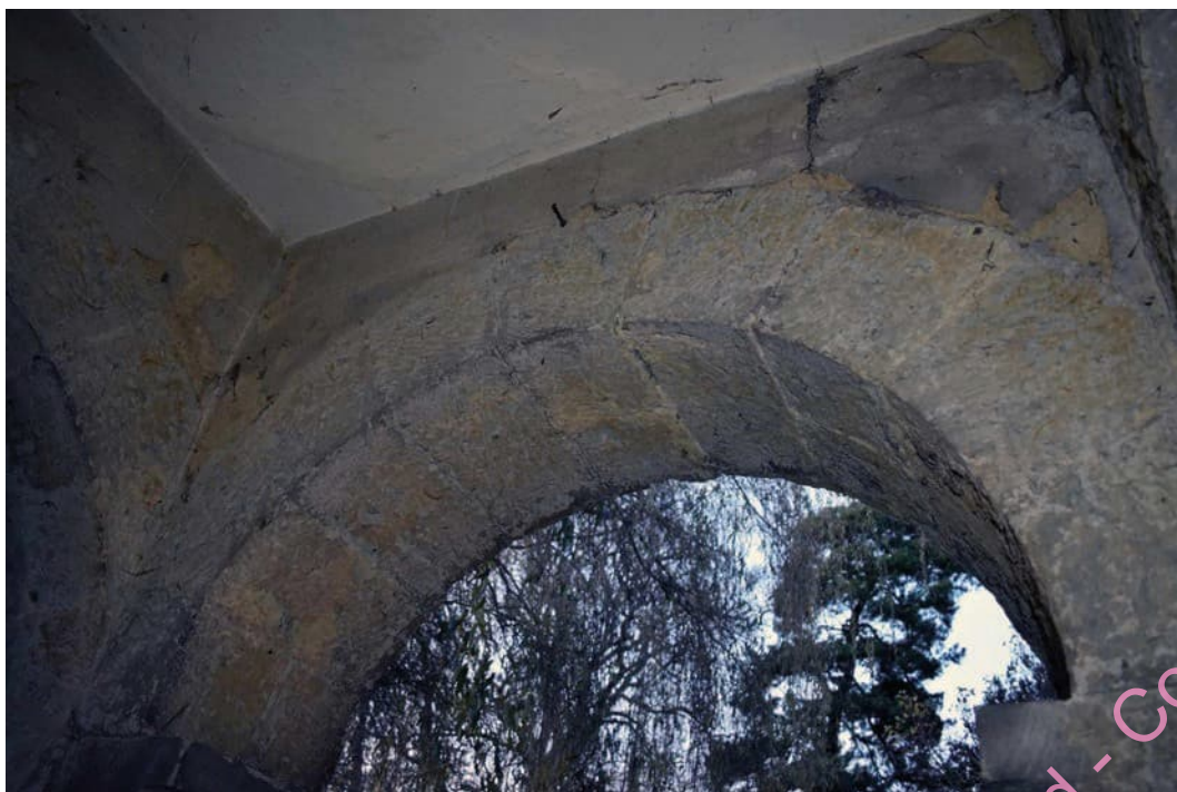
Photo B 13: Arch details to entrance porch
