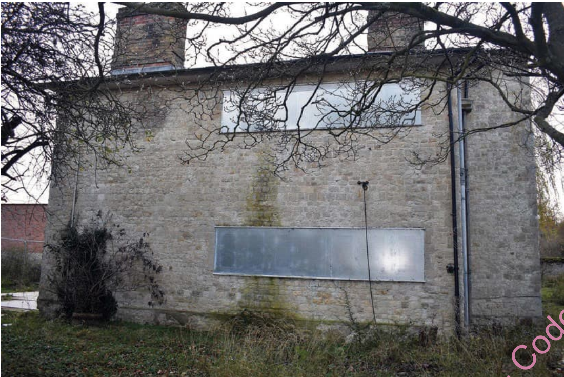
Photo B 17: East elevation
