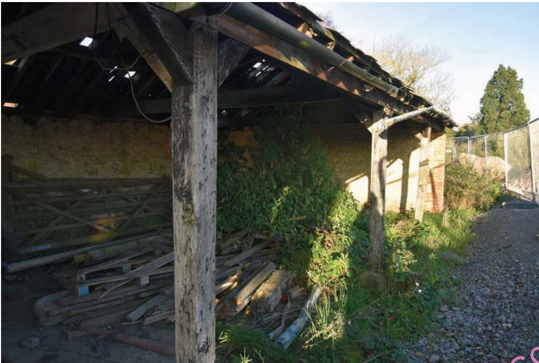
Photo B 112: South, front facing elevation
