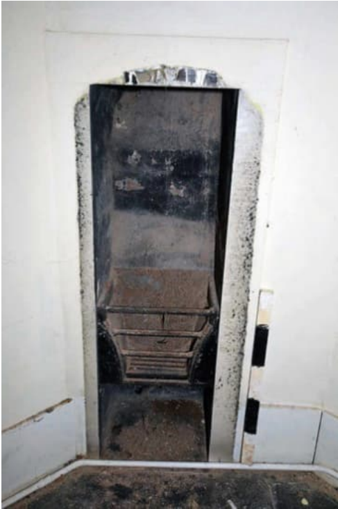
Photo B 63: Small fireplace in corner of bedroom F3
