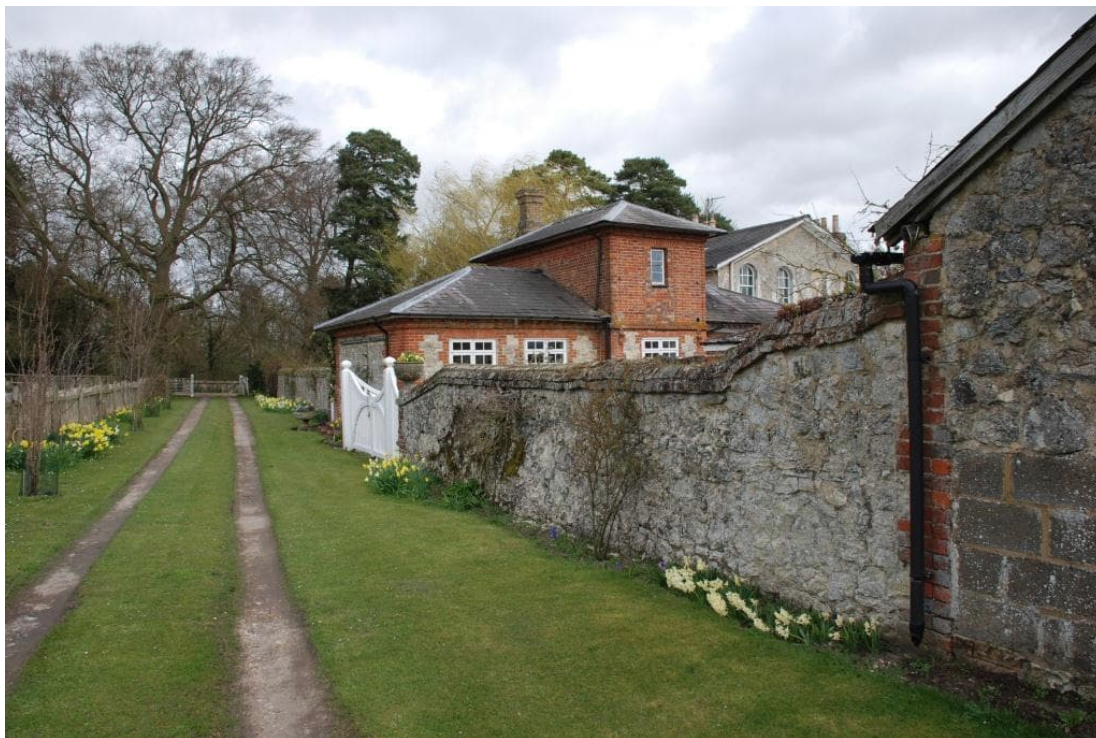
Photo 3: Access track looking north, 2017
