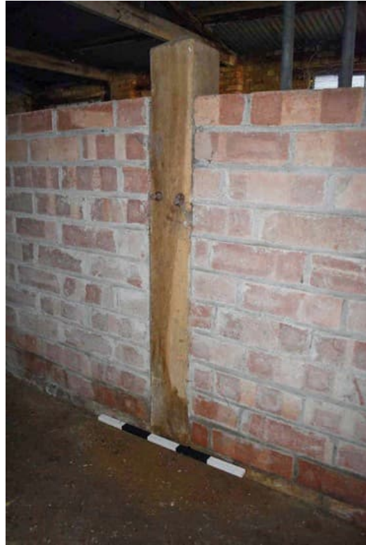
Photo B 101: Brick built rear face of the cattle trough with timber division
