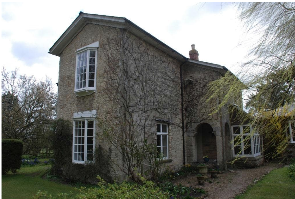
Photo 18: Front, north elevation 2017
