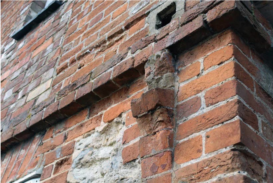
Photo B 73: Truncated bracket from platform to loading door, south elevation
