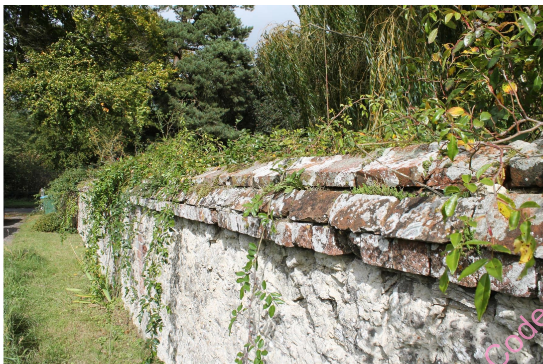
Photo 6: Boundary wall alongside front garden, 2018
