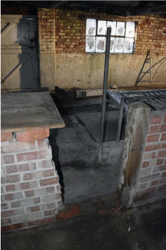
Photo B 101: Brick built rear face of the cattle trough with timber division
