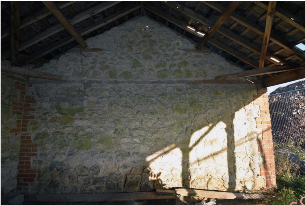
Photo B 118: Interior face of east wall
