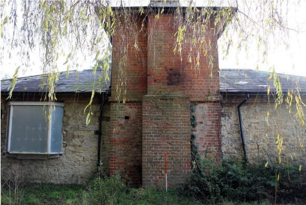
Photo B 77: North, rear elevation facing the front (west side) gardens
