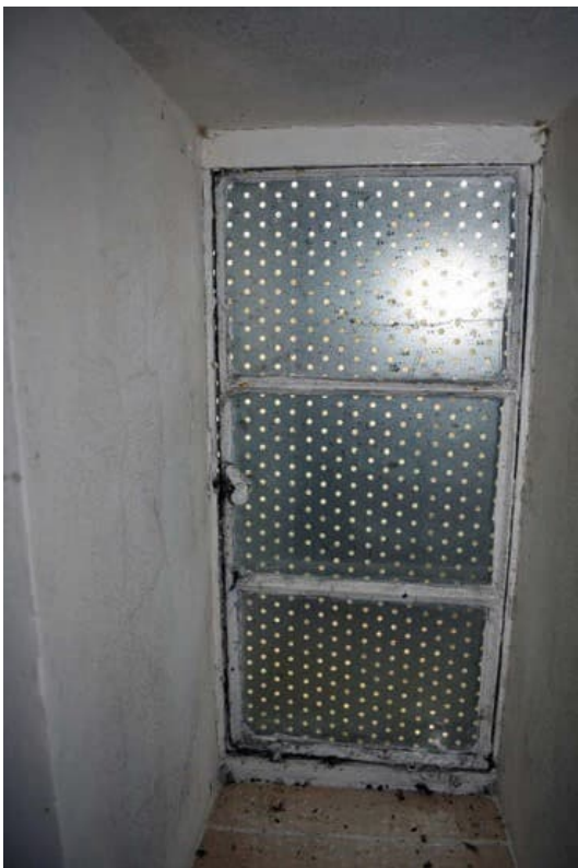
Photo B 59: Window detail to bathroom F4
