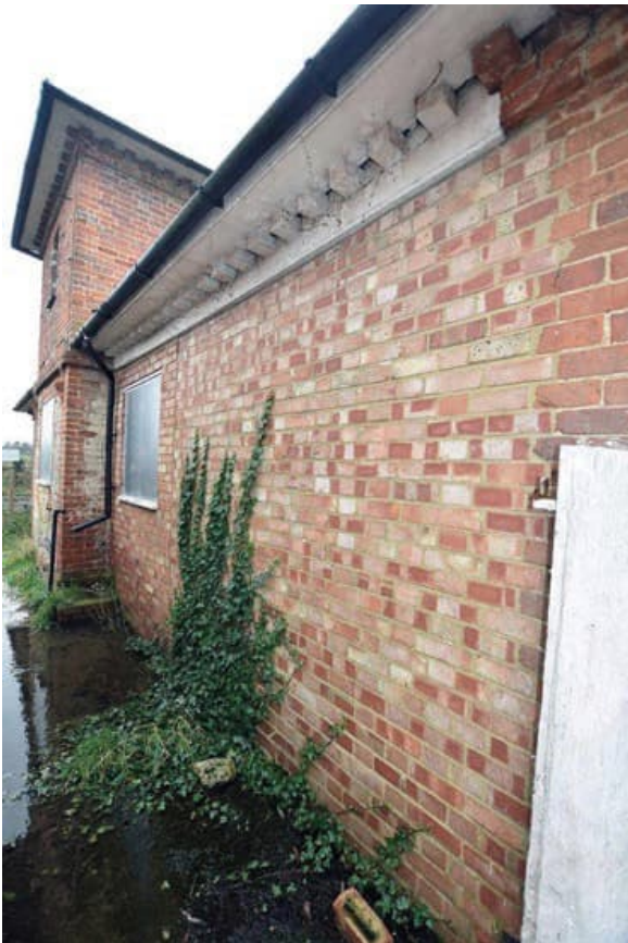
Photo B 74: Eastern end of south elevation showing modern brick infill
