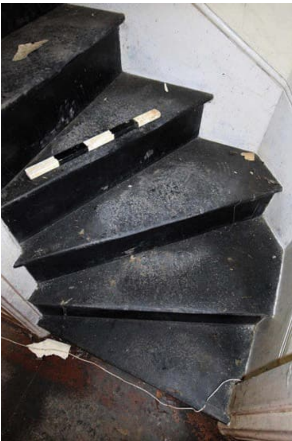
Photo B 50: Lower treads of slate stairs
