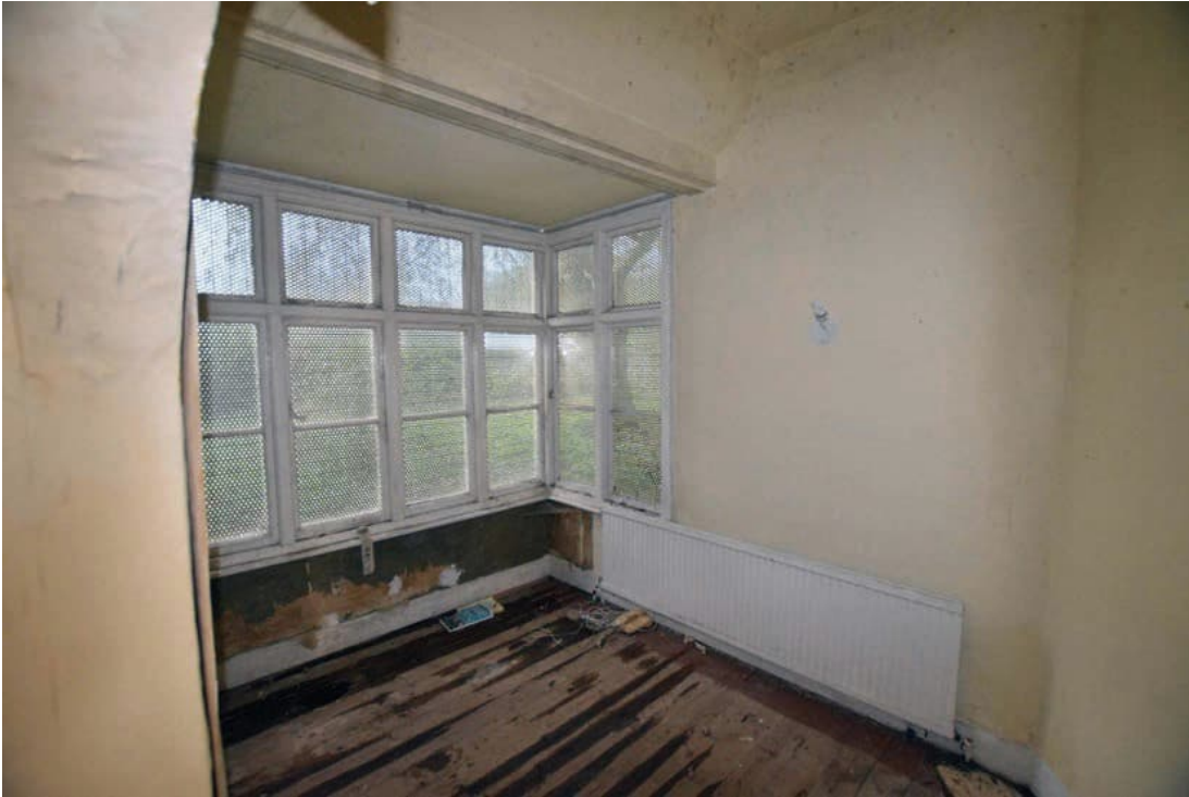
Photo B 45: Interior of western bay G4 showing corbelled ceiling detail
