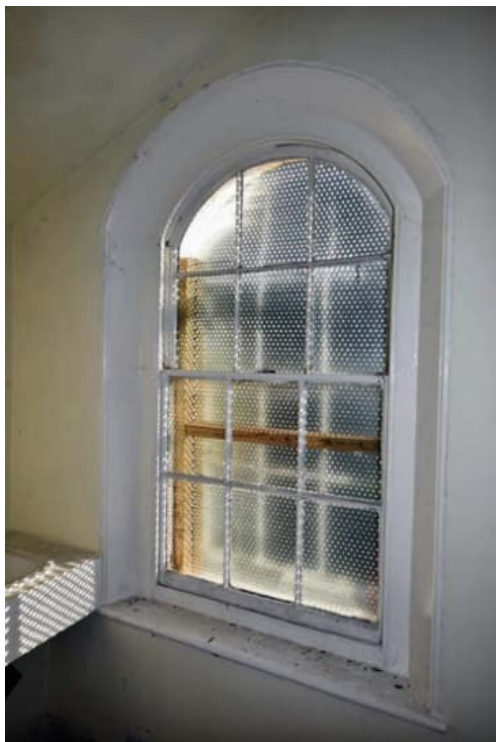
Photo B 61:Rear window in bedroom F2
