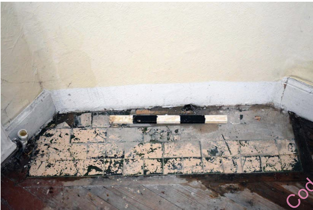
Photo B 48: Tiled hearth within west bay G4
