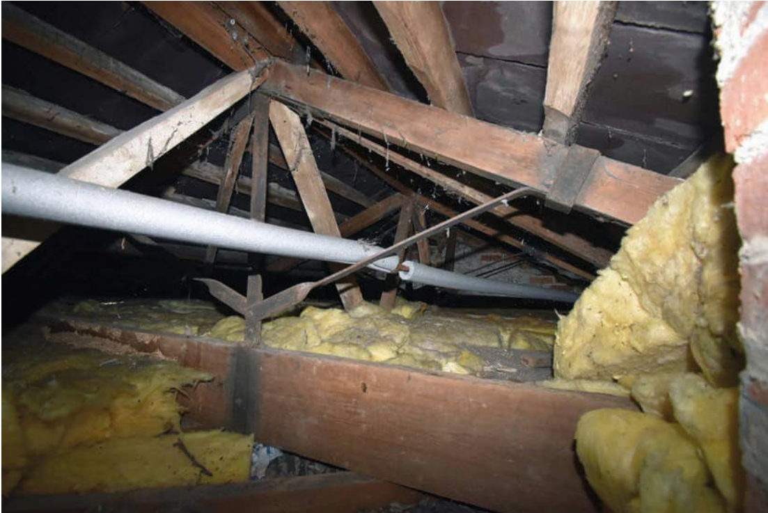
Photo B 65: Roof structure looking to the rear
