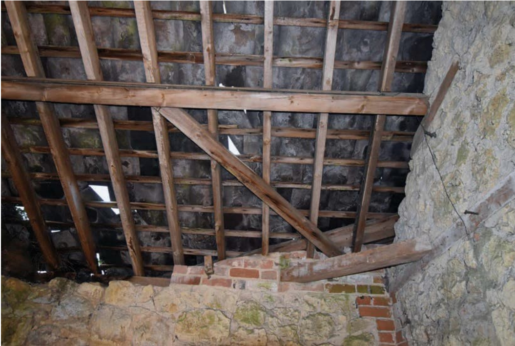
Photo B 121: Braces to north-eastern corner
