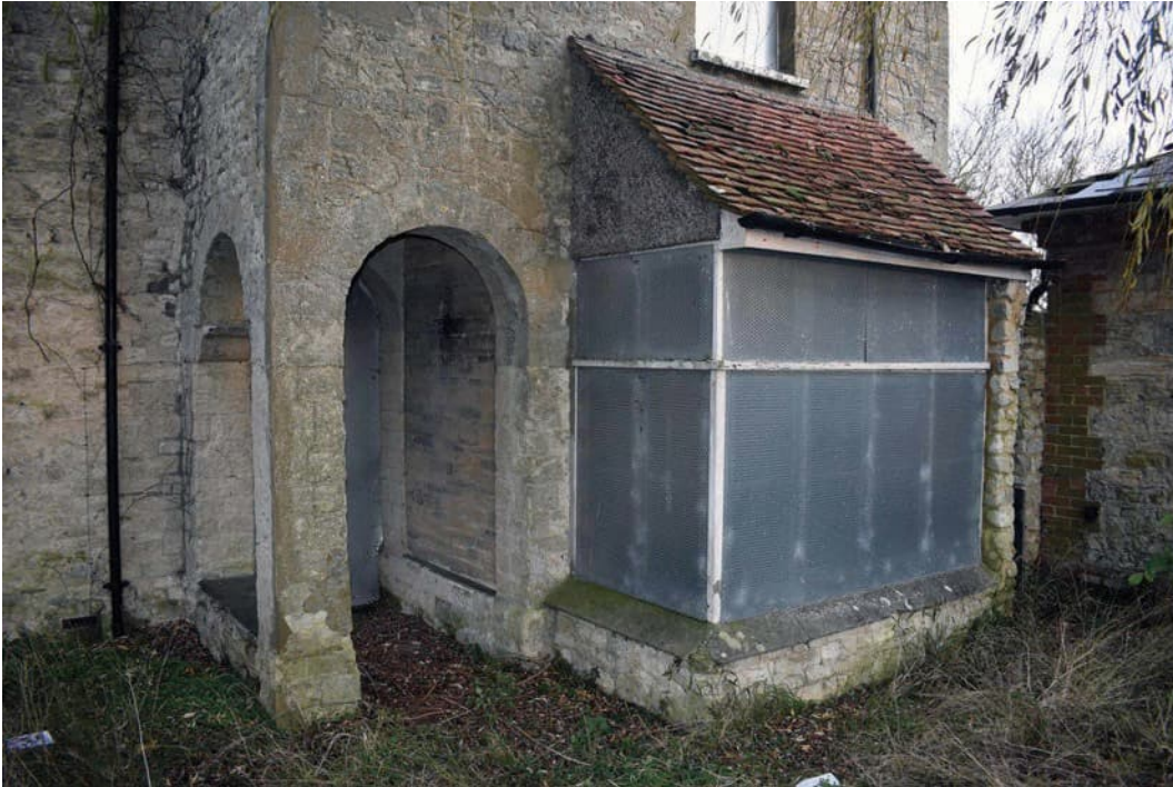
Photo B 11: West elevation with entrance porch and secondary bay
