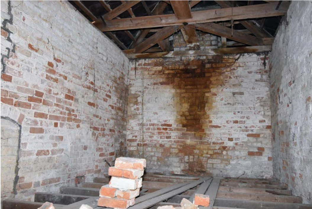
Photo B 85: Upper space within central bay looking north
