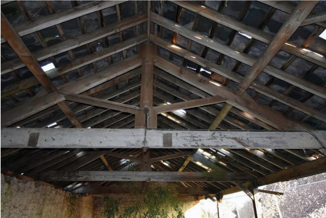
Photo B 119: Roof structure facing east
