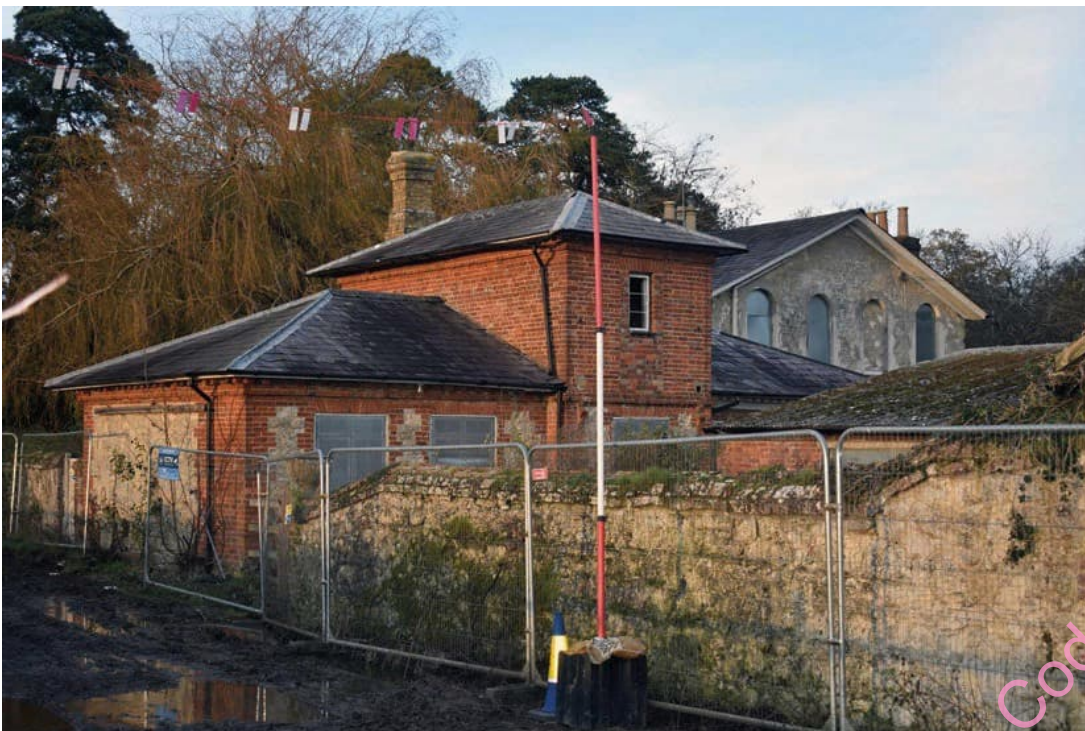
Photo B 4: Boundary wall looking north east towards dairy
