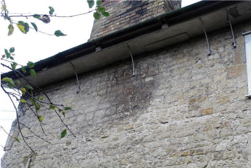
Photo B 18: Eaves brackets to east elevation
