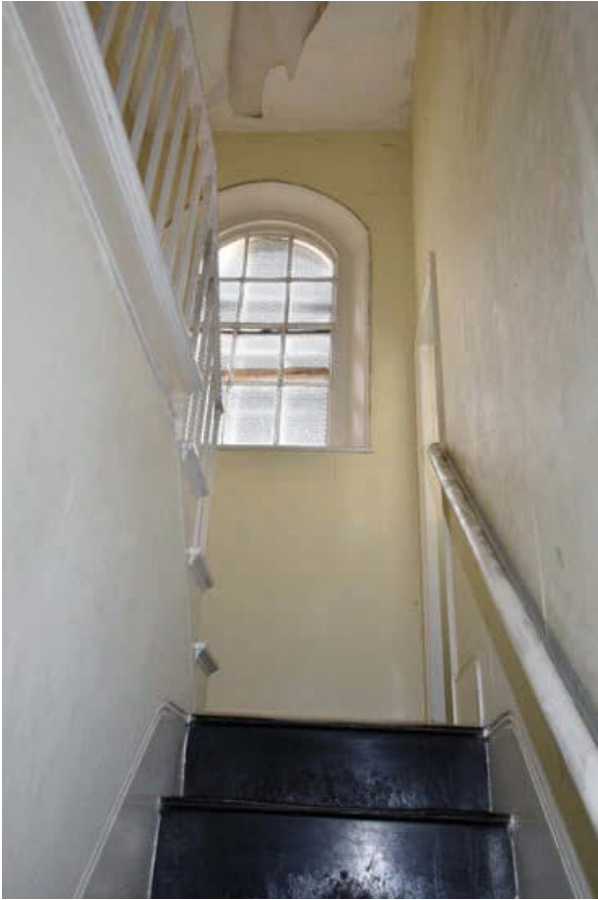
Photo B 51: Looking up stairs towards half-landing
