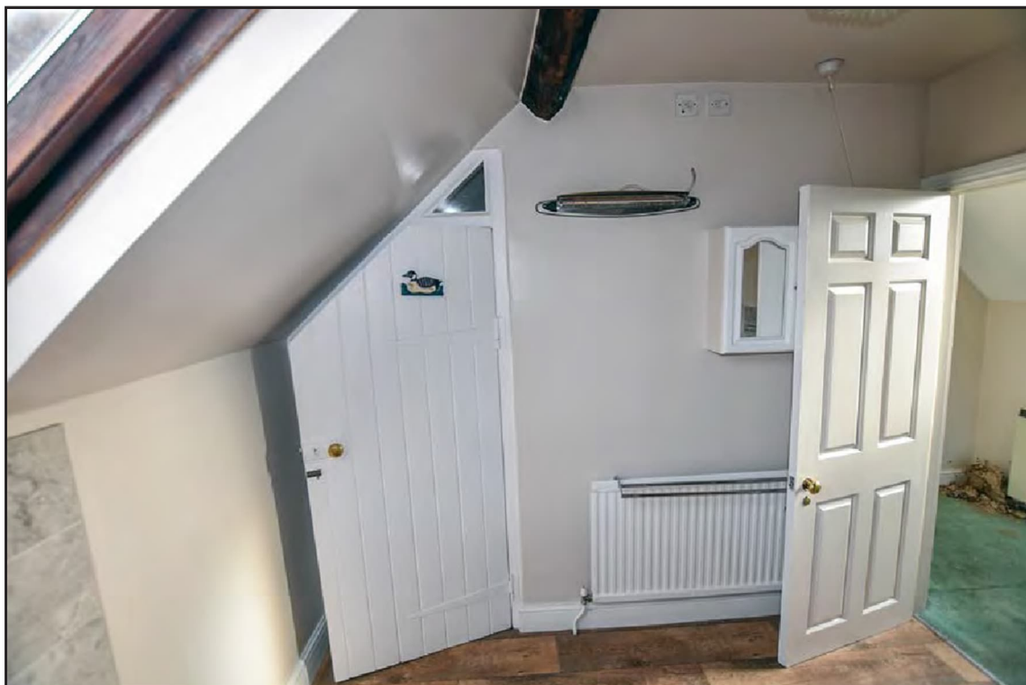
Photo A- 47: Bathroom F5 rear extension showing door to stair
