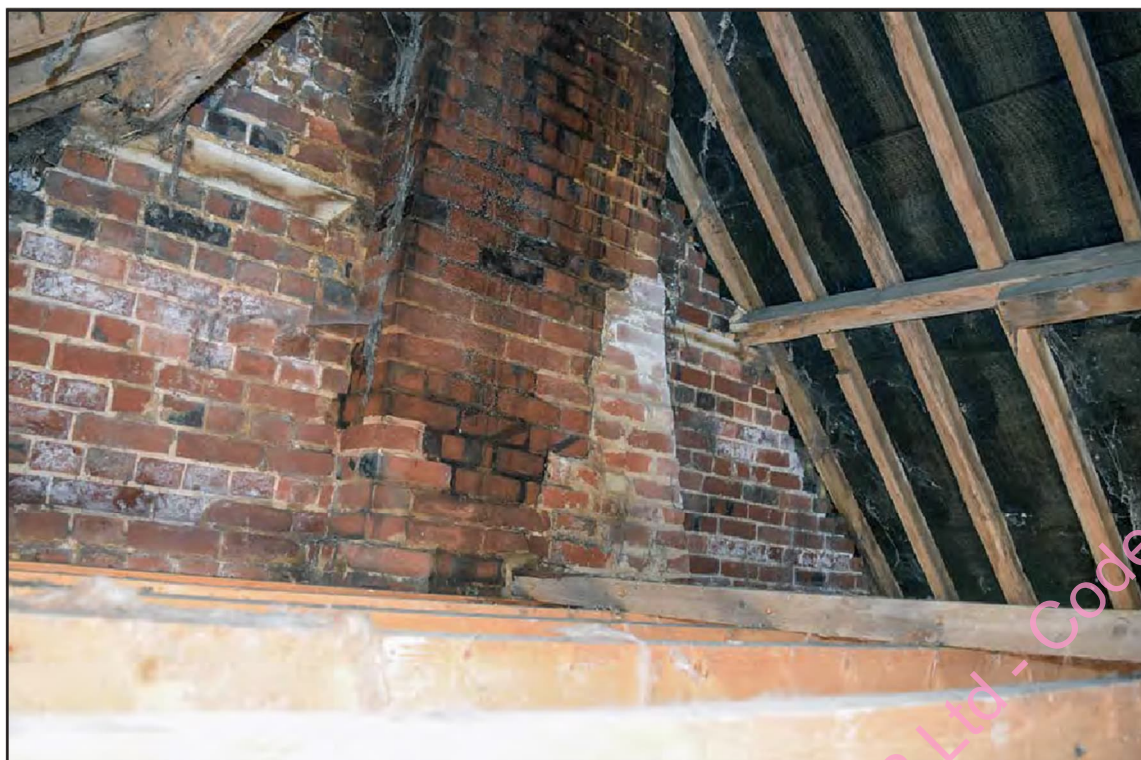
Photo A- 44: Roof structure, south gable
