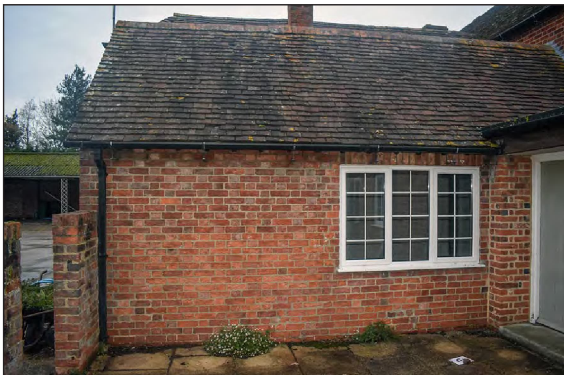
Photo A- 15: The south-west extension south elevation
