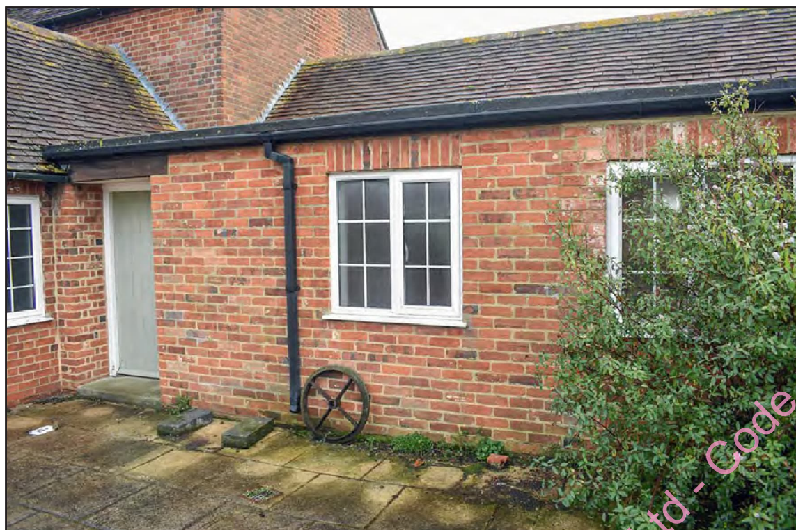
Photo A- 16: The south extension rear section
