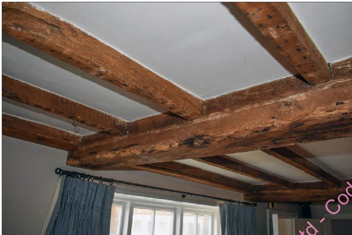
Photo A- 32: Ceiling structure to Kitchen G5 in rear extension
