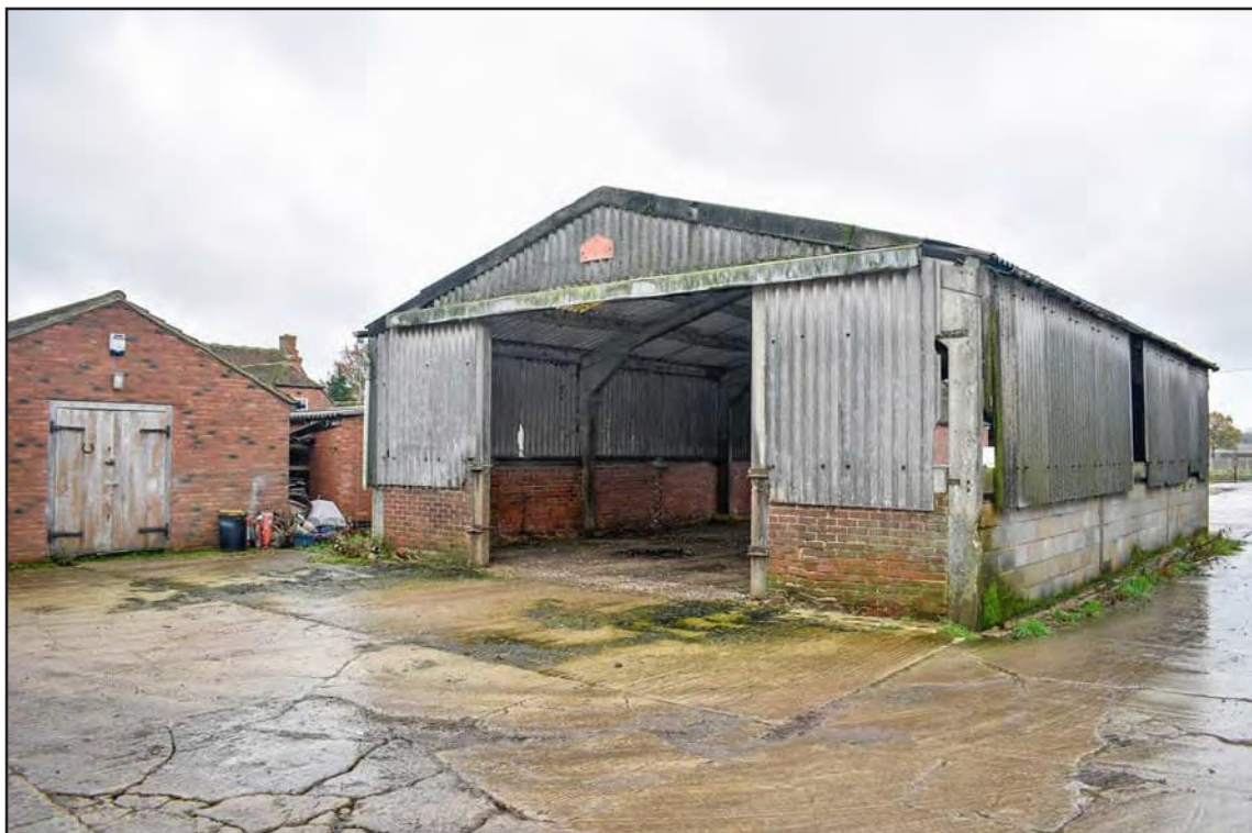
Photo A- 53: Outhouse D north facing elevation
