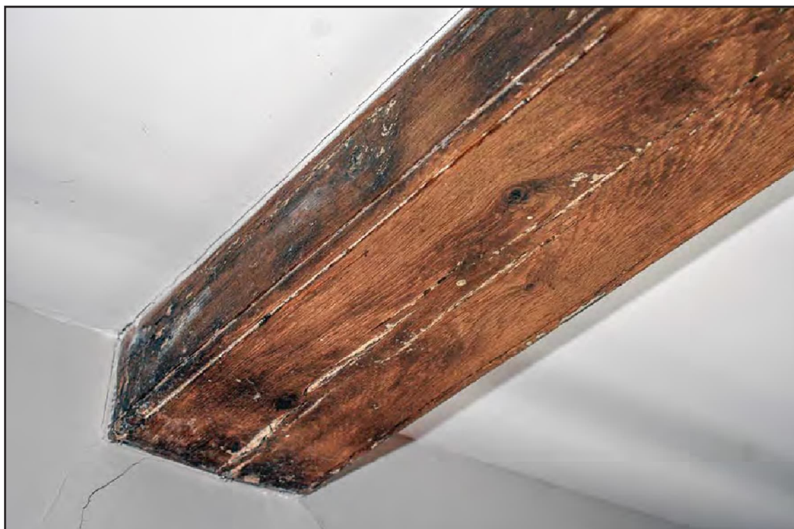
Photo A- 19: Ceiling beam in G1, north-west
