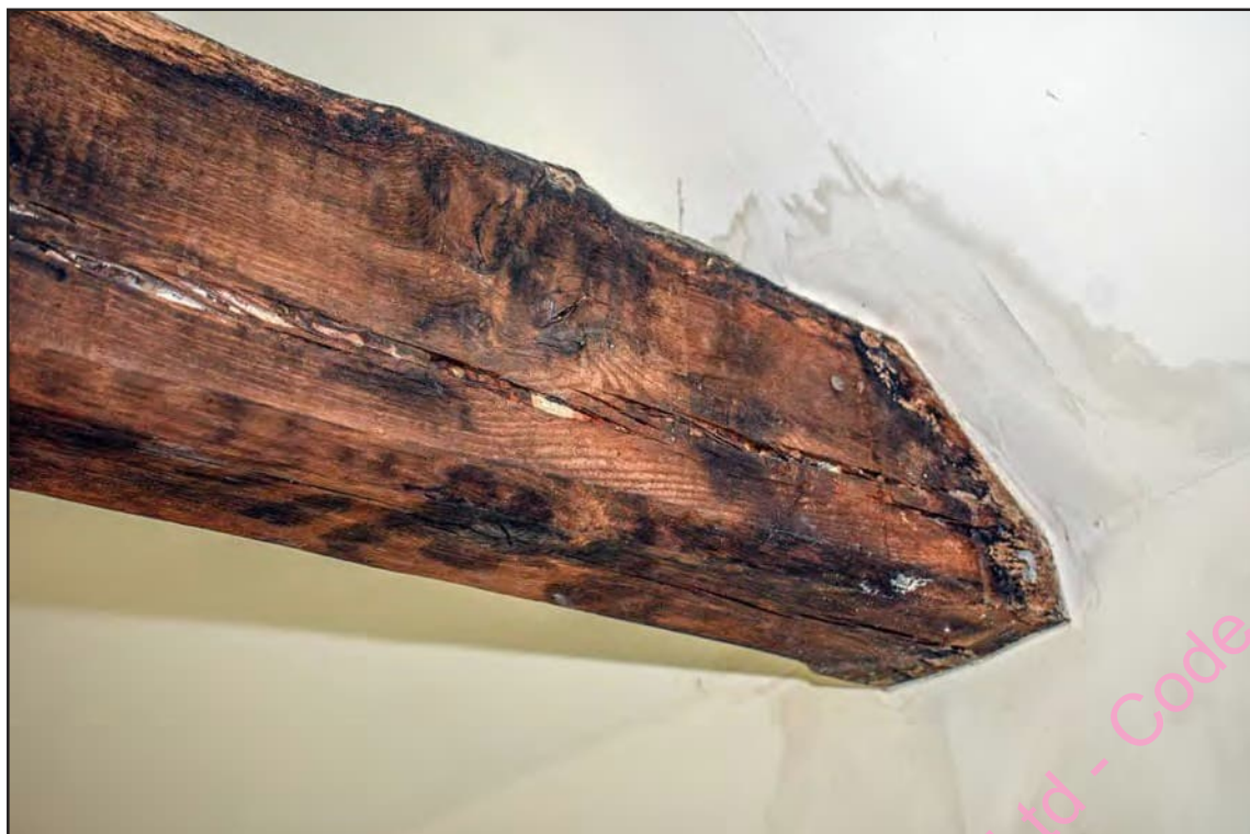
Photo A- 30: Detail of ceiling beam room G4
