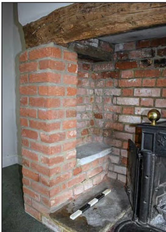
Photo A- 21: The fireplace in G1, detail
