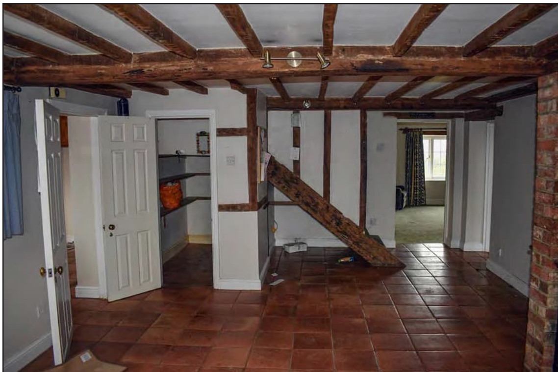
Photo A- 31: Kitchen, G5 in south extension looking to the front
