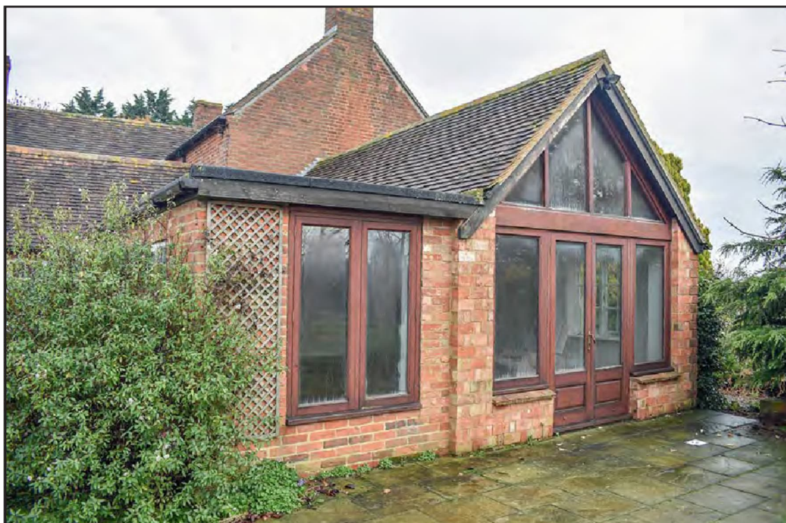
Photo A- 17: The south extension , south elevation
