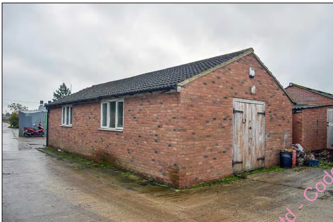
Photo A- 52: Outhouse C, north facing elevation
