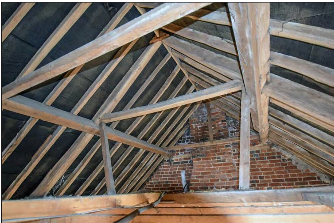
Photo A- 49: The roof structure to the farmhouse, looking north
