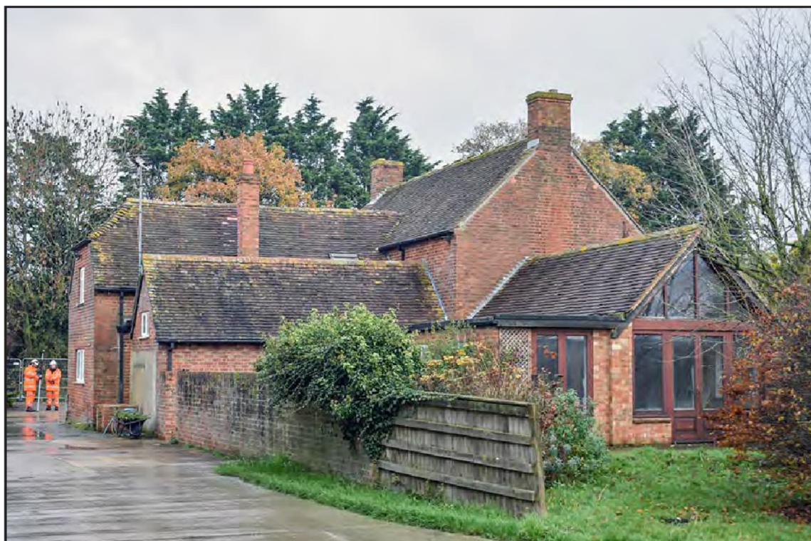
Photo A- 3: Rear aspect of the farmhouse, looking north
