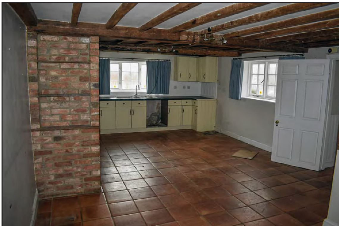
Photo A- 33: Kitchen G5 in rear extension looking to west
