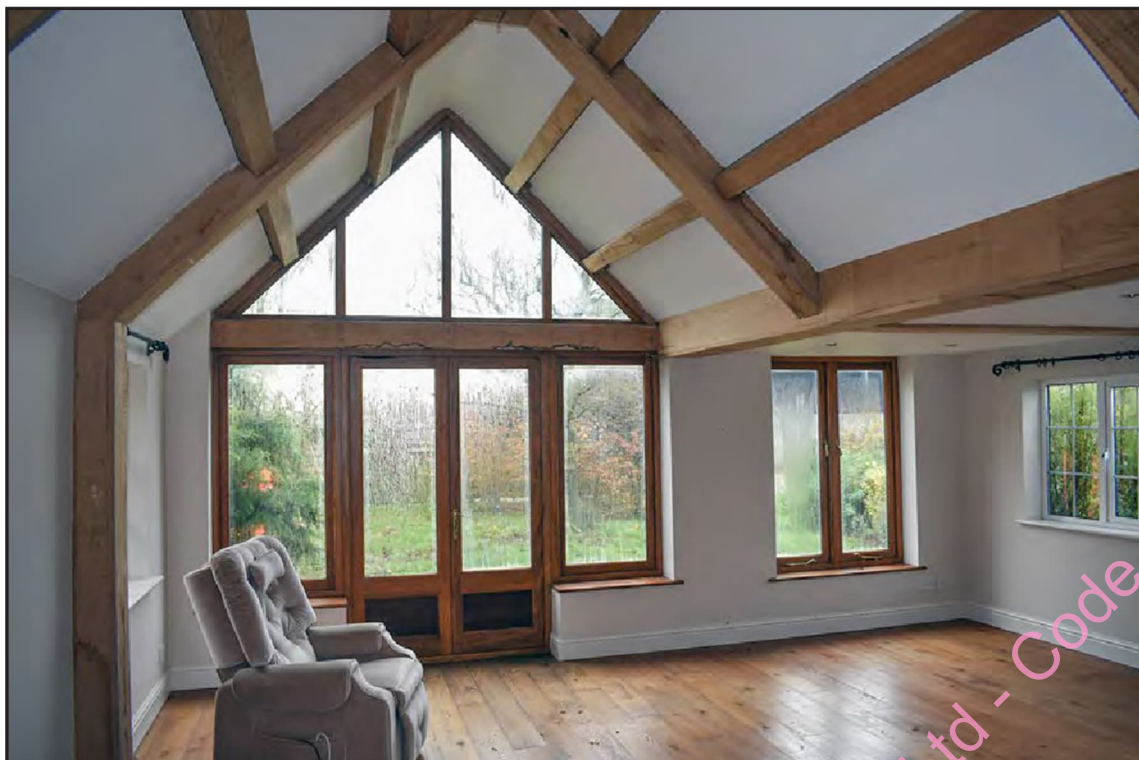
Photo A- 26: South extension G3 looking to south gable
