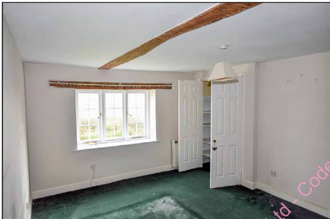
Photo A- 42: Bedroom F3 front elevation
