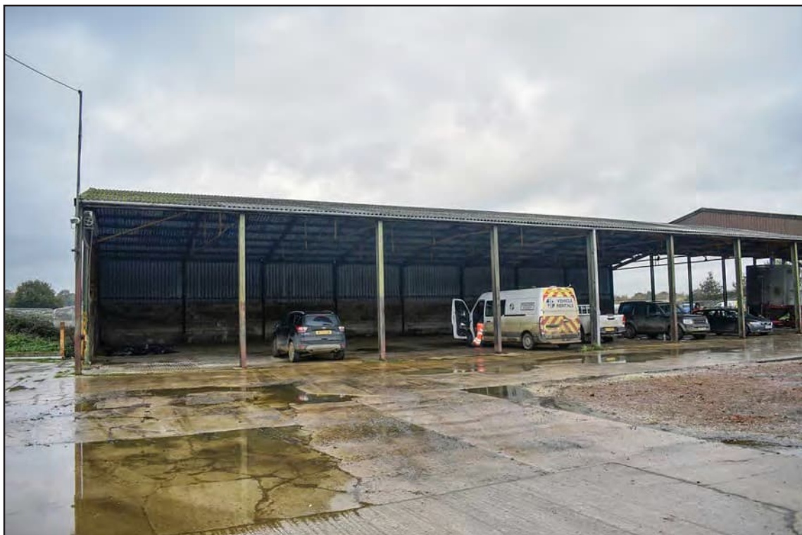
Photo A- 57: Outhouse | east facing elevation
