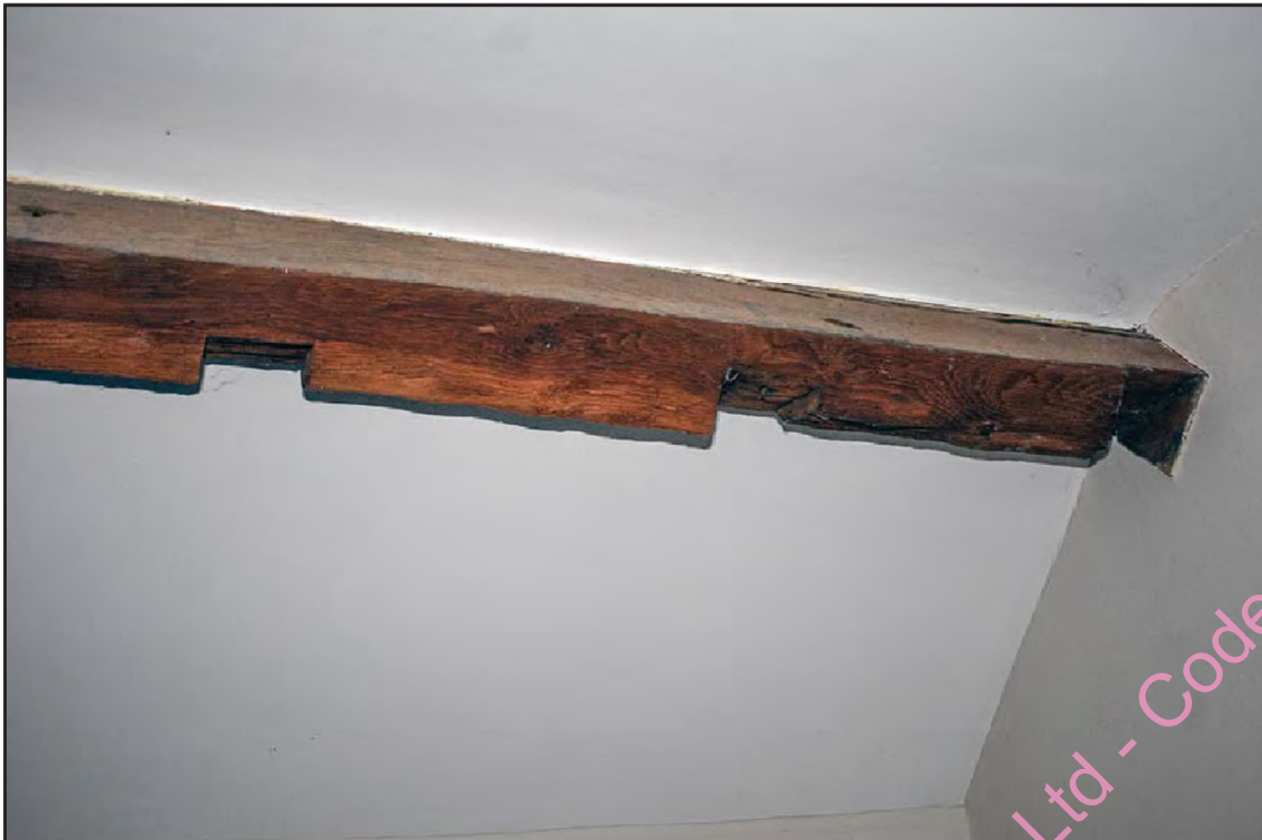
Photo A- 46: Notched purlin, south extension first floor
