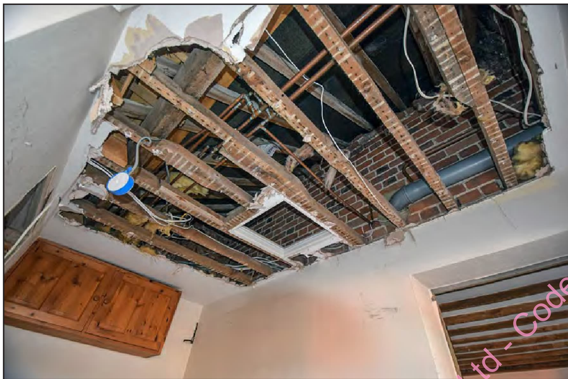
Photo A- 36: Lobby G6 during soft strip showing former exterior rear elevation
