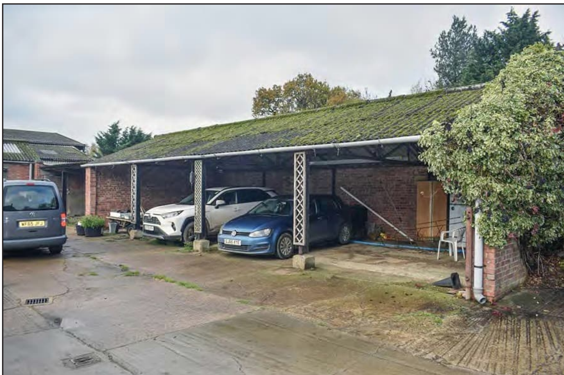
Photo A- 51: Outhouse B, south facing elevation
