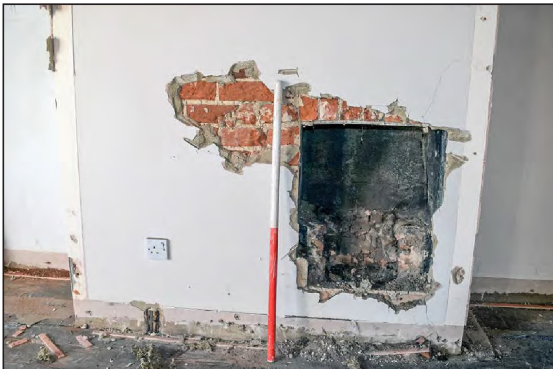
Photo A- 43: Bedroom F3 exposed fireplace in south gable
