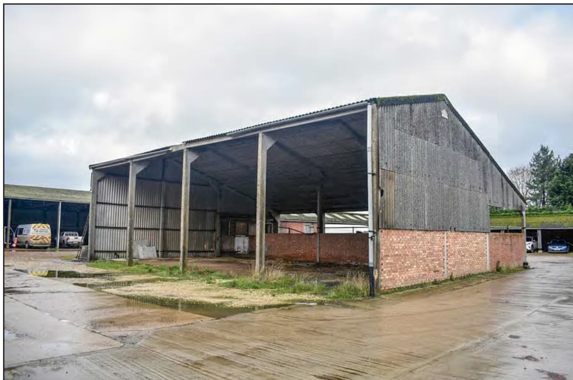
Photo A- 55: Outhouses F and G south facing elevation
