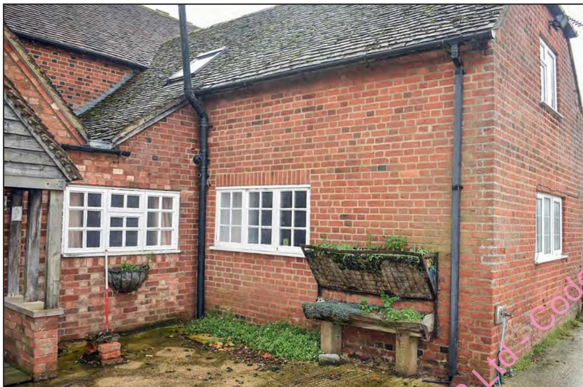
Photo A- 12: The rear extension, north side
