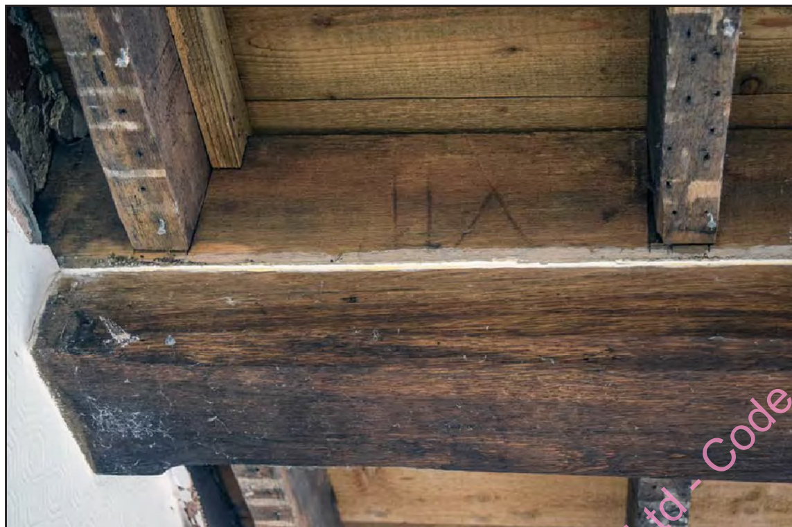
Photo A- 24: Detail of ceiling beam, G2
