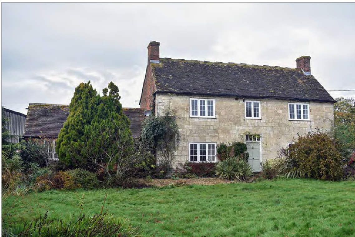
Photo A- 5: The east front elevations of the farmhouse, looking west
