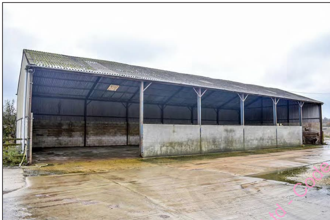
Photo A- 56: Outhouse H north facing elevation
