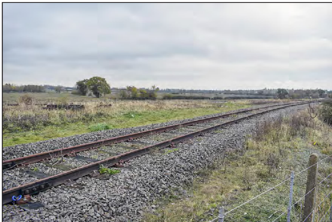
Photo A- 1: The rail loop to the west of the farmstead looking north
