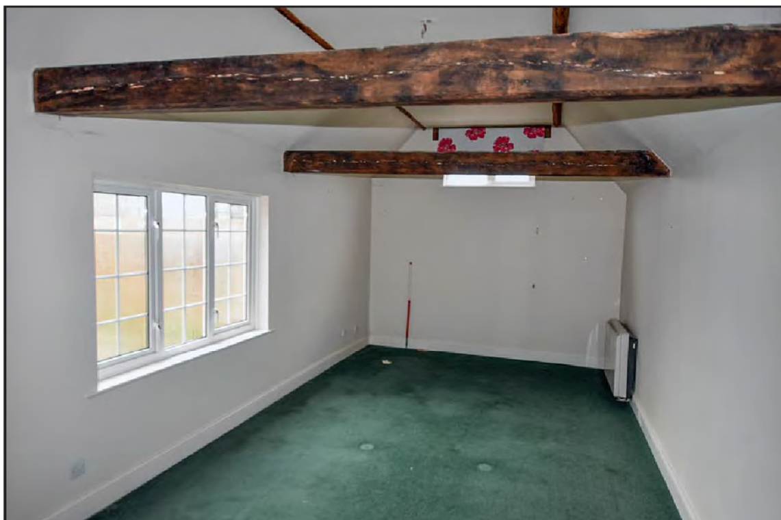
Photo A- 29: Room G4, south west extension looking west
