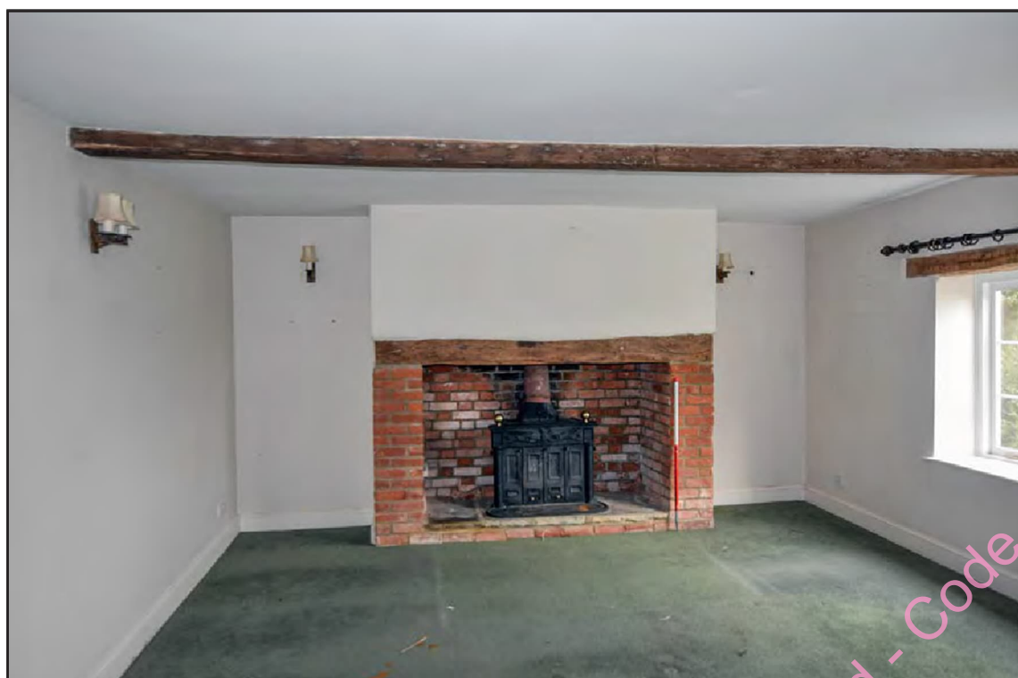
Photo A- 20: Fireplace, north gable G1
