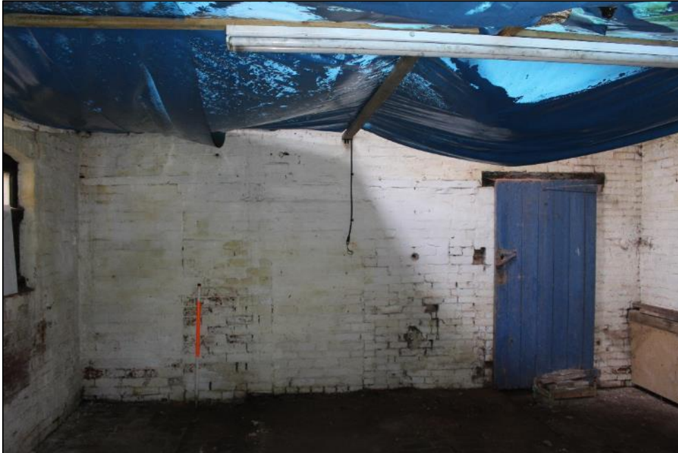
Plate 250: The western wall in Building 9.
