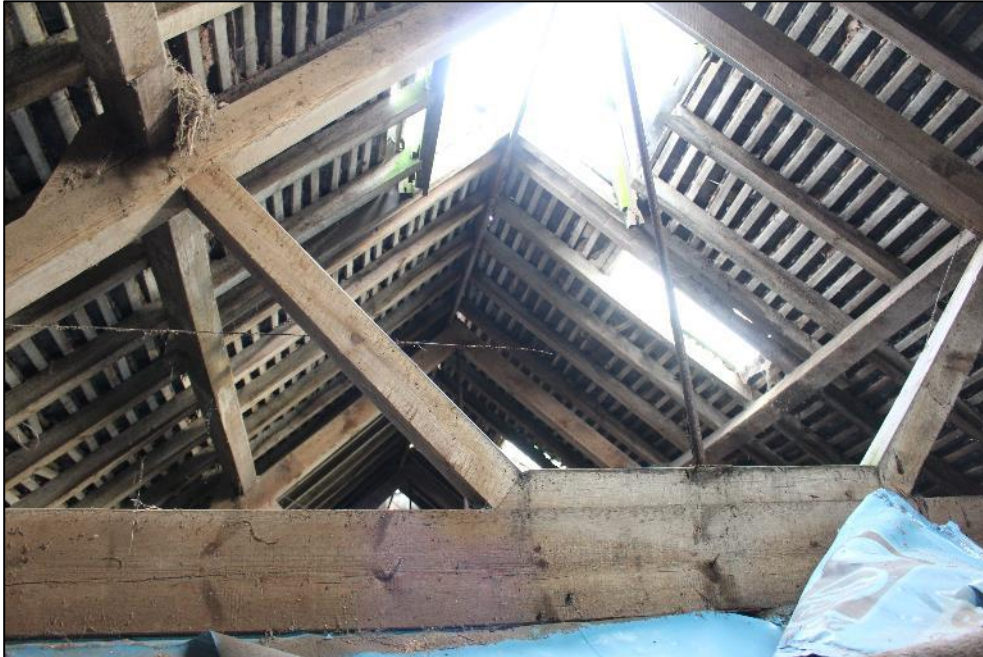
Plate 252: View of the roof structure of Building 9.
