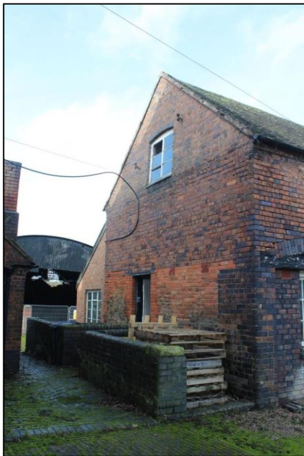
Plate 129: The southern gable of Building 3, viewed from the south-east.
