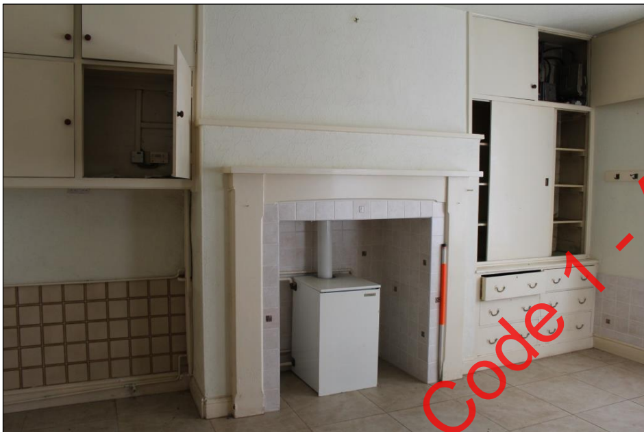
Plate 57: Fireplace and timber cupboard within the western wall of Room 7, Building 1.
