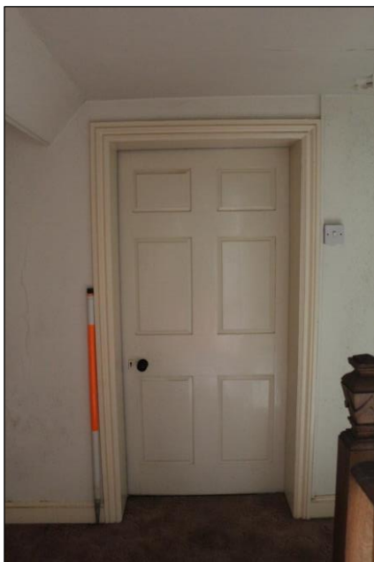
Plate 99: Six panel door between Room 33 and Room 34, Building 1.
