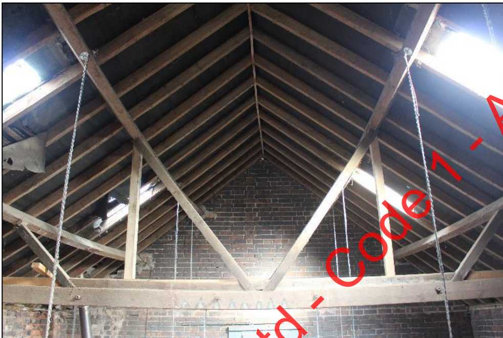
Plate 195: The roof structure of Building 6.
