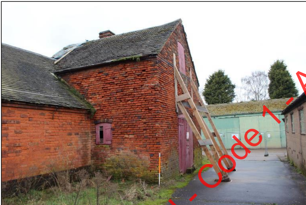
Plate 266: The northern end of the eastern elevation of Building 10b.
