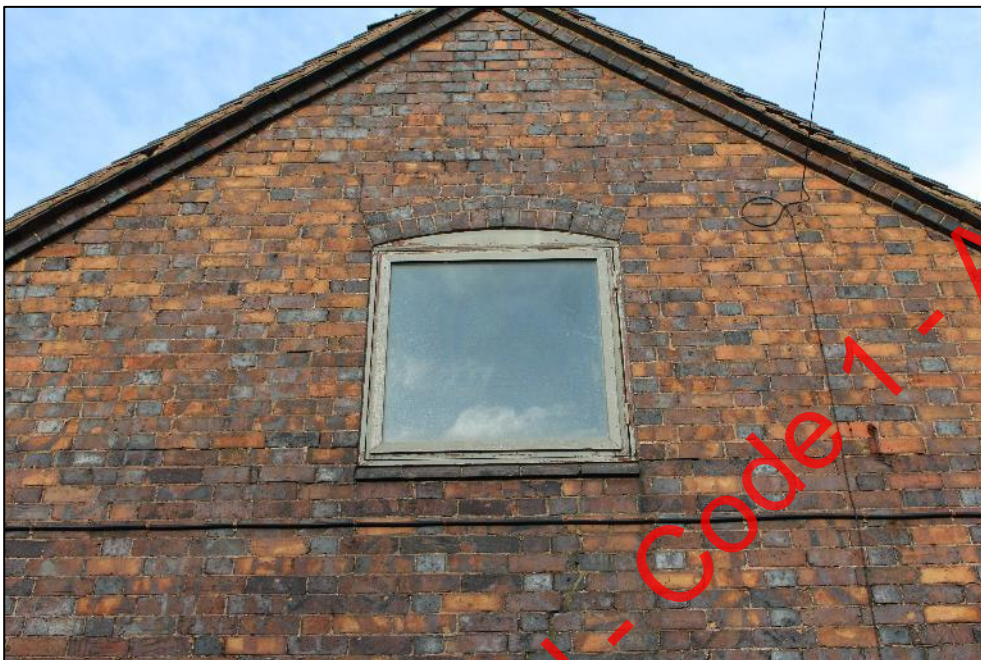
Plate 189: The first-floor window in the southern elevation of Building 6.
