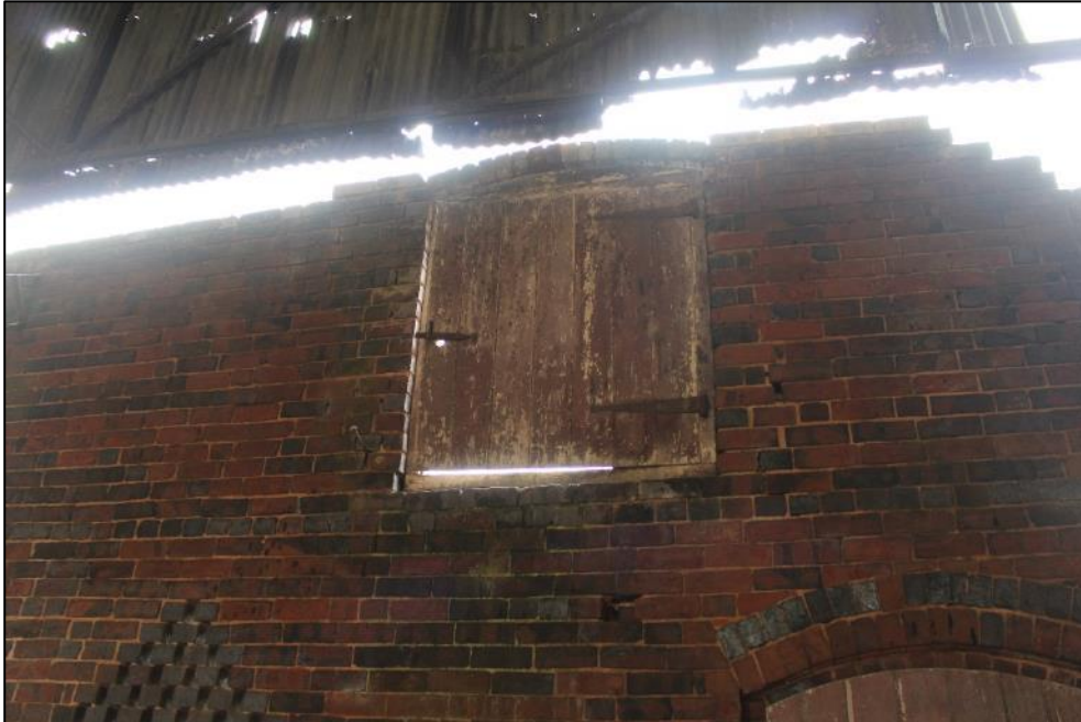
Plate 234: The first-floor pitching window in the eastern elevation of Building 8.
