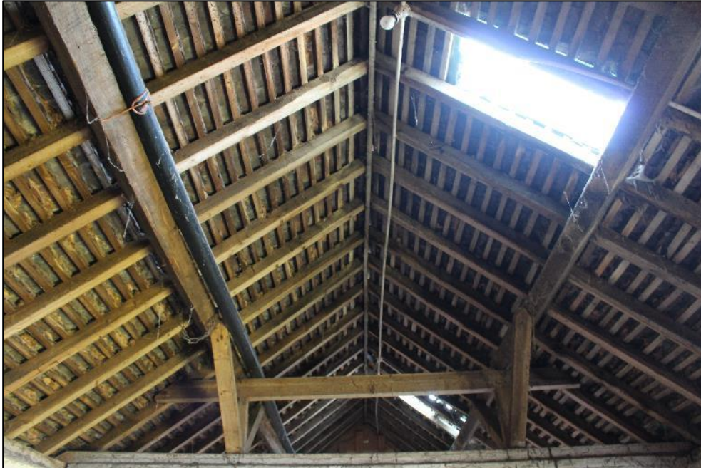
Plate 305: The roof structure of Building 12, taken from within the eastern stable.
