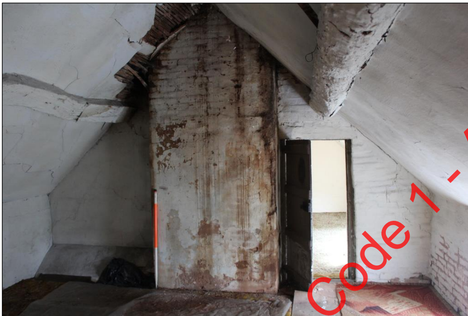
Plate 91: The eastern wall of Room 32, Building 1.
