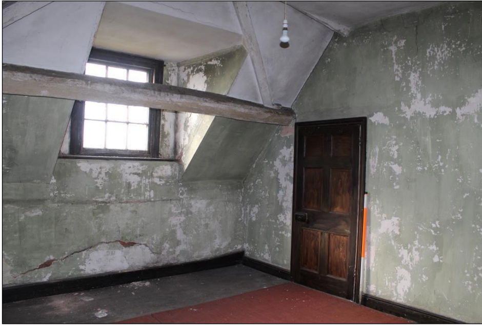
Plate 104: The southern and western walls of Room 35, Building 1.
