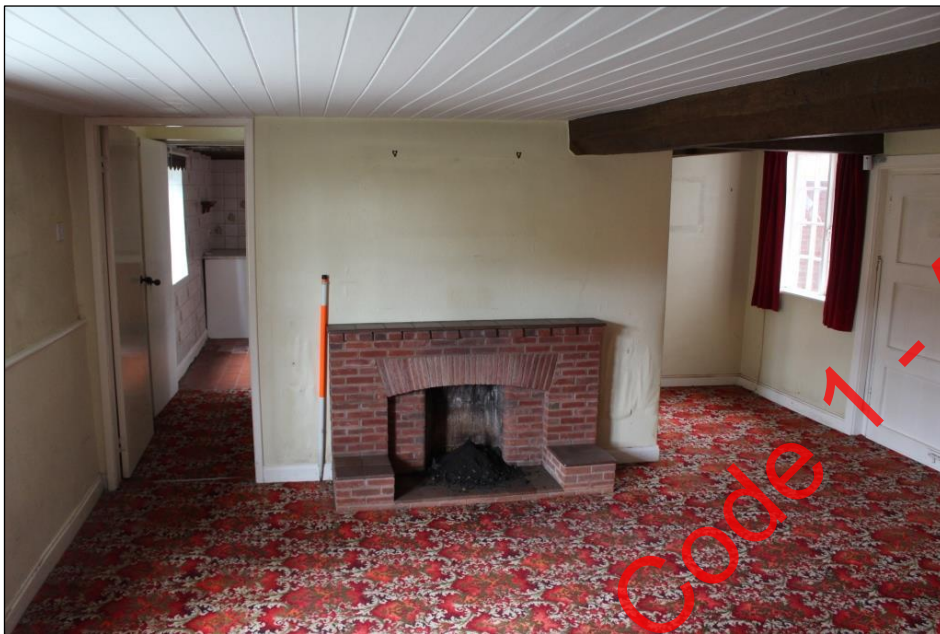
Plate 43: Fireplace set within the western wall of Room 3, Building 1.
