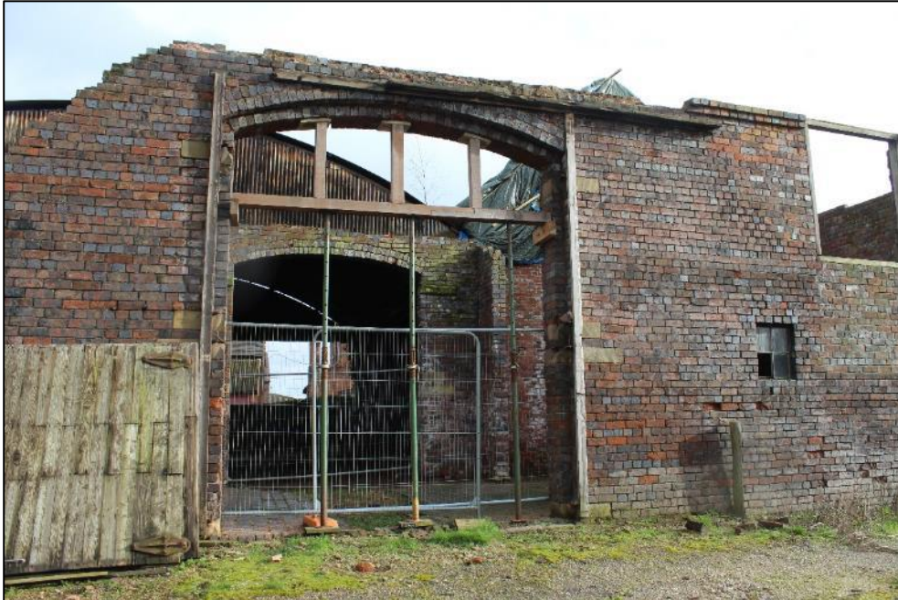
Plate 228: The western elevation of Building 8.
