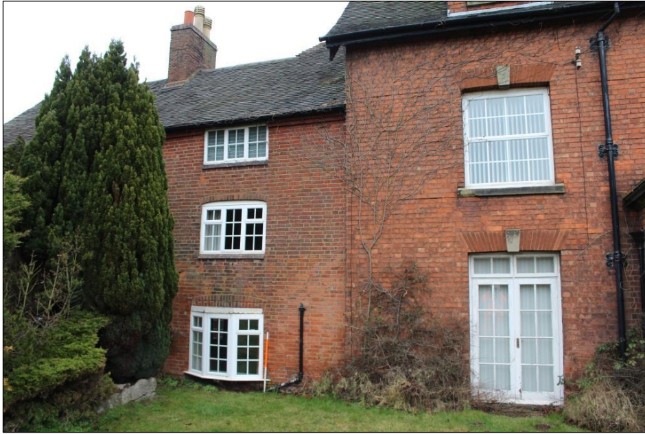
Plate 28: Joint between the eastern and western ranges of Building 1.
