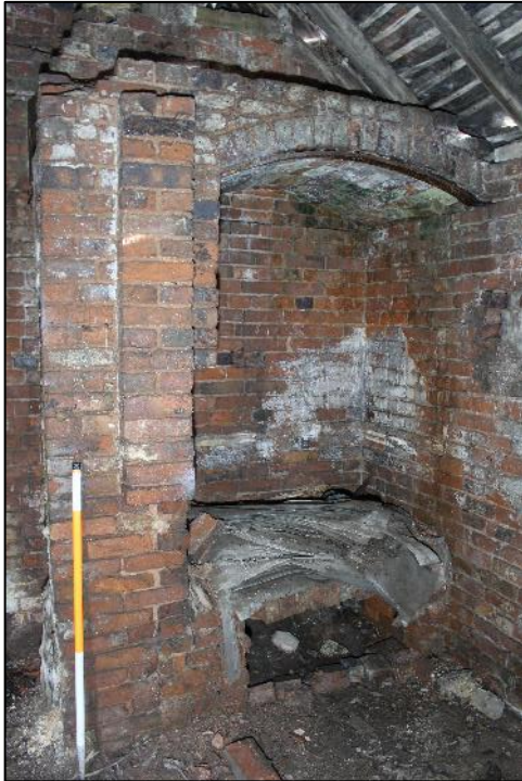
Plate 26g: The remains of the furnace in the south-eastern corner of Building 10a.
