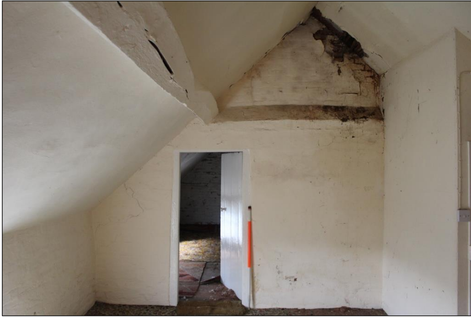
Plate 88: The western wall of Room 31, Building 1.
