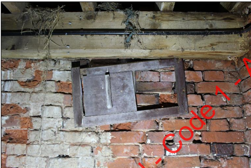
Plate 223: One of the wooden sliding vents visible within the eastern room of Building 7.
