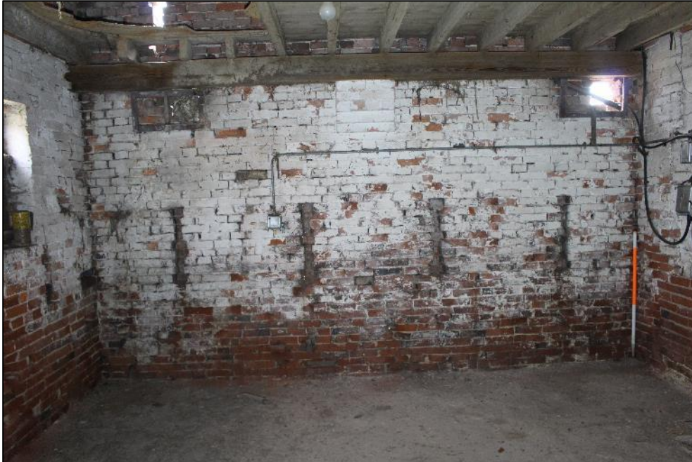
Plate 220: The southern wall in the eastern room of Building 7.
