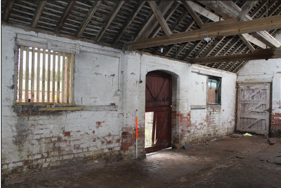
Plate 162: The southern wall of Room 8, Building 4, viewed from the north-east.
