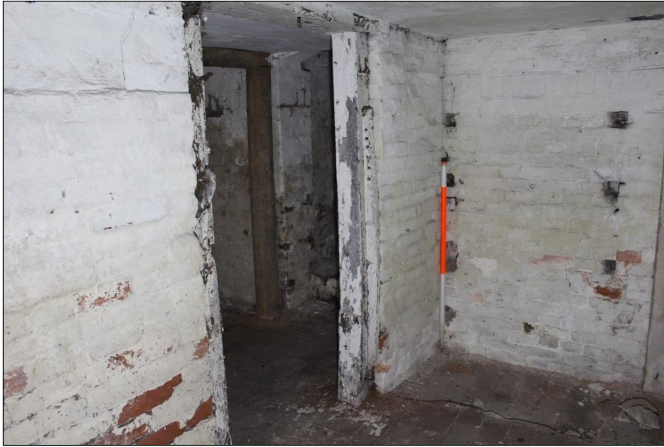
Plate 66: The southern and western walls of Room 17, Building 1.
