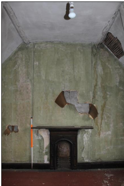
Plate 105: The fireplace within the eastern wall of Room 35, Building 1.
