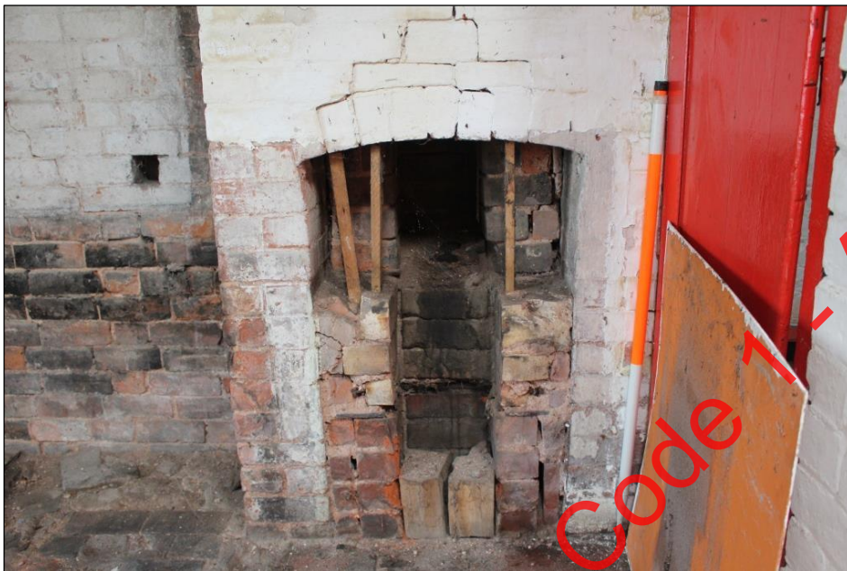
Plate 63: The fireplace set within the north-western extent of the wash house.
