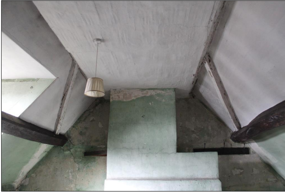
Plate 102: Overview of ceiling construction within Room 34.
