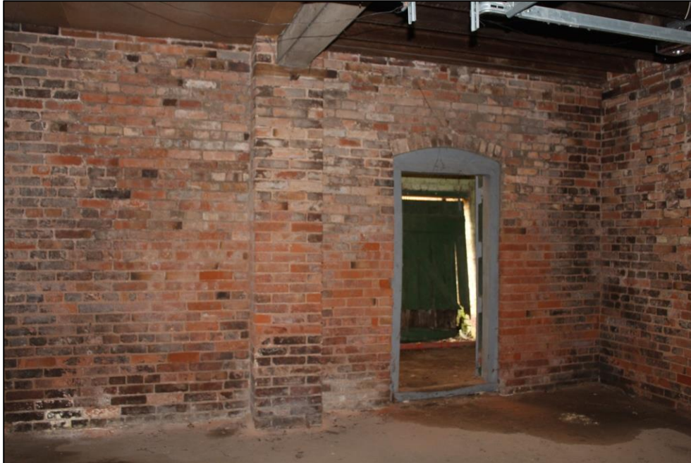
Plate 142: The western wall of Room 1, Building 3, viewed from the south-east.
