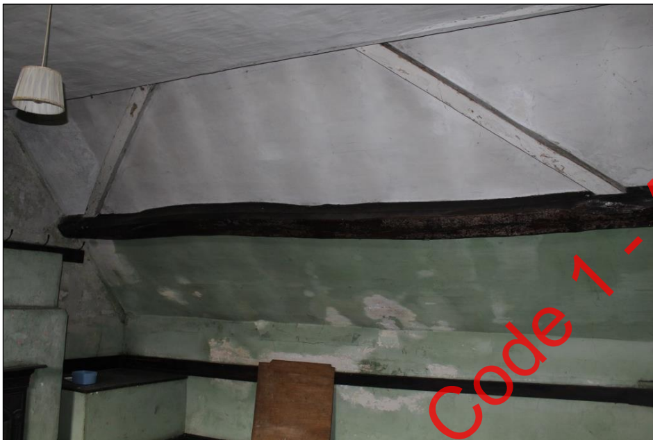
Plate 103: The northern wall of Room 34.
