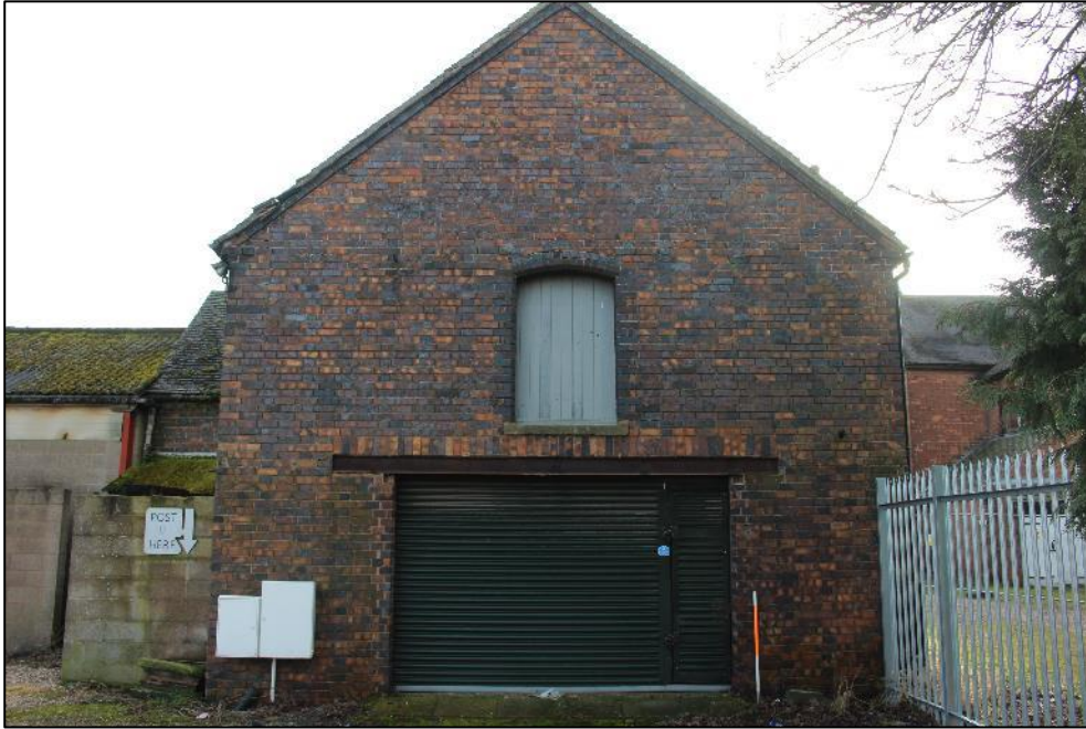
Plate 192: The northern elevation of Building 6.
