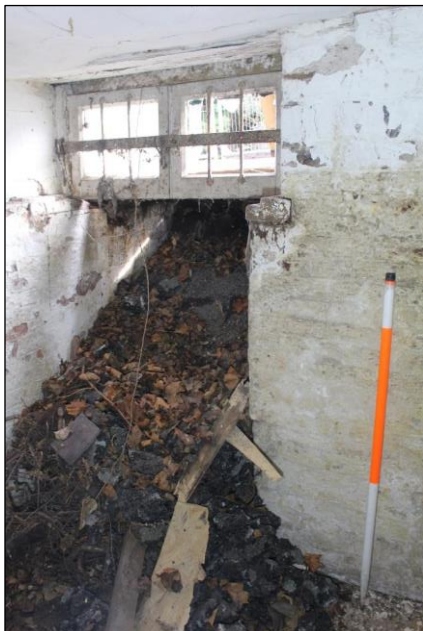
Plate 65: Coal chute and window within the eastern wall of Room 16, Building 1.
