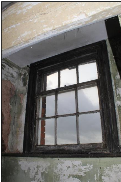
Plate 107: Timber sash window set within the dormer in the southern wall of Room 35, Building 1.
