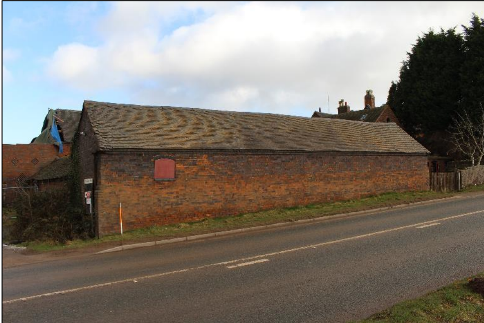
Plate 279: The southern elevation of Building 12, facing onto the main road.
