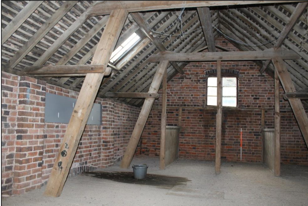
Plate 158: An overview of Room 7, Building 3 from the north-west.
