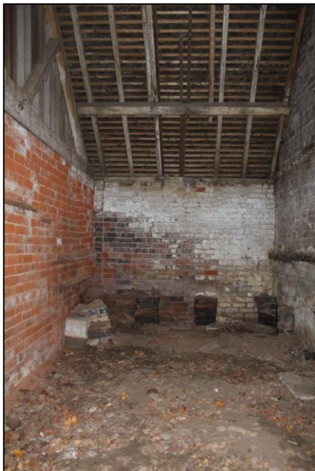
Plate 175: Overview of Room 1, Building 5 from the south.
