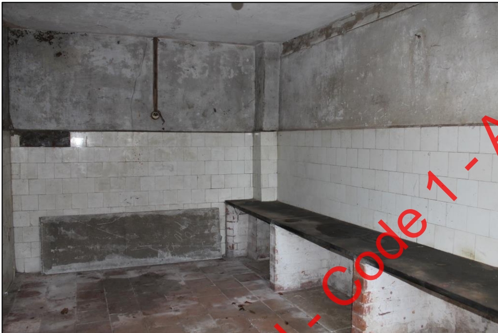
Plate 147: The western wall of Room 2, Building 3, viewed from the east.
