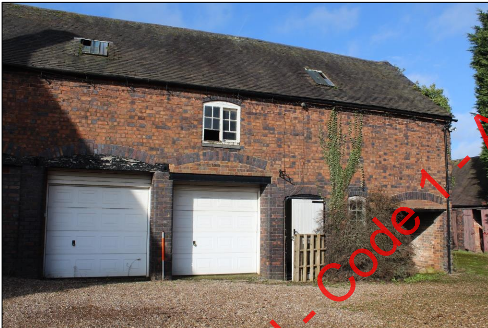
Plate 127: The northern extent of the eastern elevation of Building 3.
