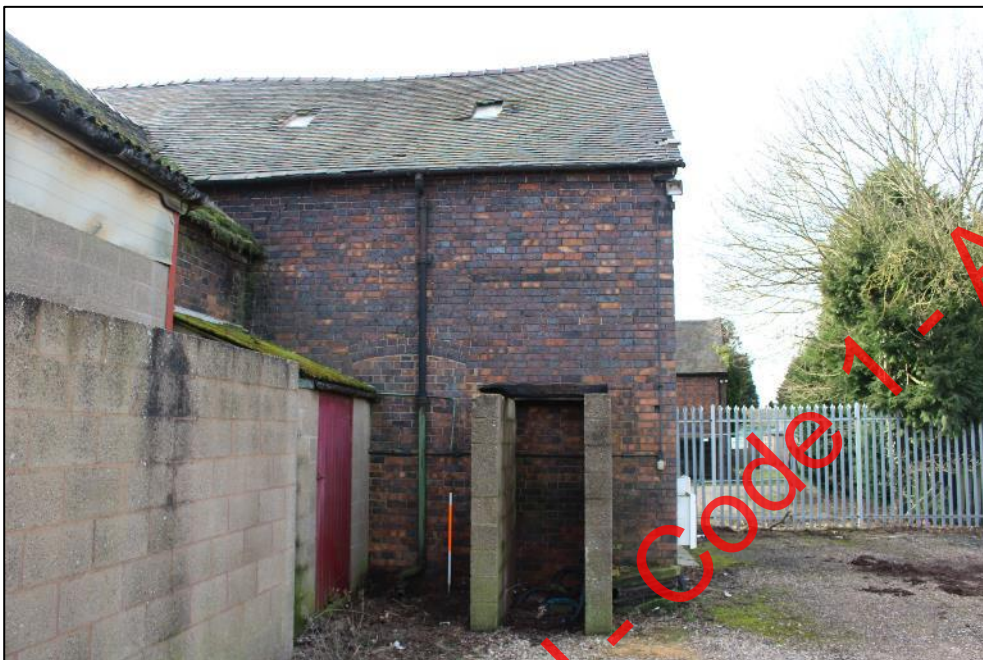
Plate 193: The northern side of the eastern elevation of Building 6.
