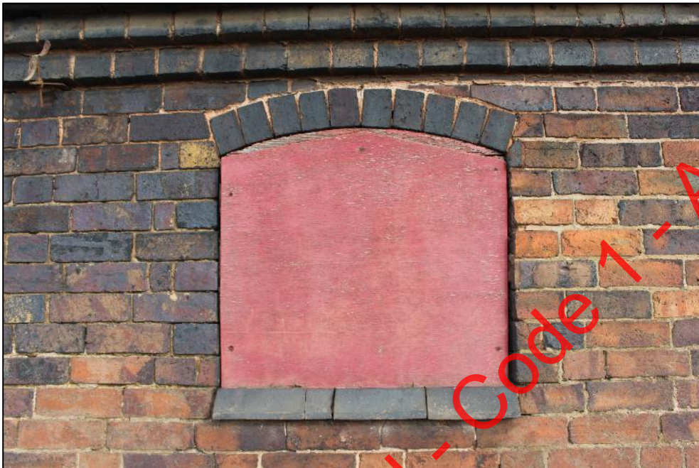
Plate 280: The window in the southern elevation of Building 12.
