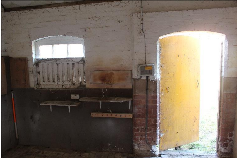
Plate 311: The northern wall in the western stable of Building 12.
