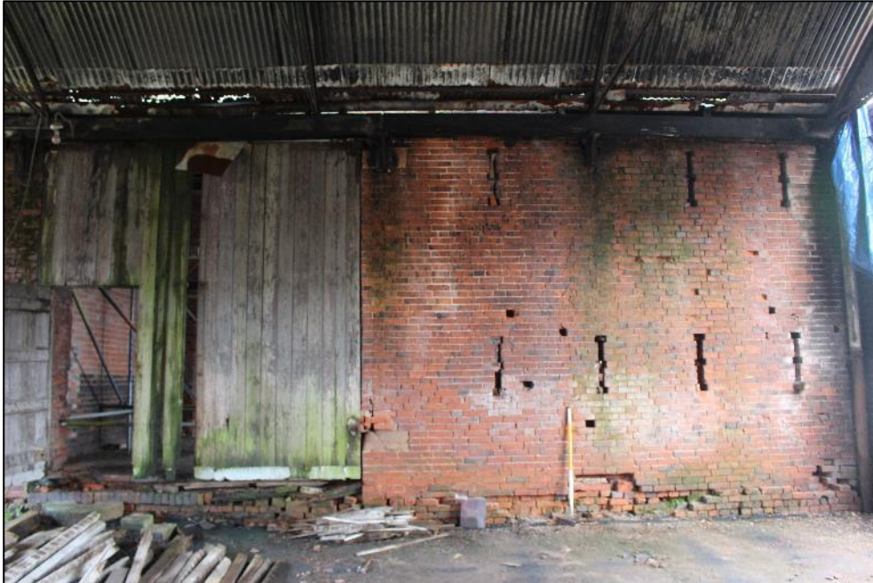
Plate 214: The western side of the northern elevation of Building 7.
