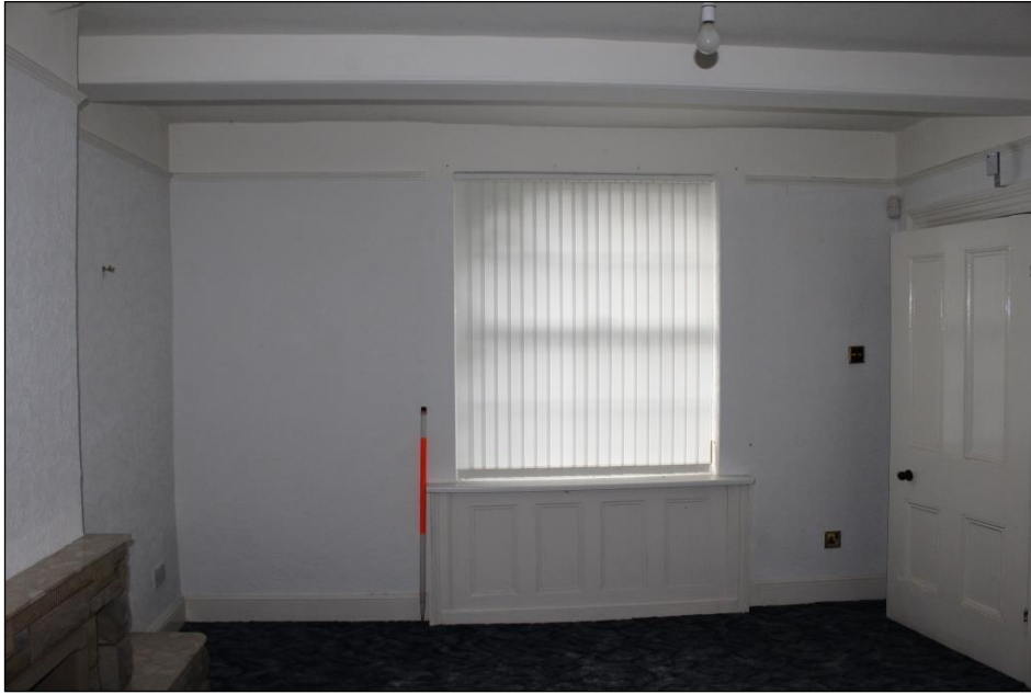
Plate 50: The southern wall of Room 5, Building 1.
