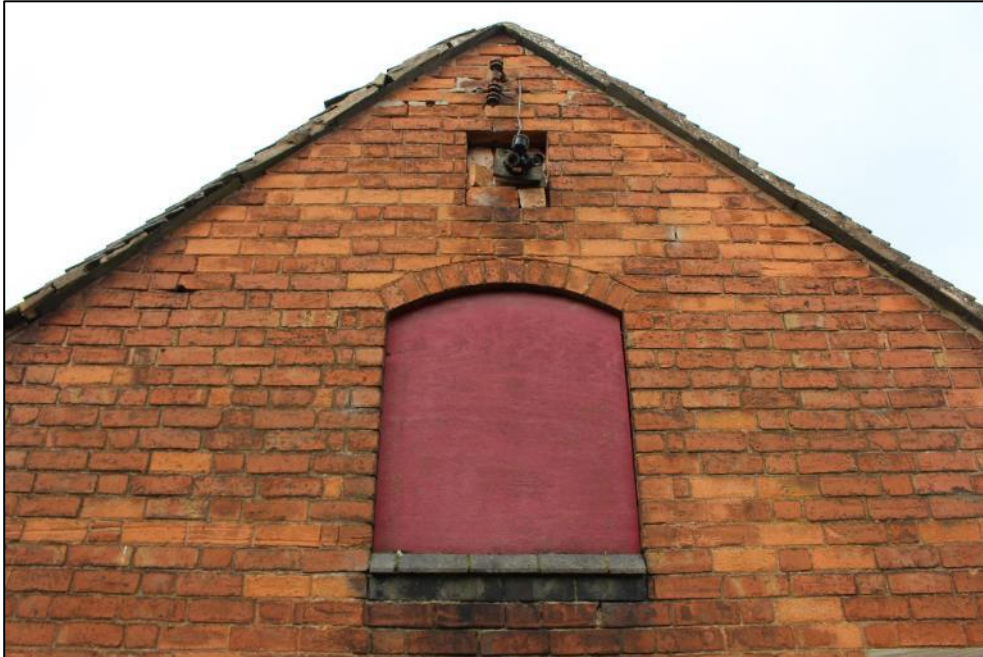
Plate 244: The pitching window in the eastern gable end of Building 9.
