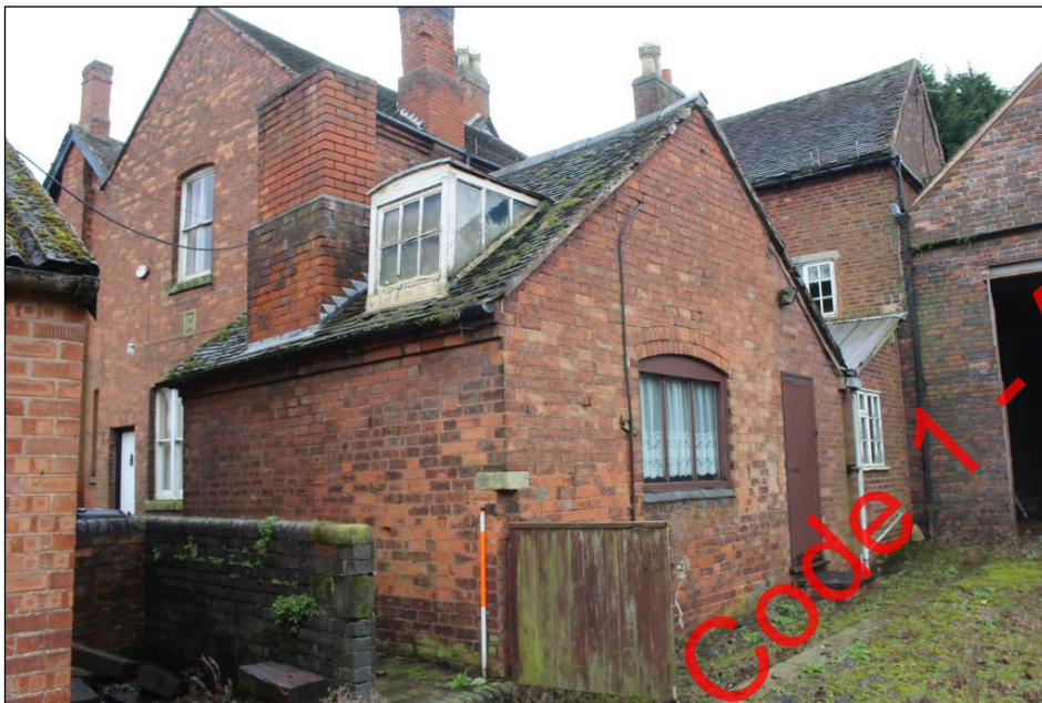
Plate 39: Building 1 and the wash house, viewed from the north-west.
