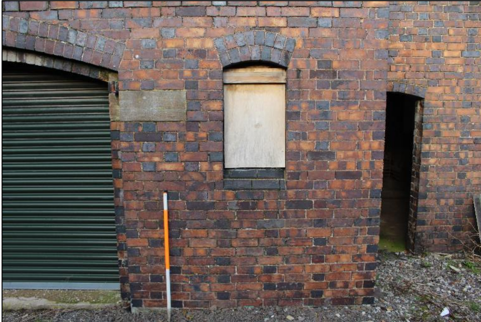
Plate 188: One of the ground-floor windows on the southern elevation of Building 6.
