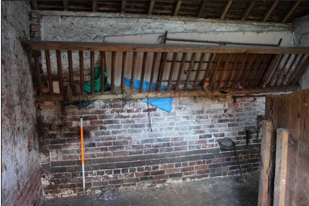
Plate 303: The southern wall in the eastern stable of Building 12, showing the wooden hay feeder.
