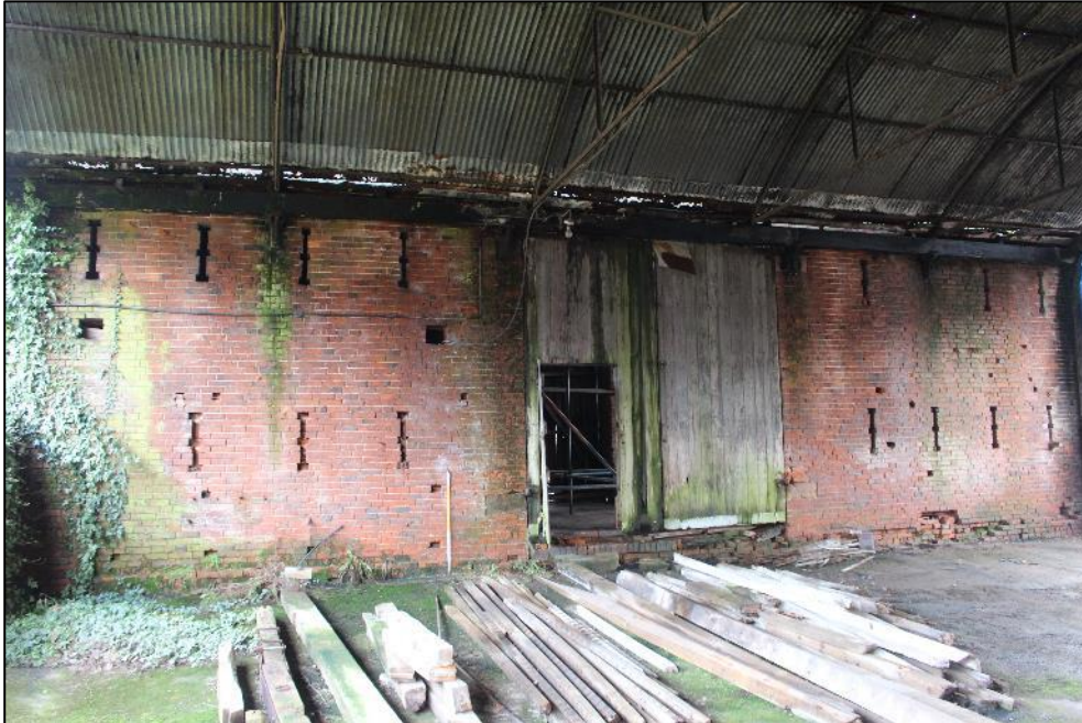
Plate 212: The northern elevation of Building 7, viewed from within the courtyard.
