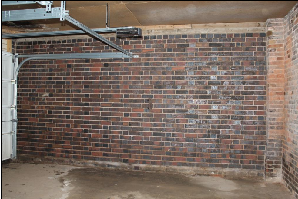
Plate 144: The southern wall of Room 1, Building 3, viewed from the north.
