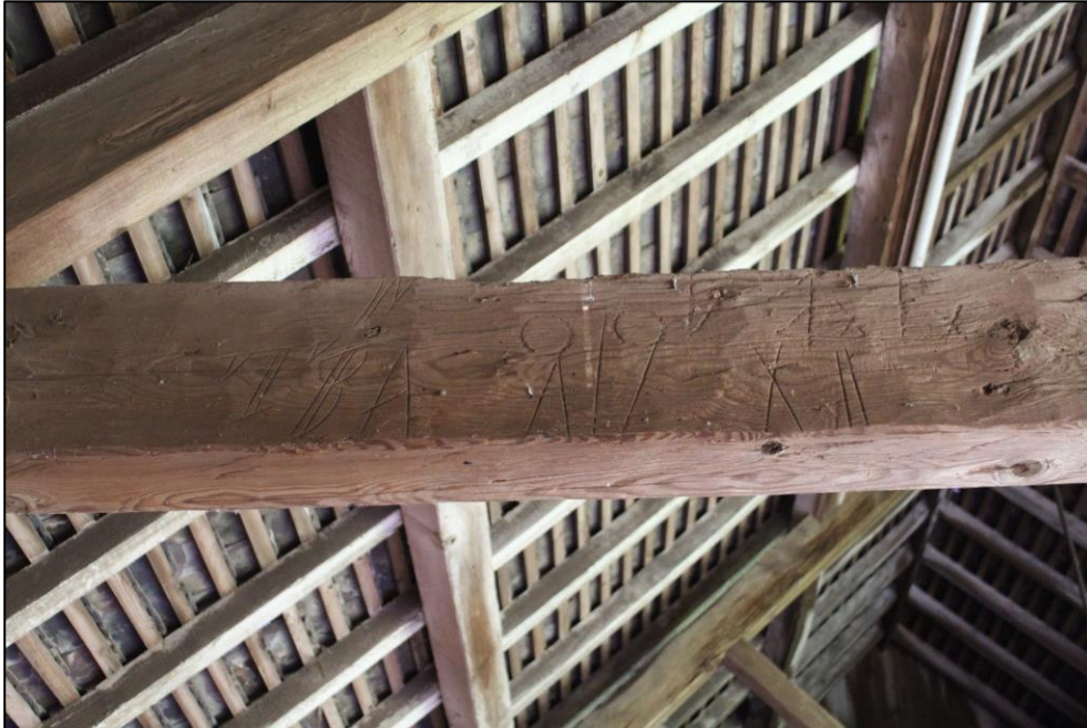
Plate 182: Detail of Baltic timber marks on the tie beam of the western truss within Room 3, Building 5.
