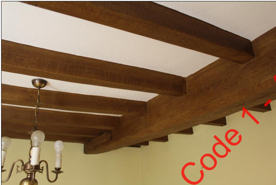
Plate 73: Detail of beam and joist ceiling construction within Room 20, Building 1.
