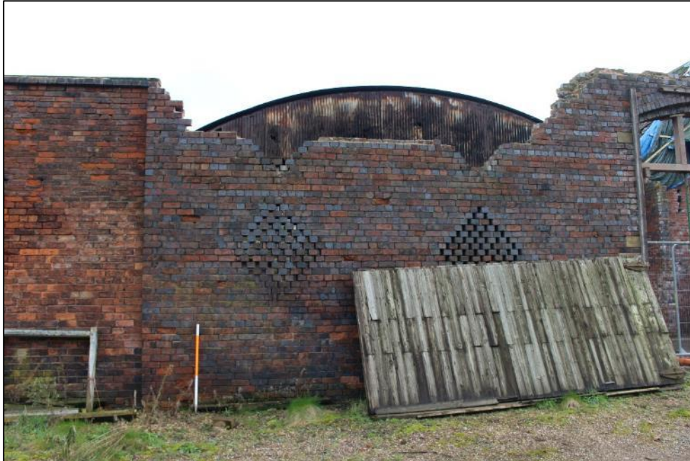
Plate 232: The northern section of the western elevation of Building 8.
