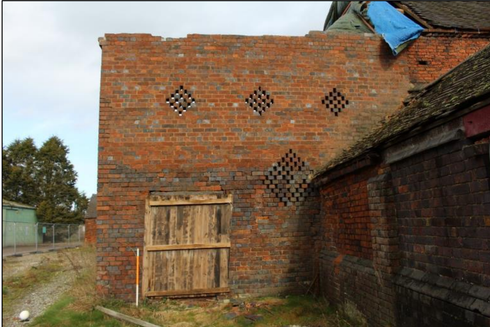
Plate 226: The southern elevation of Building 8.
