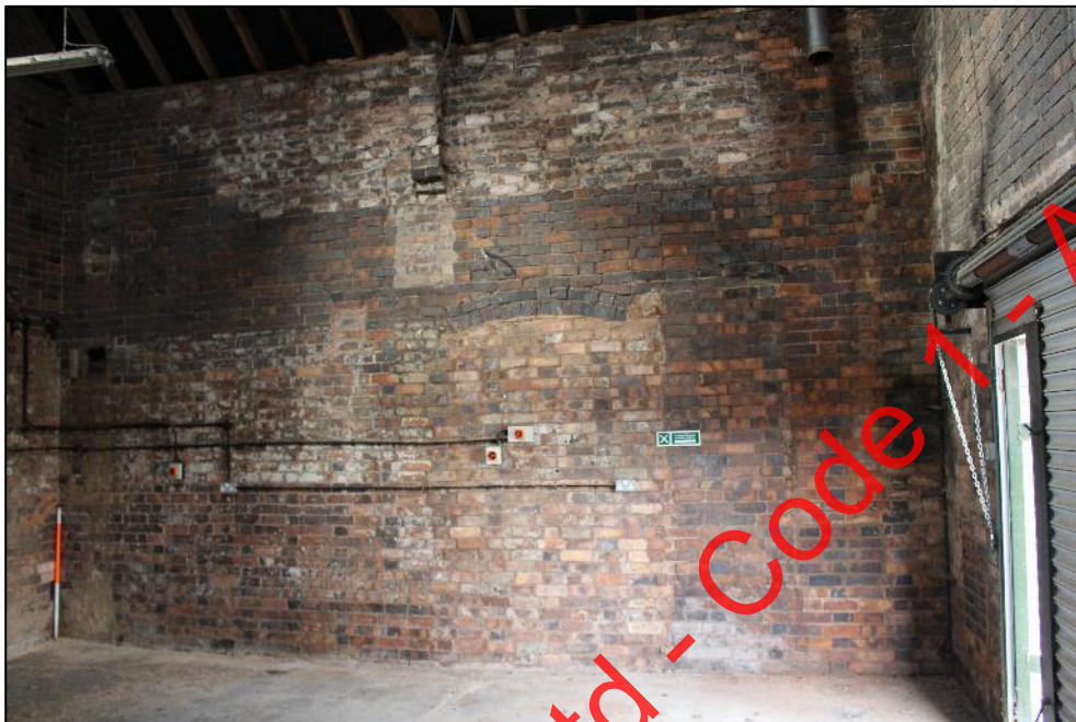
Plate 201: The western wall in the northern half of Building 6.
