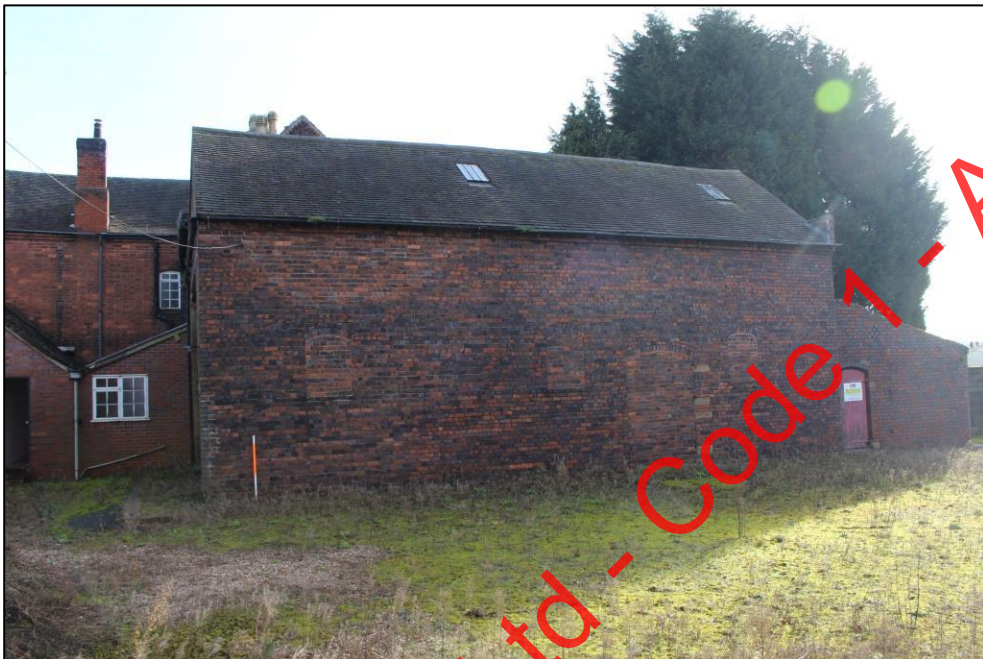
Plate 109: The western elevation of Building 2.
