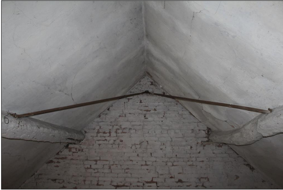
Plate 92: The western wall of Room 32, Building 1.
