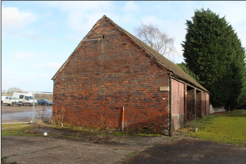
Plate 172: The western gable of Building 5.
