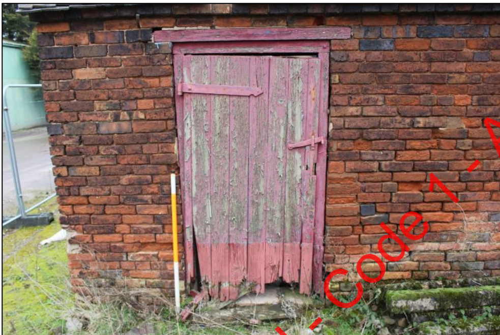
Plate 257: The doorway in the southern elevation of Building 10a.
