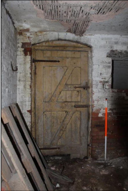
Plate 150: Door opening within the western wall of Room 4, Building 3.
