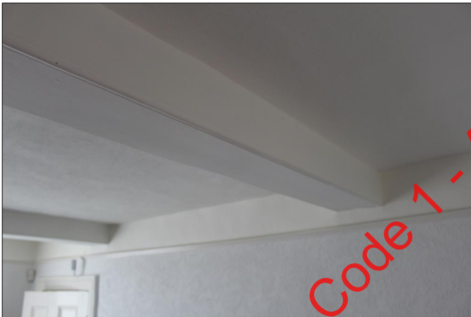
Plate 51: Boxed beams within Room 5, Building 1.
