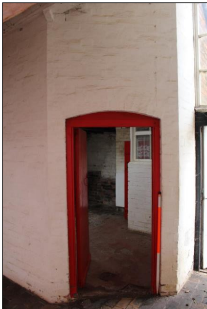
Plate 61: The door to the wash house, Building 1, set within the south-eastern wall.
