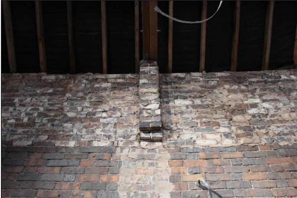
Plate 202: The brick corbel in the western wall of Building 6.
