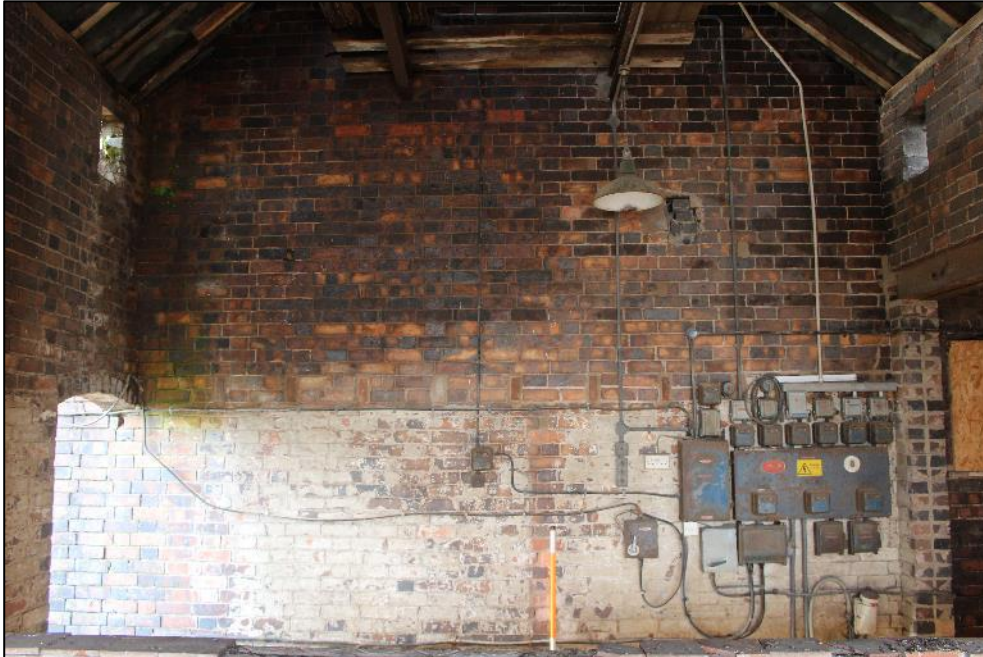
Plate 194: The section of the eastern elevation of Building 6, visible within the eastern extension.
