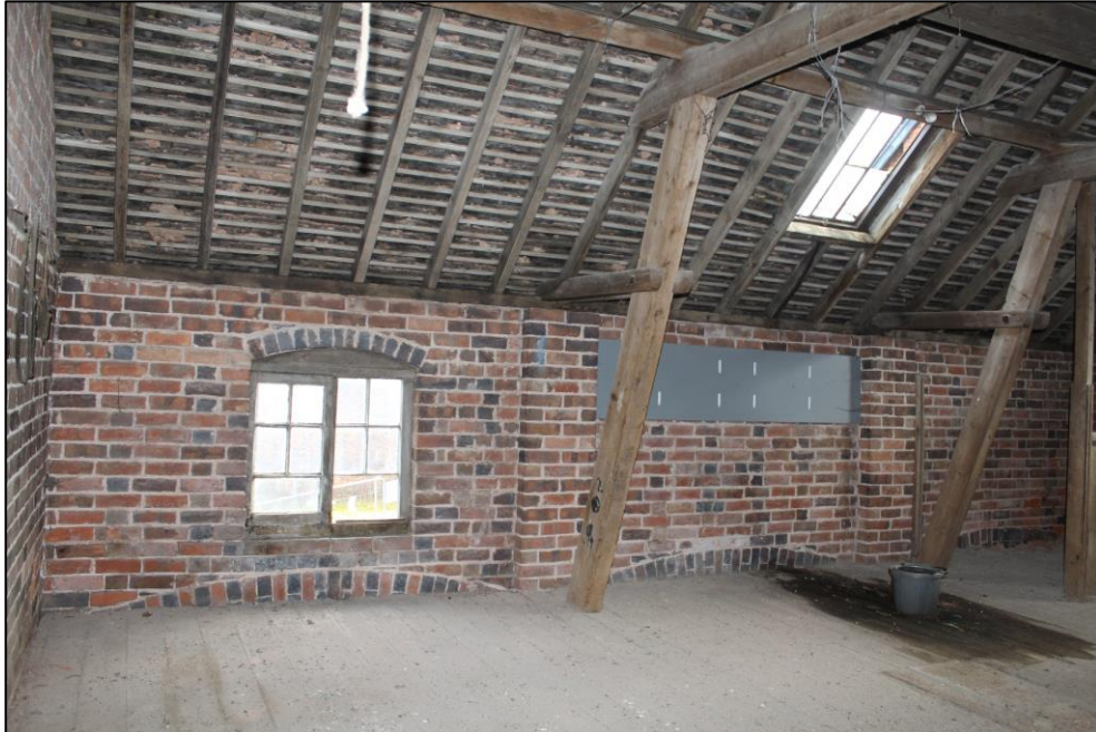
Plate 160: The eastern wall of Room 7, Building 3, viewed from the west.
