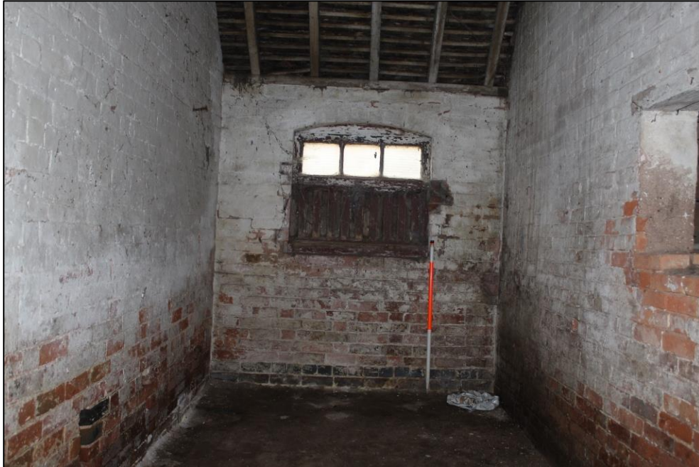
Plate 166: The northern wall of Room 9, Building 4, viewed from the south.
