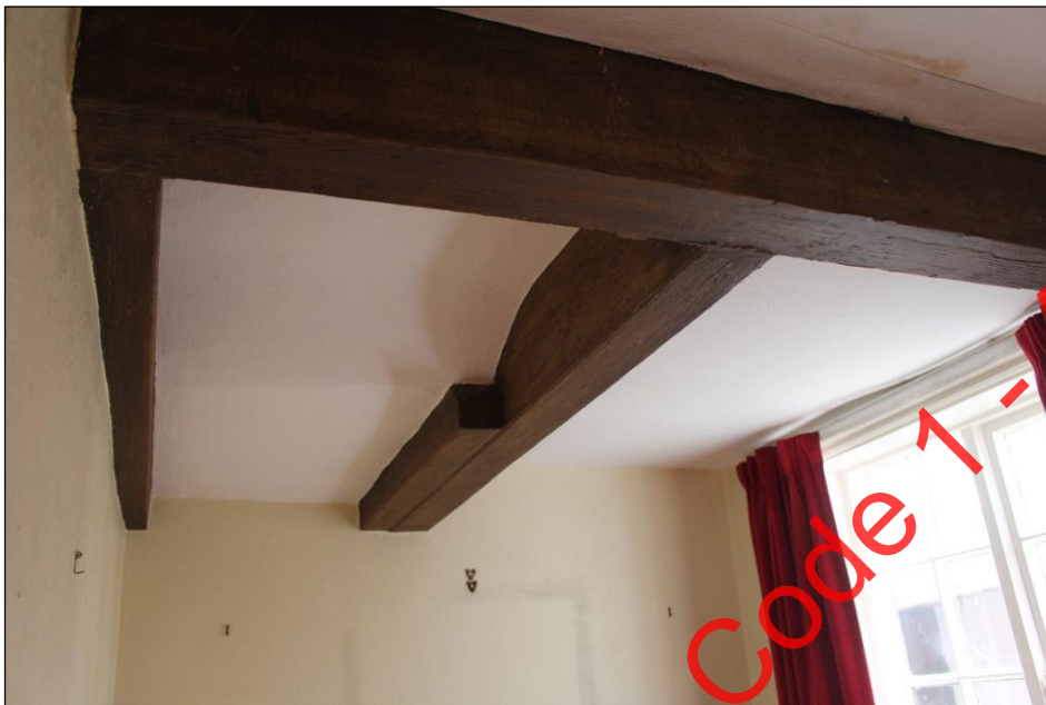
Plate 45: Detail of timber ceiling construction within the north-western corner of Room 3.
