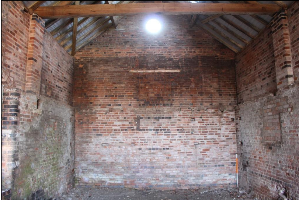
Plate 120: The interior of Building 2 (Room 13) from the north.
