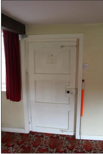
Plate 44: Door opening within the northern wall of Room 3, Building 1.
