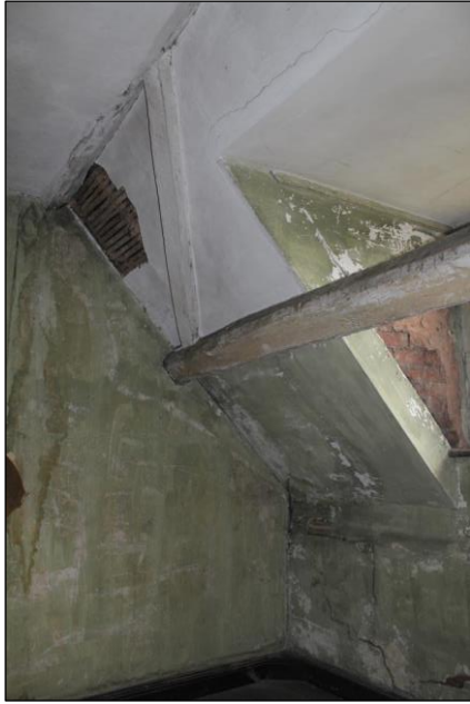
Plate 106: The southern wall of Room 35, Building 1.
