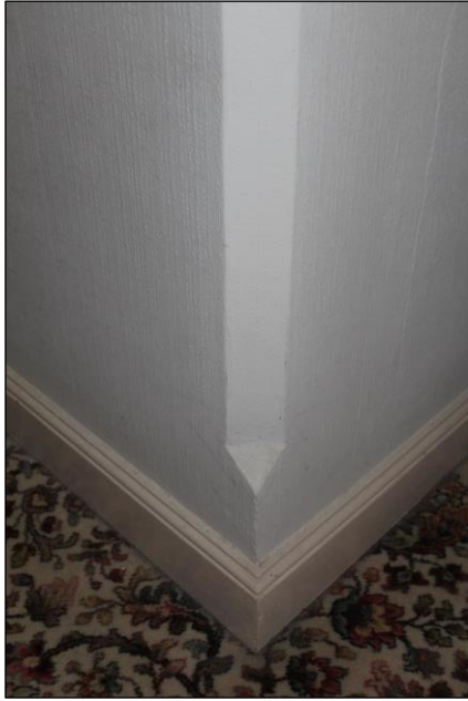
Plate 78: Detail of chamfered corner at the north-western corner of Room 22, Building 1.
