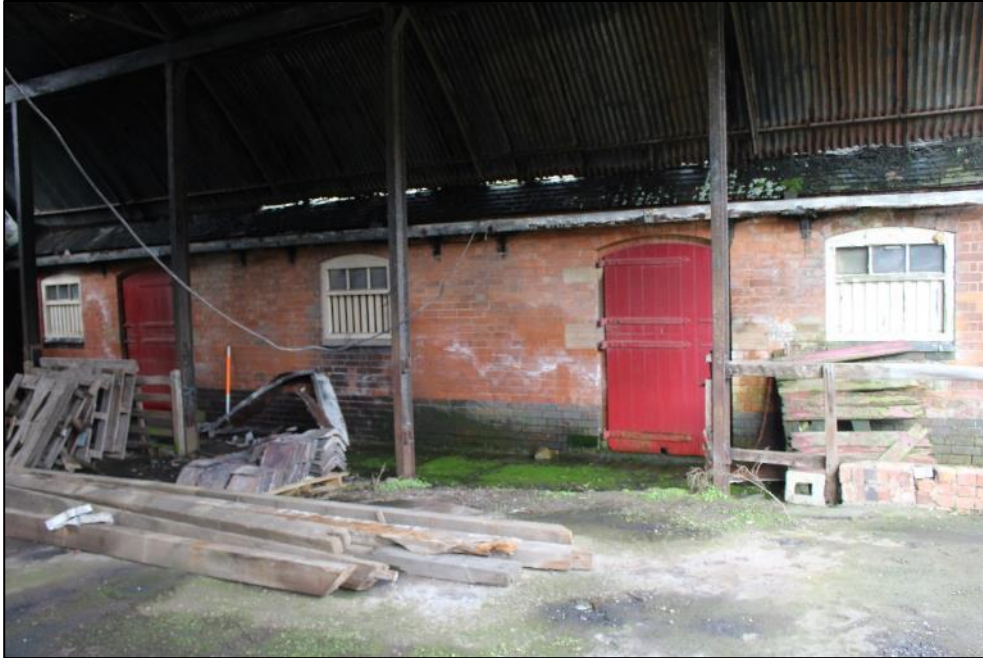
Plate 240: The southern elevation of Building 9.
