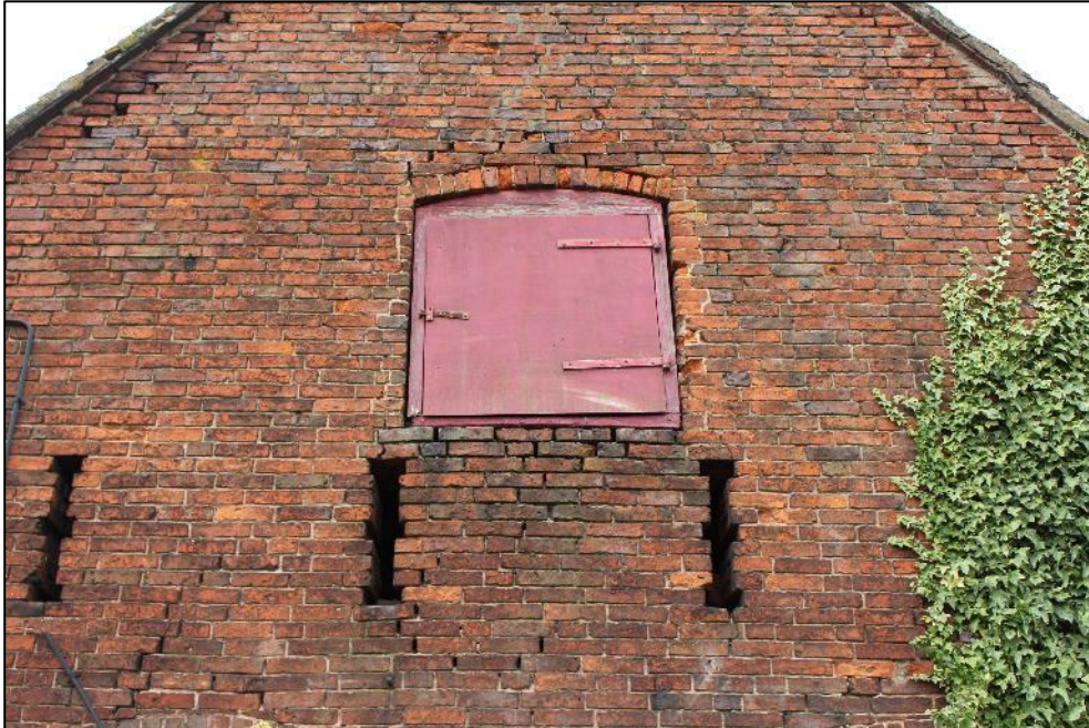
Plate 206: The pitching hole in the eastern elevation of Building 7.
