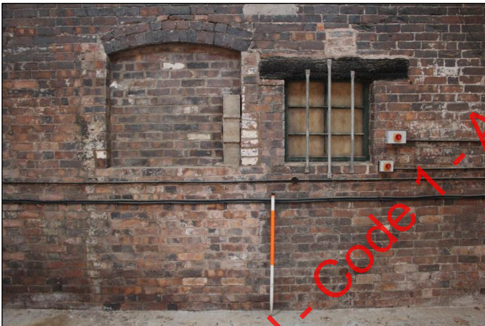
Plate 199: Detail of the two blocked windows in the eastern wall of Building 6.
