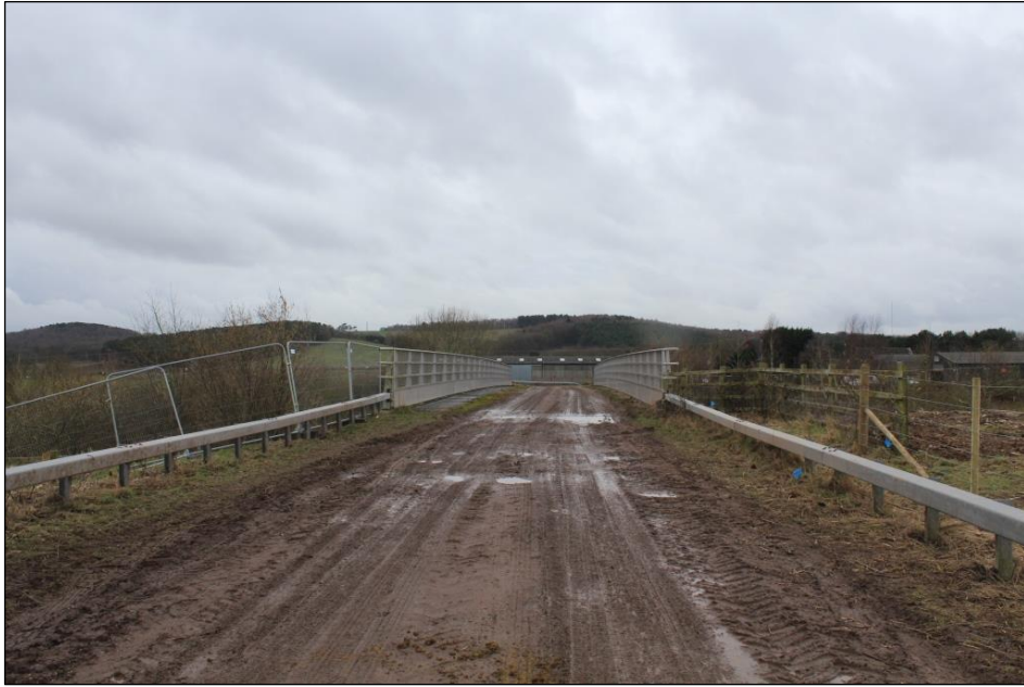
Plate 24: View south across the footbridge over the course of the A5.
