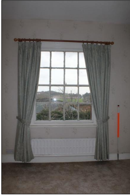
Plate 82: Sash window within the eastern wall of Room 26, Building 1.
