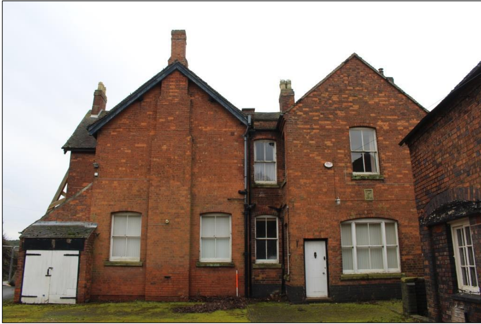
Plate 34: The northern elevation of Building 1.
