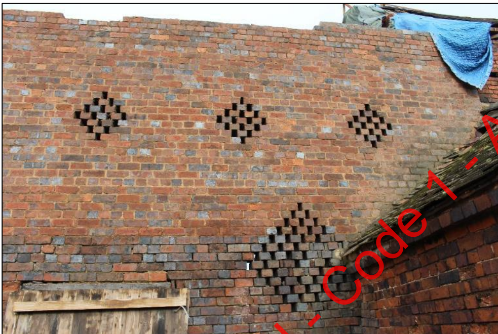
Plate 227: The diamond shaped ventilator brickwork in the southern elevation of Building 8.
