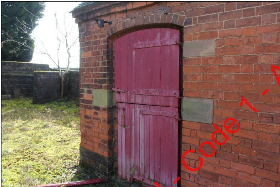
Plate 286: One of the stable doors in the northern elevation of Building 12.
