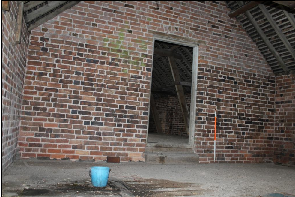
Plate 156: The southern wall of Room 6, Building 3, viewed from the north-east.
