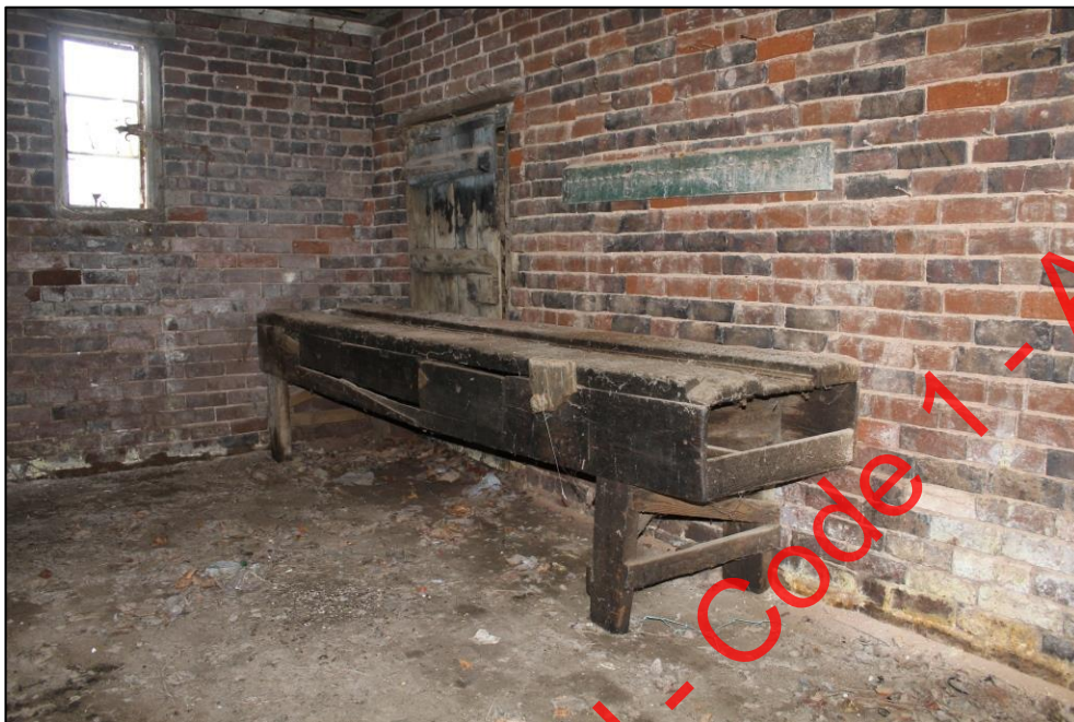
Plate 185: The northern and eastern walls of Room 4, Building 5.
