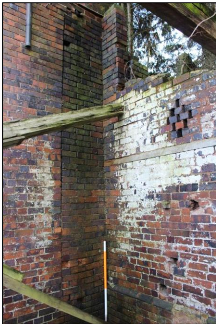
Plate 117: The south-eastern corner of the eastern stable (Room 15).
