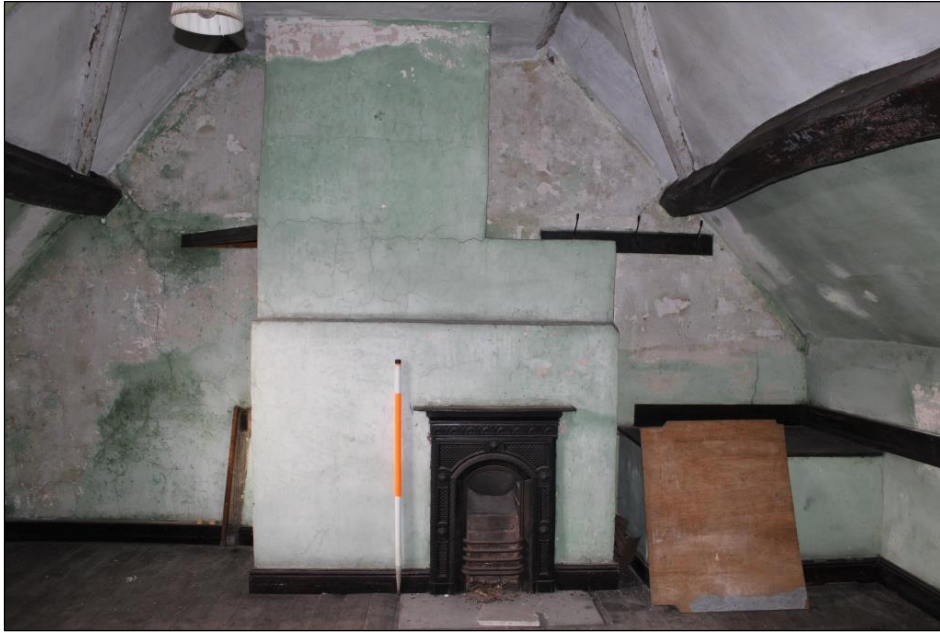
Plate 100: The western wall of Room 34.
