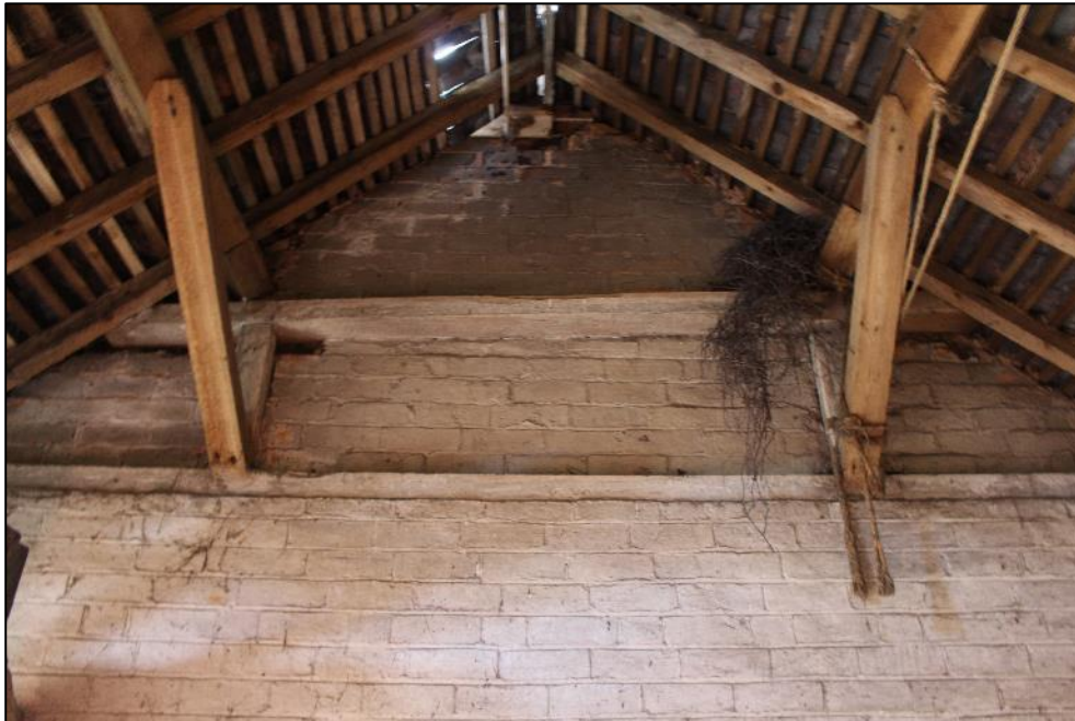
Plate 299: The eastern wall in the southern room of Building 11.
