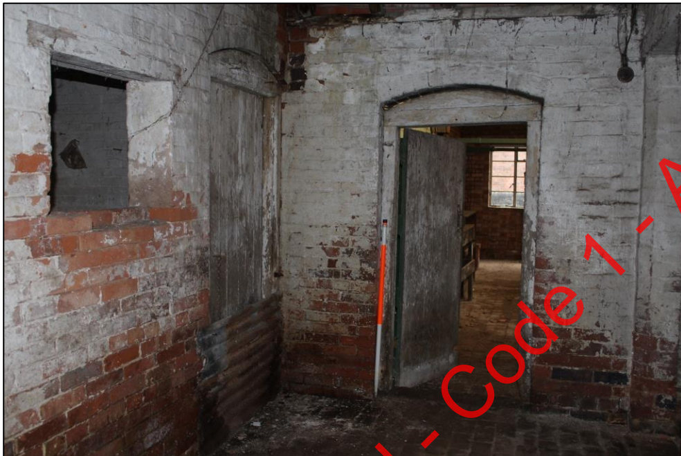
Plate 167: The southern and eastern walls of Room 9, Building 4.
