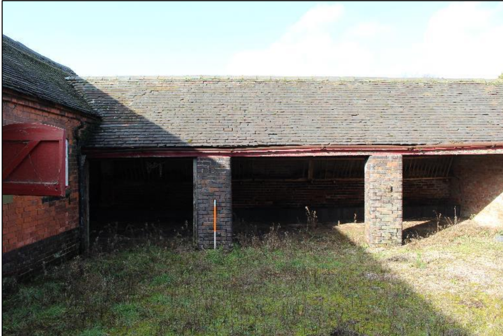
Plate 287: The southern side of the eastern elevation of Building 11.
