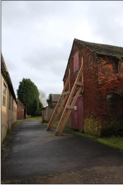
Plate 20: View east across the northern half of the farm complex.
