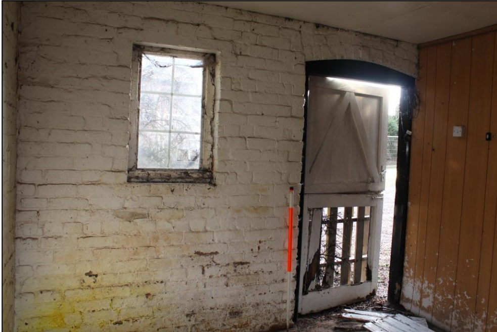
Plate 148: The eastern wall of Room 3, Building 3, viewed from the west.
