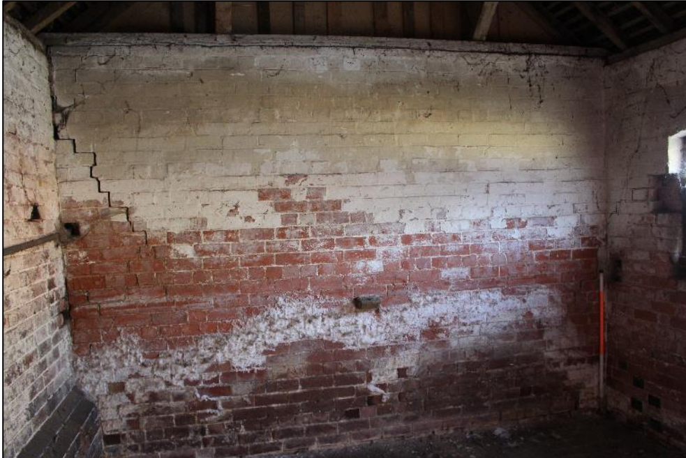
Plate 307: The western wall in the central stable of Building 12.
