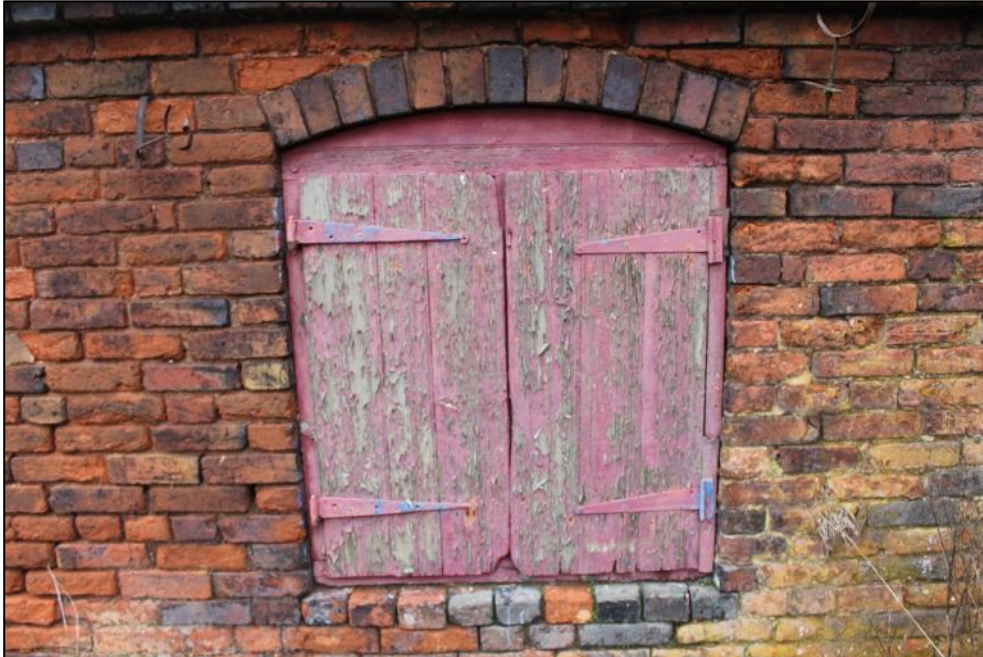
Plate 256: The hinged window in the southern elevation of Building 10a.
