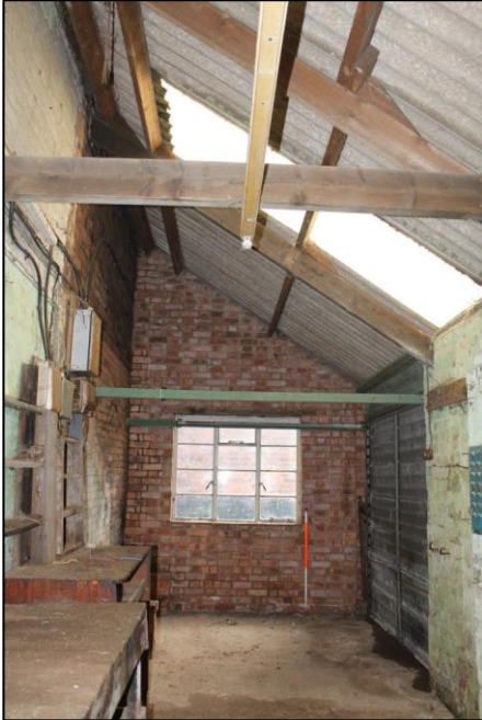
Plate 170: The southern extent of Room 10, Building 4, viewed from the north.
