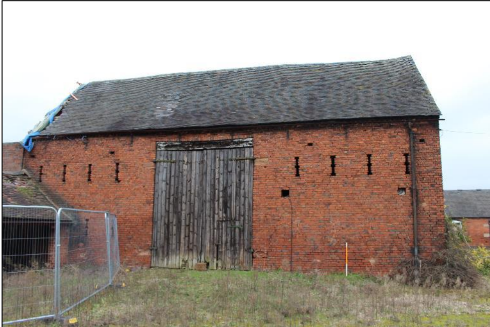
Plate 208: The southern elevation of Building 7.
