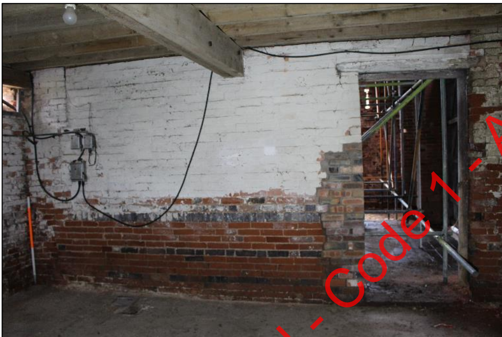
Plate 221: The western wall in the eastern room of Building 7.
