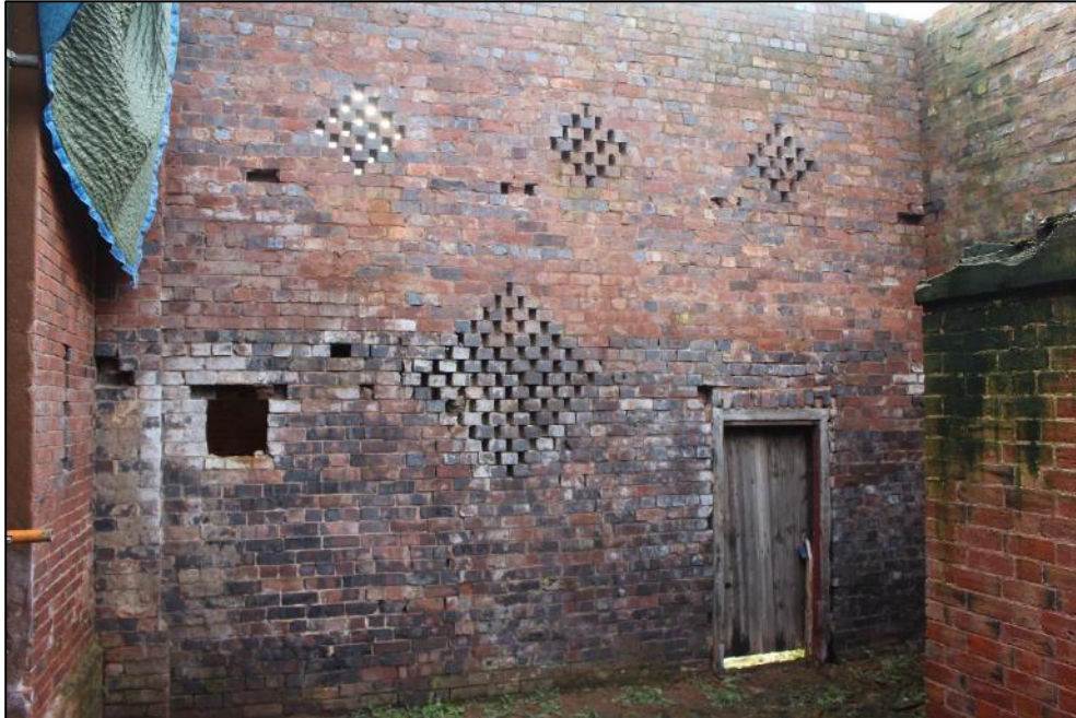
Plate 238: The southern wall inside Building 8.
