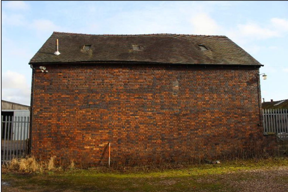
Plate 190: The western elevation of Building 6.
