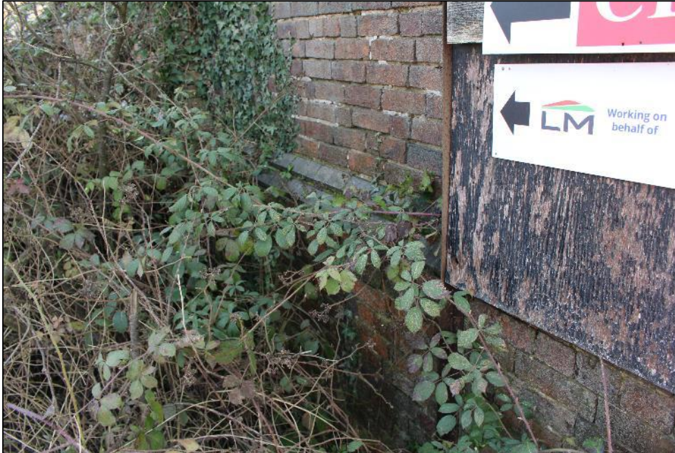
Plate 291: The plinth on the western elevation of Building 11.
