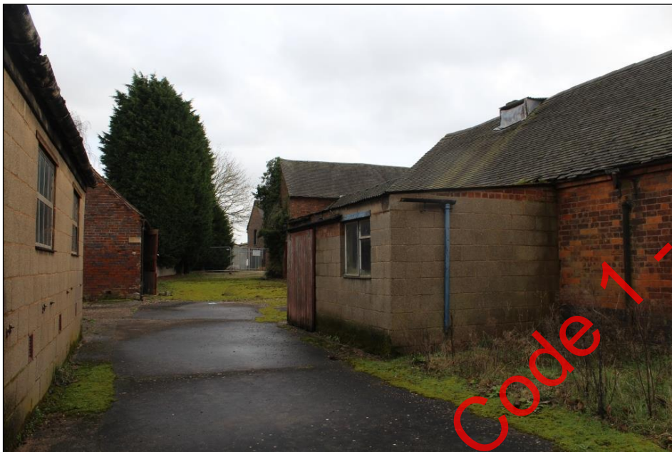
Plate 19: View east across the northern half of the farm complex.
