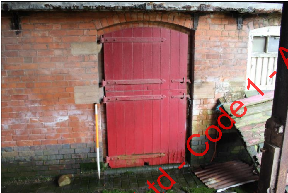
Plate 241: One of the timber doorways in the southern elevation of Building 9.
