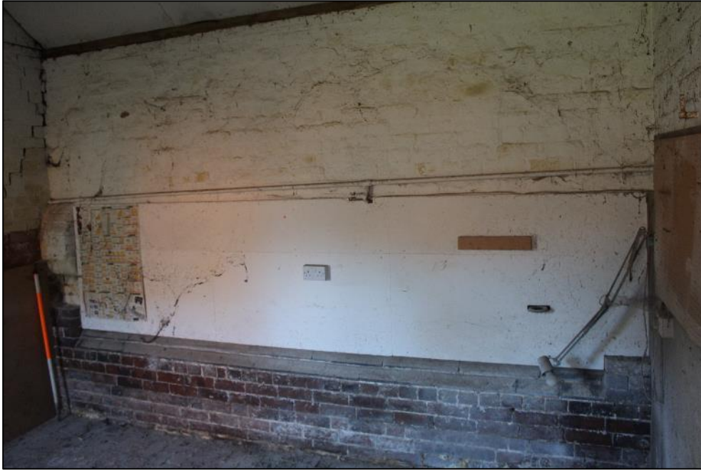
Plate 309: The southern wall in the western stable of Building 12.
