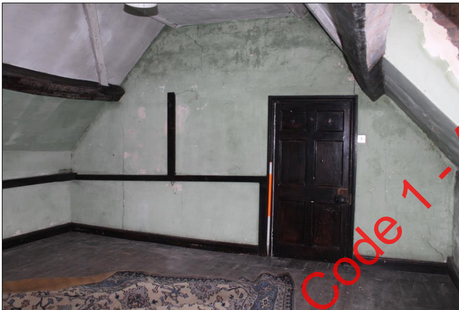
Plate 101: The eastern wall of Room 34.
