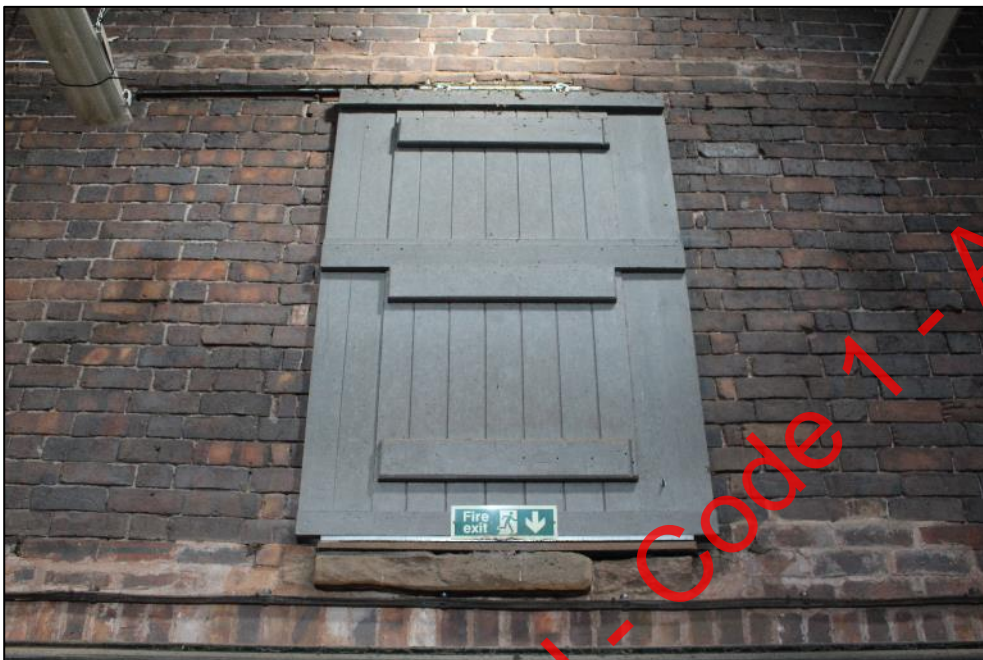
Plate 197: The first-floor window in the northern wall of Building 6.
