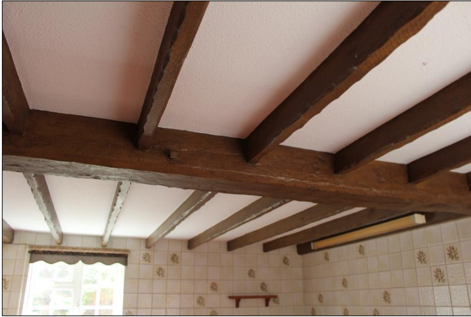
Plate 42: Cross beam and joist ceiling construction within Room 2, Building 1.
