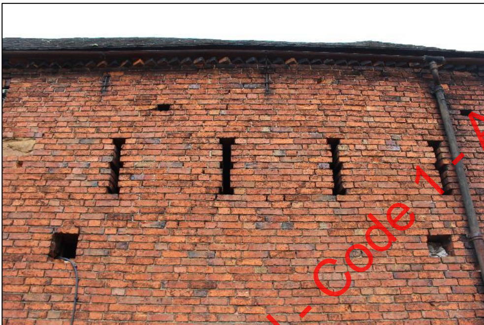
Plate 209: The ventilation slits and holes in the southern elevation of Building 7.
