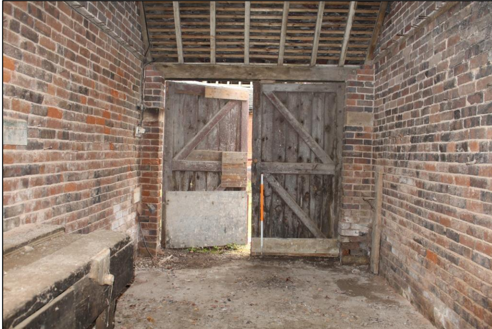
Plate 184: The southern wall of Room 4, Building 5.
