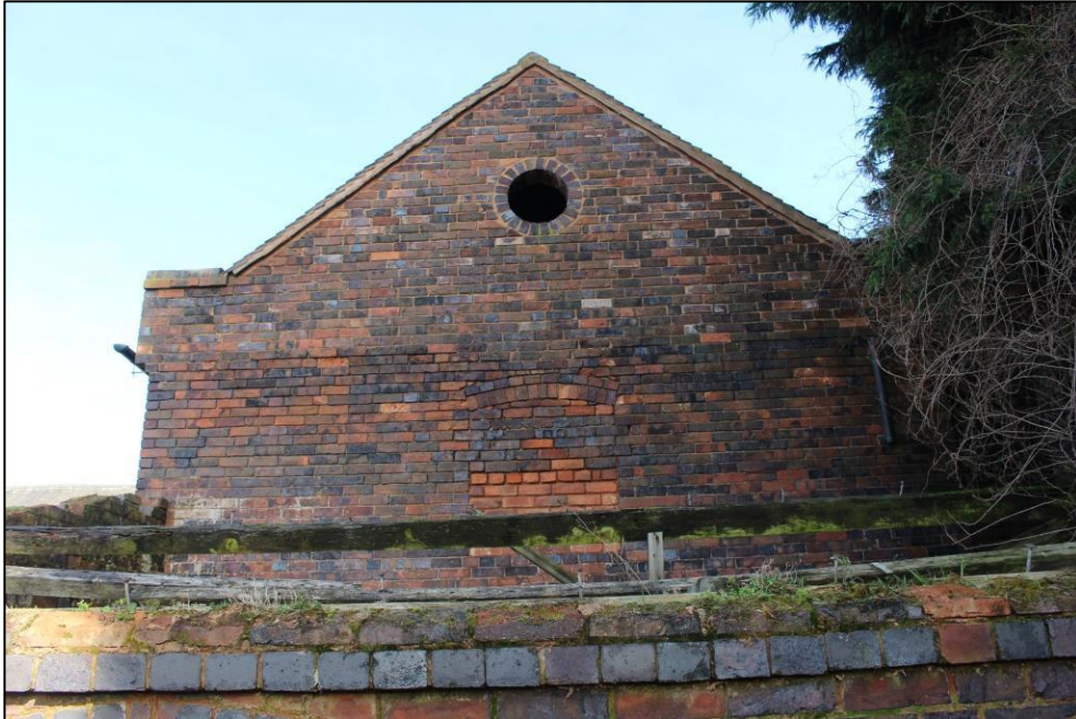
Plate 114: The southern gable of Building 2.
