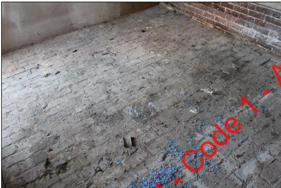
Plate 312: The floor surface of the western stable of Building 12. The floors are identical in all three of the stables.
