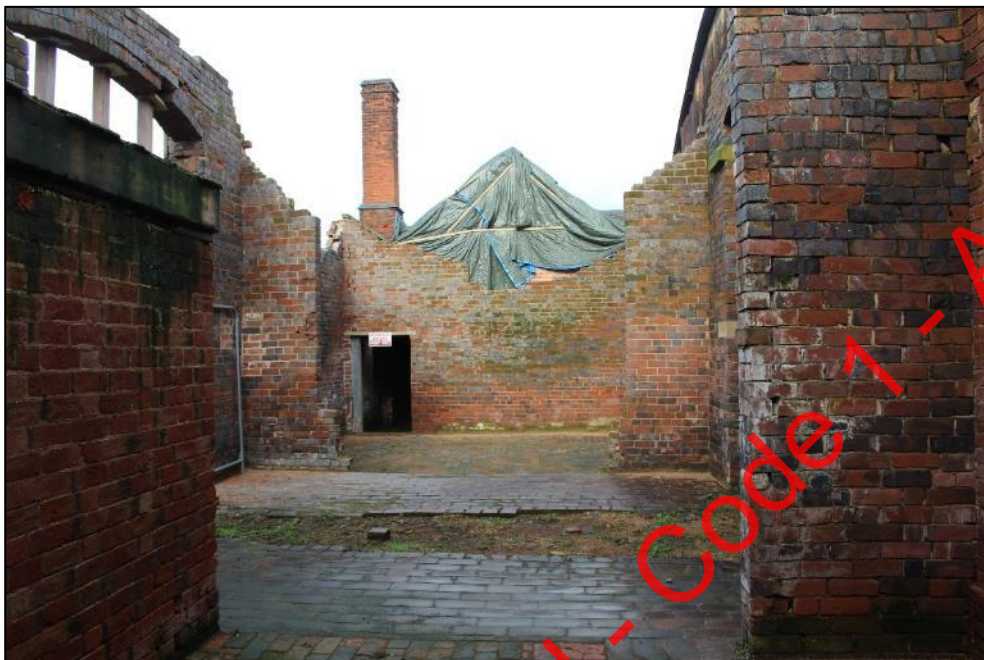
Plate 239: Facing north from the southern end of Building 8.
