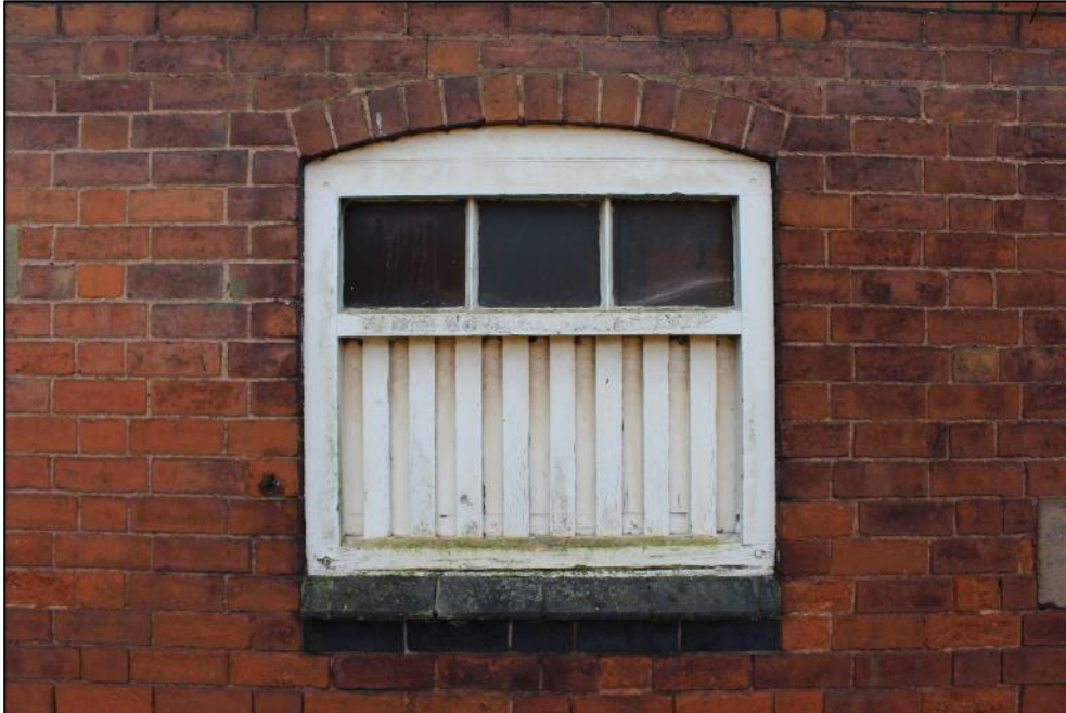
Plate 285: One of the louvred windows in the northern elevation of Building 12.
