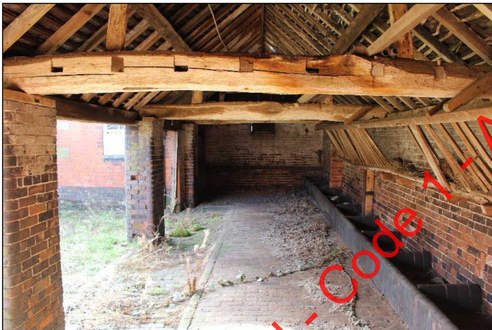
Plate 300: The southern room in Building 11, showing the detail of the northernmost truss.
