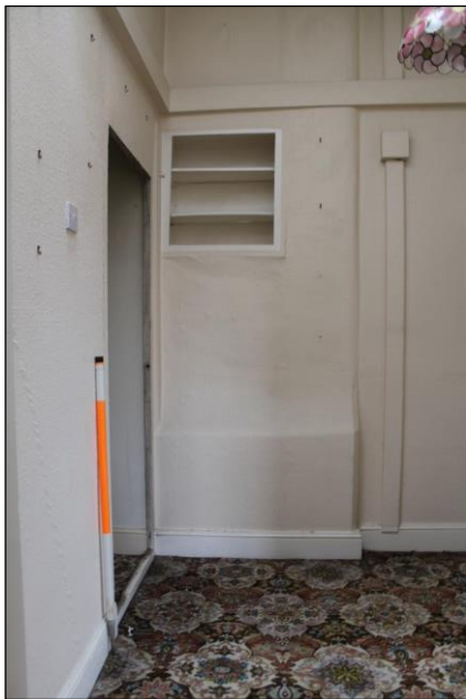
Plate 83: The south-eastern extent of Room 23, Building 1.
