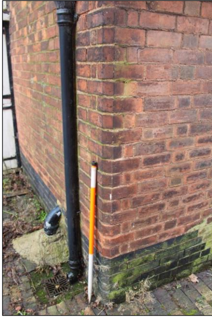
Plate 38: Chamfered brickwork detail to the north-eastern corner of the wash house.
