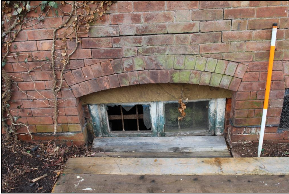
Plate 32: Cellar window set at ground level within the eastern elevation.
