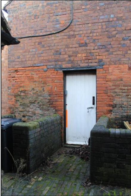
Plate 130: Detail of door opening within the southern gable of Building 3.
