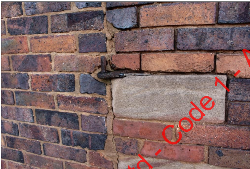
Plate 111: Detail of quoin stones with former door pintel adjacent to the blocked door opening within the western elevation of Building 2.
