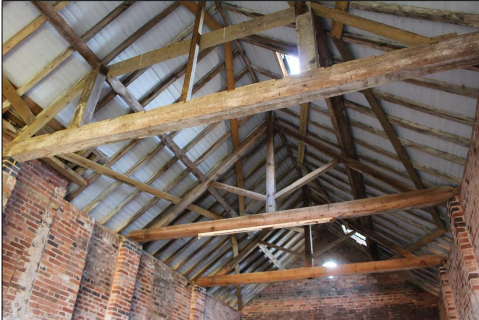
Plate 124: Overview of the roof structure of Building 2, viewed from the north-west.
