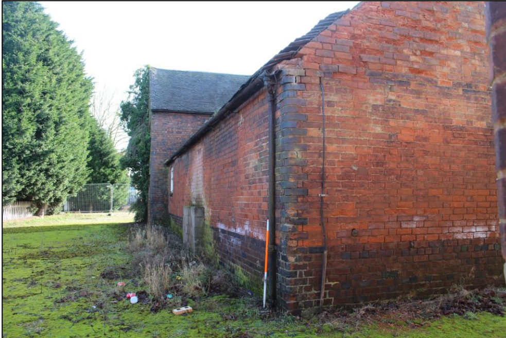
Plate 136: The western extent of the northern elevation of Building 4.
