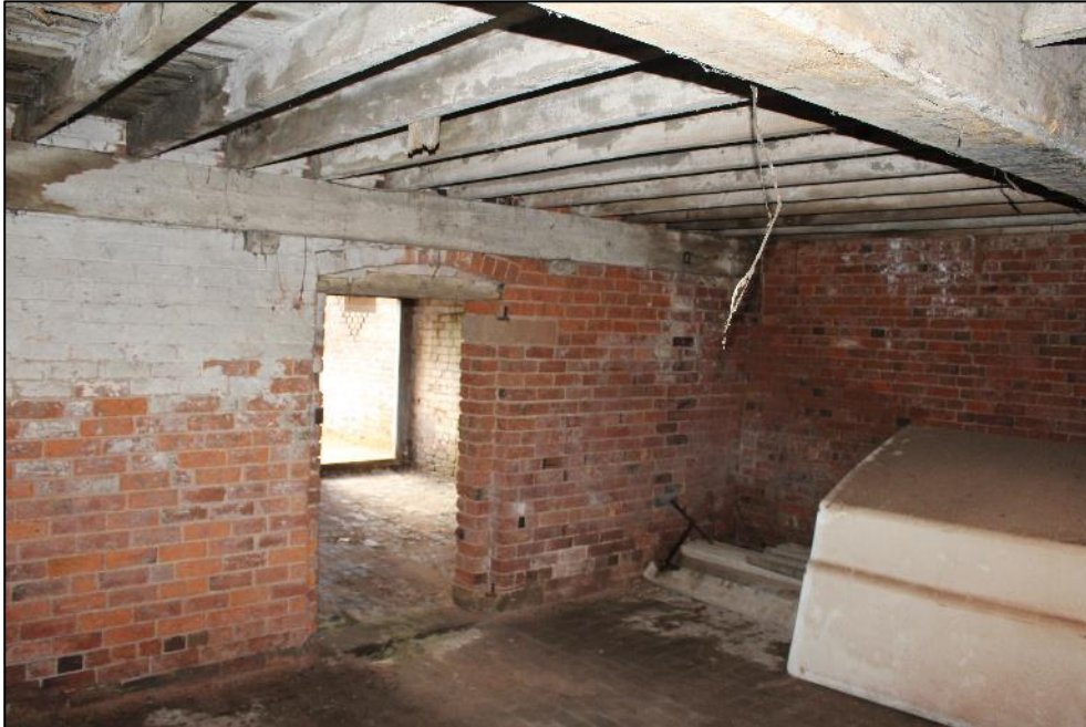
Plate 277: The brick dividing wall in the centre of Building 10b.
