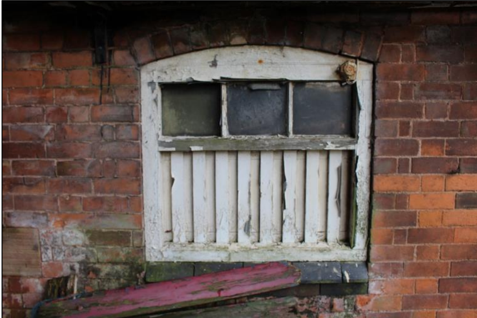
Plate 242: One of the louvred windows in the southern elevation of Building 9.
