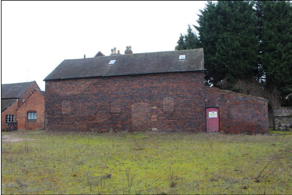
Plate 108: An overview of Building 2 from the west.
