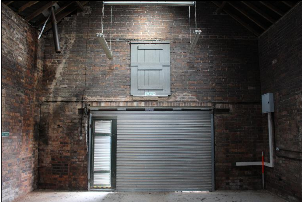
Plate 196: The northern wall in the northern half of Building 6.
