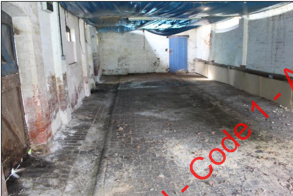
Plate 249: Facing west in Building 9.
