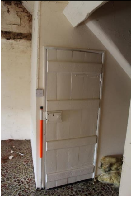
Plate 90: Timber plank door within the north-western corner of Room 31, Building 1.
