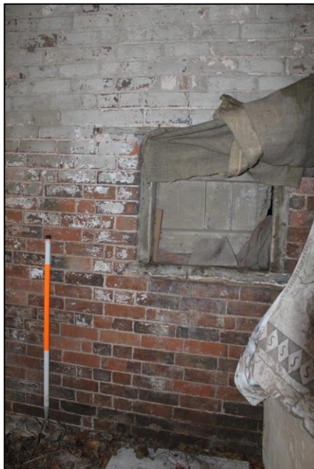
Plate 153: Detail of hatch opening within the southern wall of Room 5, Building 3.
