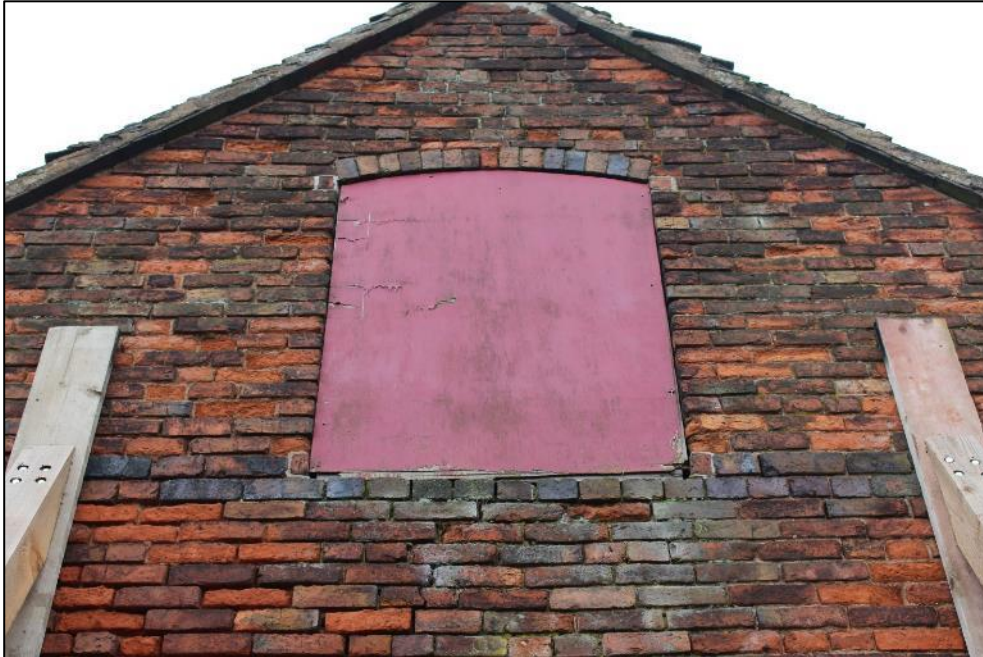
Plate 265: The pitching window in the northern gable end of Building 10b.
