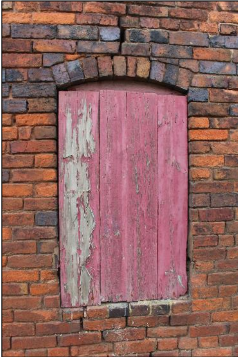
Plate 260: The window in the eastern gable end of Building 10a.
