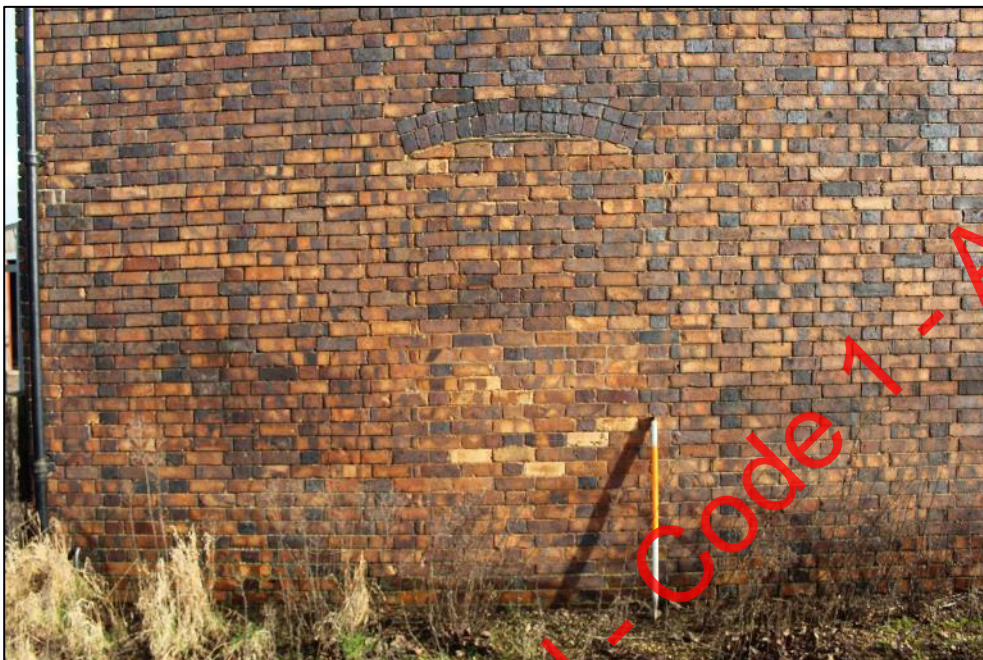
Plate 191: The blocked feature in the western elevation of Building 6.
