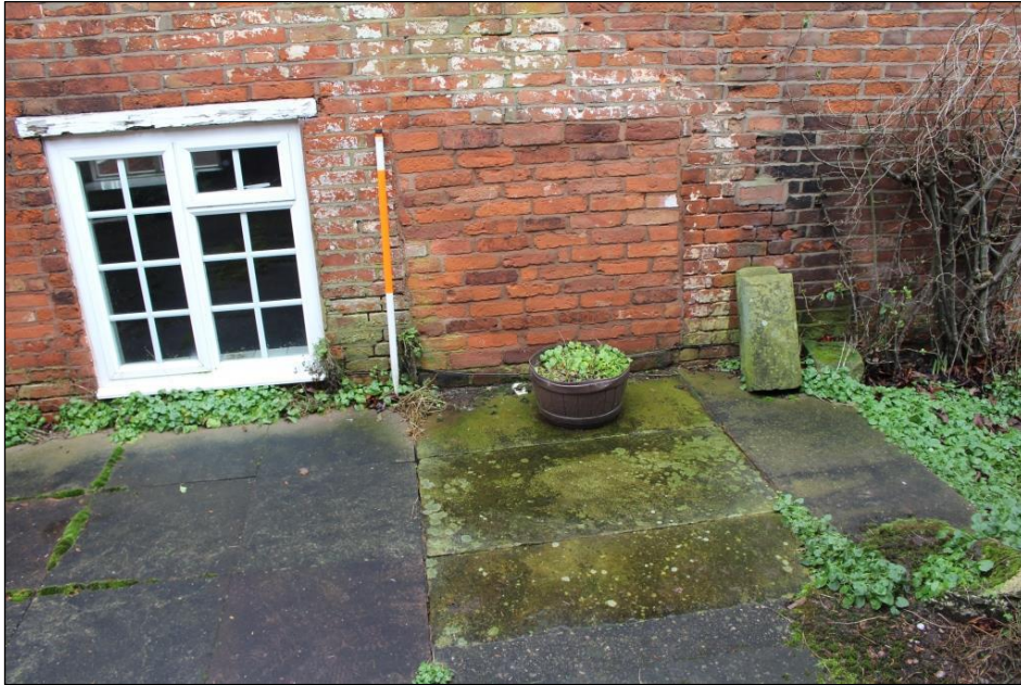
Plate 30: Blocked opening and covered steps to the southern elevation of the western range.
