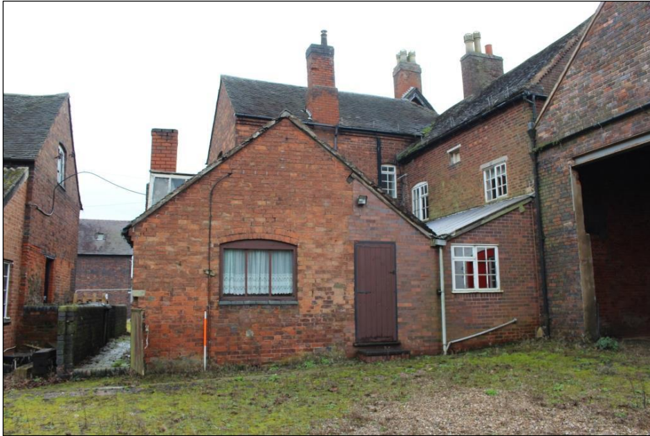
Plate 40: Building 1 and the wash house, viewed from the west.
