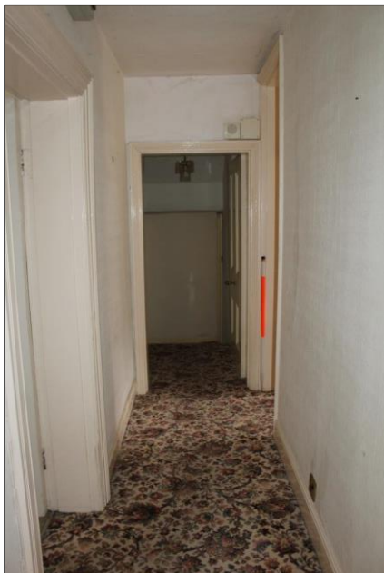
Plate 47: Overview of Room 4 from the east.
