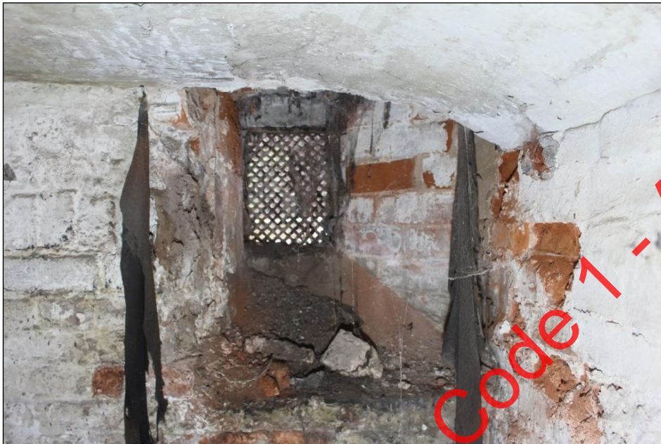
Plate 69: Vent and ash box within the western wall of Room 17, Building 1.
