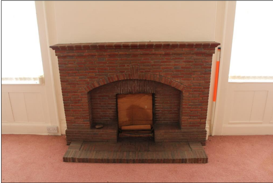
Plate 54: Fireplace set within the northern wall of Room 10, Building 1.
