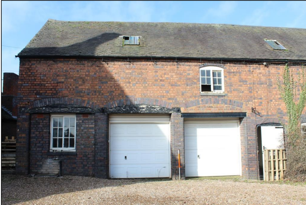
Plate 126: The southern extent of the eastern elevation of Building 3.
