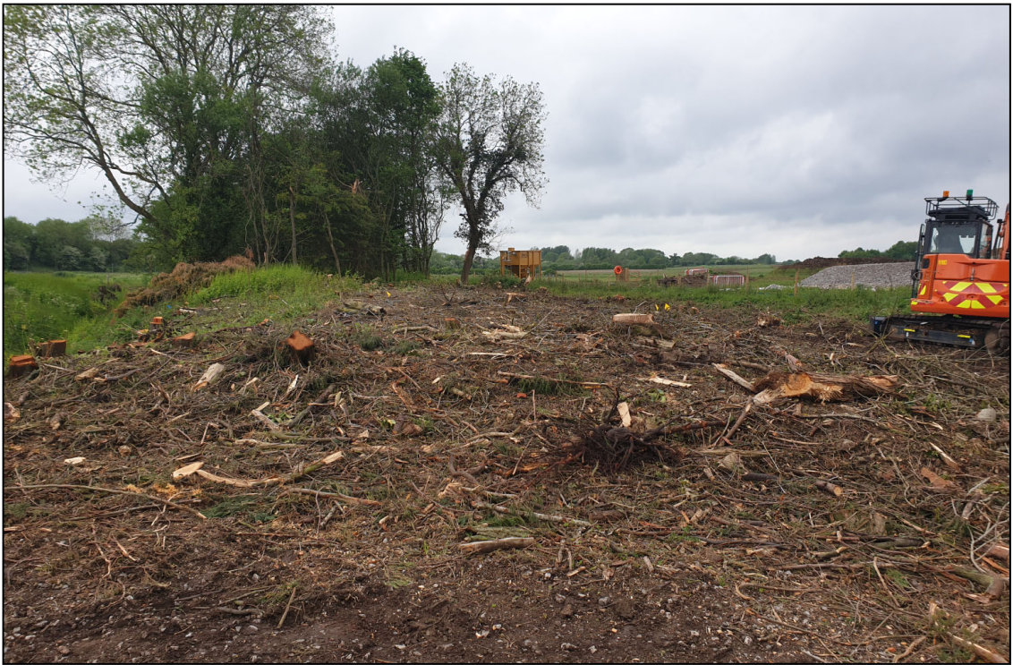
Monitoring of tree root removal, looking west.
