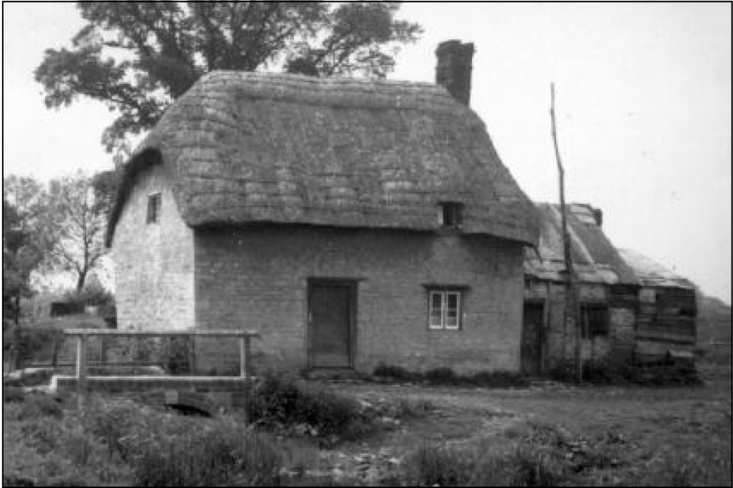
Old mill house in 1939
