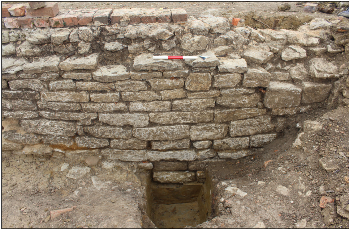
Northern head race/mill race wall 184, looking north-east (0.3m scale)
