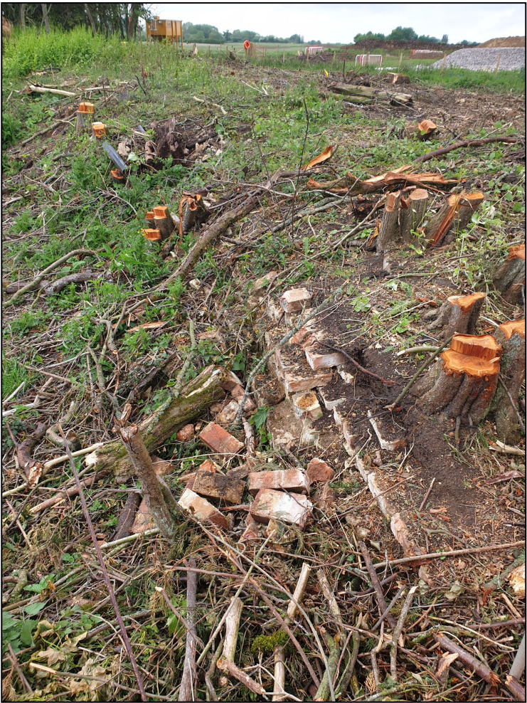
Head race/mill race wall 184 prior to tree root removal, looking west.
