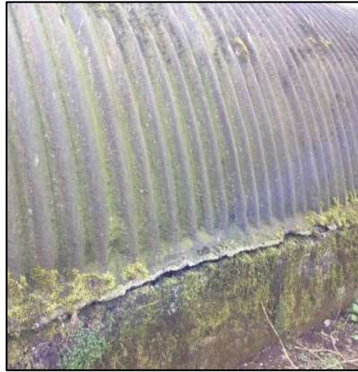
4. Asbestos sheeting & concrete base
