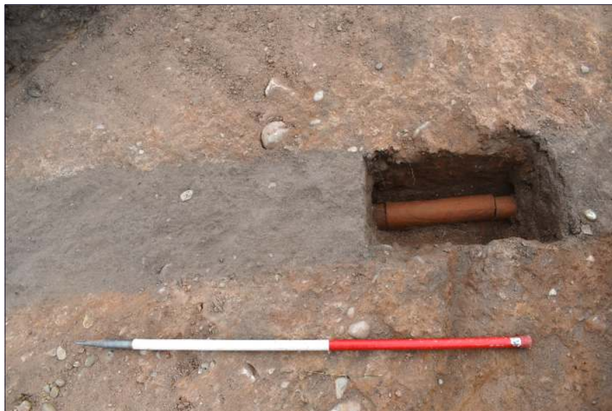
Plate 8: Excavated section of a land drain (1m scale)
