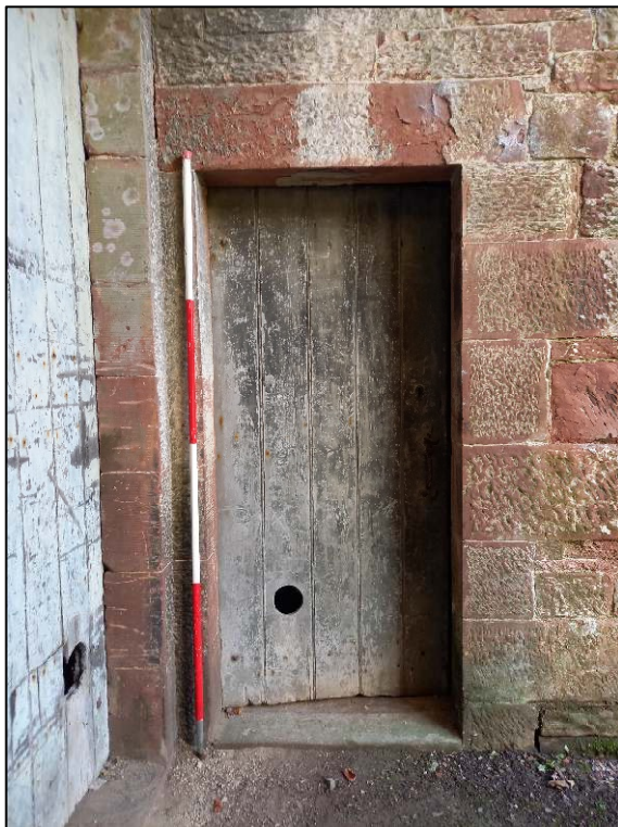
Plate 34: Door in north elevation of the southern projection (Scale = 2m)
