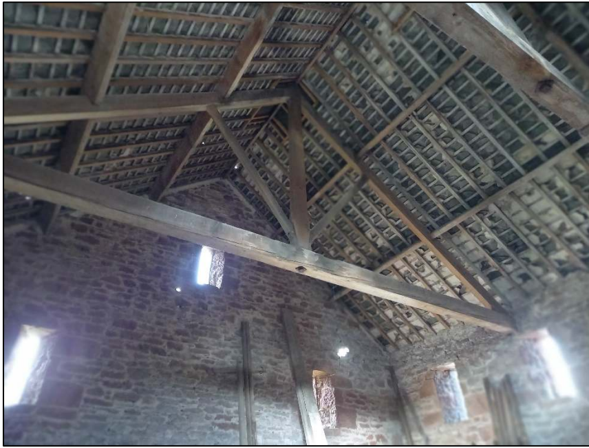
Plate 71: Detail of roof structure, first floor of barn
