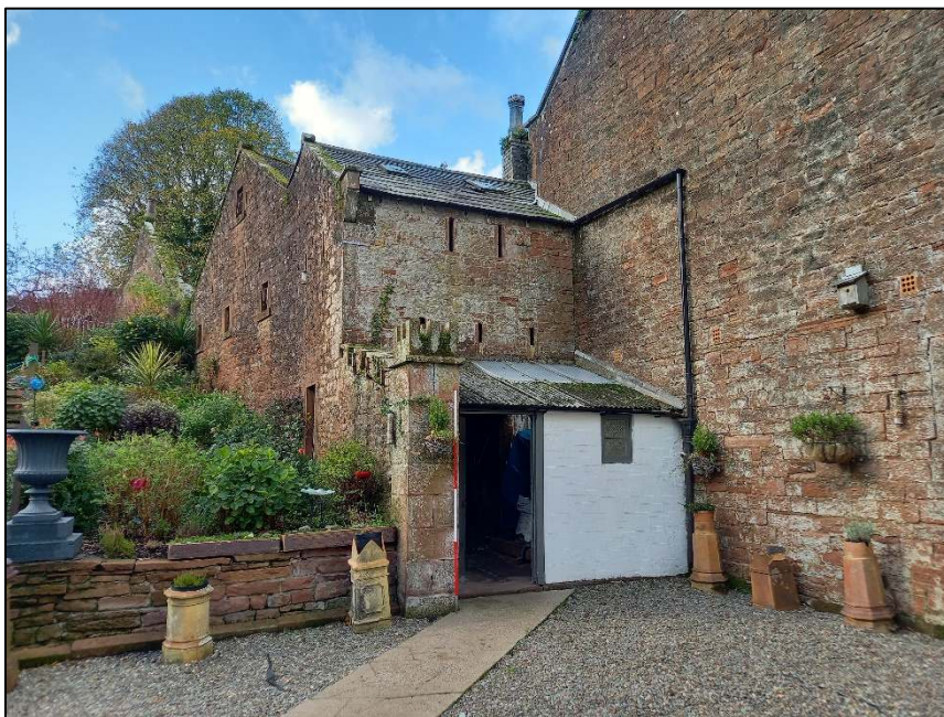
Plate 22: View looking west from the rear of the house showing the south elevation of the barn (right) and later additions including a white-washed lean-to defined to its south side by a section of crenellated wall
