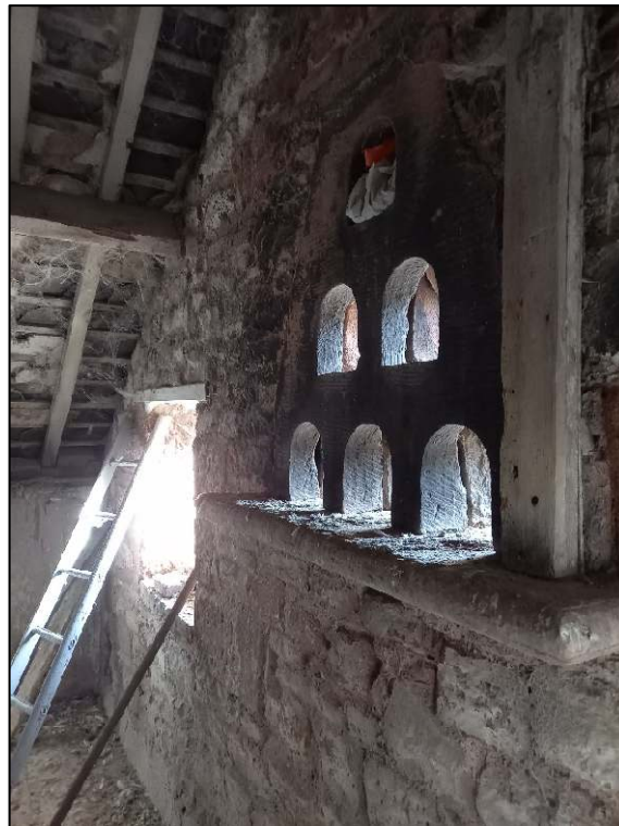
Plate 68: Detail of pigeon holes, southern gable of the barn
