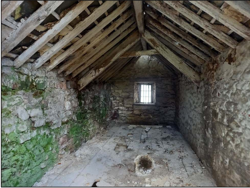
Plate 107: View looking east showing the first floor of the Henry-Piggery
