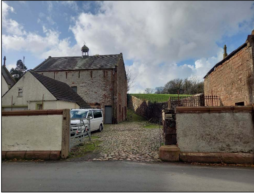
Plate 5: View looking west towards the barn from Morass Road, showing the cobbled yard, entrance gateway and Hennery-Piggery to right of photograph
