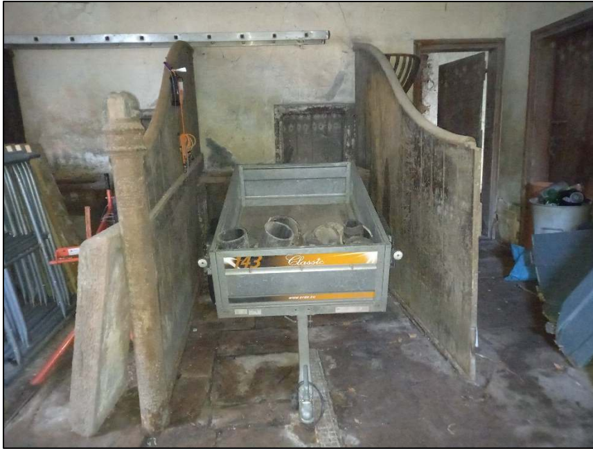
Plate 43: Detail of one of the stalls showing the dividers and the small door at the rear of the stall for moving feed into the racks (Room A)
