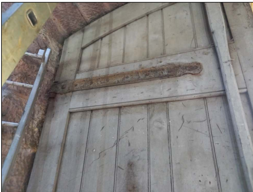
Plate 70: Detail of strap hinge, door to first floor of barn, west elevation
