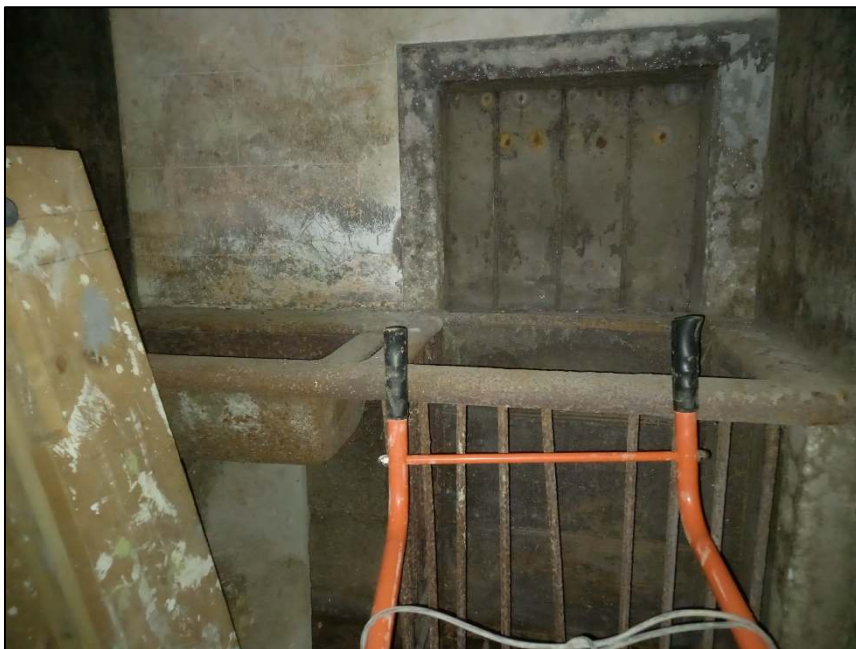
Plate 44: Detail of metal feeding trough and rack, with wooden feeding door, west wall of one of the stable stalls (Room A)
