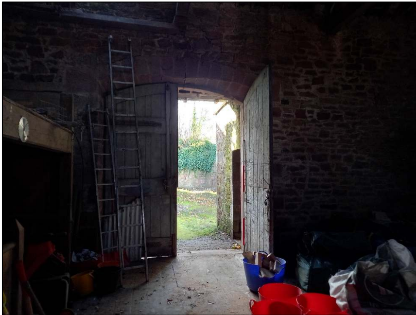
Plate 69: Detail of large doorway into the first floor of the barn, west elevation
