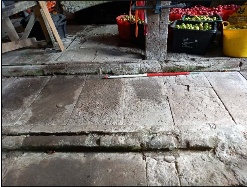
Plate 51: View looking east showing the central passageway/manure channel with slots for possible former wooden stall dividers (Room B) (Scale = 1m)
