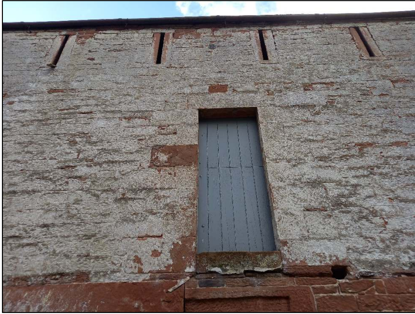
Plate 15: First floor winnowing or pitching door, east elevation of barn
