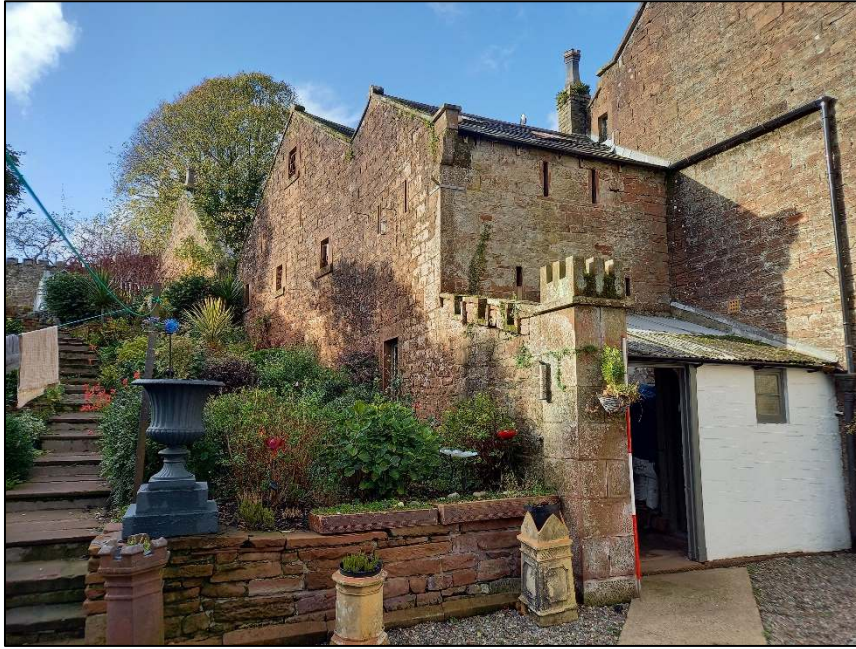
Plate 77: View looking west showing the ancillary buildings constructed to the west of the earlier barn
