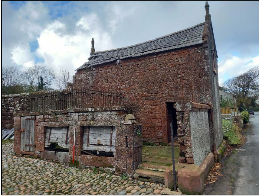
Plate 97: South elevation of the Hennerly-Piggery
