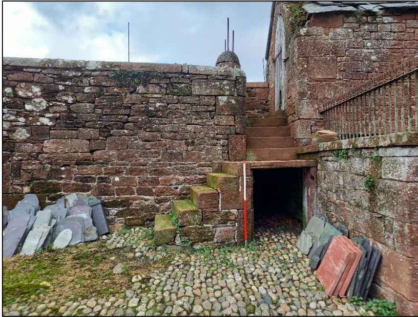
Plate 105: Stone staircase at the west side of the Hennery-Piggery (Scale = 1m)
