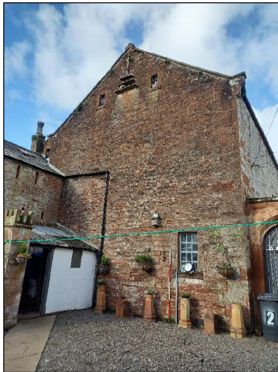
Plate 20: South elevation of the barn (Scale = 2m)
