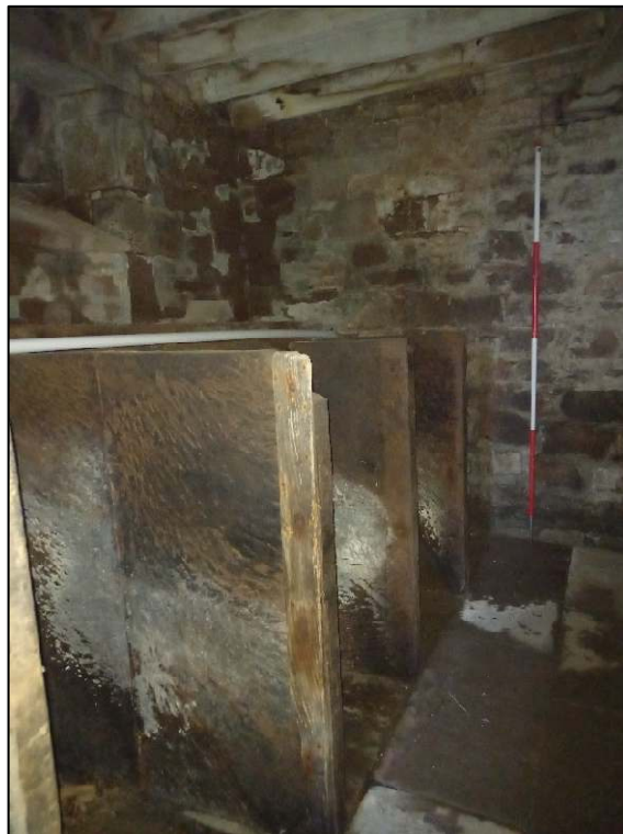
Plate 54: View looking north in Room E showing the stone bay dividers and stone flagged floor (Scale = 2m)
