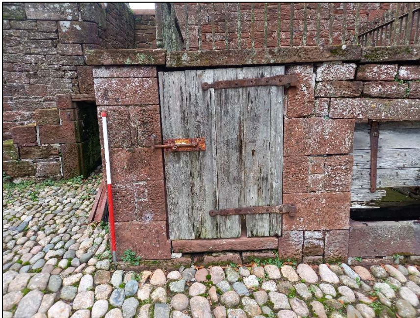
Plate 100: Detail of access door, south elevation of Hennerly-Piggery (Scale = 1m)
