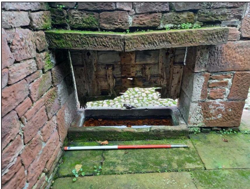
Plate 102: Internal view of one of the feeding troughs, Hennery-Piggery (Scale = 1m)
