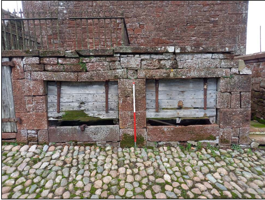
Plate 101: Detail of feeding hatches, south elevation of Hennery-Piggery (Scale = 1m)
