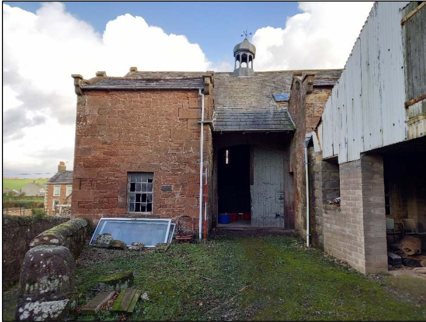
Plate 25: West elevation of the barn
