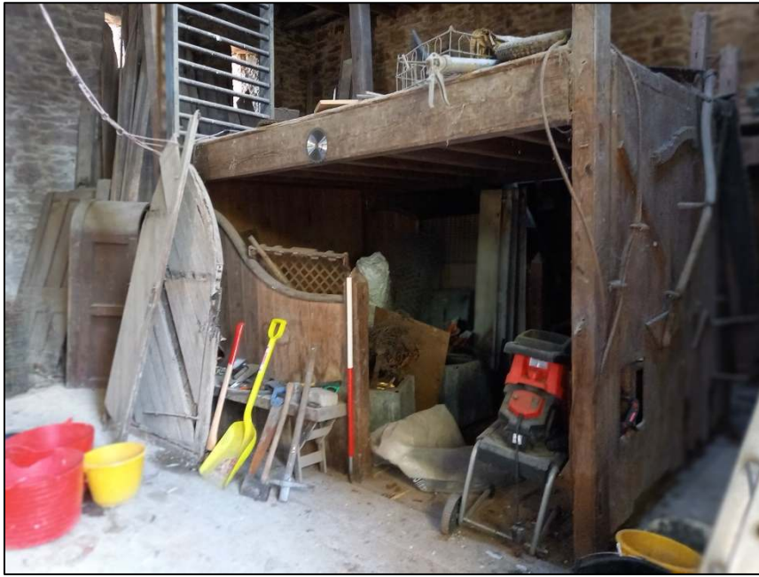
Plate 75: Possible reset stable dividers located on the first floor of the barn (Scale = 1m)
