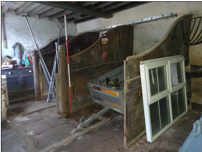
Plate 40: Ground floor of barn, showing stable stall dividers
