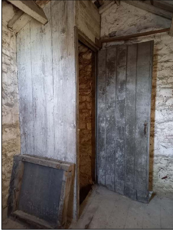
Plate 63: Upper floor of the southern projection showing the doorway set in a boarded partition
