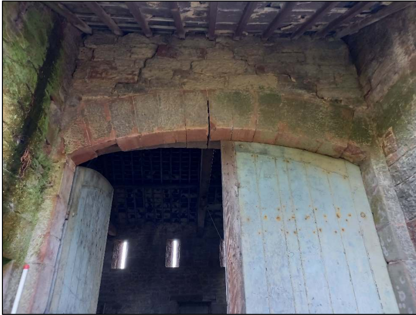
Plate 27: Detail of arched head of barn entrance, west elevation
