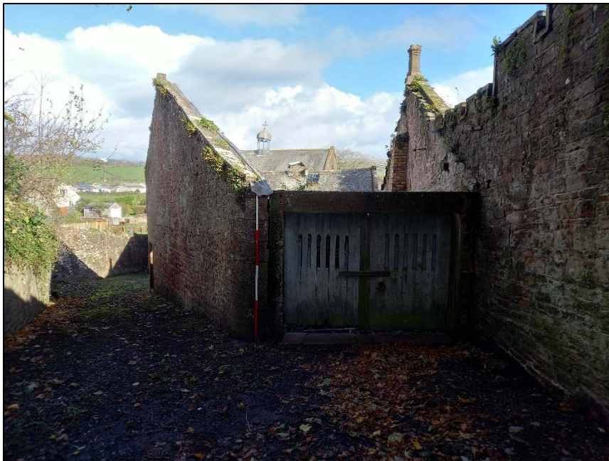
Plate 94: View looking east showing the west end of the ancillary buildings
