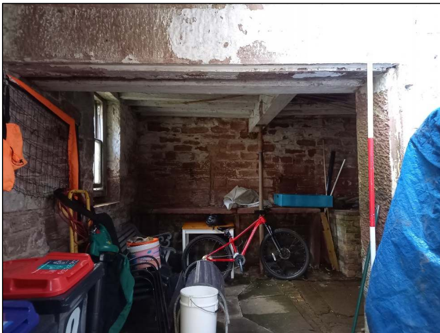
Plate 86: Large doorway in the east wall of the Wash House
