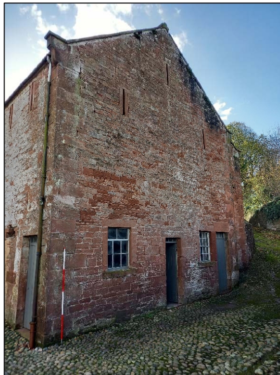
Plate 16: North elevation of the barn (Scale = 2m)
