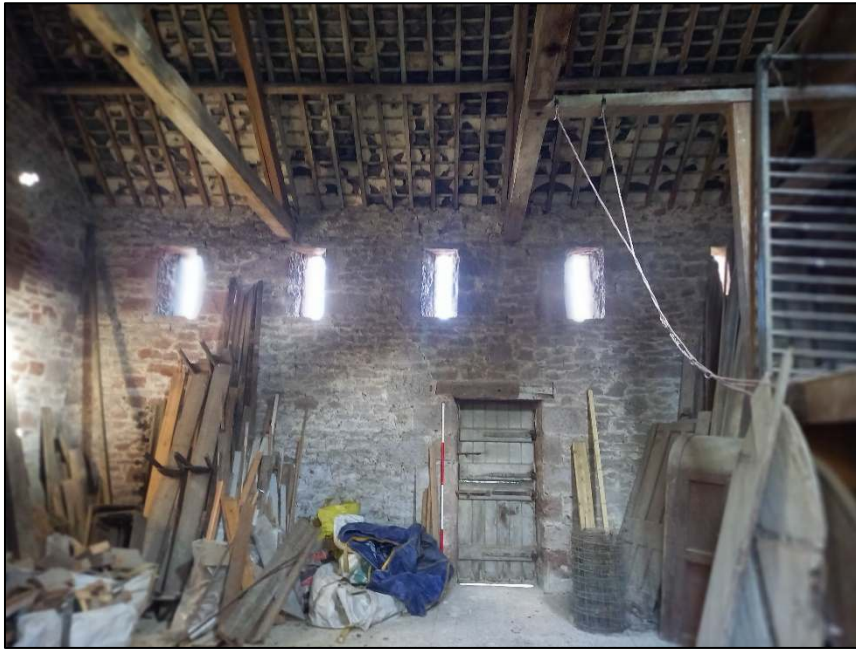
Plate 73: View looking east showing the doorway and ventilation slits in the east elevation, first floor of barn
