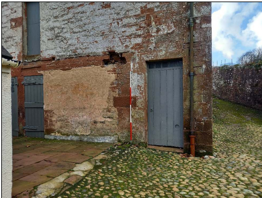
Plate 8: East elevation of the barn showing the northern doorway and scarring and stone floor of a former building (Scale = 2m)
