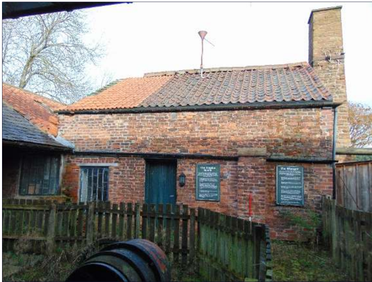
Plate 28: Southwest elevation of Building D, looking [12]
