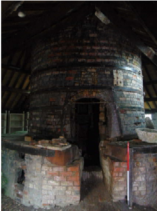
Plate 39: Beehive kiln (Building A), showing kiln entrance and central stack with iron belts, looking east
