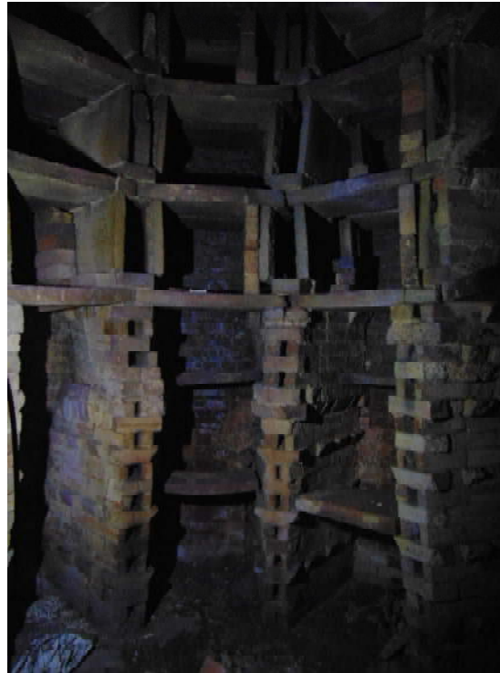
Plate 40: Detail of cupboards in the centre of the kiln, with shelves made of slabs of fireclay, looking east
