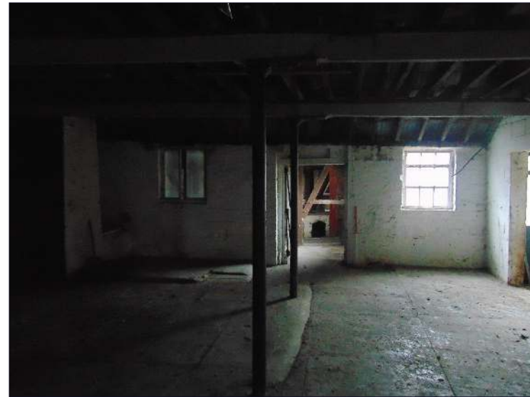
Plate 51: South end of the drying shed from Building C, looking northwest
