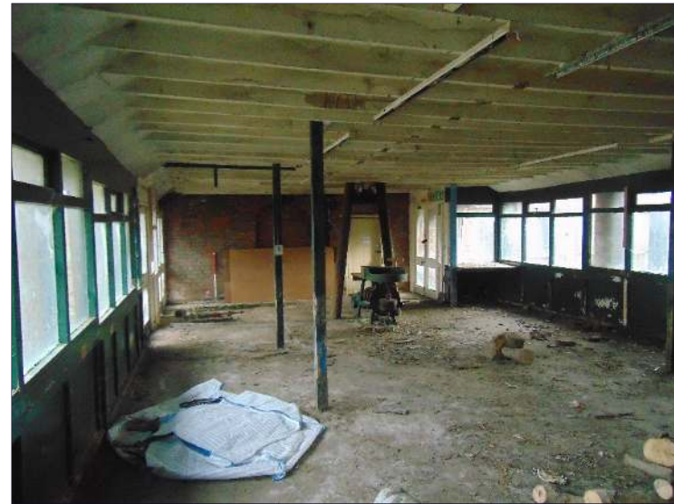
Plate 55: North end of the drying shed (Building C), looking northeast
