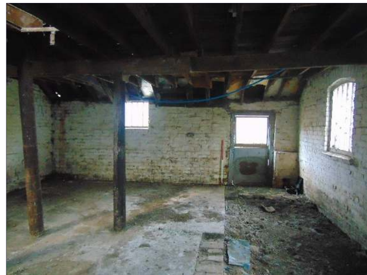
Plate 57: Workshop (Building D) with loft above, looking northwest
