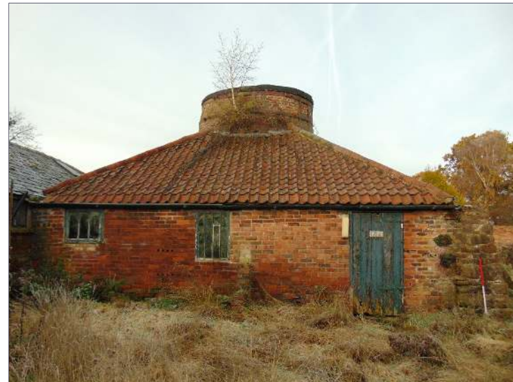
Plate 12: Southeast elevation of Building B, looking northwest [4]
