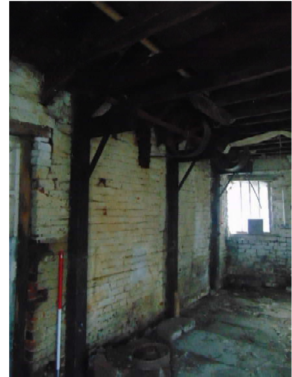
Plate 64: Drive belts in workshop, looking south
