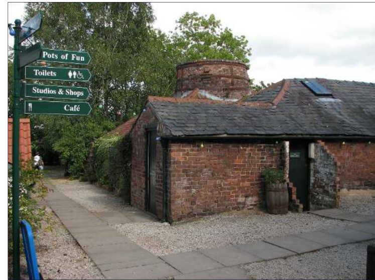
Plate 2: Area north of the beehive kiln and drying room in 2007
