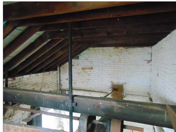
Plate 61: Rafters and power belt in engine room, looking northwest
