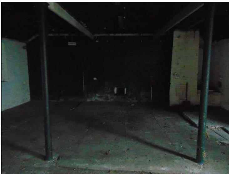
Plate 52: South end of Building C with chimney stack, looking southwest
