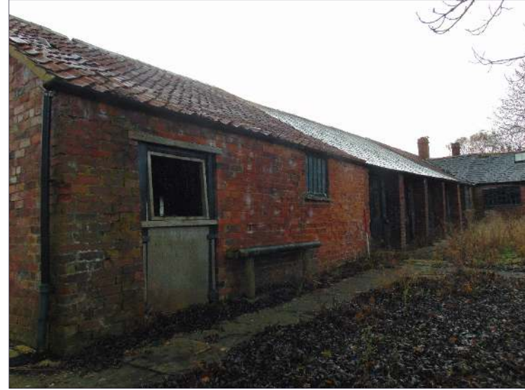
Plate 25: Northeast elevation of Building C and Building D, looking south [10]
