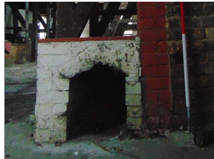
Plate 49: South end of drying shelf with chimney, looking northwest
