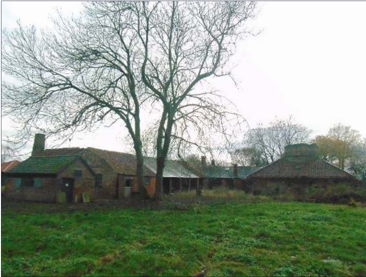
Plate 9: Location of survey buildings (A-D), looking south
