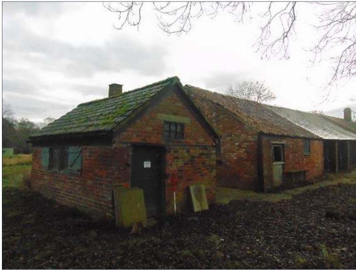
Plate 65: Pottery shed on the north side of the site, looking south [17]
