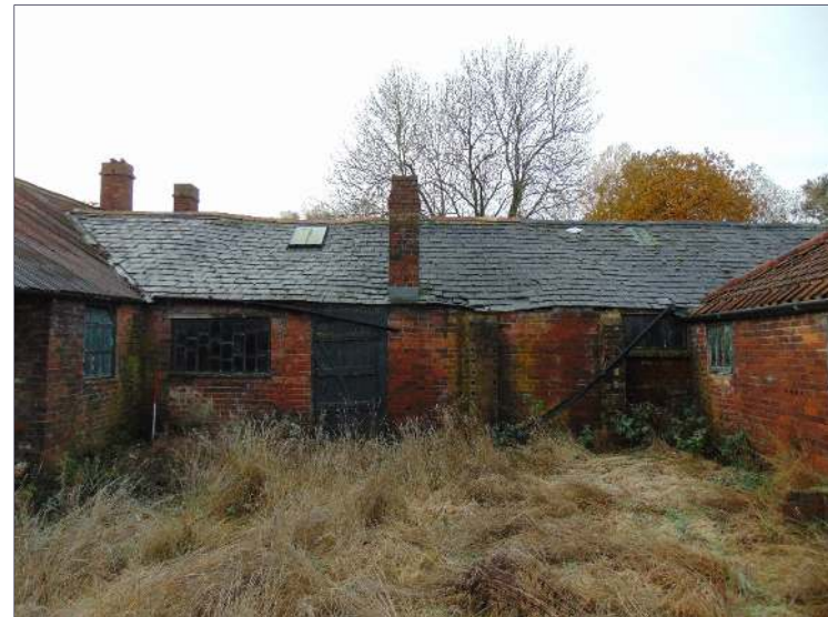
Plate 19: Northeast elevation of Building B, looking southwest [5]
