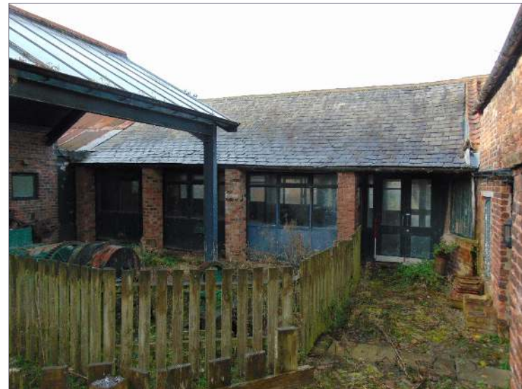
Plate 27: Southwest elevation of Building C, looking east [11]
