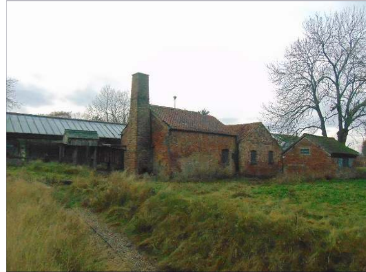
Plate 10: Location of boiler/engine house (D) and blunger (E), looking west [18]
