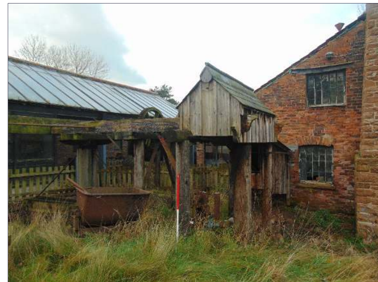
Plate 31: Southeast elevation of Building D with blunger, looking west
