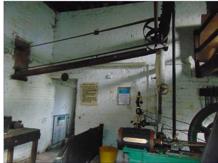
Plate 59: Engine room in Building D, looking north toward boiler room
