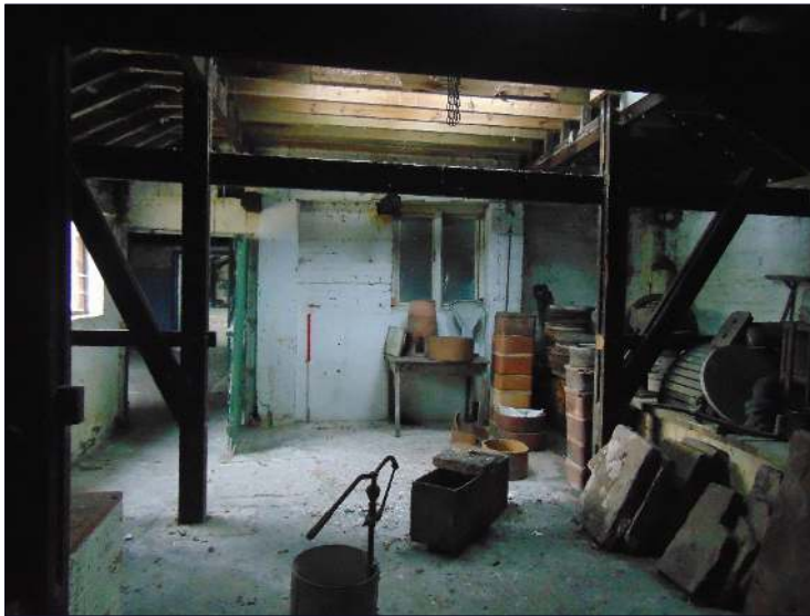
Plate 50: South end of the drying shed (Building B), looking southeast
