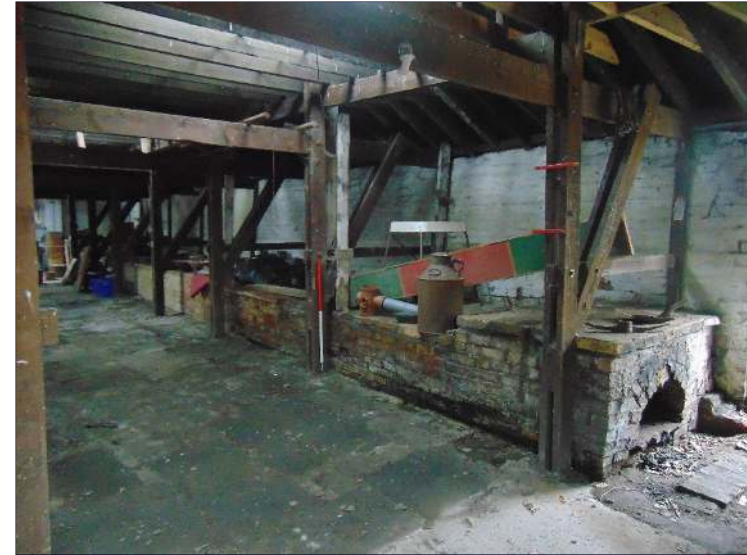
Plate 47: South side of the drying shed showing drying shelf, looking south
