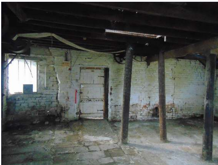
Plate 56: Deviding wall between Building C and Building D, looking southwest
