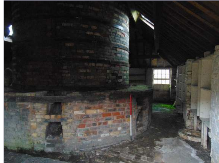
Plate 43: North side of the beehive kiln and fireboxes, looking northwest
