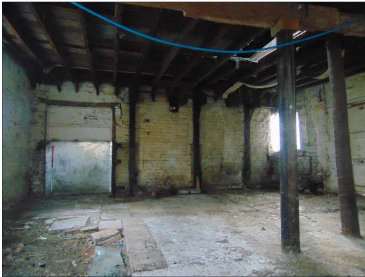
Plate 58: Workshop (Building D), looking southeast
