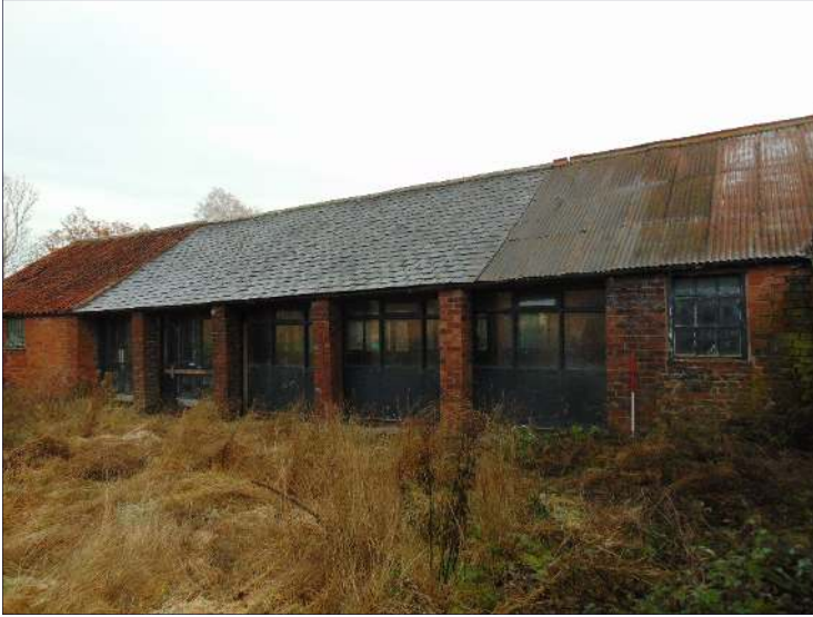
Plate 24: Northeast elevation of Building C, looking west [9]
