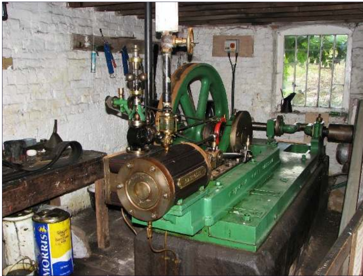
Plate 5: Inside the engine house at Wetheriggs Pottery in 2007
