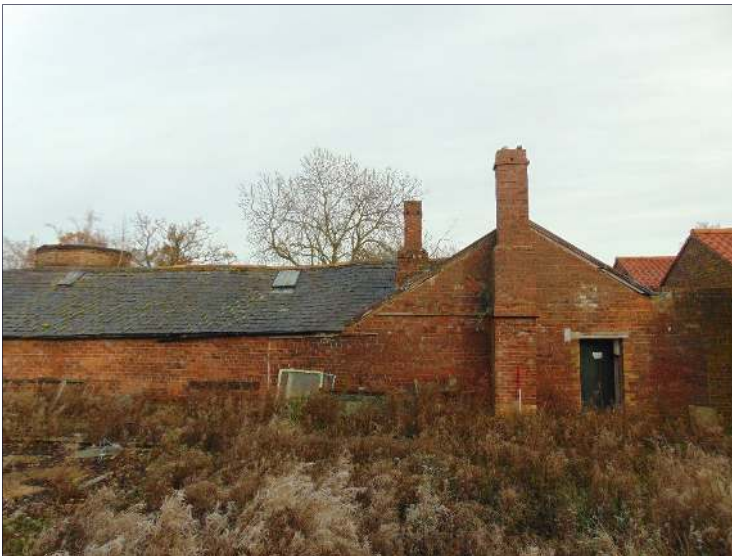
Plate 18: Southwest elevation of Building C, looking northeast [6]
