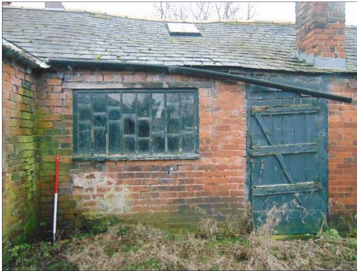
Plate 20: Detail of door and window in northeast elevation of Building B
