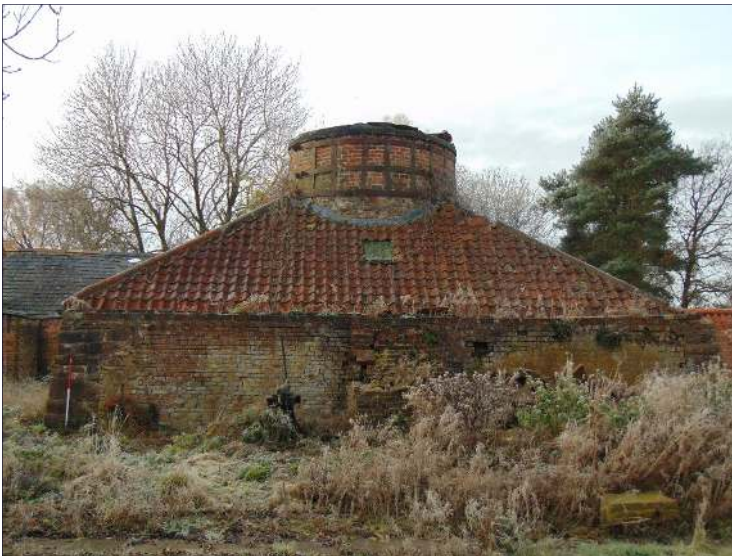
Plate 11: Northeast elevation of Building A, looking southwest [1]
