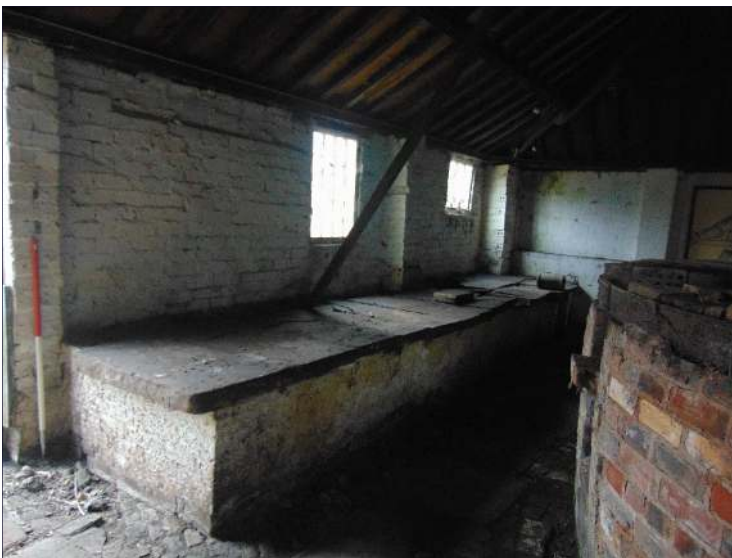
Plate 44: Drying shelf southeast of the beehive kiln, looking south
