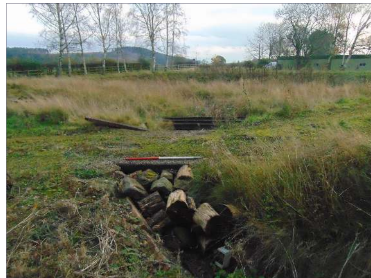
Plate 38: Outlet channel running beneath tramway to settling pan, looking east
