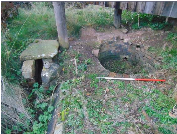
Plate 37: Outlet channel and well to north of the blunger, looking west
