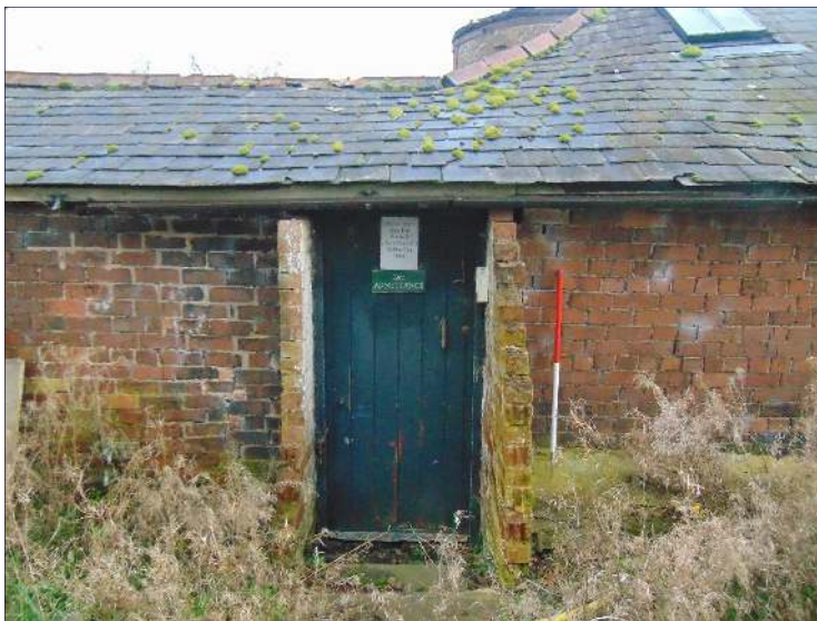
Plate 22: Door in southwest elevation of Building B, looking northeast
