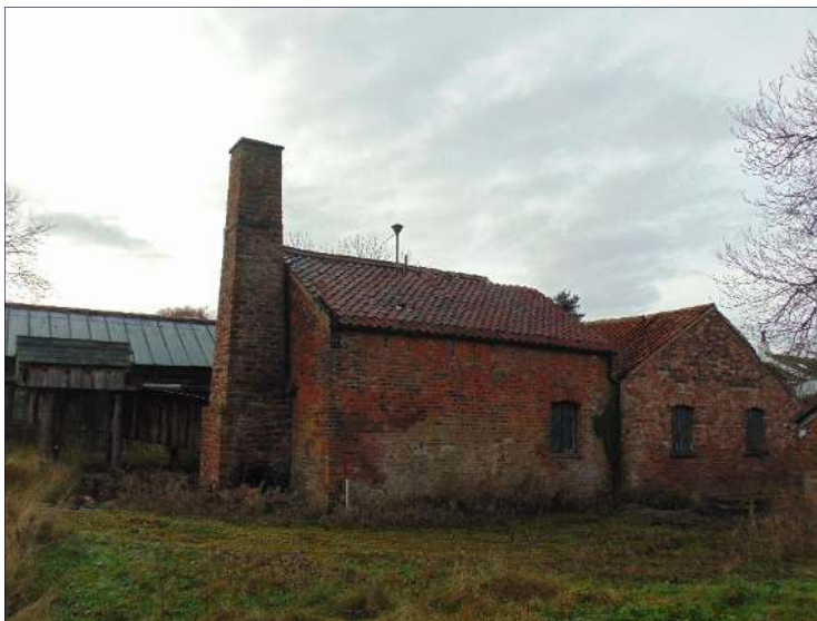
Plate 30: Northeast elevation of Building D, looking west [15]
