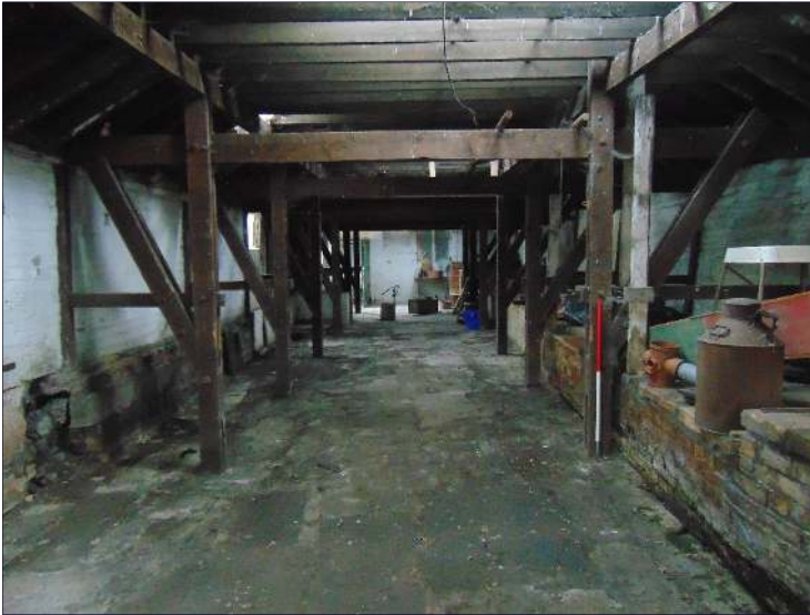
Plate 46: Interior of the drying shed (Building B), looking southeast
