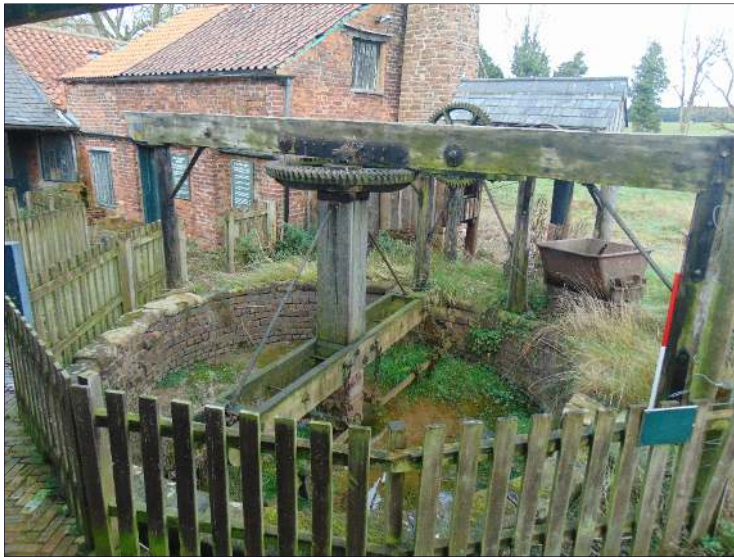
Plate 35: Support structure for the blunger (Building E), looking north [20]
