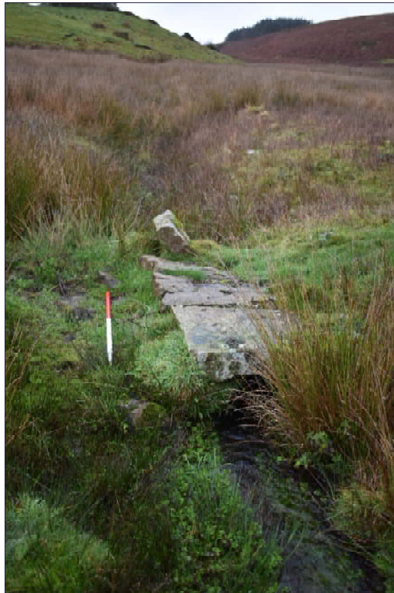
Plate 10: Stone bridge over the Dike Beck [1], looking west
