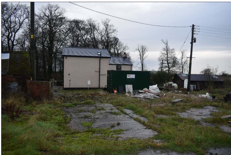
Plate 7: Foundations of modern agricultural structures, looking northwest
