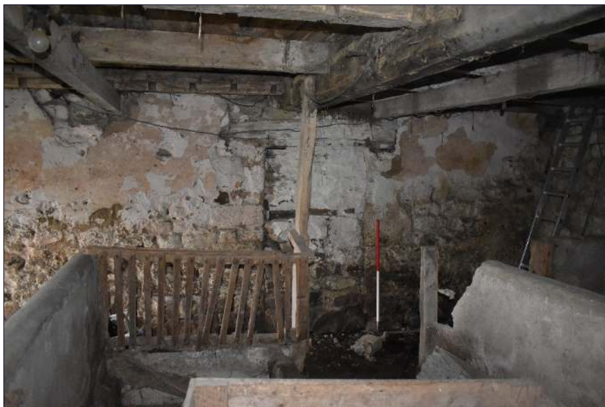
Plate 17: South wall of the northern room showing blocked internal doorway, looking south.
