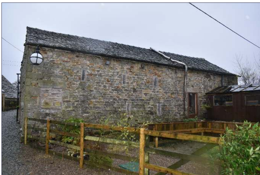
Plate 35: The Bothy (C) showing ventilation slits, looking southwest
