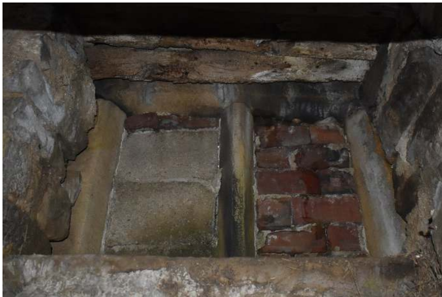
Plate 21: Blocked mullion window between floors in the west wall, looking west.
