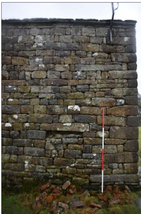
Plate 11: Blocked window in the west-facing elevation, looking northeast.
