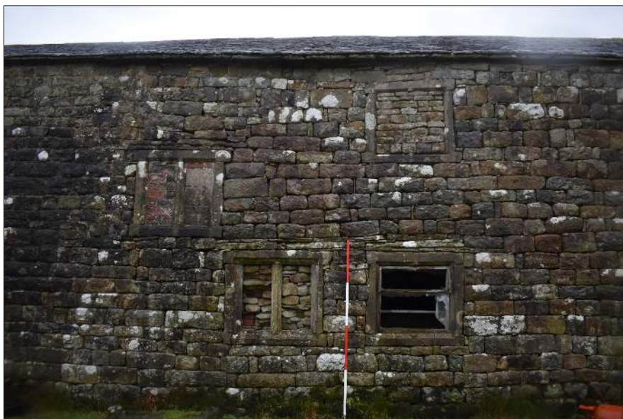
Plate 10: Mullion windows in the west-facing elevation of the survey building, looking northeast.
