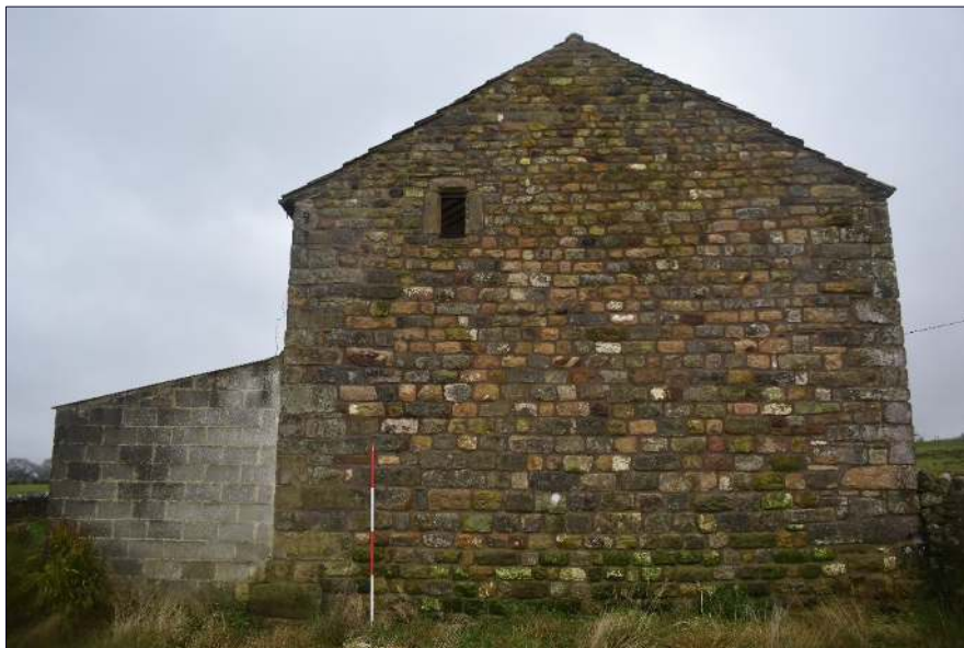
Plate 13: North-facing elevation with modern lean-to, looking southeast.
