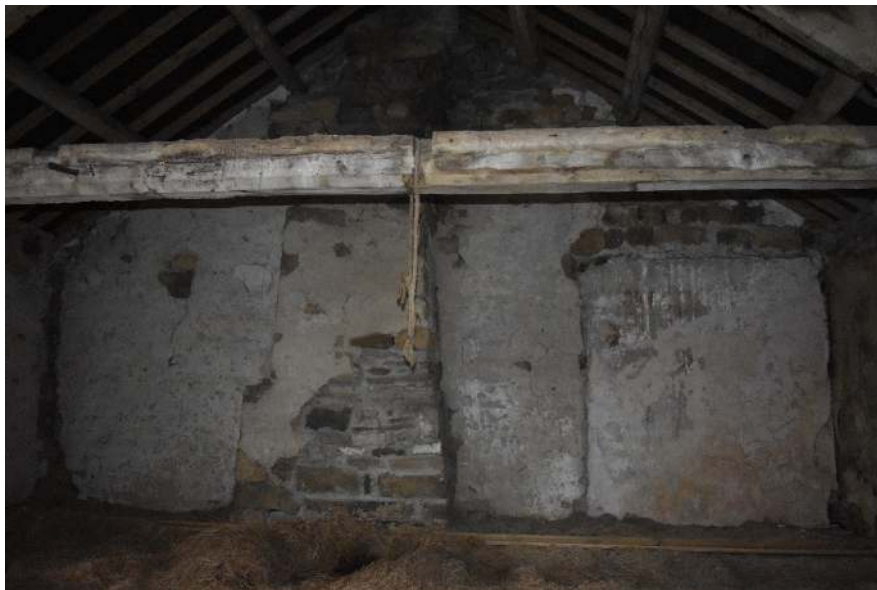
Plate 29: Central room on the first floor showing chimney breast, looking south.
