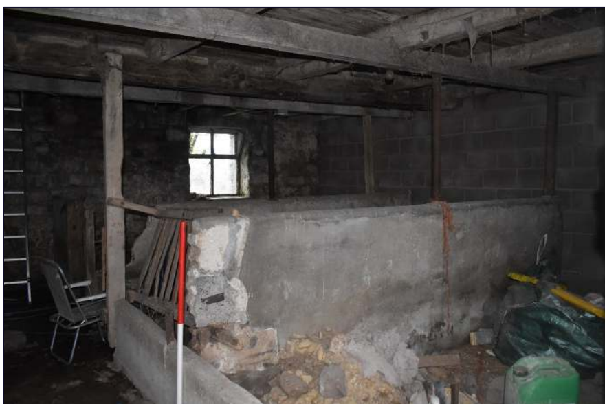
Plate 15: Interior of the northern room showing concrete partitions, looking northwest.
