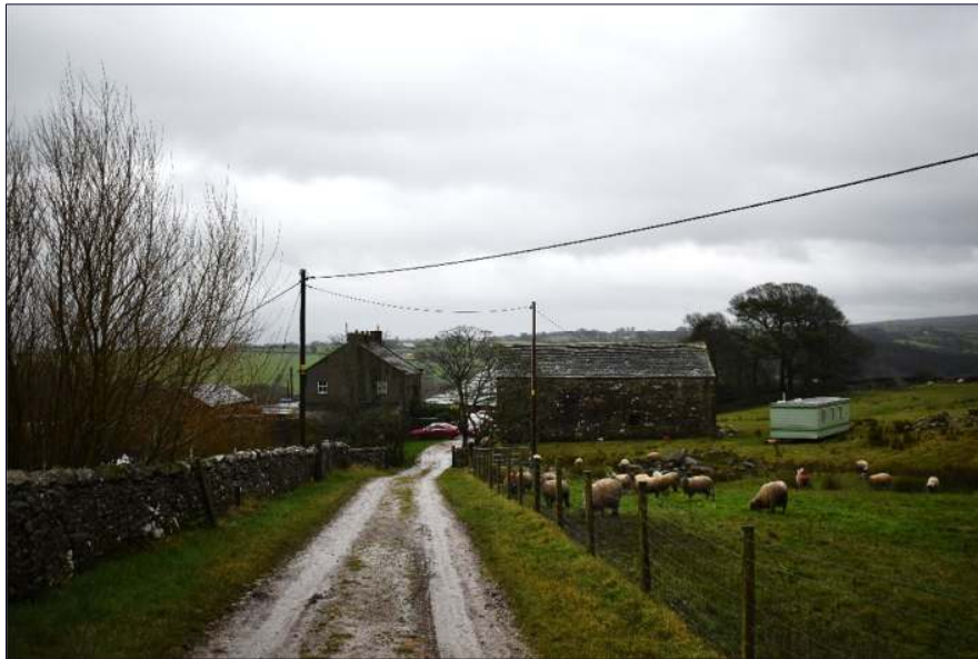
Plate 4: View of the survey building (right) at Lower House Farm from the west, looking east.
