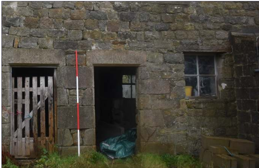
Plate 8: Ground floor window inserted into a blocked opening, looking west.
