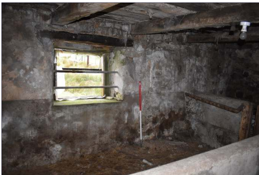
Plate 19: Former mullion windows in the west wall of the central room, looking northwest.
