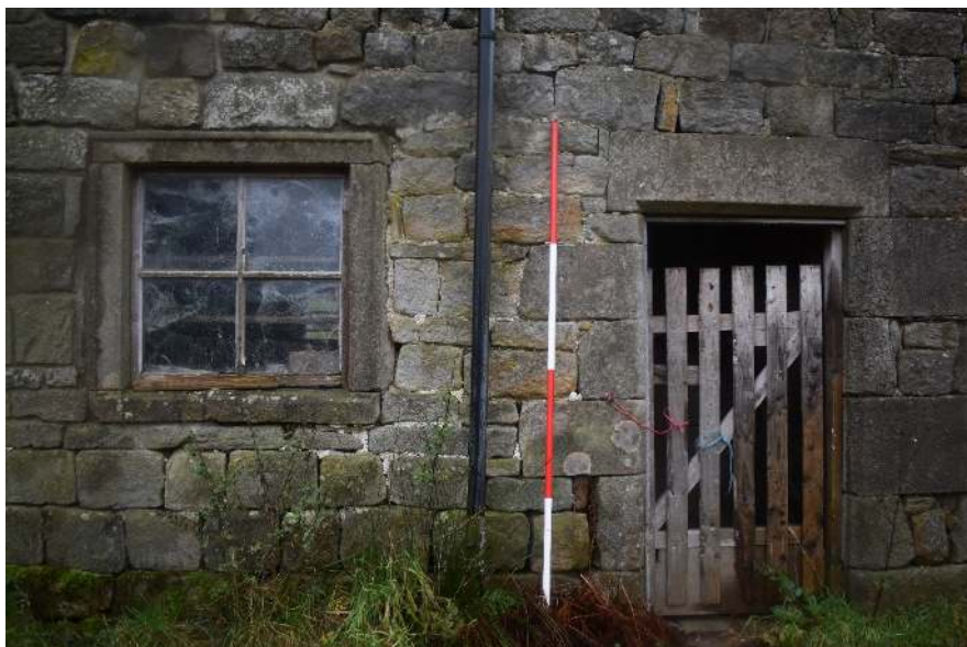
Plate 7: Detail of adapted former mullion window and stone door frame, looking west.
