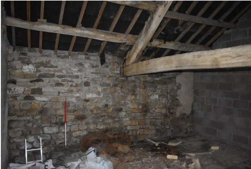
Plate 24: Northern room on the first floor, looking northwest.
