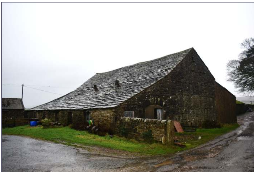
Plate 32: Stone barn (B) showing outshut to west side, looking east.
