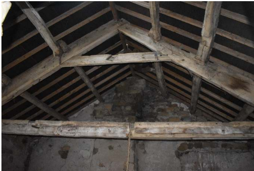
Plate 31: Roof timbers in the central room, looking south.
