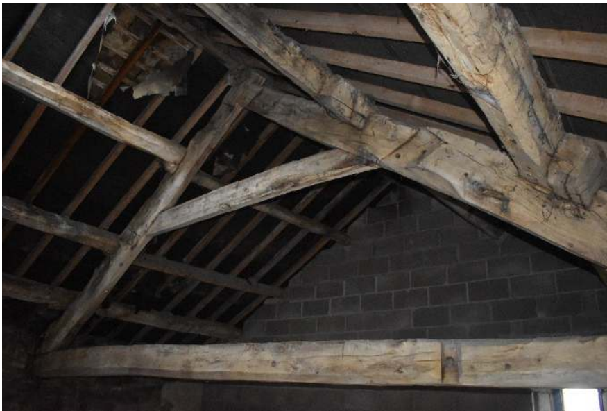
Plate 25: Roof timbers in the northern room, looking northwest.
