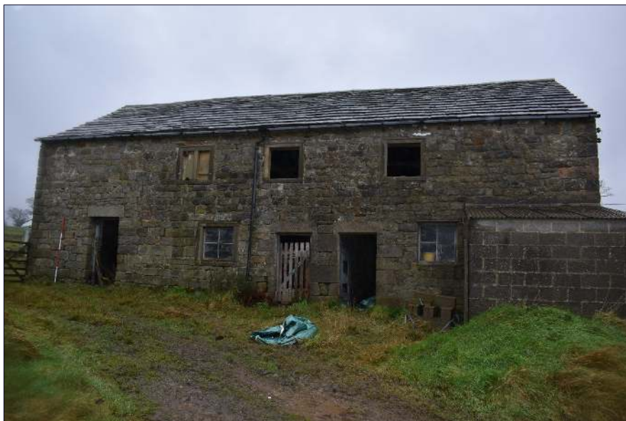
Plate 5: East-facing elevation of the survey building, looking southwest.
