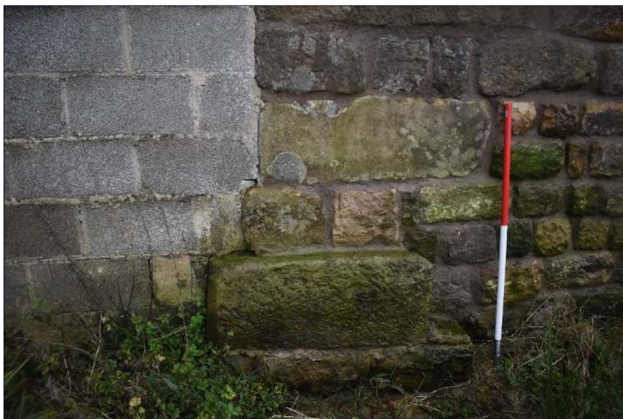
Plate 14: Foundation stones underlying the modern lean-to, looking south.
