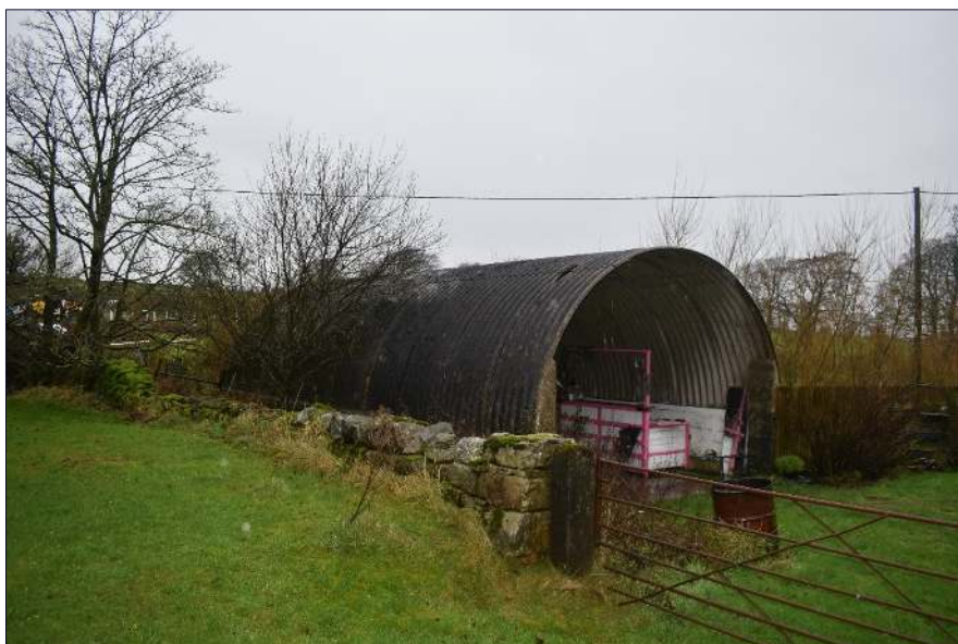
Plate 37: Corrugated iron shelter (E), looking west.
