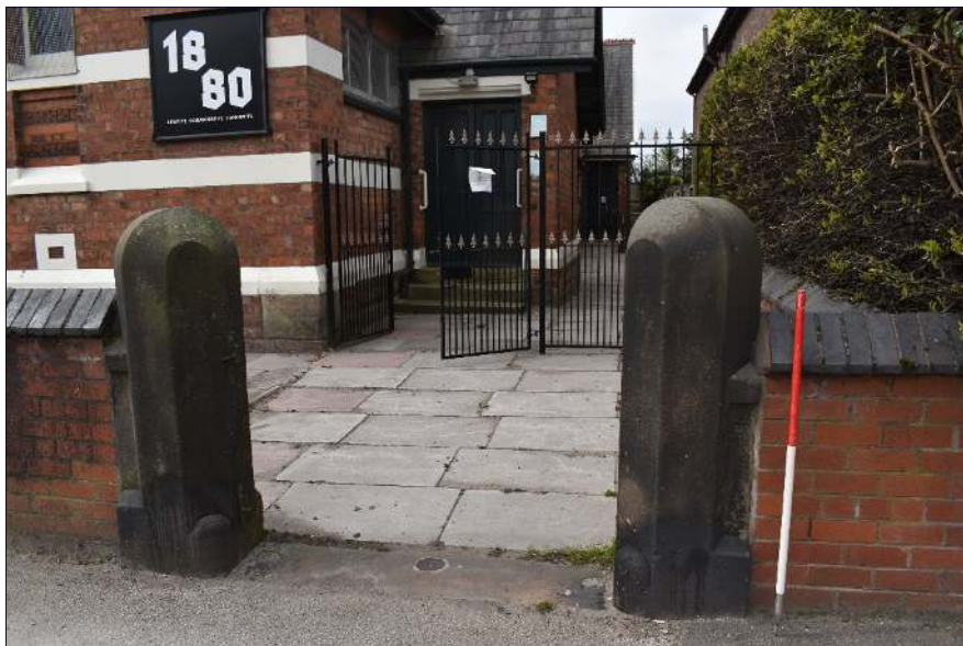
Plate 3: Northern site entrance showing gate piers with church entrance beyond, looking west (1 x 1m scale)
