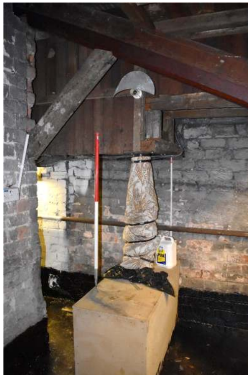
Plate 44: Basement room showing the base of the organ, looking north (1 x 1m scale)
