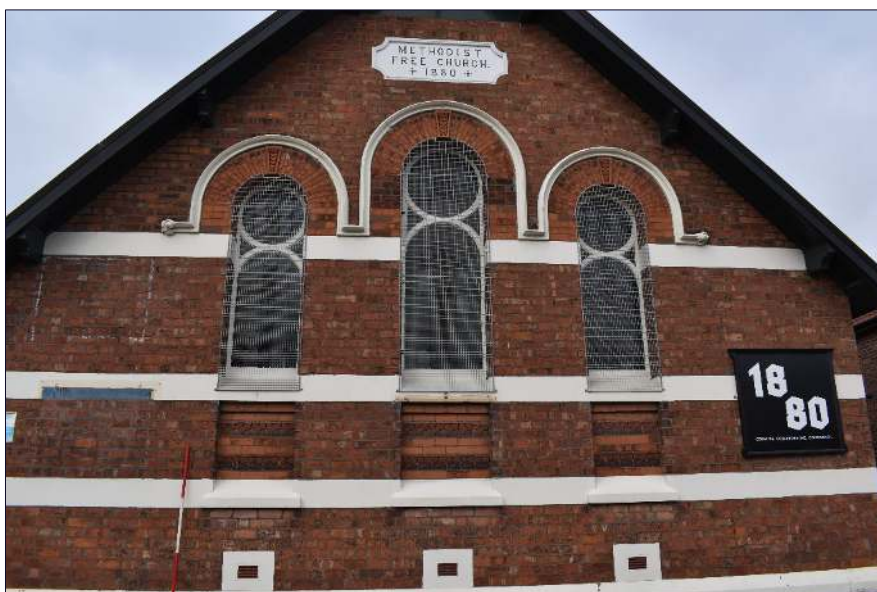
Plate 7: Window detail in the east elevation, looking west (1 x 2m scale)
