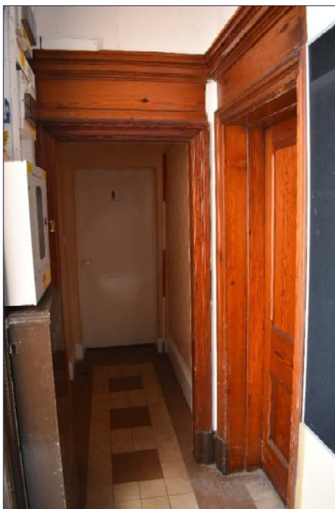
Plate 42: Corridor to modern toilet block, looking south (1 x 2m scale)
