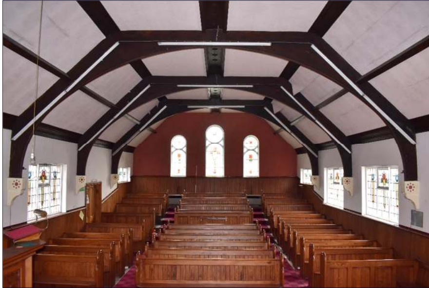
Plate 19: Church interior, looking east (1 x 2m scale)
