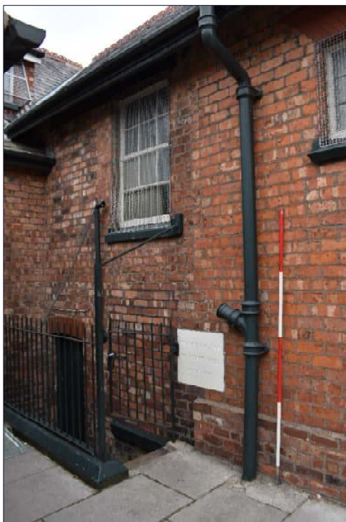
Plate 13: Construction break in the south elevation, looking northwest (1 x 2m scale)
