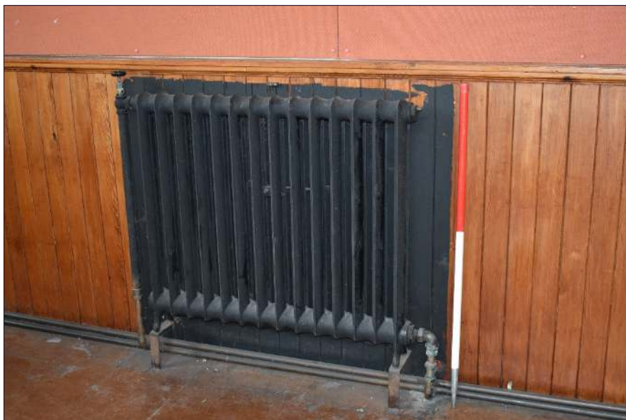
Plate 36: Detail of paneled wall and cast iron radiator, looking east (1 x 1m scale)
