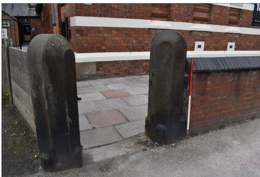
Plate 4: Southern site entrance showing matching gate piers with later brick wall, looking west (1 x 1m scale)
