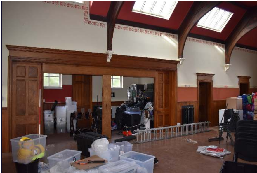
Plate 37: Room to the west of the main hall, looking northwest (1 x 2m scale)
