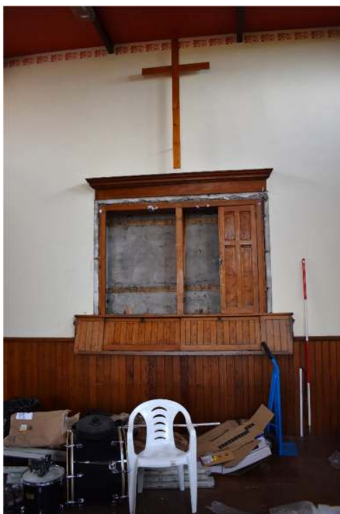
Plate 35: Detail of , looking south (1 x 2m scale)
