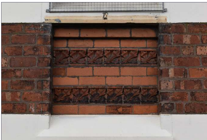
Plate 6: Detail of decorative brick panel in the east gable, looking west
