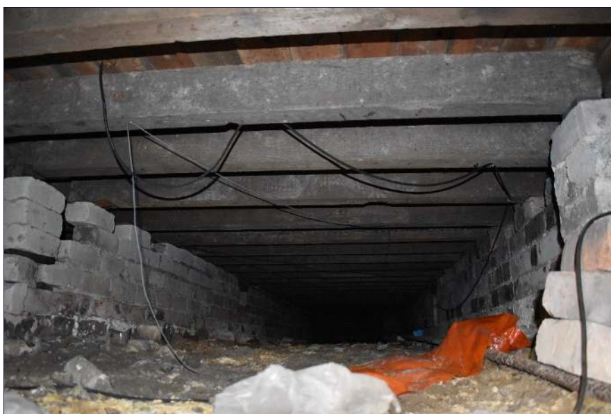
Plate 46: Timber floor in the nave, looking east
