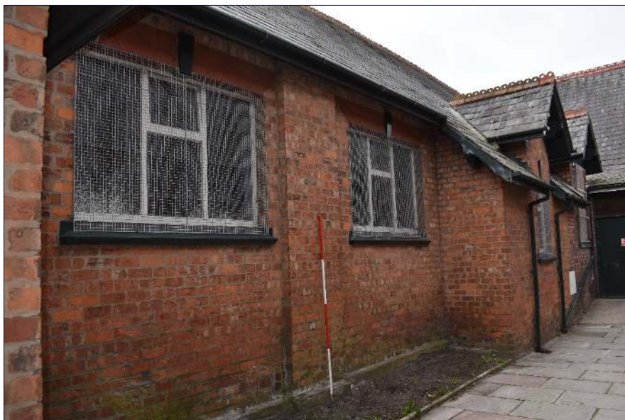
Plate 10: Windows in the north elevation, looking west (1 x 2m scale)
