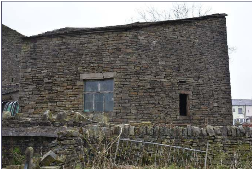
Plate 6: Western elevation of the stable (Building A), looking east
