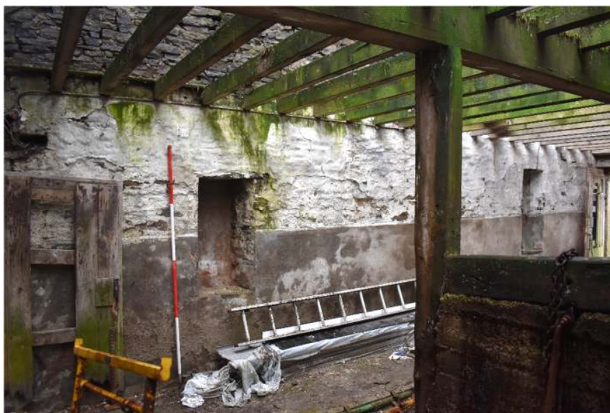
Plate 22: West wall of the barn (Building B) showing blocked windows, looking northwest
