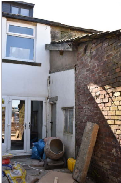
Plate 37: North elevation of the extension (Building D), looking south (taken 24th April 2020)
