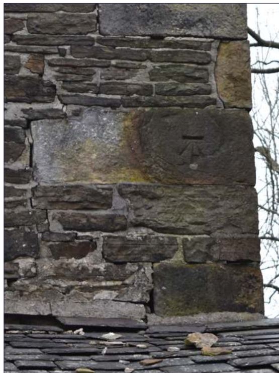
Plate 28: Benchmark on the west end of the barn (Building B), looking west
