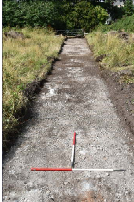
Plate 2: Trench A, looking northwest (2 x 1m scales)
