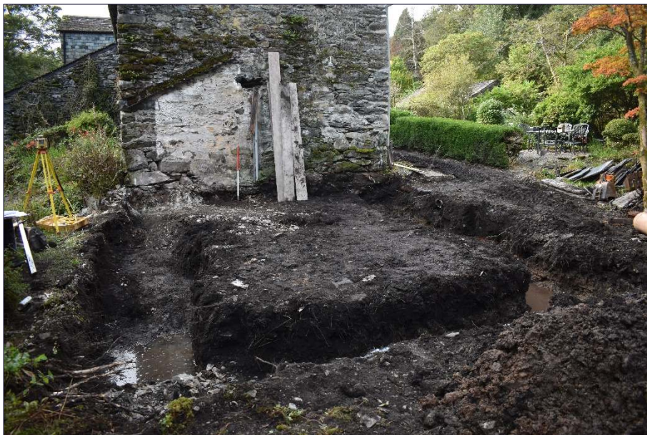
Plate 1: Area excavated for the new extension, looking west
