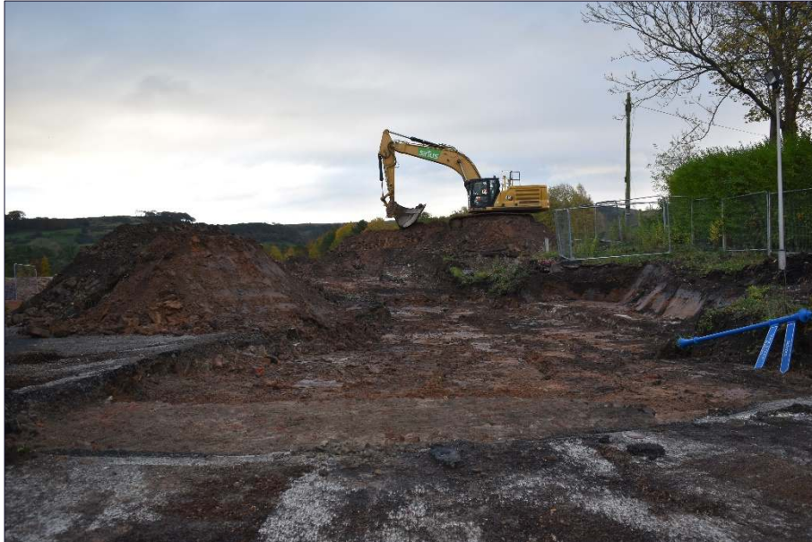
Plate 3: Excavated area south of the main building, looking east
