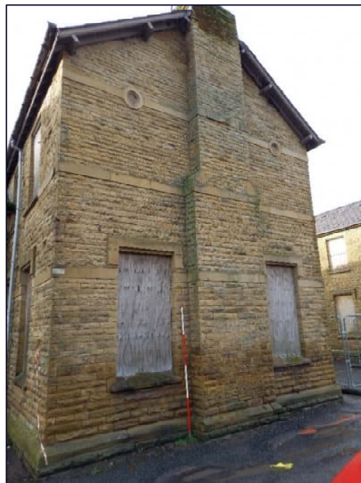
Plate 22: North-east elevation of Cottage 4, Block B showing the round ventilation grilles
