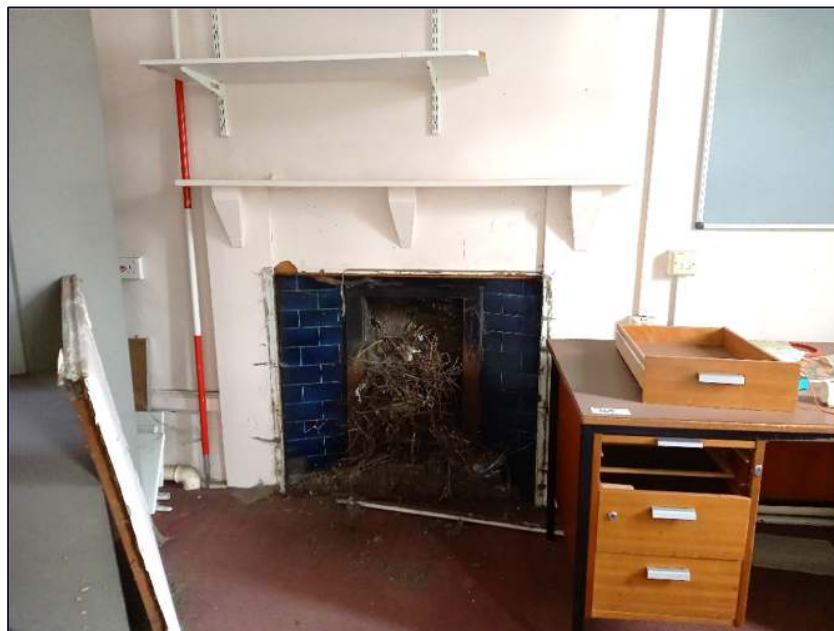
Plate 29: Surviving fireplace, first floor of Block C
