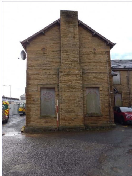
Plate 3: North-east elevation of Cottage 1, Block A, showing the projecting chimney flue
