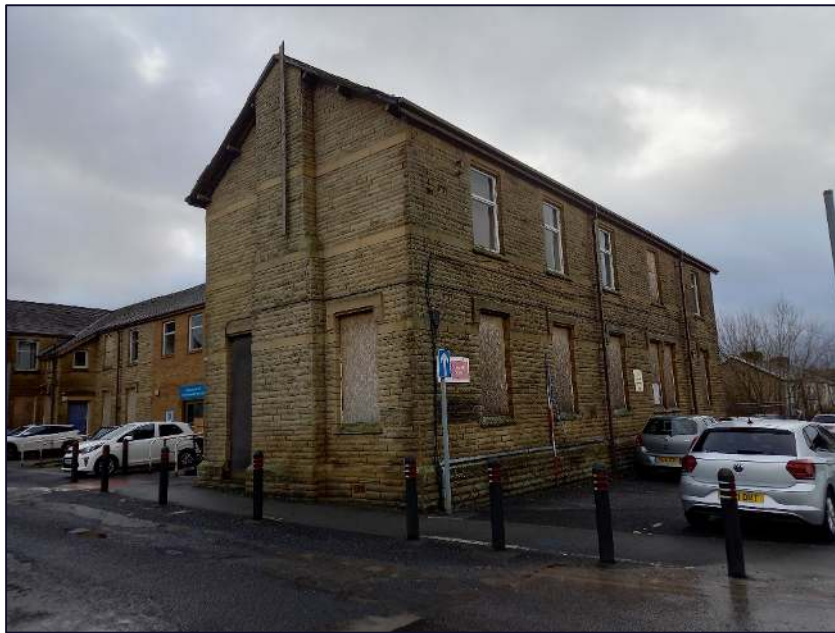
Plate 23: North-east and north-west elevations of Cottage 6, Block C, showing lack of round ventilation grilles
