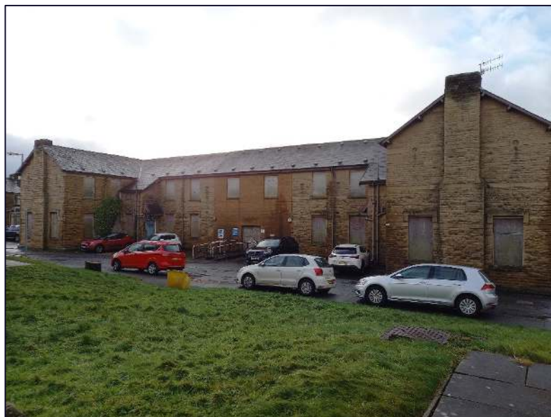
Plate 4: North-east facing elevations of Block A showing the projection for a doorway to Cottage 1
