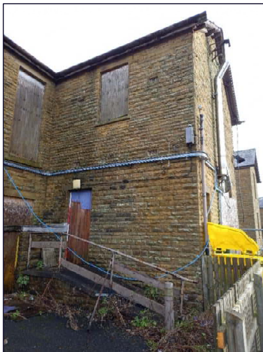
Plate 12: Inserted doorway, north-west facing elevation of Cottage 3, Block B
