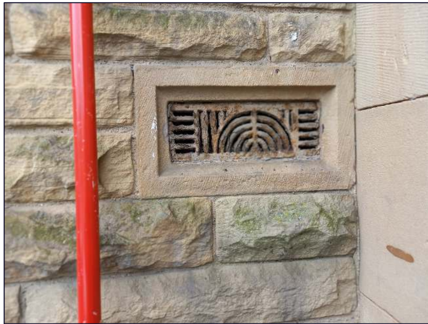
Plate 21: Decorative ventilation grille, Cottage 4, Block B
