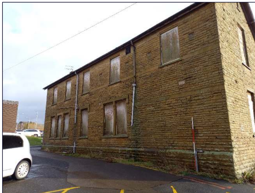
Plate 14: North-west elevation of Cottage 2, Block A showing the fenestration and plinth
