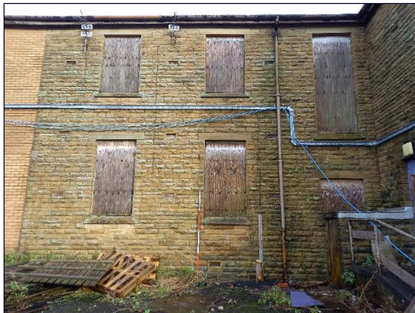
Plate 18: South-west elevation of Cottage 3, Block B showing plain lintels and sloping sills of the windows
