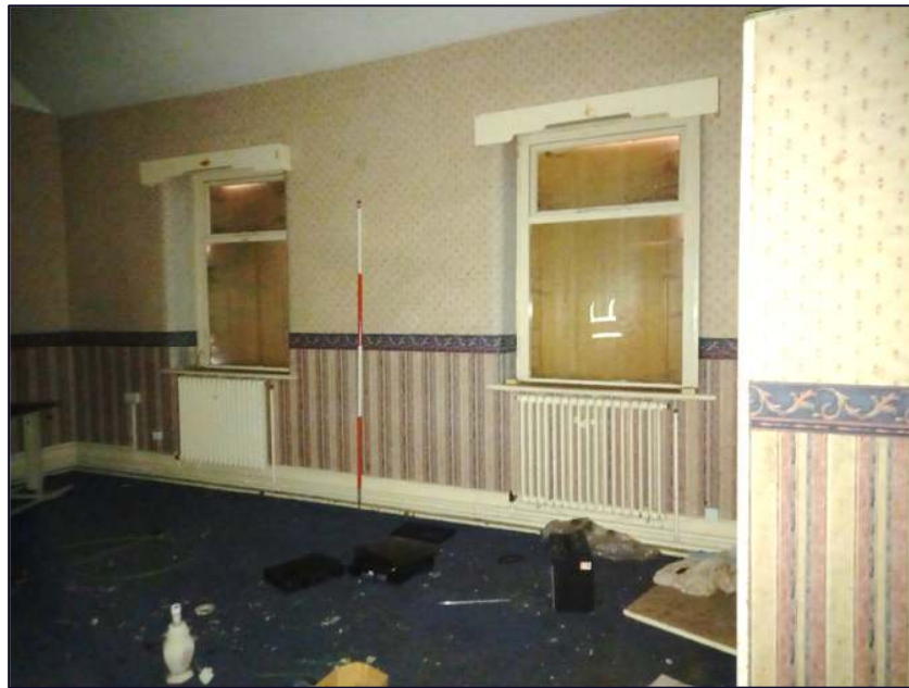
Plate 30: Examples of historic radiators, first floor of Block A (Scale = 2m)
