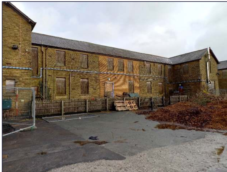
Plate 17: South-west facing elevations of Block B showing the fenestration with plain sills and lintels
