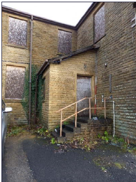
Plate 10: South-west elevation of Block C showing an apparent later doorway to Cottage 5 (Scale = 2m)
