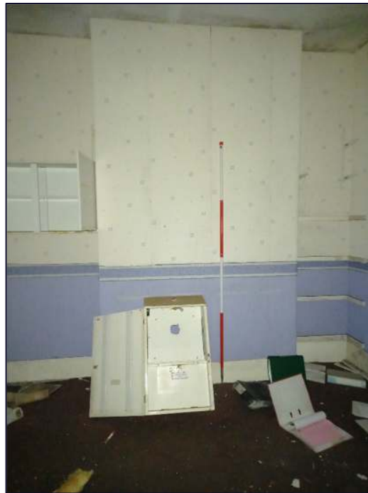
Plate 28: Projecting chimney breast, Block A (Scale = 2m)
