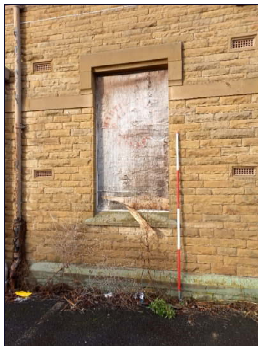
Plate 16: Detail of window in south-east elevation of Cottage 1 showing decorative lintel (Scale = 2m)
