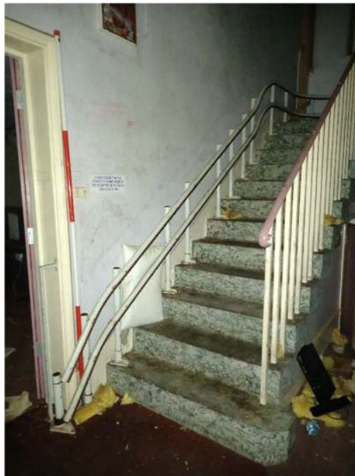
Plate 31: Detail of staircase, Block A (Scale = 2m)
