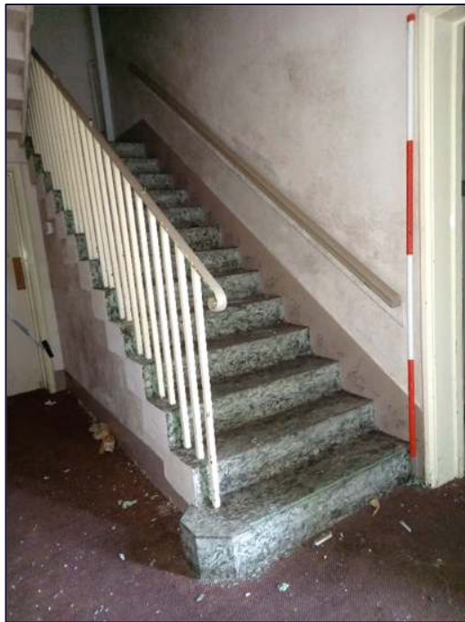
Plate 32: Detail of staircase, Block C
