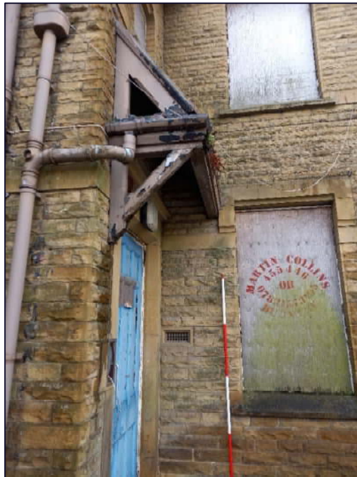
Plate 7: Projecting canopy above the main entrance to Cottage 1, Block A, north-east elevation
