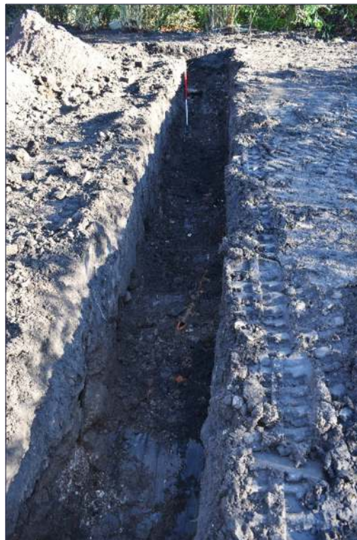
Plate 5: Southern foundation trench showing made ground ( 102 ), looking west (1m scale)
