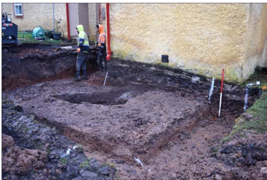
Plate 3: Excavated area showing the foundations of the existing outbuilding, looking south-west (1m scale)
