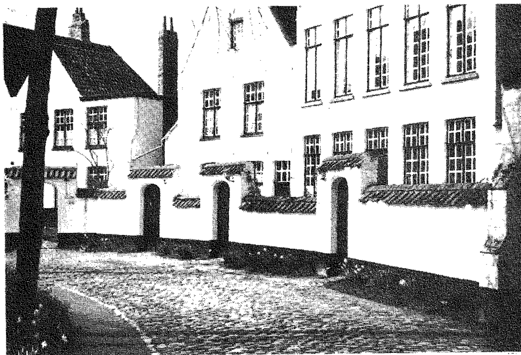
Fig. 6. Ceramic flat tiles and ridge tiles capping walls in modern Brugge. Account rolls suggest that similarly-looking wall tops must have been commonplace in central and southern England during the Middle Ages (photo: S. Moorhouse)
