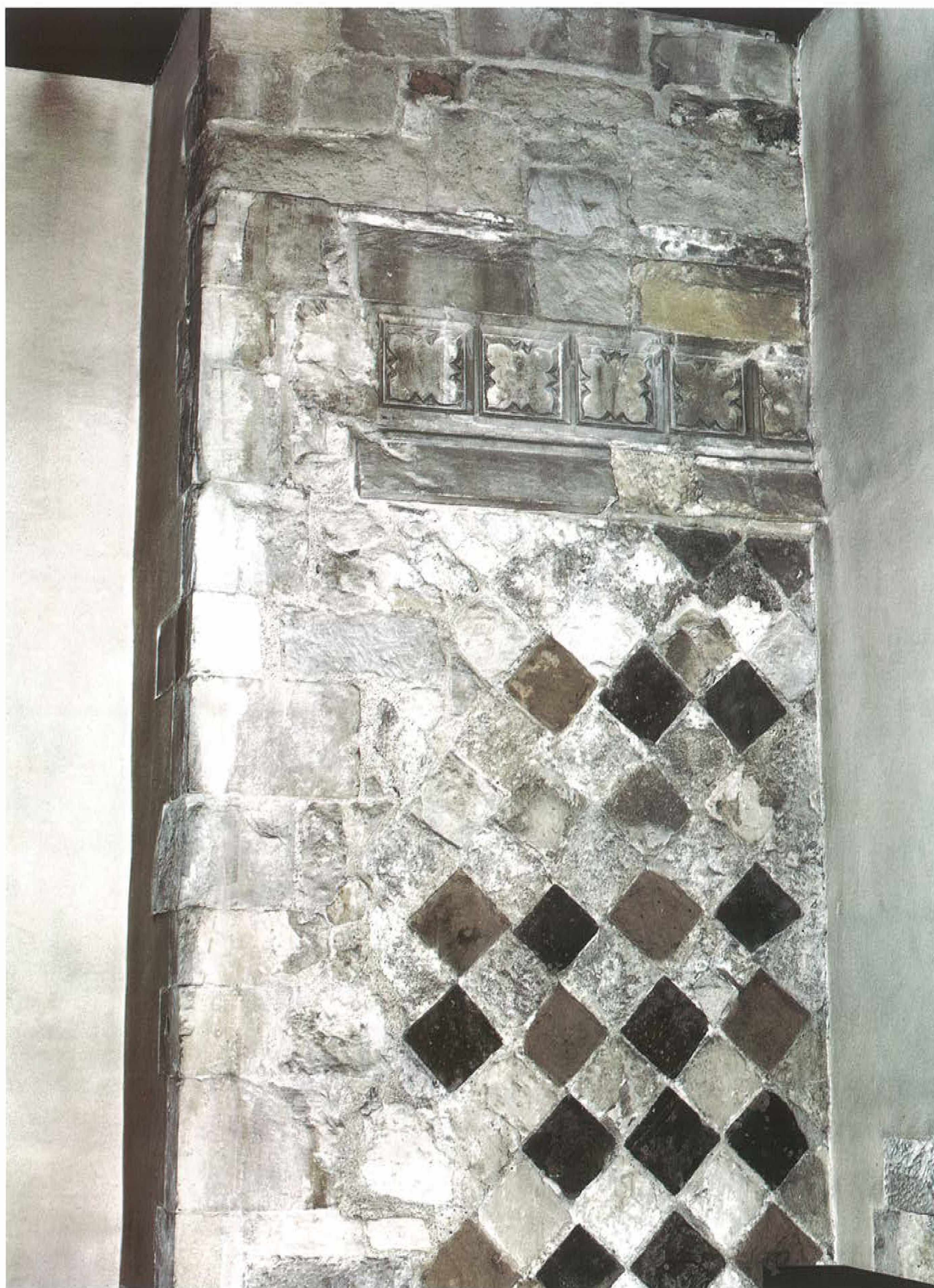
Glazed eleventh-century wall tiles from London in Cheyneygates, Westminster Abbey, showing decorative arrangement of stone blocks and glazed wall tiles. Photograph by courtesy of the Dean and Chapter of Westminster Abbey (see pp. 19–24).
