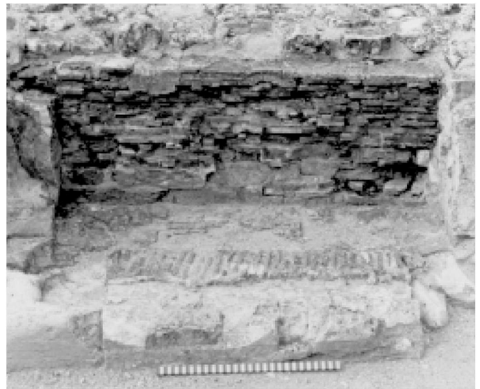
Fig. 3 Farnham Castle – great bricks and tiles in the West Turret hearth. Scale 50cm.
