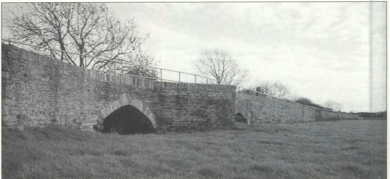
Fig 60 Harrold bridge: the causeway from the north-west
