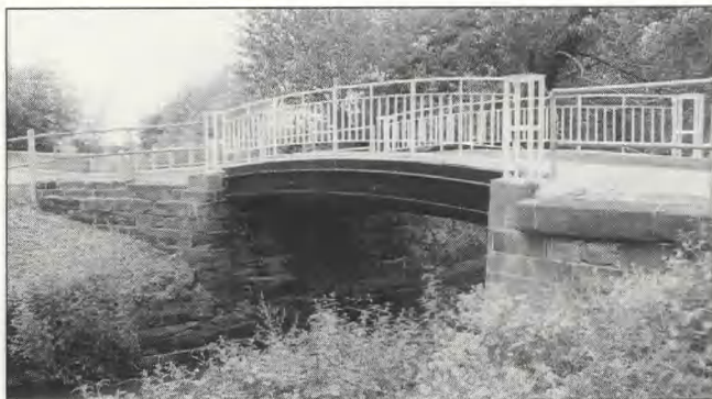
Fig 114 Blunham navigation bridge: from the south-east
