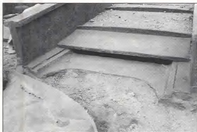
Fig 120 Lock bridge, Broom: close-up of ironwork over east abutment
