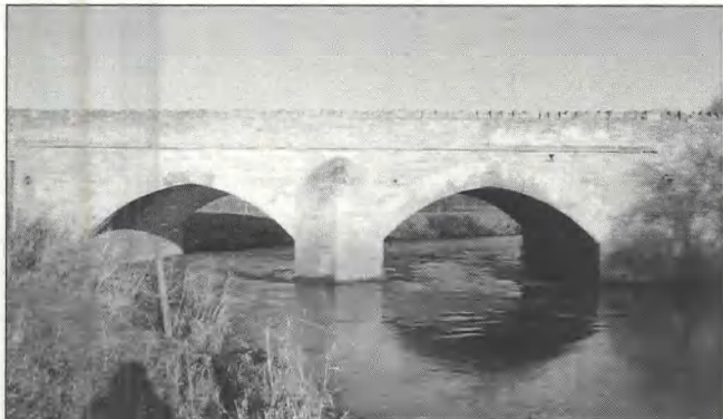
Fig 77 Turvey bridge: south face of arches 1 and 2
