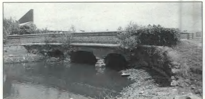
Fig 104 Chicksands bridge: west face
