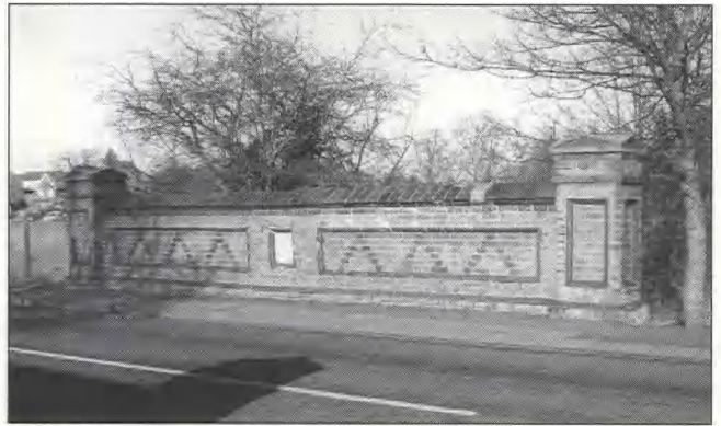
Fig 96 Tannery bridge, Potton: inside face of north parapet
