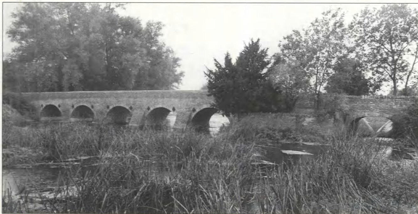
Fig 48 Oakley bridge: river bridge and mill arch from the north-east
