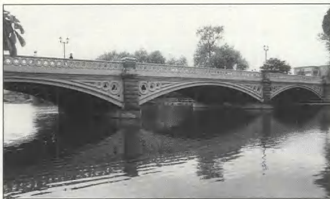
Fig 31 Cauldwell bridge, Prebend Street, Bedford, before demolition in 1992
