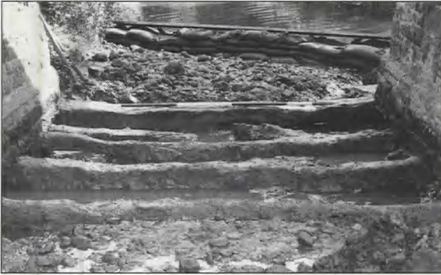
Fig 92 Sutton bridge: timber foundation under west arch, during excavation
