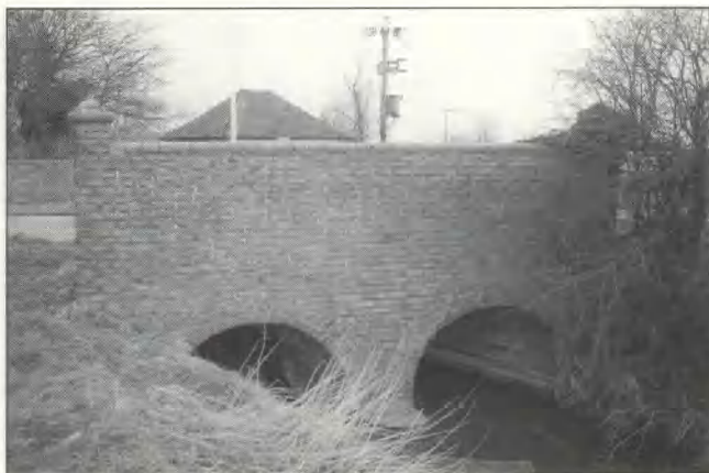
Fig 109 Eaton Bray bridge: south-east face
