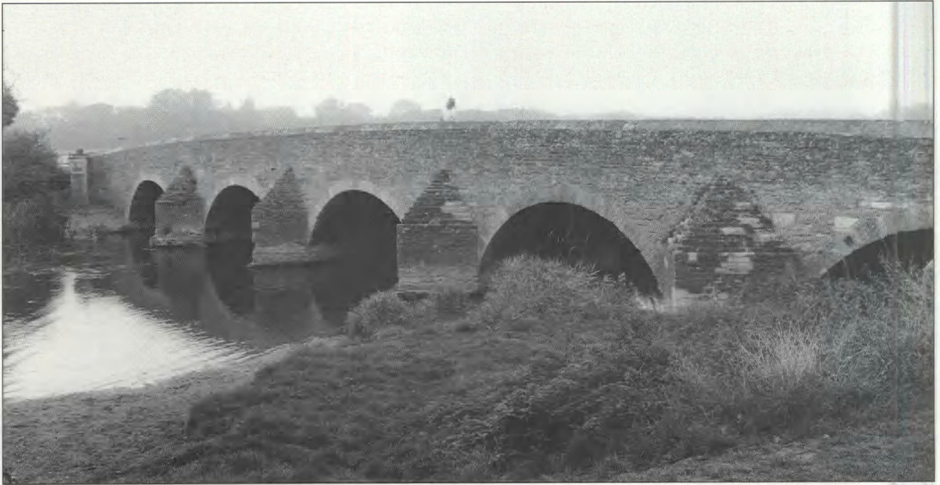
Fig 57 Felmersham bridge: from the south-west (Beds Photographic Services)
