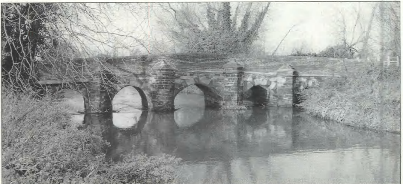
Fig 80 Blunham river bridge: from the south
