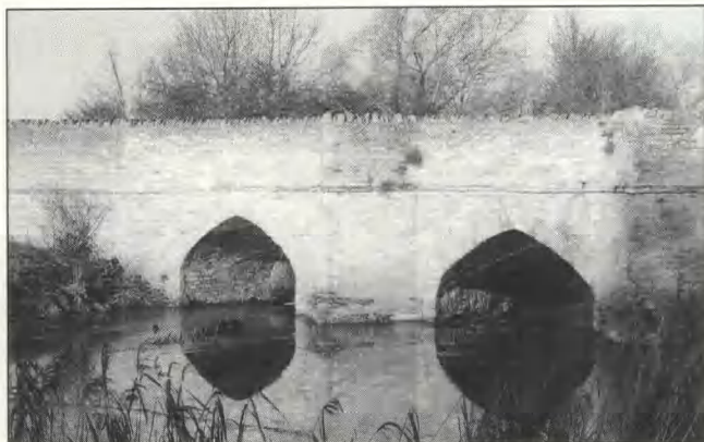
Fig 76 Turvey bridge: south face of arches 5 and 6
