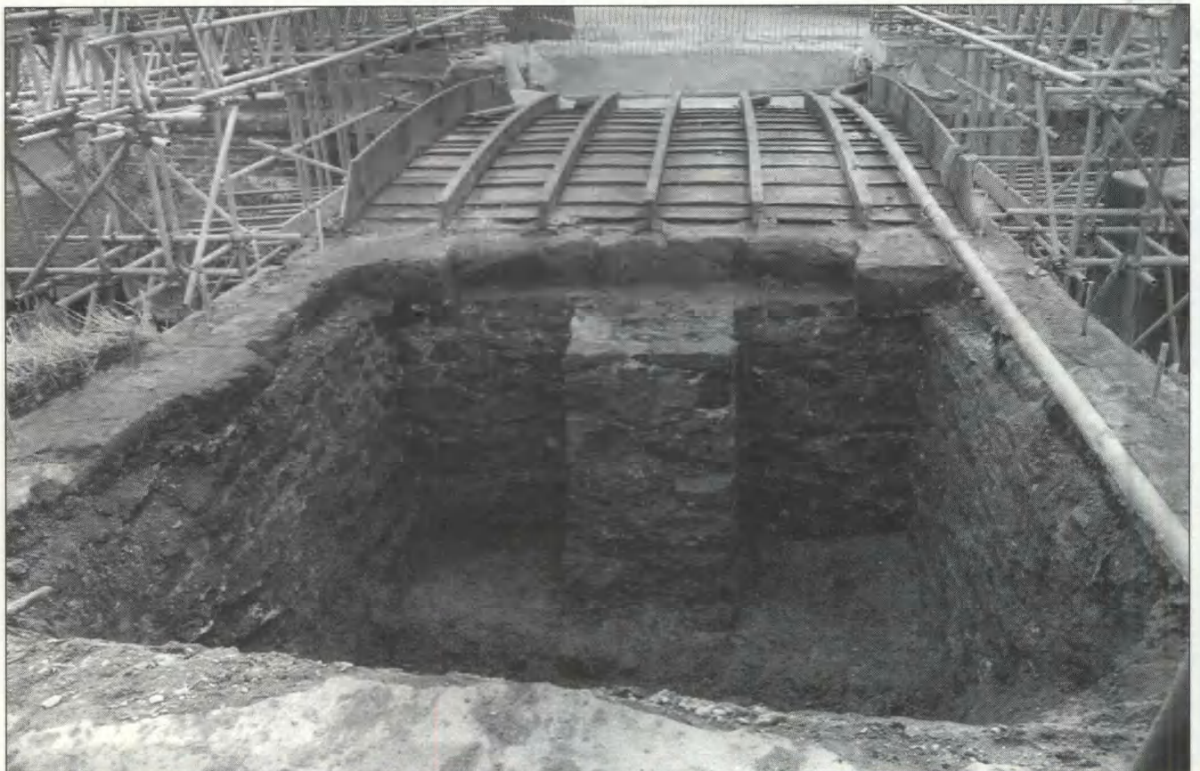
Fig 119 Lock bridge, Broom: excavated abutment and ironwork, from the west
