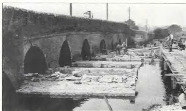
Fig 78 Turvey bridge: north face during widening works, 1930
