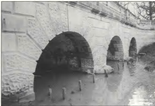
Fig 127 Basin bridge, Woburn Park: north-west face, overlooking Basin Pond
