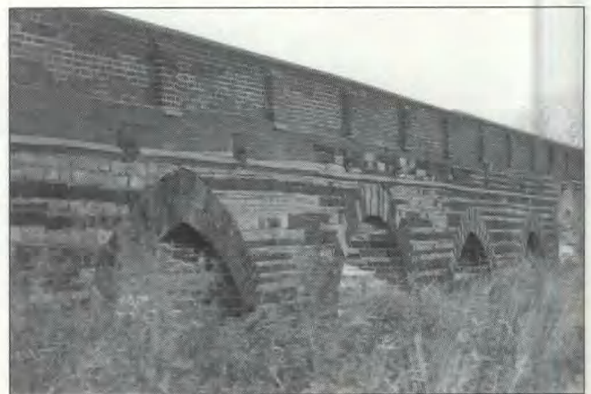
Fig 22 Barford bridge: east face of flood arches (arch 4 in foreground)
