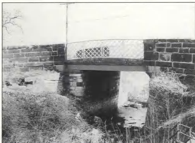
Fig 122 Clifton navigation bridge: before demolition in 1968 (Co Engineer)
