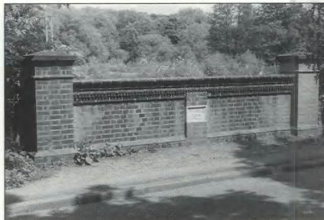
Fig 107 Flitwick bridge: north parapet
