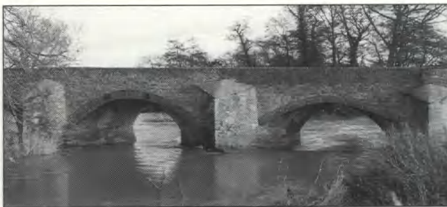
Fig 68 Harrold bridge: west face of arches 11 and 12, showing 1857 widening
