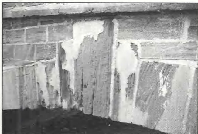
Fig 136 Girtford bridge: keystones
