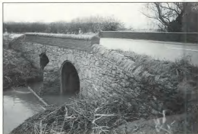
Fig 32 Kempston Hardwick bridge from the south-east
