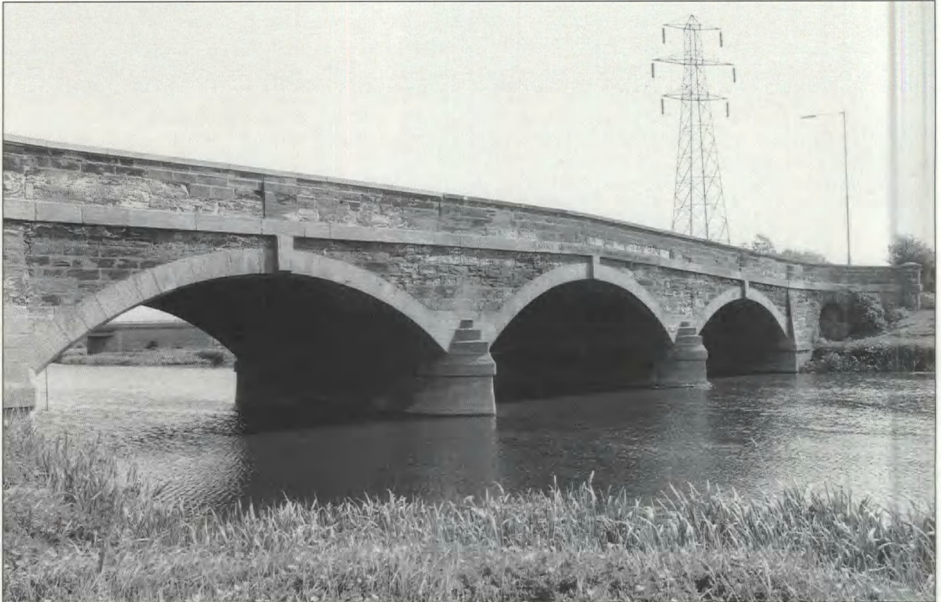
Fig 15 Tempsford bridge: south face of river bridge (Beds Photographic Services)
