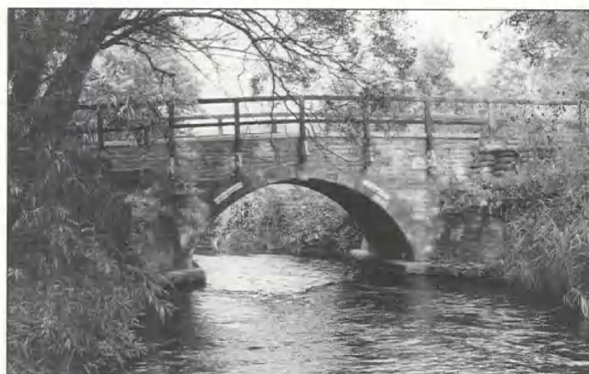
Fig 49 Oakley South bridge (Beds Photographic Services)
