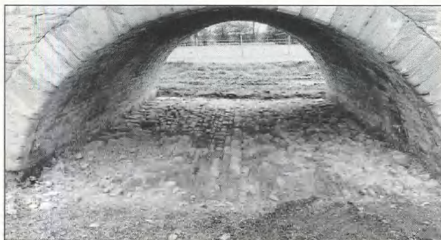
Fig 41 Bromham bridge: limestone invert
