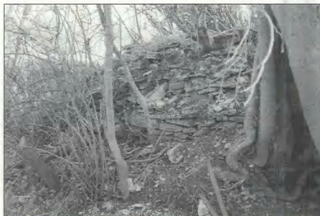
Fig 72 Turvey bridge: remains of foot causeway
