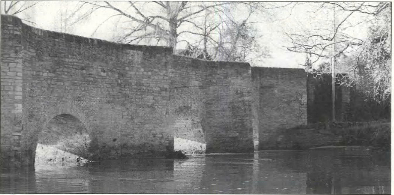
Fig 36 Bromham bridge: north face of river bridge
