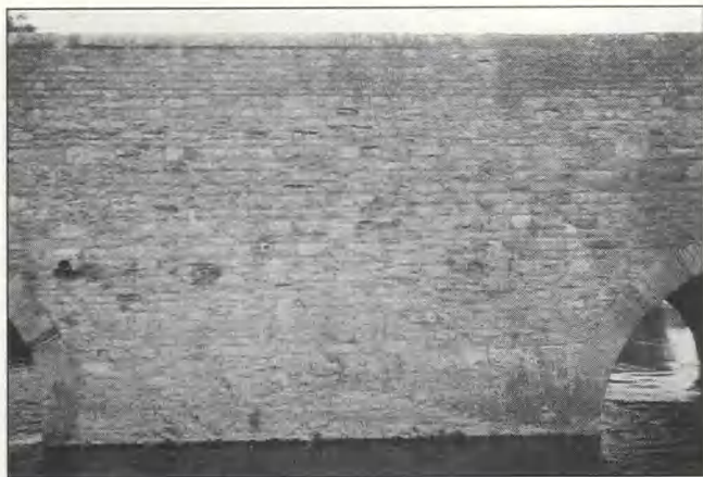
Fig 138 Bromham bridge: squared coursed limestone walling, 1902
