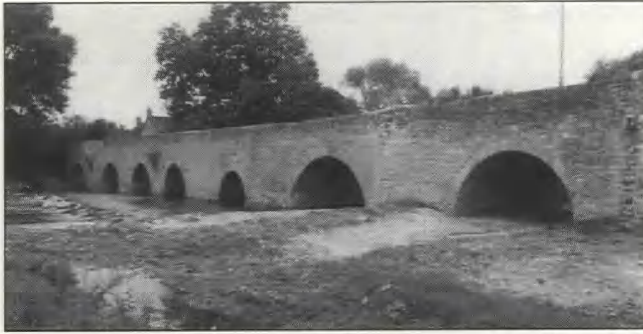
Fig 42 Bromham bridge: south face of river bridge, showing 1902 widening
