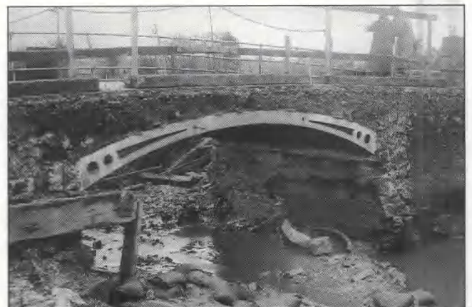
Fig 98 Langford bridge: under demolition, 1946 (Co Engineer)
