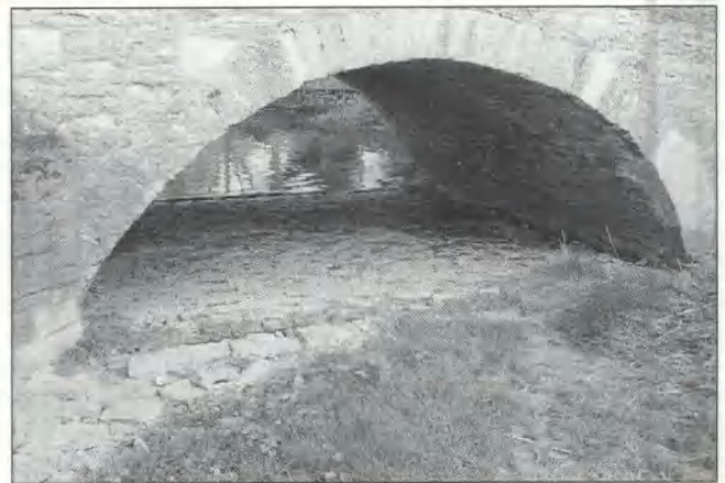
Fig 59 Felmersham bridge: invert, arch 1
