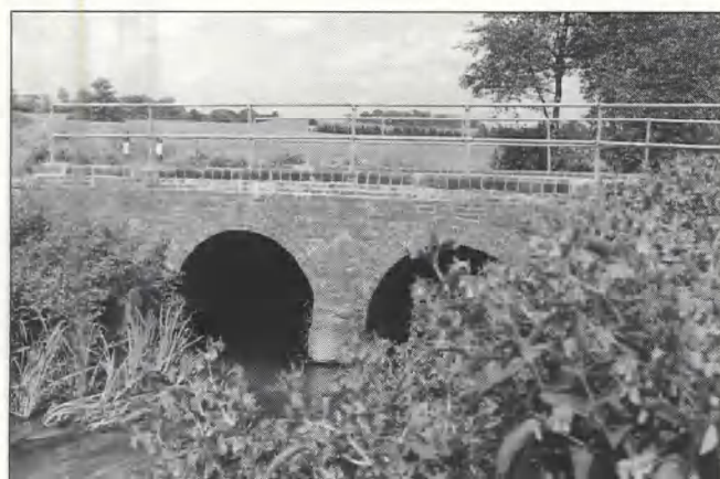
Fig 105 Beadlow bridges: arches over main channel, west face
