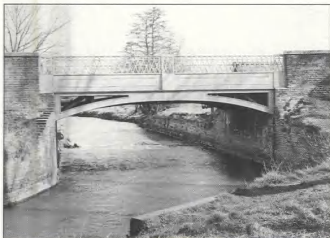
Fig 102 Clay bridge, Clifton: iron bridge before demolition, c.1968 (Co Engineer)
