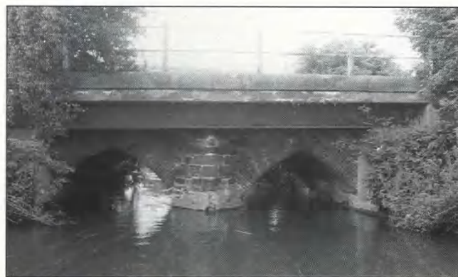
Fig 100 Arlesey bridge: south face
