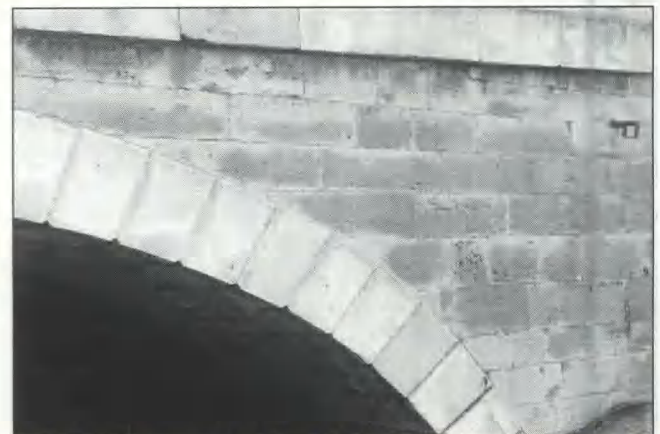
Fig 135 Bedford bridge: voussoirs and ashlar walling
