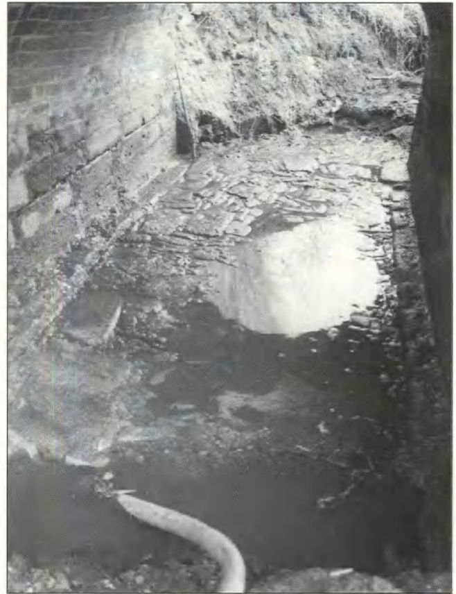
Fig 83 Blunham river bridge: invert, arch 5
