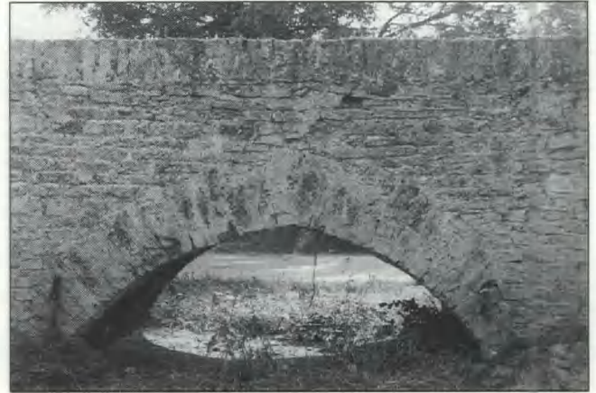
Fig 134 Harrold causeway: rubble limestone arch and walling
