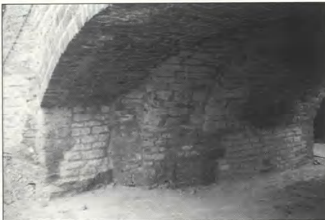
Fig 65 Harrold bridge: flood arch 6 from west, showing successive widenings
