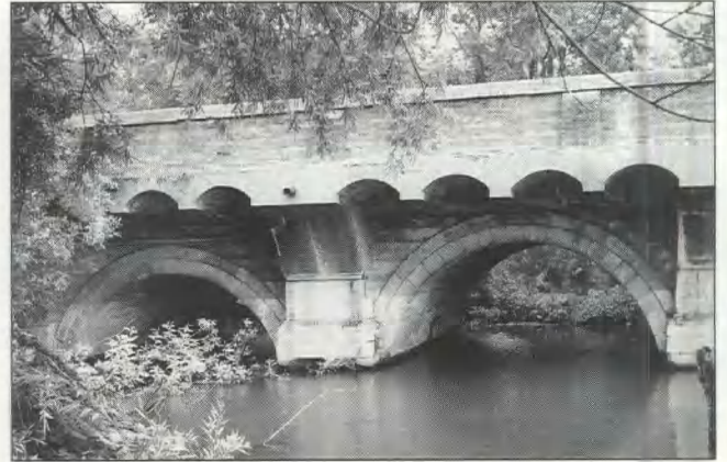
Fig 11 St Neots bridge: causeway arches 8 and 9, north face (Co Engineer)
