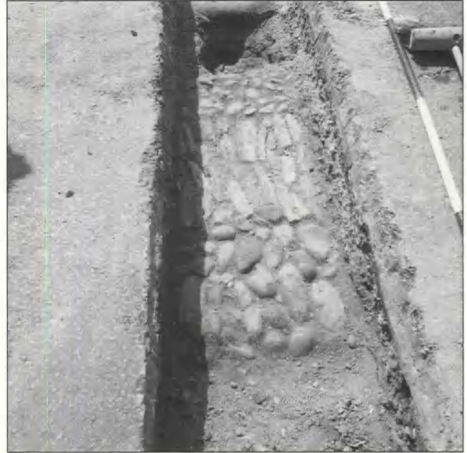
Fig 139 Barford bridge: 18th century cobble and limestone road surfacing
