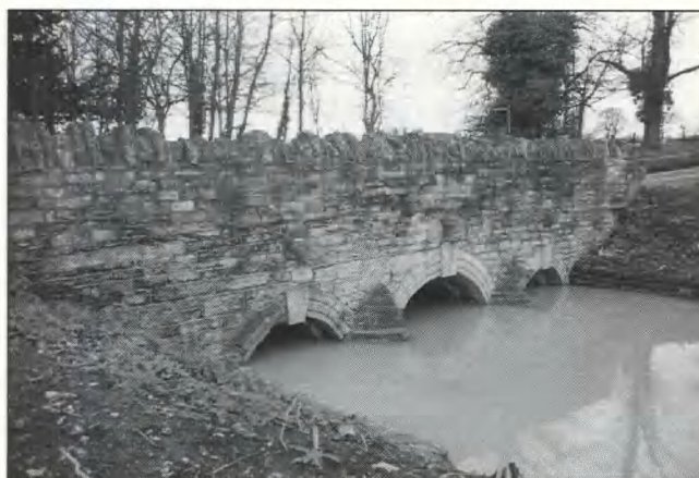
Fig 3 Hinwick bridge: south face
