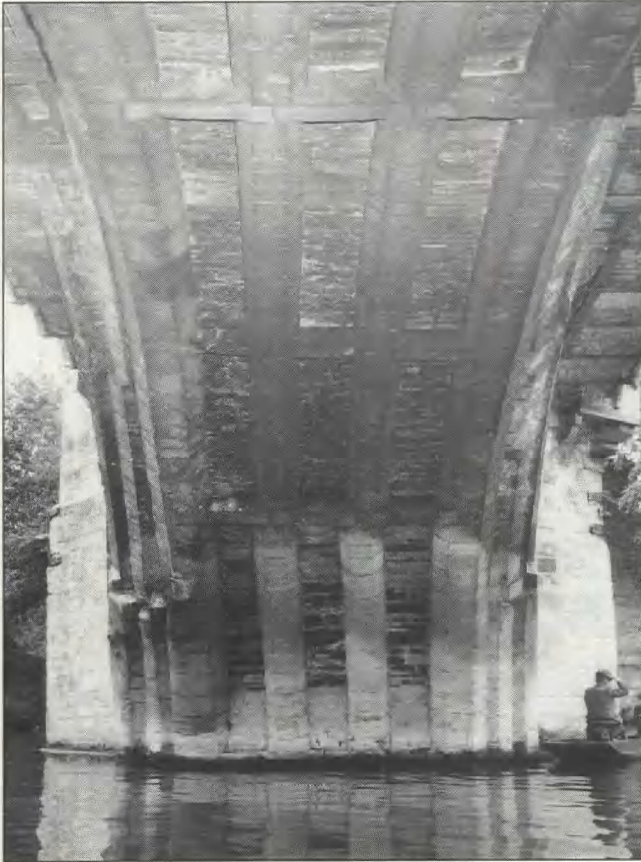
Fig 9 St Neots bridge: arch 2 ribbing (Co Engineer)
