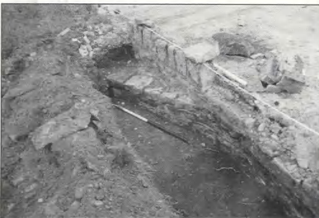
Fig 62 Harrold bridge: footing of early causeway approach ramp, between arches 5 and 6
