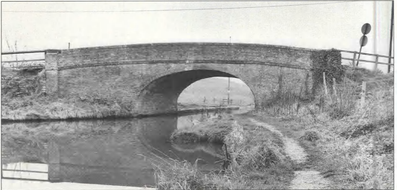
Fig 124 Sandhole canal bridge: south face (Beds Photographic Services)
