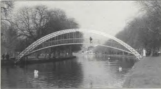
Fig 26 Suspension bridge, Bedford, from the east
