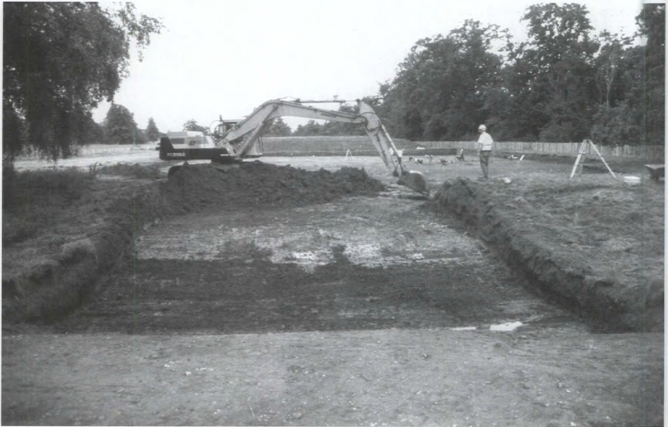
Plate 2. The southern moat being stripped of soil cover, looking south-east.
