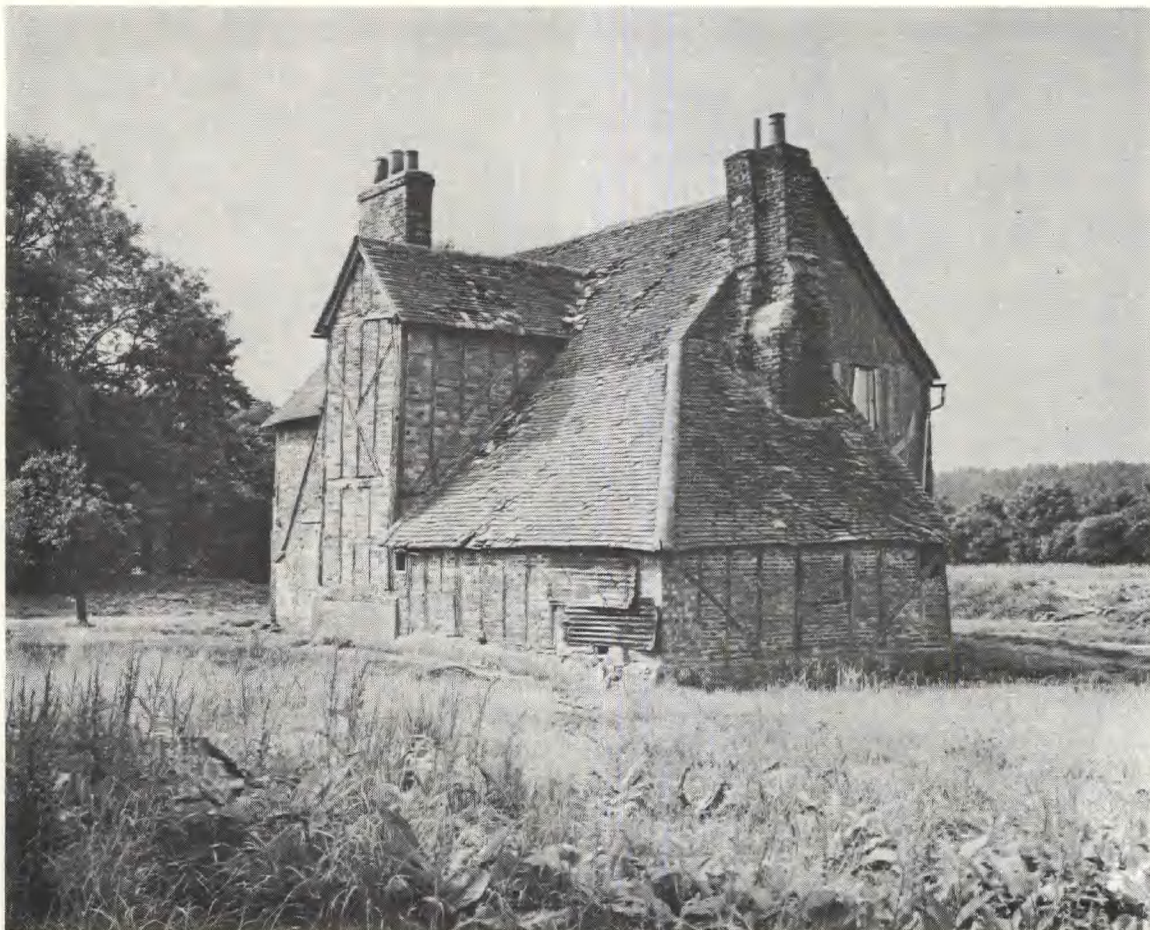
Plate 1 Calcutt Farm, Houghton Regis, in 1969, looking at the east and the north fronts. (Photograph: Bedfordshire County Council)
