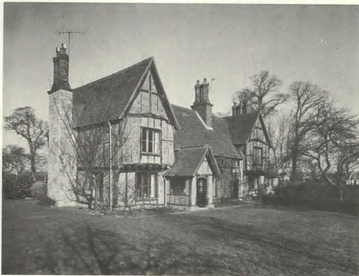
Pl 1 Exterior from south of Moat Farm, Marston Moretaine.
