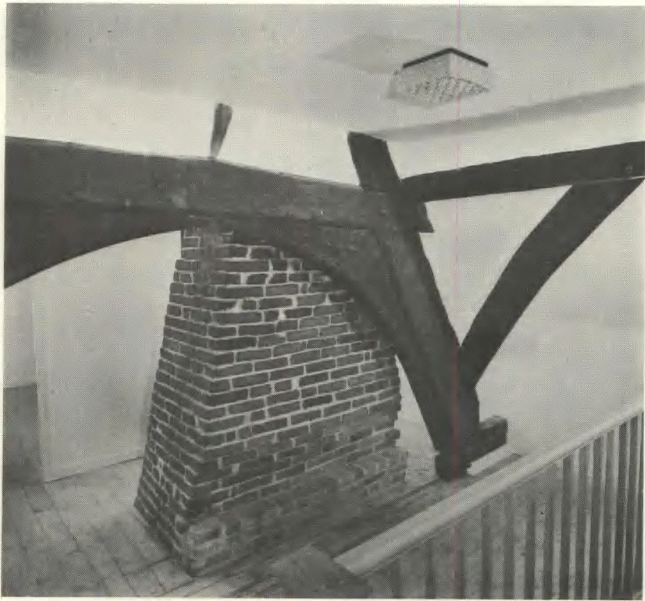
Pl 6 Detail of hall cruck, Husbourne Crawley. [Photograph: Bedfordshire County Council.]
