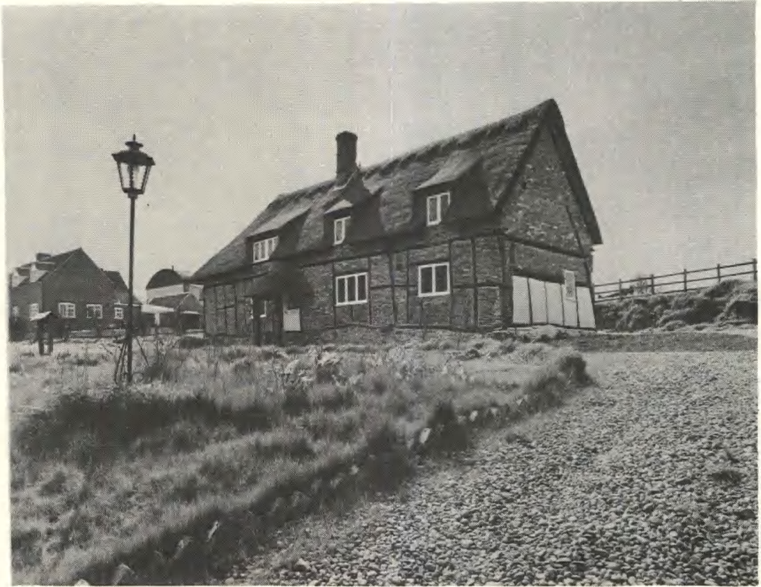
Pl 8 Exterior from north-east after conversion, Husbourne Crawley. [Photograph: Bedfordshire County Council]
