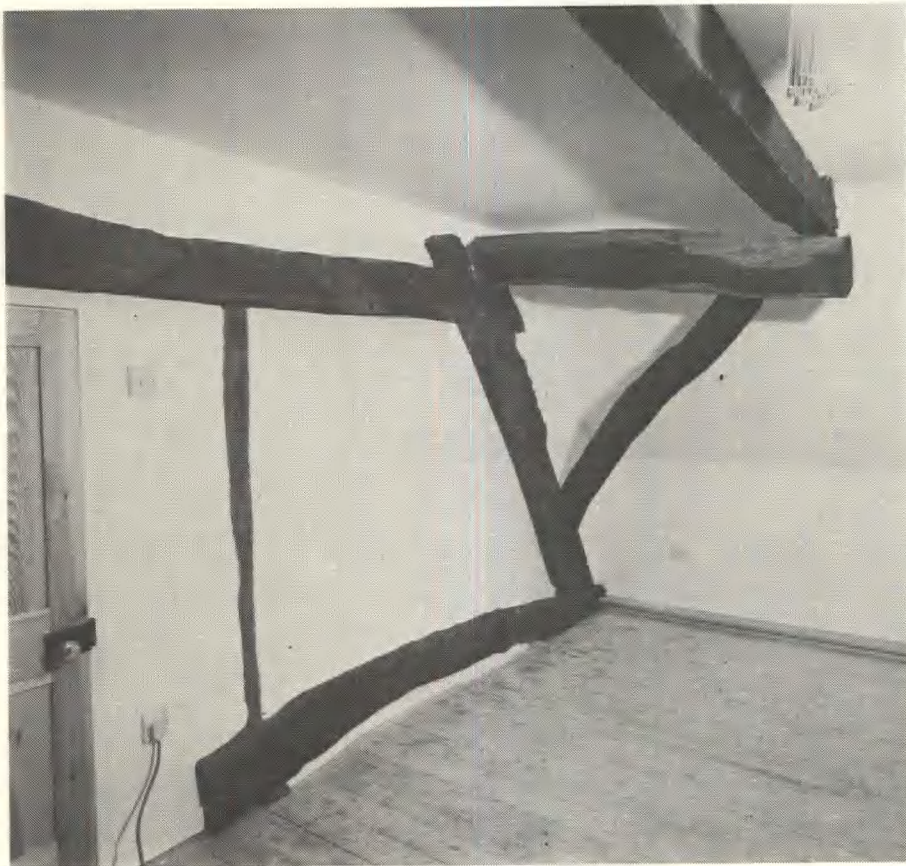
Pl 7 Detail of 'flying purlins', Husbourne Crawley. [Photograph: Bedfordshire County Council.]
