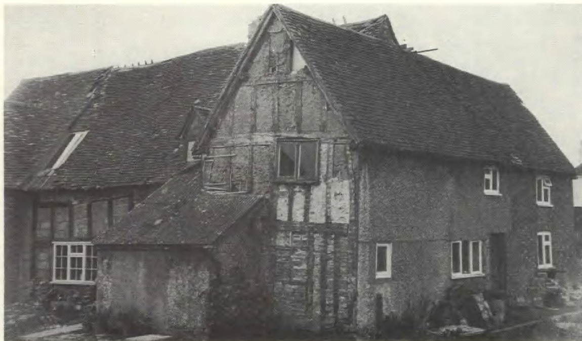
Plate 1 Lower Roxhill Farm, Marston Moretaine: from east.
