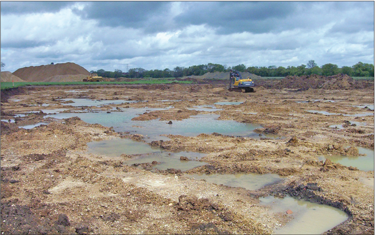
Plate 1: Ground conditions once machining had been stopped in the cemetery area
