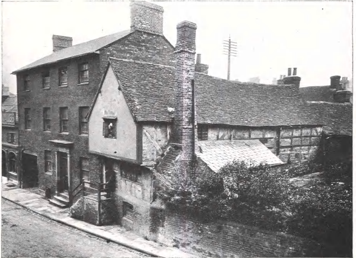
Plate 5 Demolished Timber-Framed Building, formerly in Upper George Street, Luton (after W. Austin History of Luton ).
