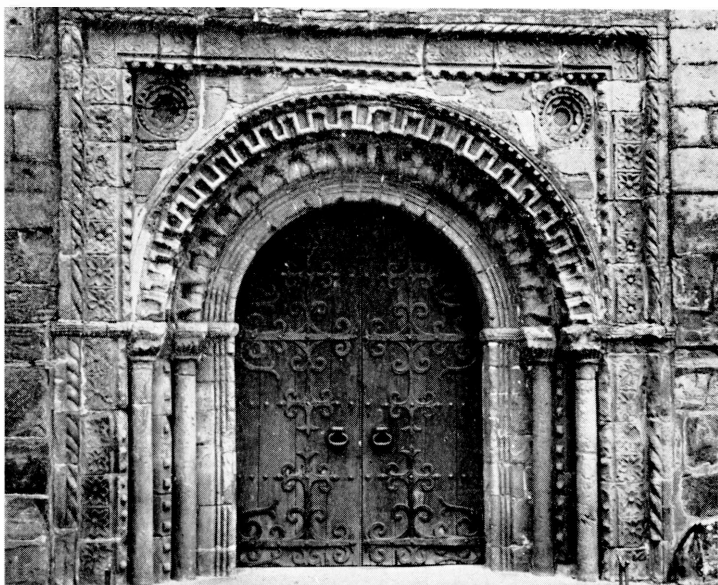
PLATE 1b—KENILWORTH (WARWICKS.) ST. NICHOLAS W. DOORWAY
