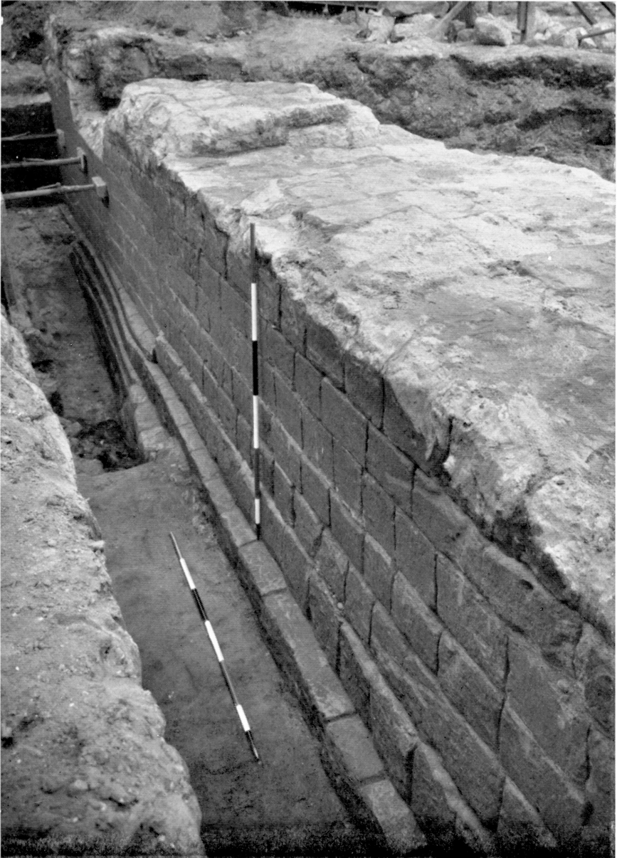
PLATE 1 View of wall looking east, showing front face
