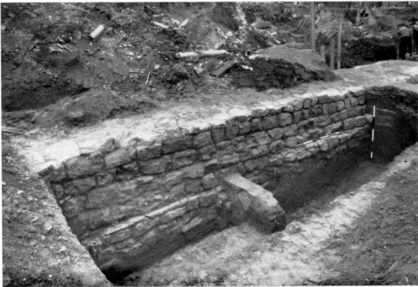
PLATE 4(b) Rear of wall south of AB, showing stepped construction trenches
