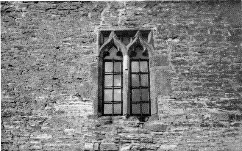
PLATE 2b Window in south-east wall of tower house
