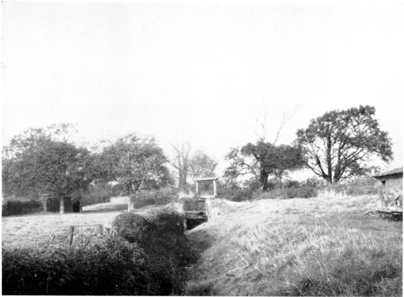
PLATE 2(b) Looking upstream from the Mill. The by-pass leat and sluice are in the centre and the main mill stream bank can be seen running to the right
