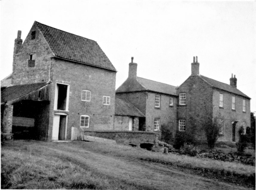
PLATE 1(a) The Mill and the farmhouse from the ford downstream. The 1816 extension to the house forms the main frontage
