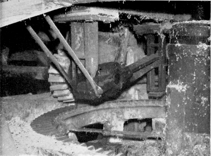
PLATE 3(b) The face-gear wheel and pinion drive to the dressing machine
