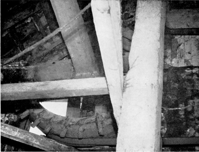
PLATE 4(a) The upper driving wheel to the sack hoist mounted on the gable end of the mill.
