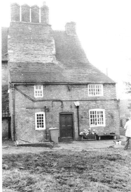
PLATE 4 Chimney stack and rear extension.
