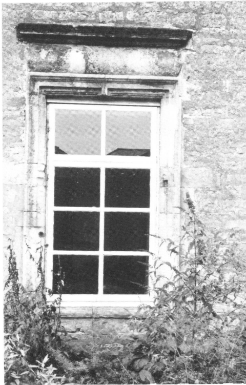
PLATE 5 Former doorway, now window.
