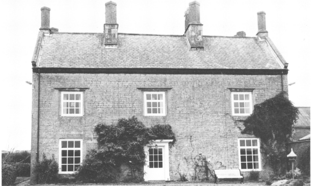
PLATE 2 South front of Manor Farm.
